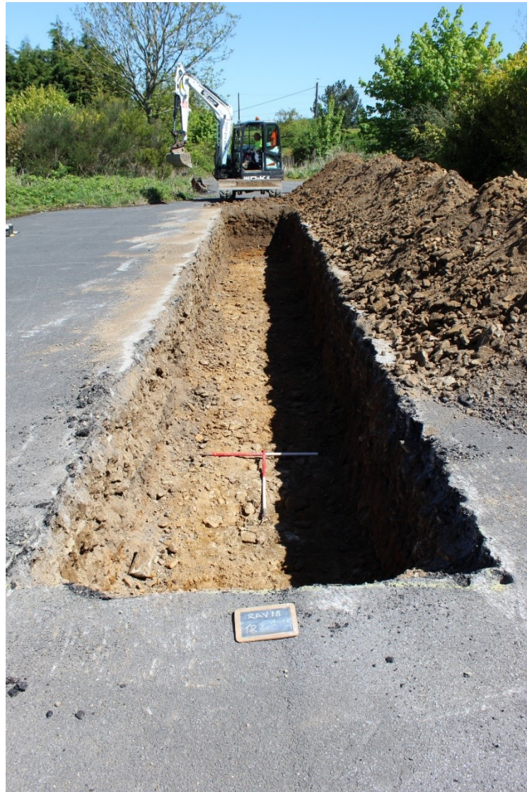
Figure 6 Trench 2, facing east. Scale 2x1 m
