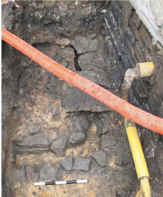
Figure 5 Culvert/ drain (011), looking east. Note north wall of outshot to right. Scale 1x50 cm
