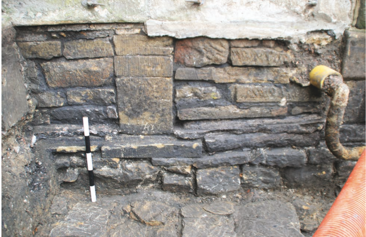
Figure 2 North elevation of outshot at west side of Heworth Hall after ground reduction. Scale 1x25cm
