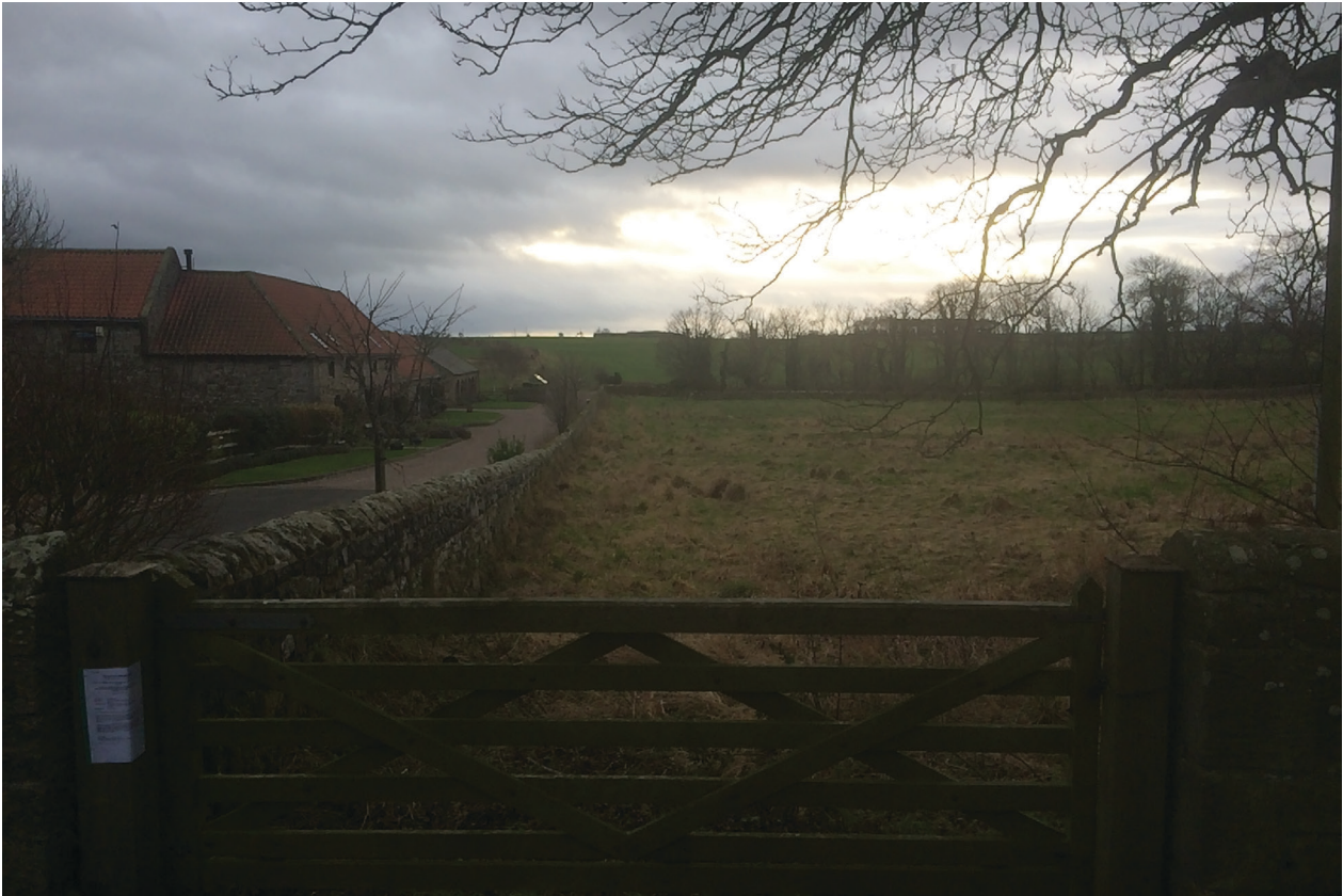
Fig. 5 View south across the proposed development area showing the proximity of the Listed Friary Farm buildings and their current 'open' setting at the western edge of the village
