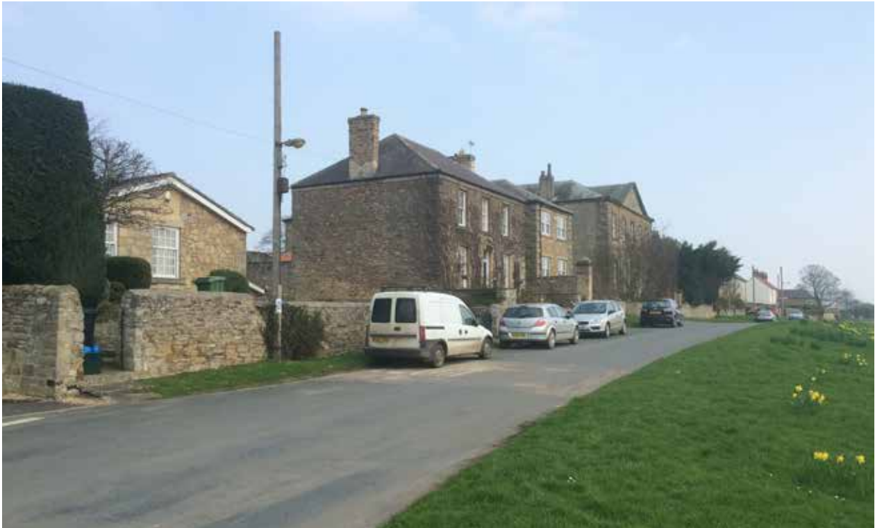
Figure 8 Looking south-east along the prominent row of houses with a varied architectural style (the Old Hall is masked by the overgrown evergreen hedge). A bungalow in the foreground is late 20th century in date and is noticeably at stylistic odds with the 18th-19th century character of the historic buildings
