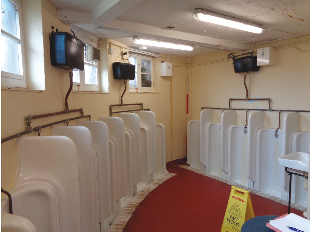
Figure 13 Room G1, detail of urinals, facing north-east. Scale 1x2m
