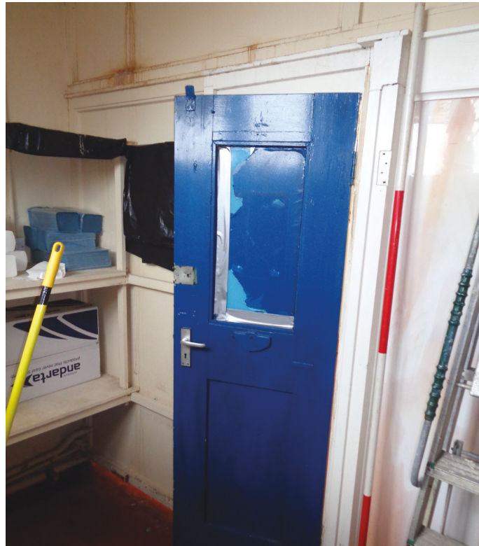
Figure 17 Room G2, facing south-west. Note location of previous hinges to right of current door. Scale 1x2m
