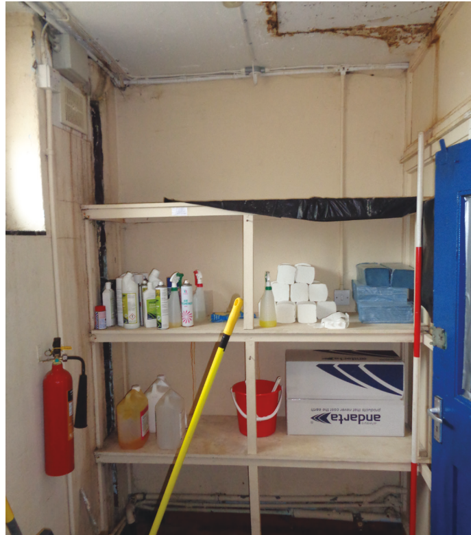
Figure 16 Room G2, facing south-east. Scale 1x2m
