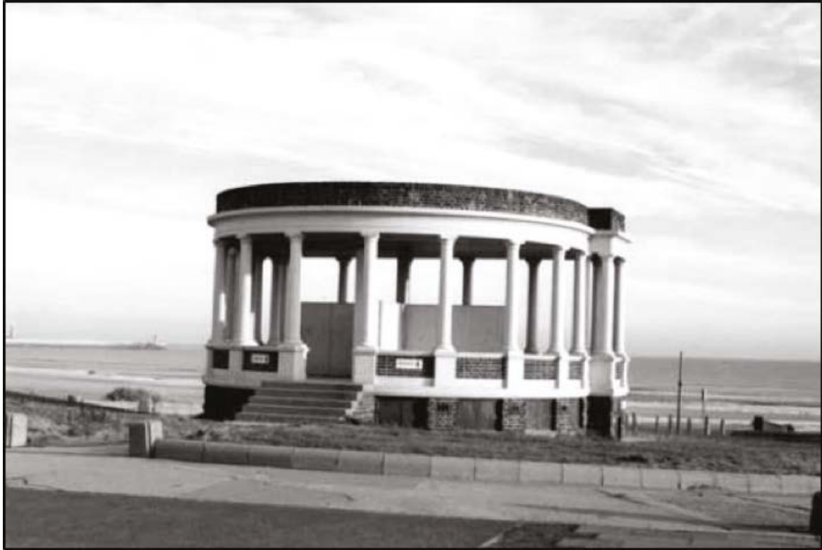
Figure 4 Photograph taken in 1982, showing internal T-shaped partitions for seating still in place. (South Tyneside Libraries)
