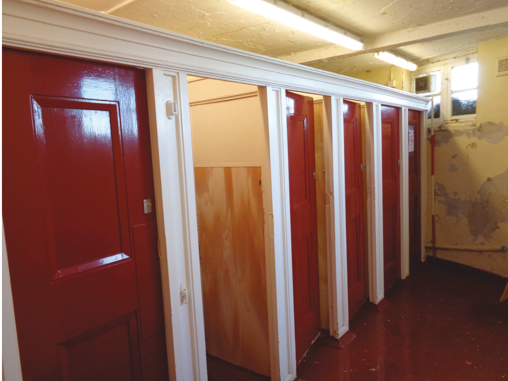
Figure 19 W.C. stalls within Room G3, facing south-west. Scale 1x2m
