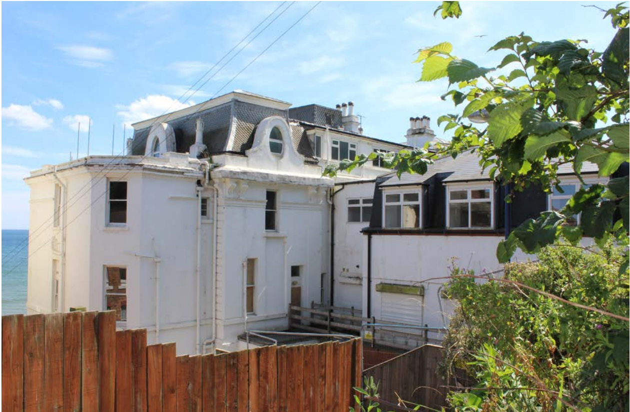
Figure 7 View across rear of property from public footpath, facing south-east
