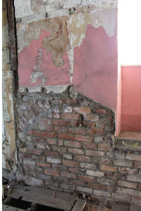
Figure 16 Remnant of former round-headed window opening, now blocked
