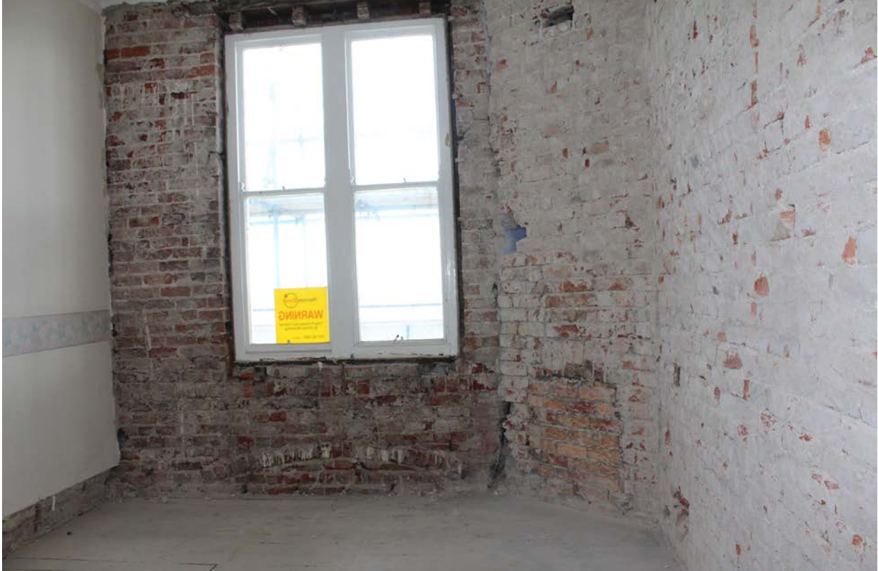
Figure 12 Later inserted fireplace, now blocked
