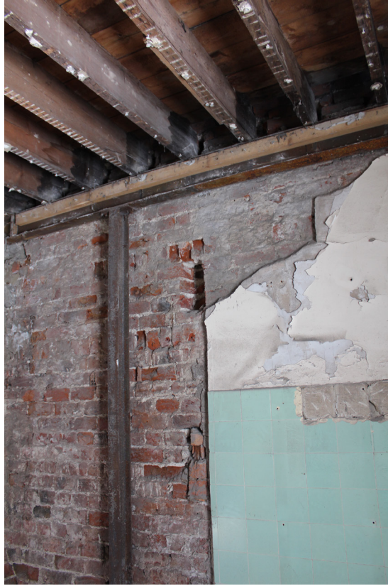
Figure 21 Reinforced timber beams
