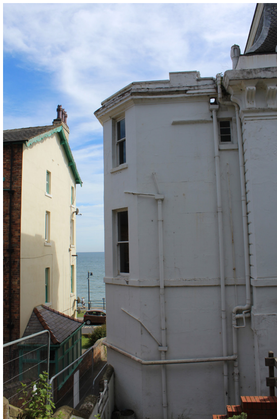
Figure 8 North extension, facing east
