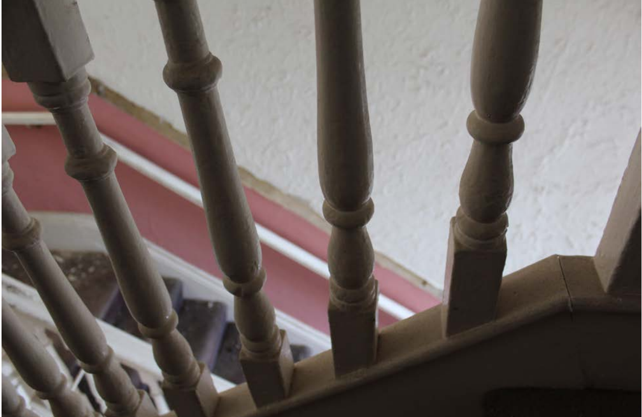
Figure 17 Example of alterations to spindle alignment
