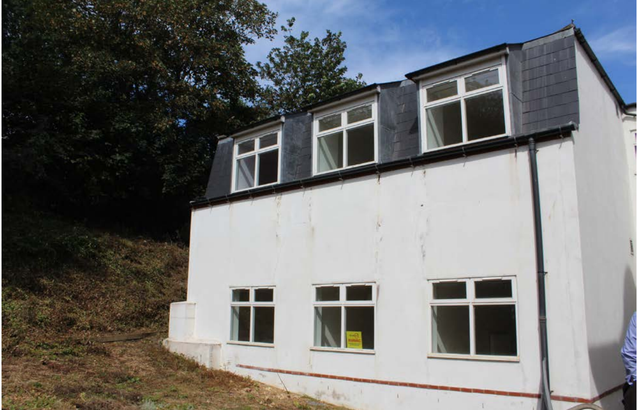
Figure 5 Rear extension, facing north-west
