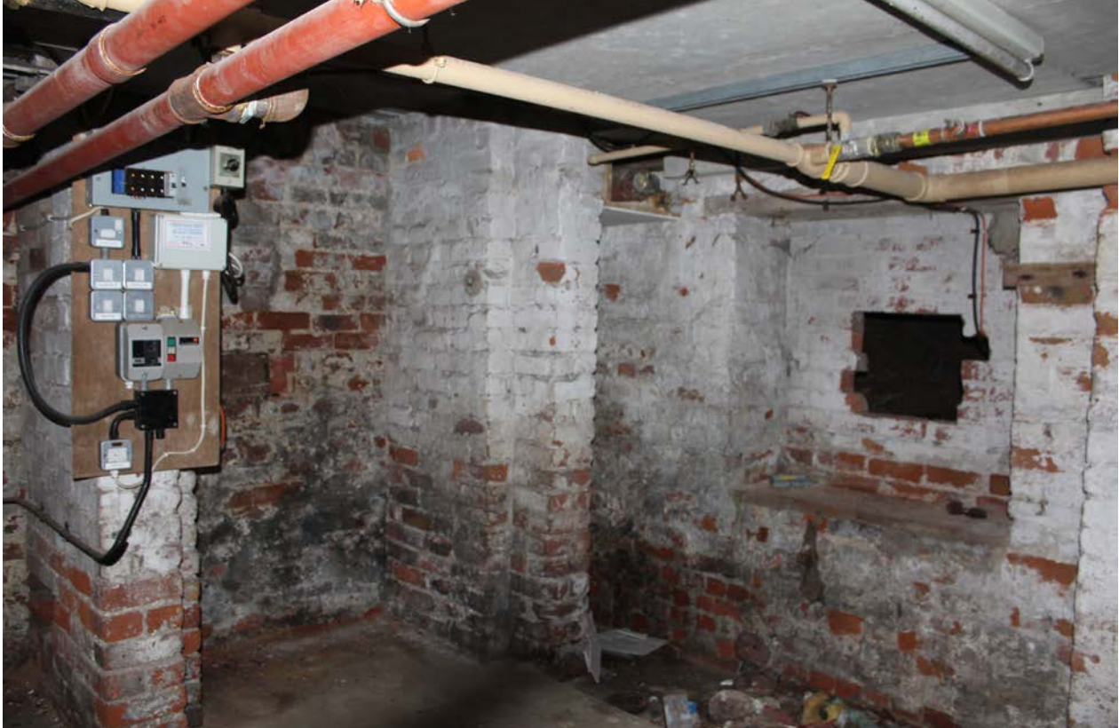
Figure 20 Interior of basement
