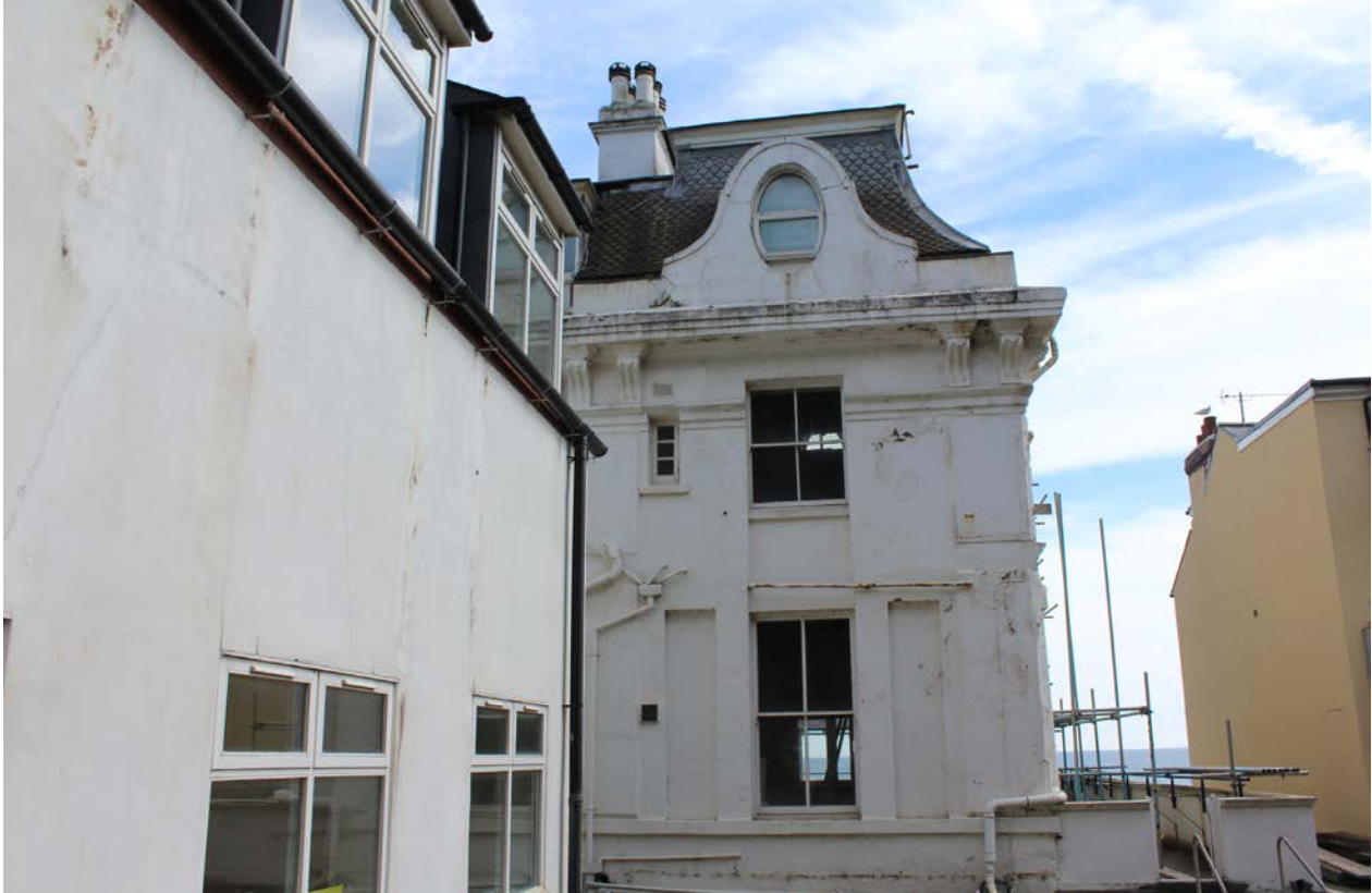
Figure 6 Southern extent of western elevation, facing east
