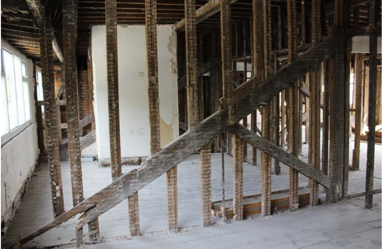
Figure 22 Raised roof timbers on third floor
