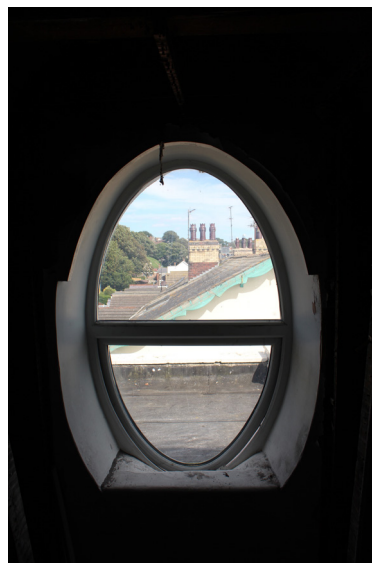
Figure 25 Third-floor oval window, facing onto existing flat roof
