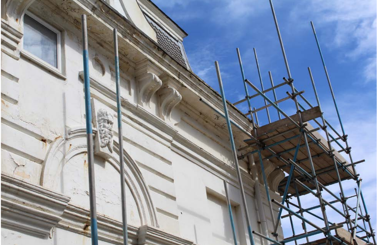
Figure 10 Decorative arch formed from earlier blocked window and other features on southern elevation
