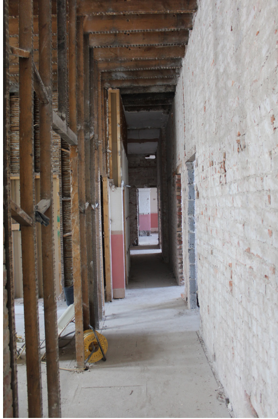
Figure 11 Central hallway, aligned north to south
