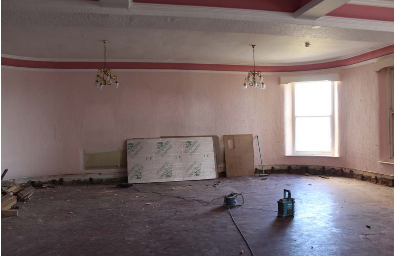
Figure 14 Interior of northern extension
