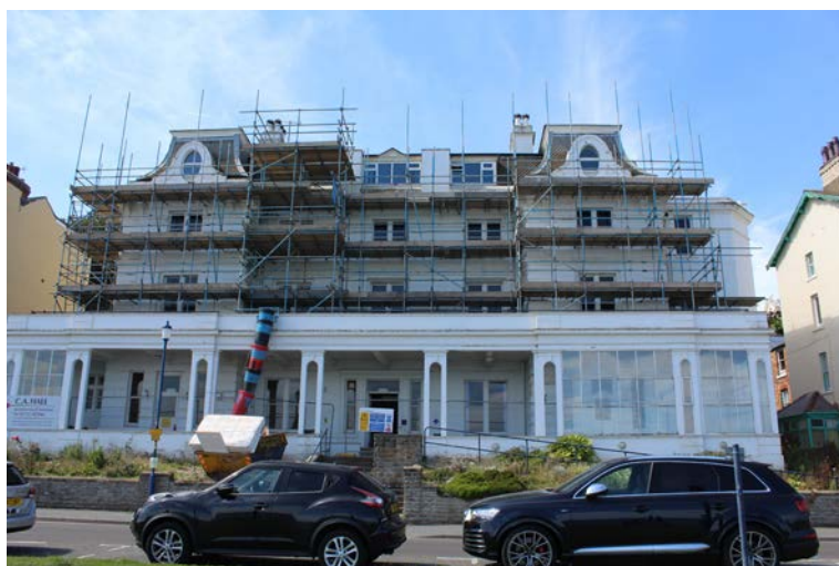
Figure 2 Principal eastern façade facing west
