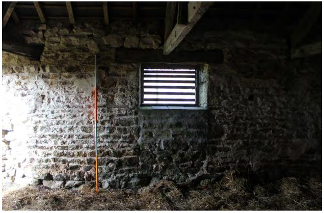
Figure 12 Blocked doorway in west wall of Room G2. Scale 1 x 2 m
