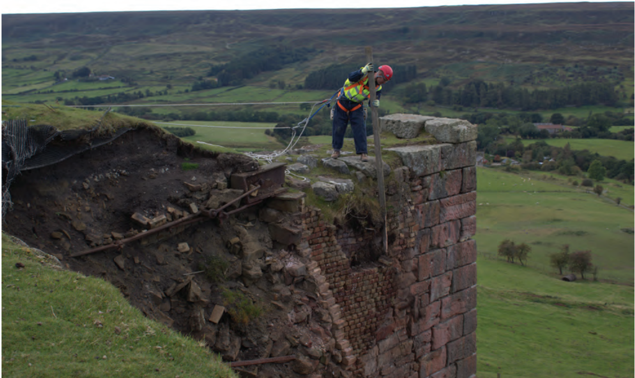
Figure 11 Work underway on the north side of Pier 3, looking south-west
