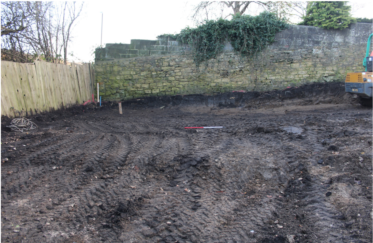
Figure 3 Eastern boundary wall, facing east. Scale 1 x 1 m.
