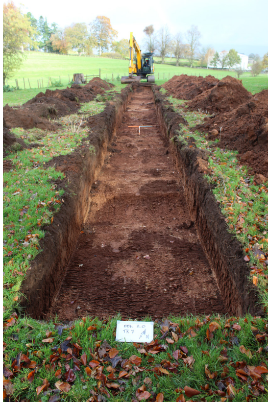
Figure 15 Trench 7, facing north. Scale 1 x 1 m, 1 x 2 m
