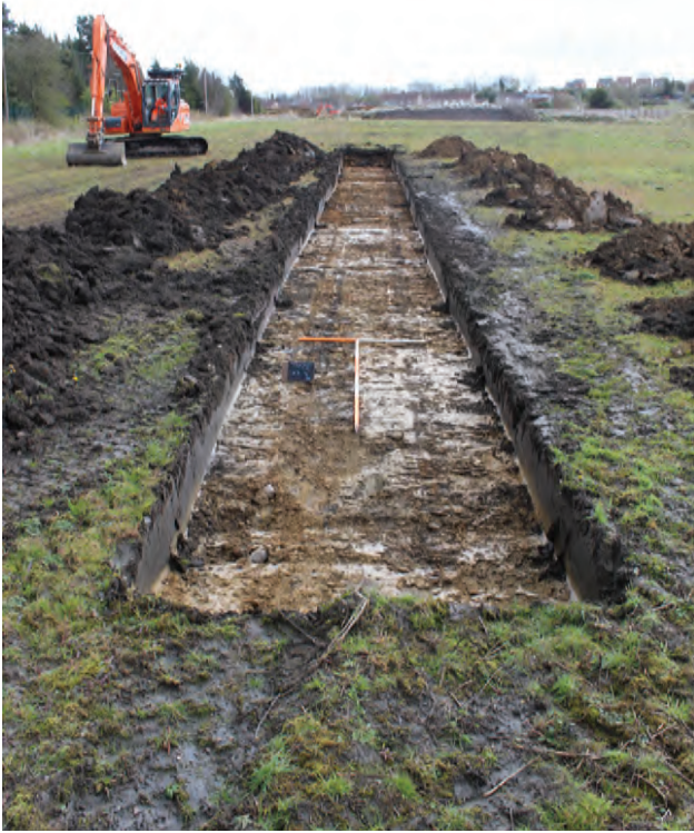
Figure 7 Trench 3, facing north-east. Scale 1x1 m, 1x2 m
