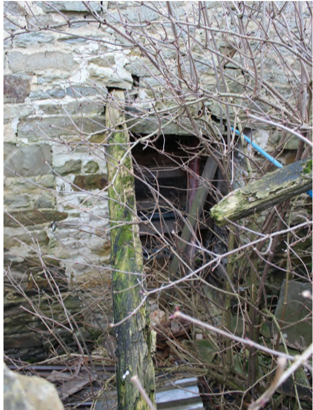
Figure 16 East wall of Room LG2, facing south-east. No scale
