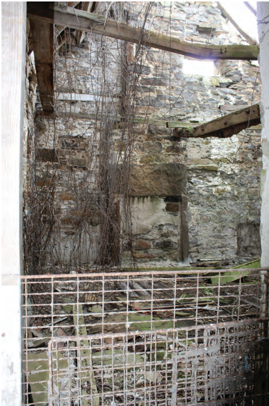
Figure 31 South wall of Room F1, facing south. No scale
