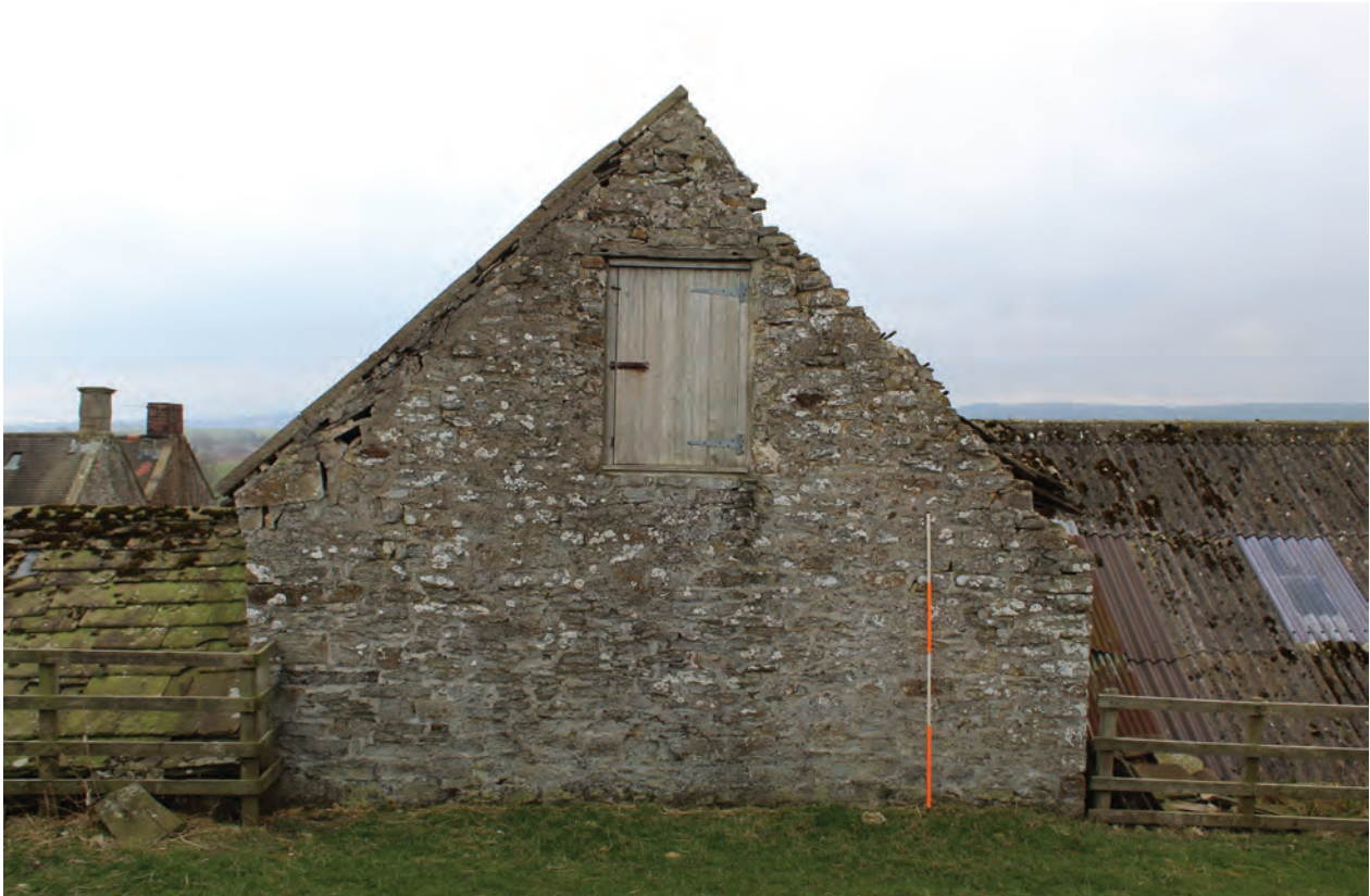
Figure 7 North-facing gable elevation, facing south. Scale 1x2 m
