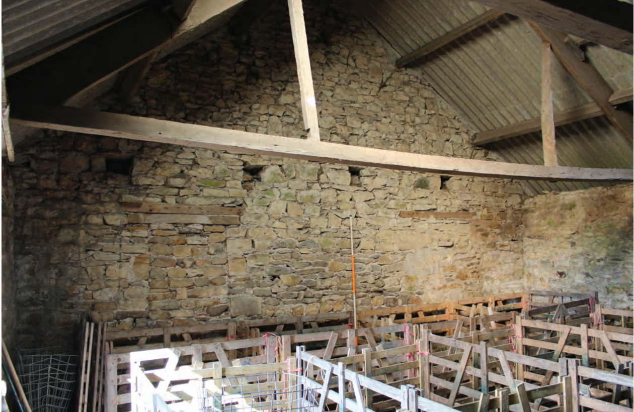
Figure 18 Room G1, west wall, facing north-west. Scale 1x2 m
