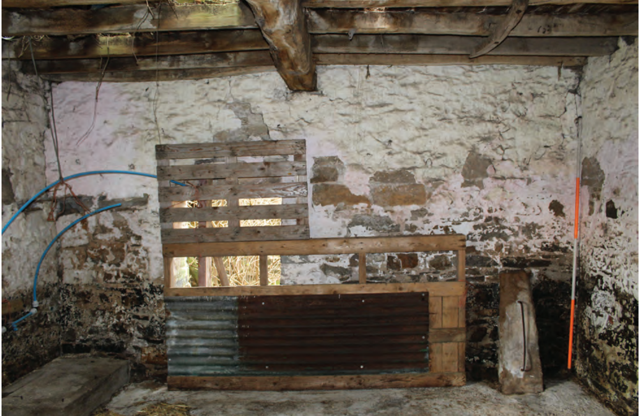
Figure 14 West wall of Room LG1, facing west. Scale 1x2 m
