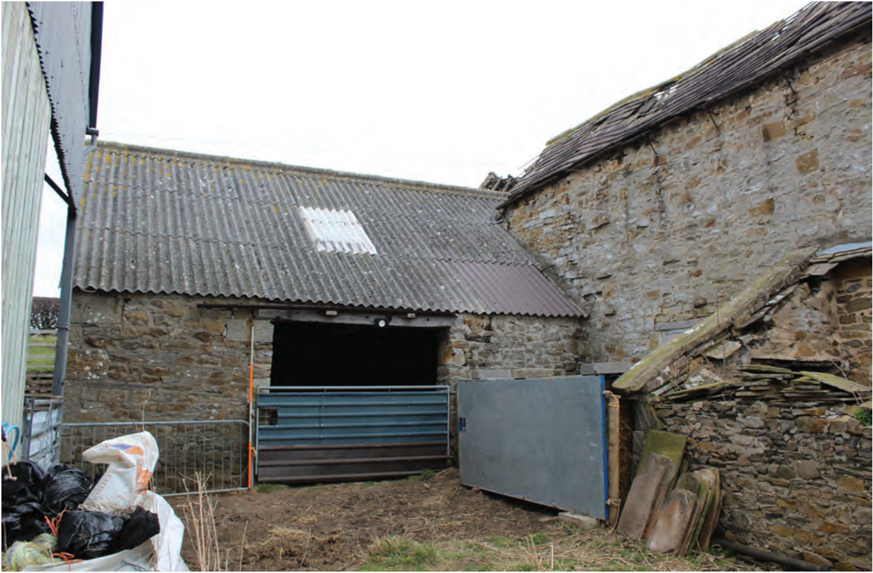
Figure 5 South elevation of wheelhouse, facing north-east. Scale 1x2 m
