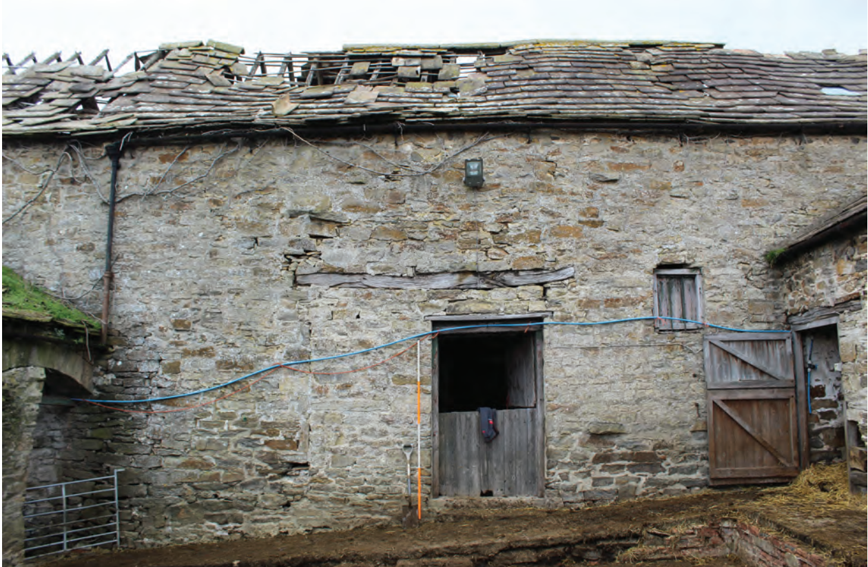
Figure 9 Detail of centre of east-facing elevation. Scale 1x2 m
