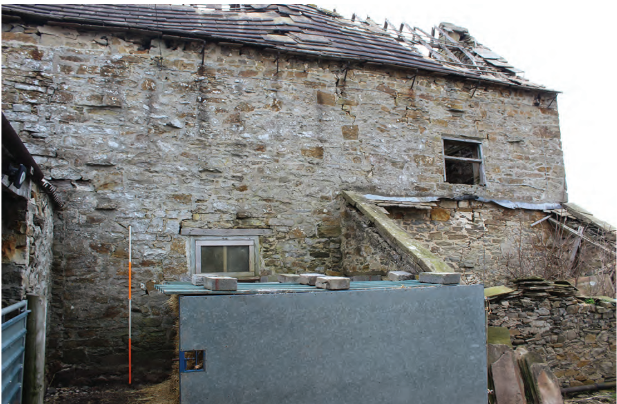
Figure 4 Central section of west-facing elevation, facing south-east. Scale 1x2 m
