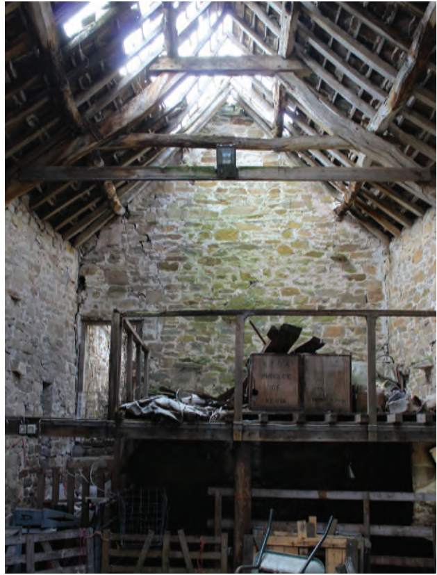
Figure 22 South wall of Room G2, facing south. No scale
