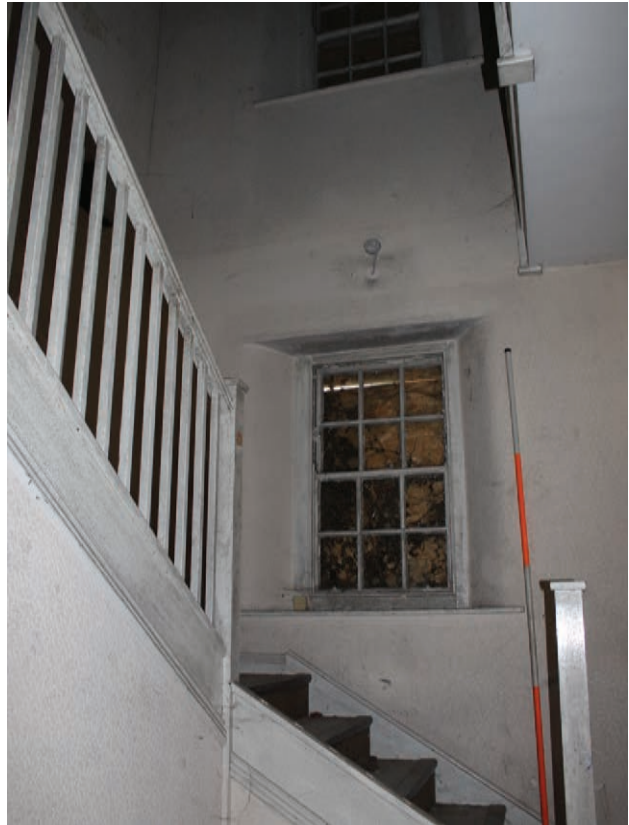
Figure 60 South wall of Room G41, facing south. Scale 1x2 m
