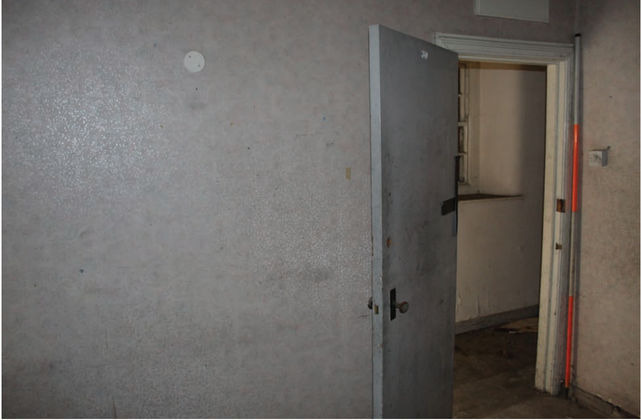
Figure 51 North wall of Room G38, facing north-east. Scale 1x2 m
