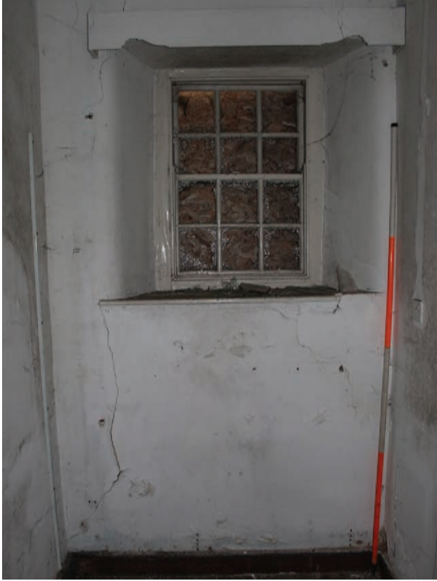
Figure 48 Room G34, facing west. Scale 1x2 m
