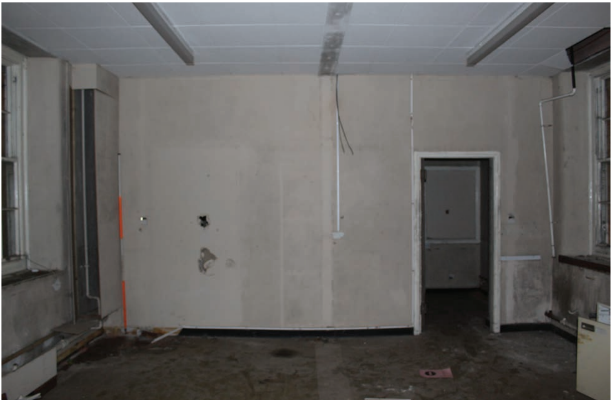
Figure 217 East wall of Room G4, facing east. Scale 1x2 m
