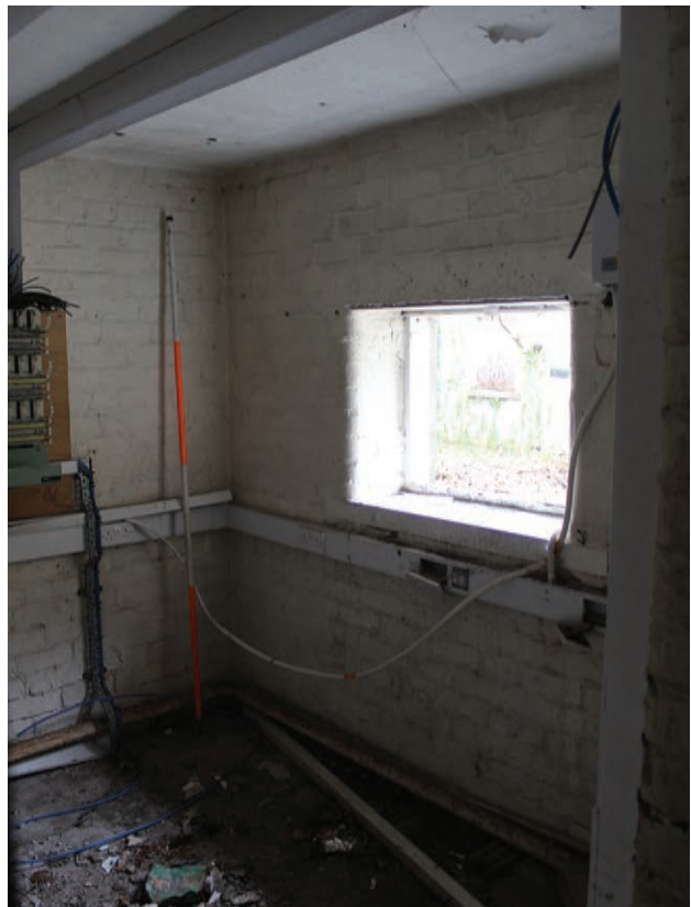
Figure 146 Room G23, facing south-west. Scale 1x2 m
