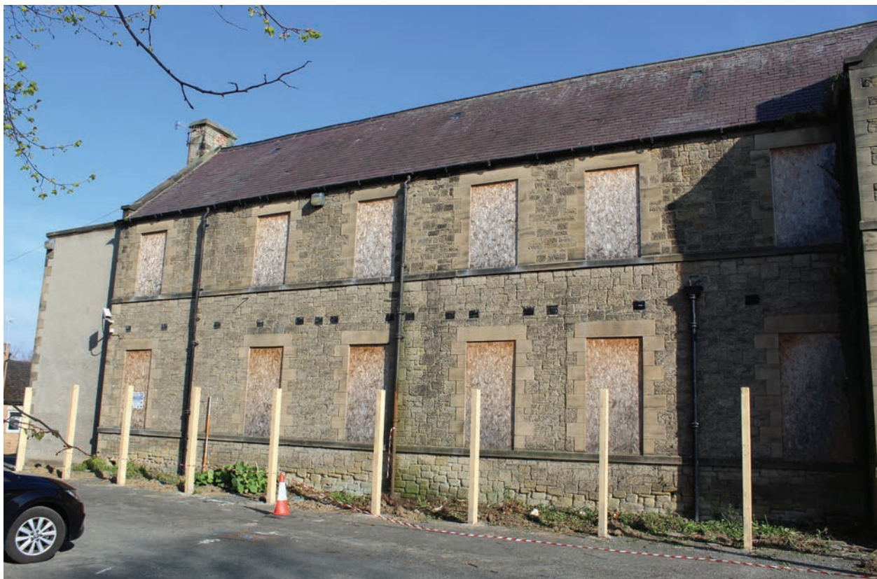
Figure 8 Western end of south elevation of Building A, facing north. Scale 1x2 m
