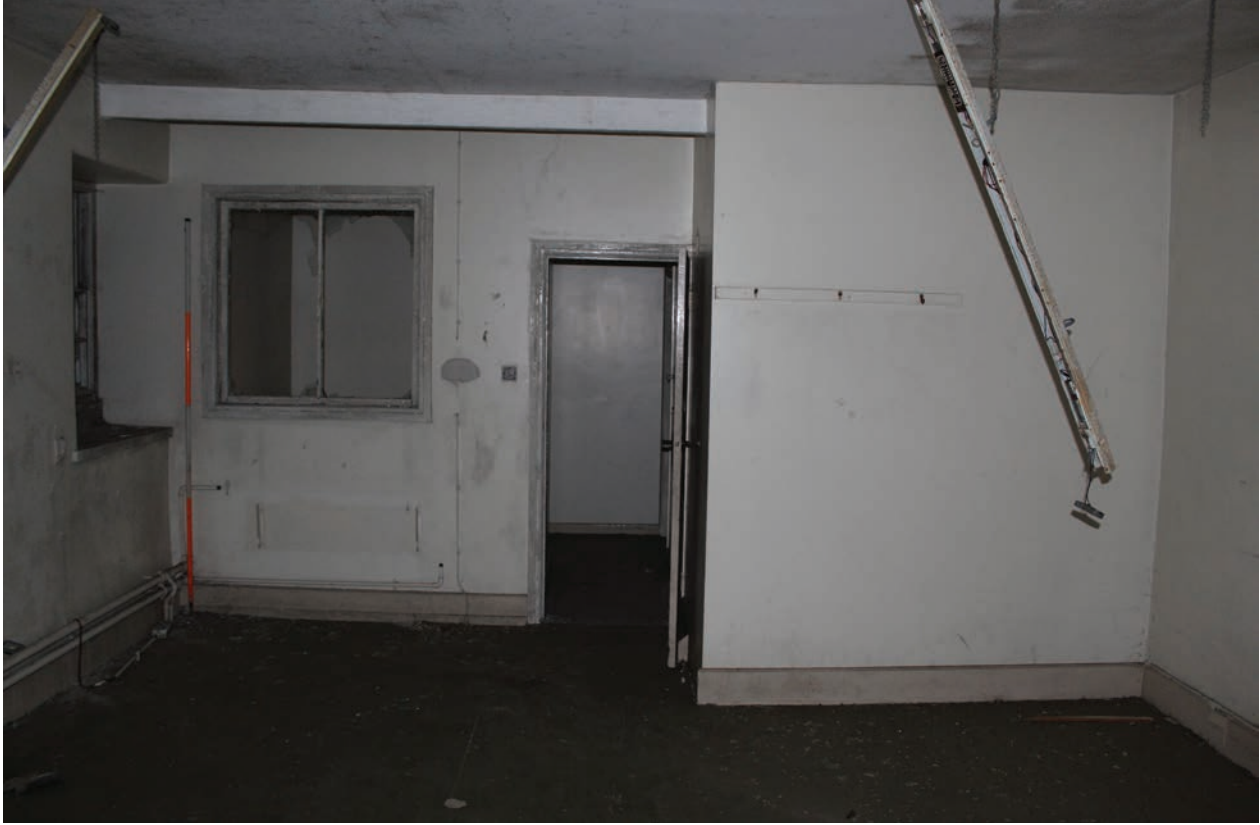
Figure 168 Room F10, facing east. Scale 1x2 m
