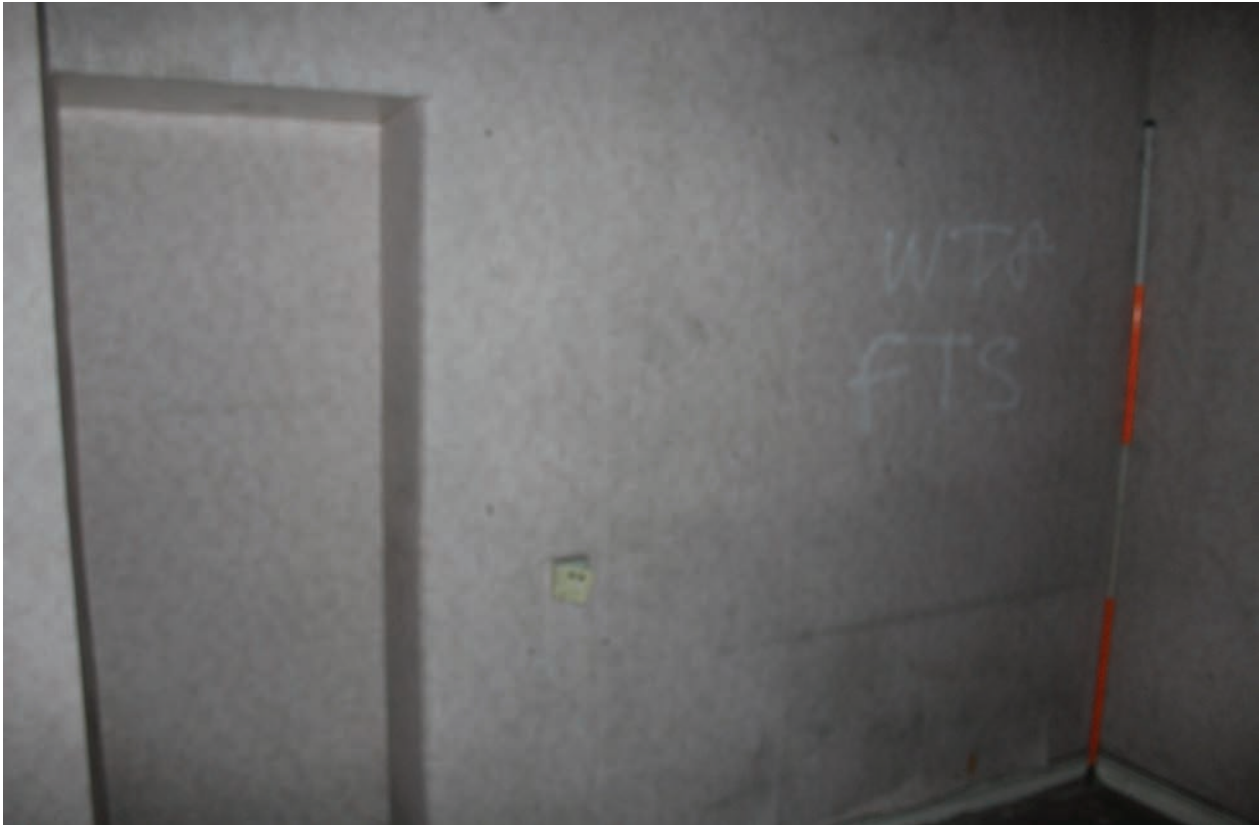
Figure 75 West wall of Room F24, facing north-west. Scale 1x2 m
