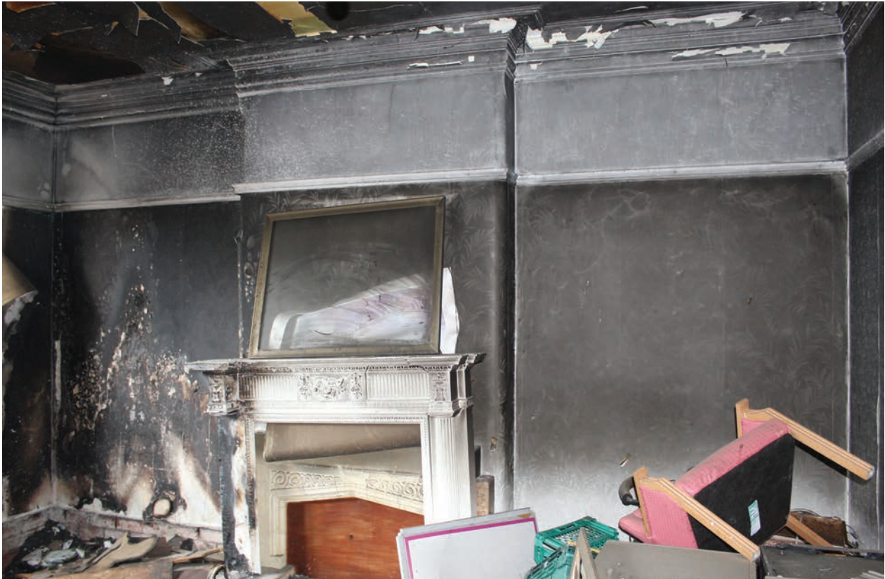
Figure 114 North wall of Room G1, facing north. No scale
