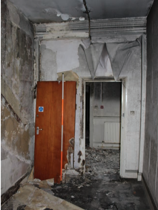
Figure 116 Room G2, looking south. Scale 1x2 m
