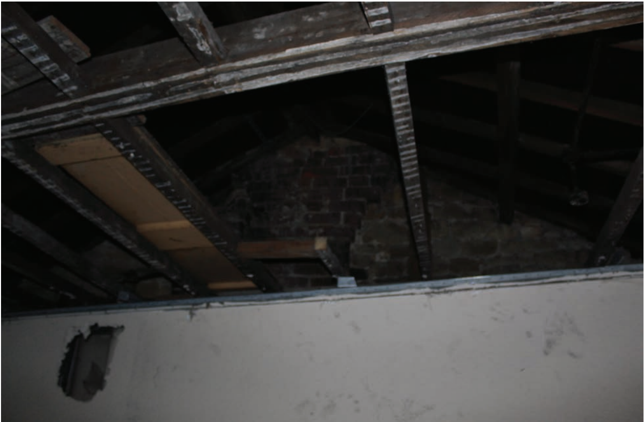
Figure 64 East gable wall of Room F37, facing east
