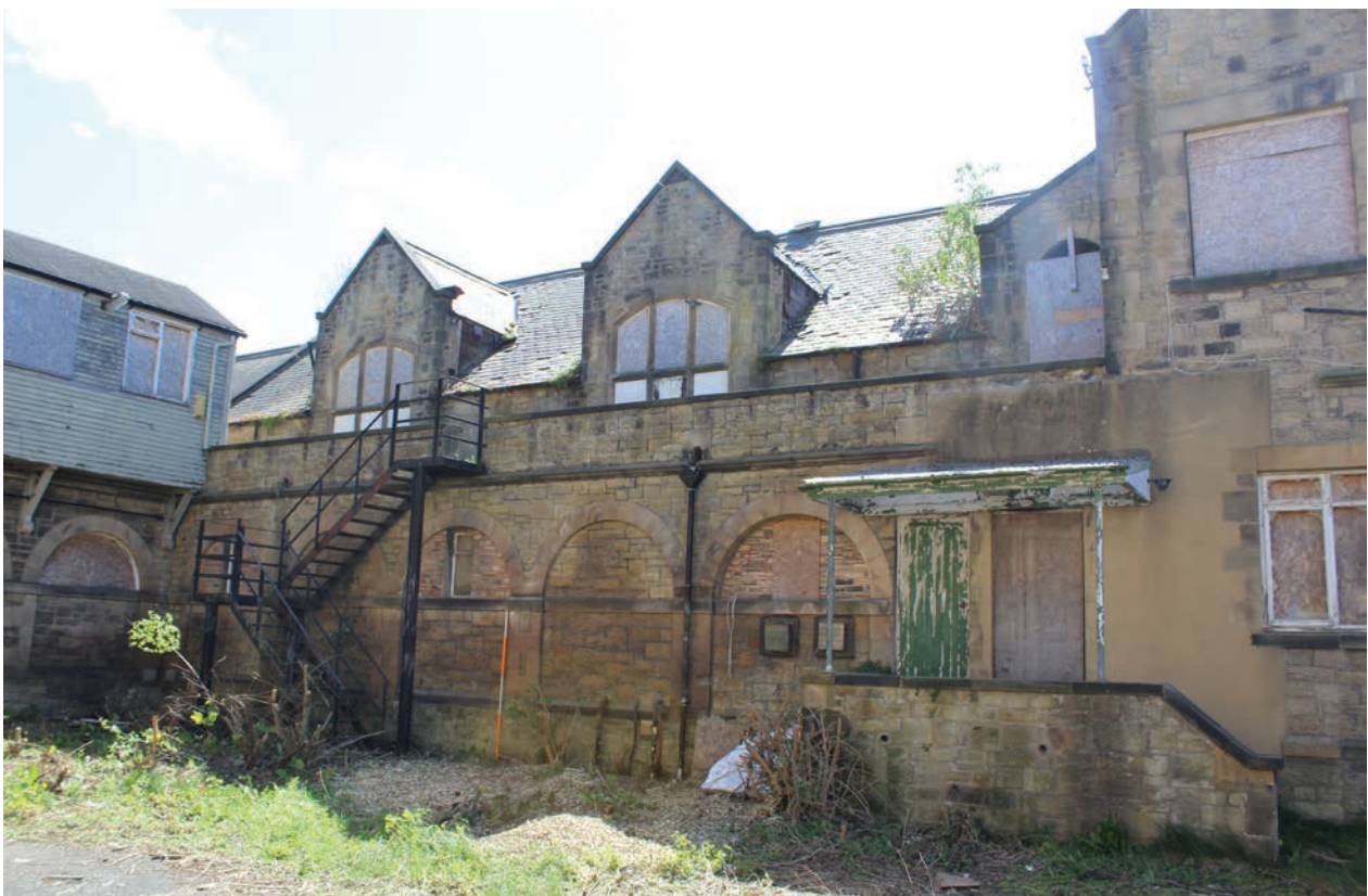
Figure 109 North elevation of the dining hall in Building B, facing south-east. Scale 1x2 m
