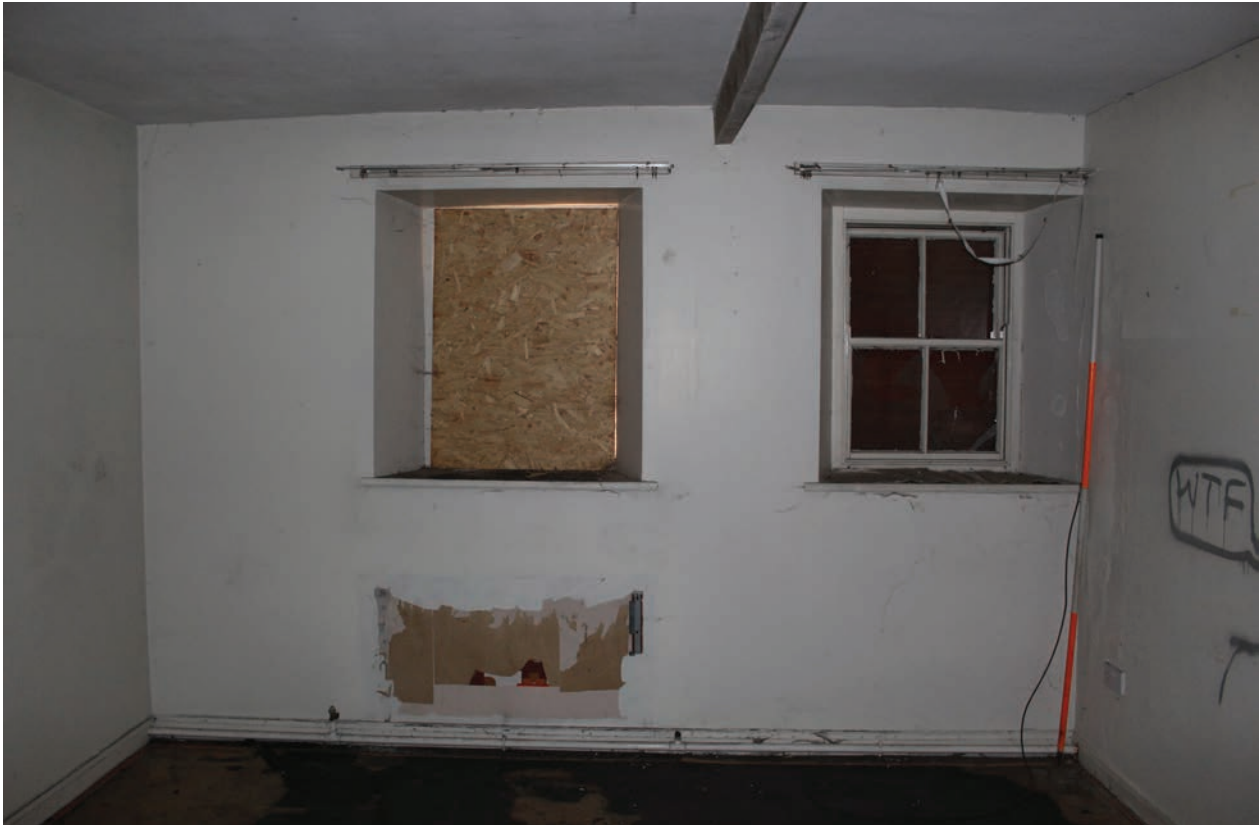
Figure 173 South wall of Room F16, facing south. Scale 1x2 m
