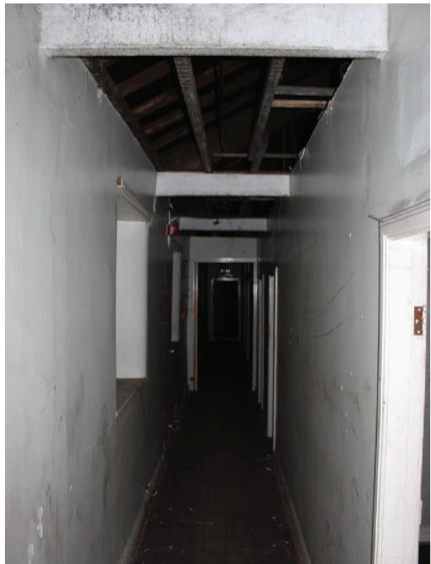
Figure 73 Room F18, facing east. Scale 1x2 m
