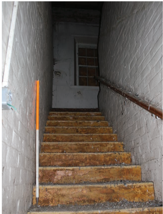
Figure 221 Looking south-west up the stairwell in Room G12. Scale 1 x 1 m
