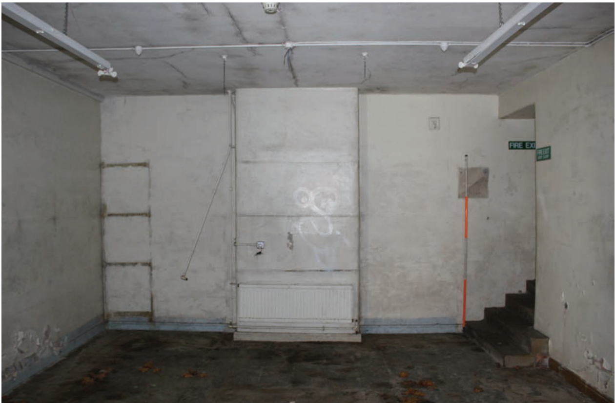
Figure 148 Room G24, facing west. Scale 1x2 m
