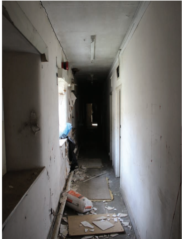
Figure 39 Room G27, facing east. Scale 1x2 m
