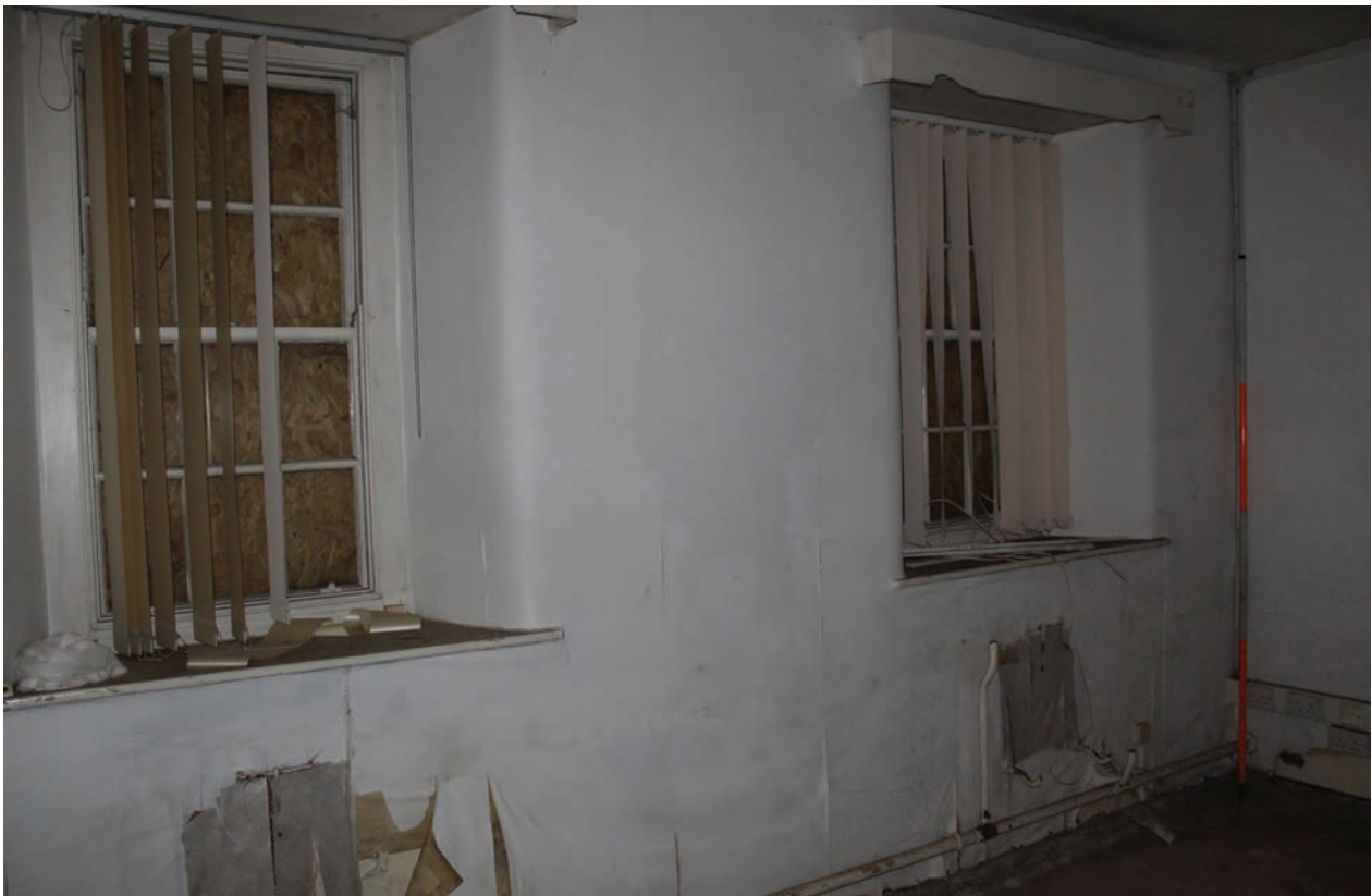
Figure 47 South wall of Room G33, facing south. Scale 1x2 m
