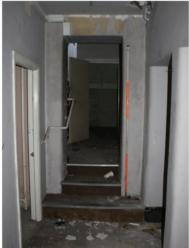
Figure 35 Room G22, facing west. Scale 1x2 m
