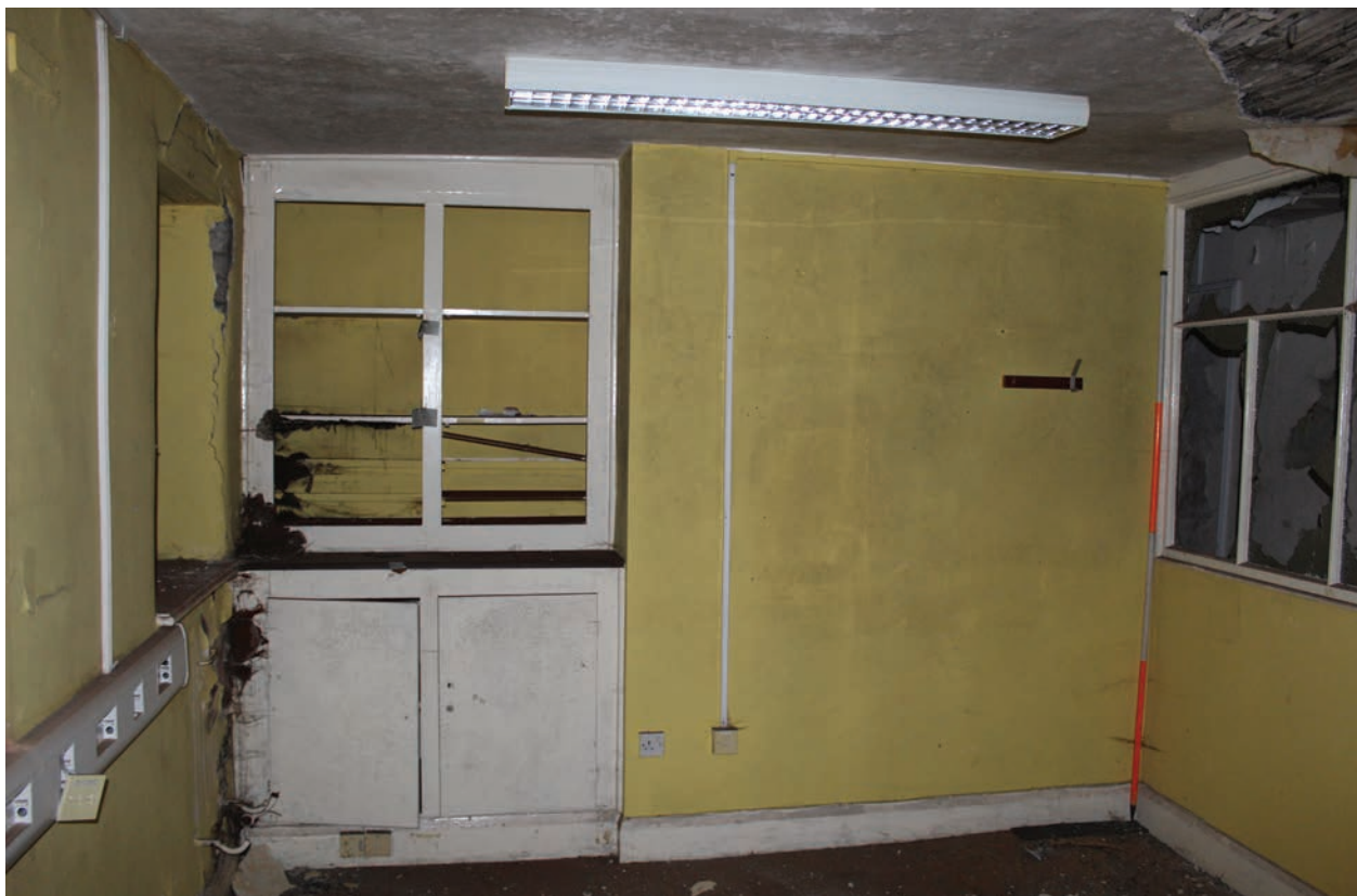
Figure 229 West wall of Room G20, facing west. Scale 1x2 m
