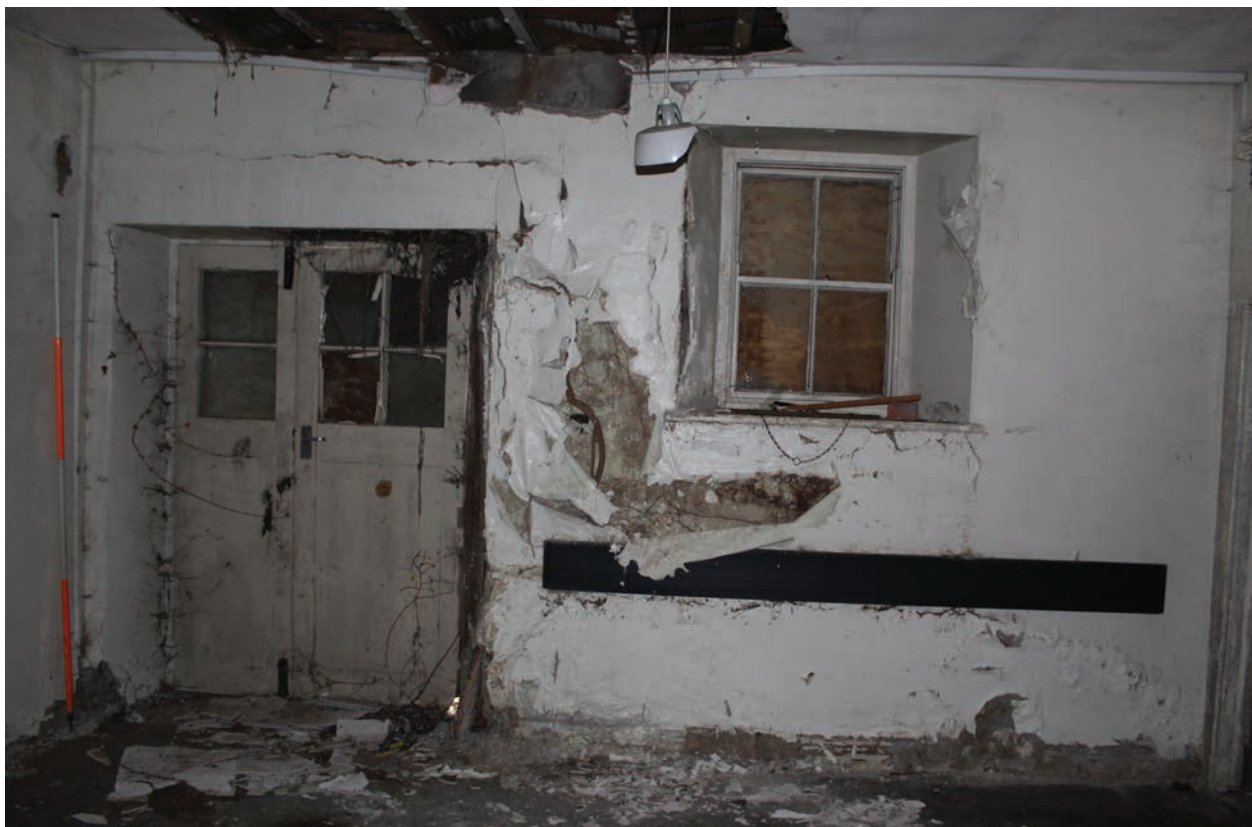
Figure 155 South wall of Room G30, facing south. Scale 1x2 m
