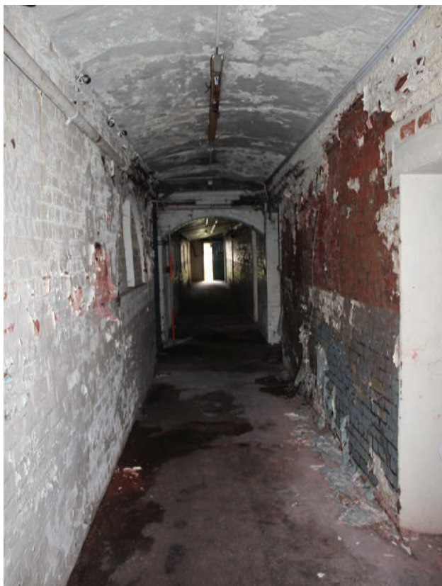
Figure 134 Corridor G12, facing east. Scale 1x2 m
