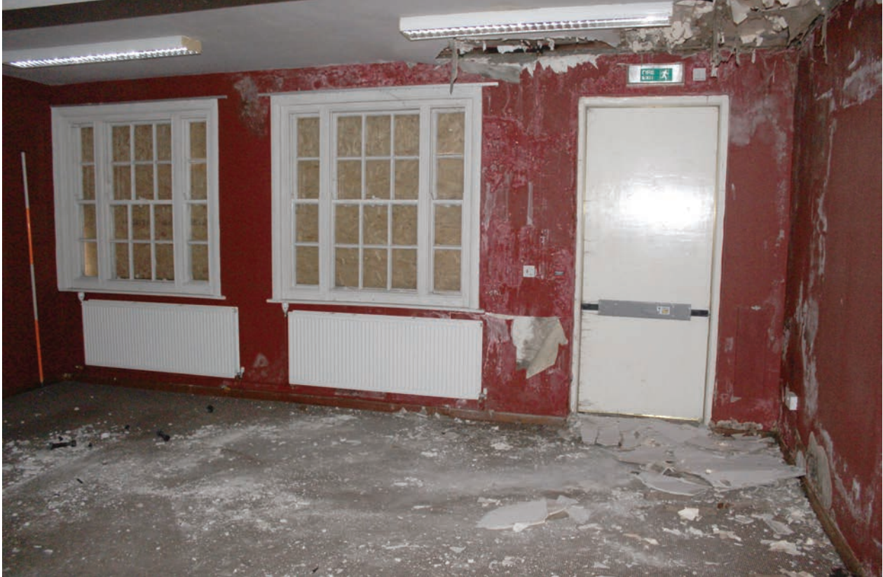
Figure 27 West wall of Room G13, facing west. Scale 1x2 m
