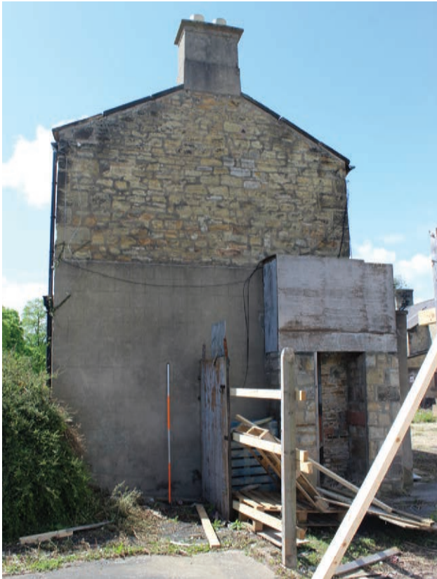
Figure 19 East elevation of Building A, facing west. Scale 1x2 m
