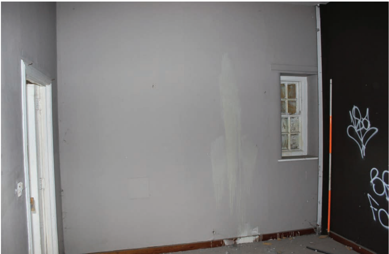
Figure 70 East wall of Room F13, facing south-east. Scale 1x2 m
