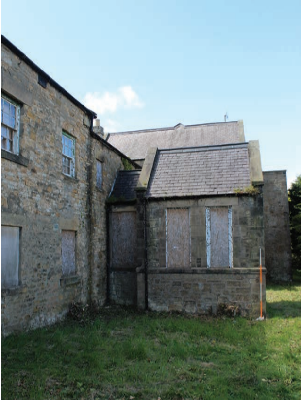
Figure 199 Eastern end of the north elevation of Building C, facing west. Scale 1x2 m
