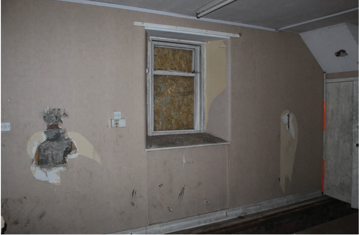
Figure 236 North wall of Room G24, facing north-east. Scale 1x2 m
