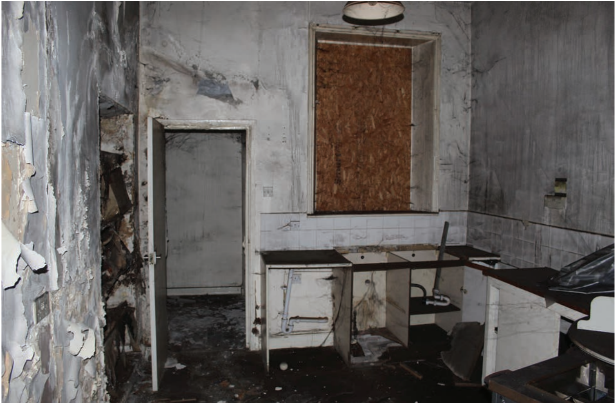
Figure 121 Room G7, looking south. No scale
