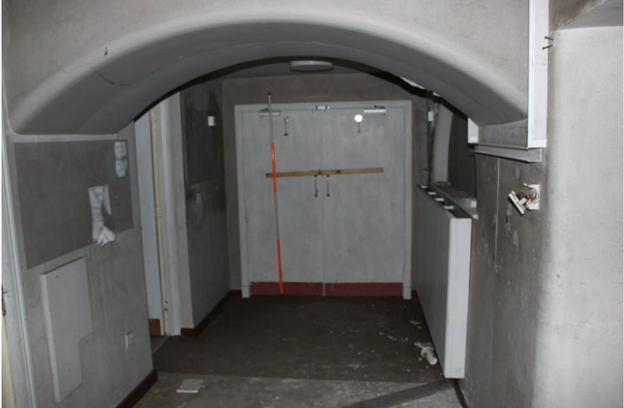
Figure 29 Room C16, facing north. Note blocked lunette window at right and supporting arch. Scale 1x2 m
