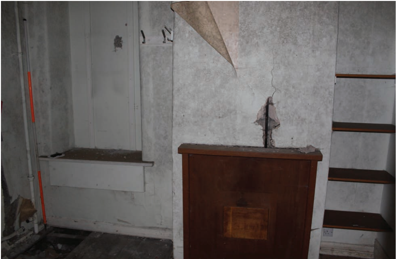
Figure 226 West wall of Room G16, facing south-west. Scale 1x2 m
