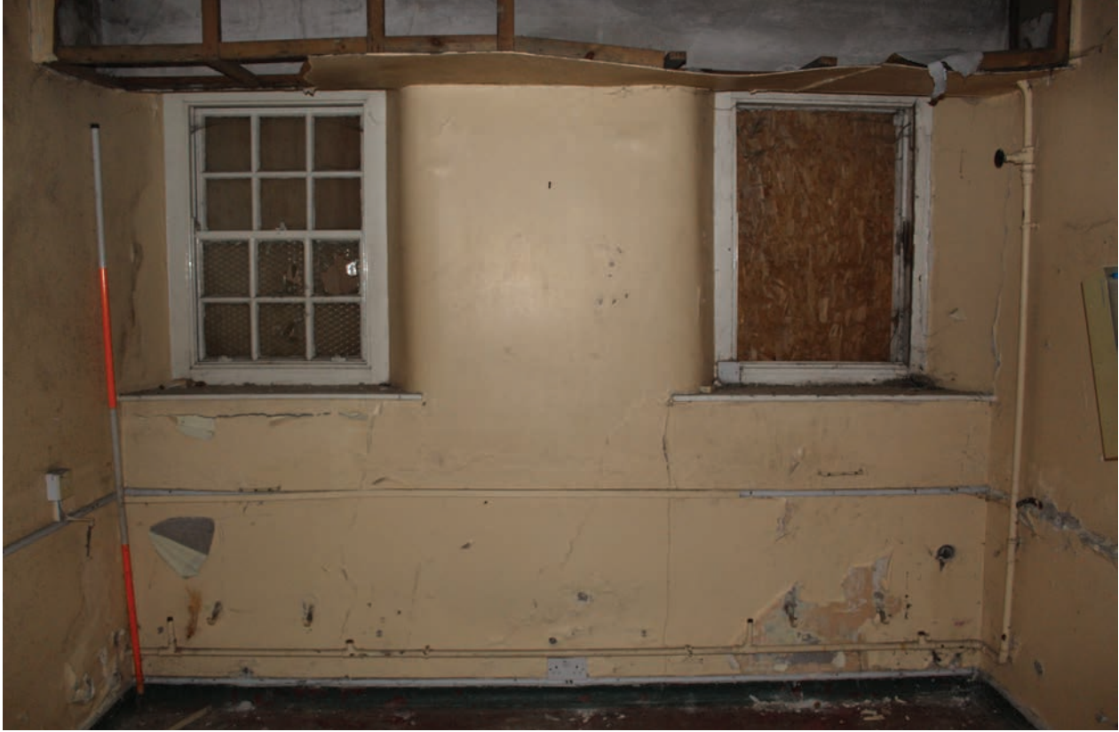
Figure 156 Room G36, looking east. Scale 1x2 m
