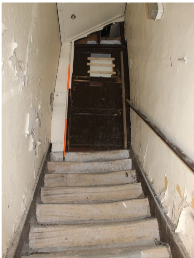
Figure 165 Room G46, facing north. Scale 1x2 m
