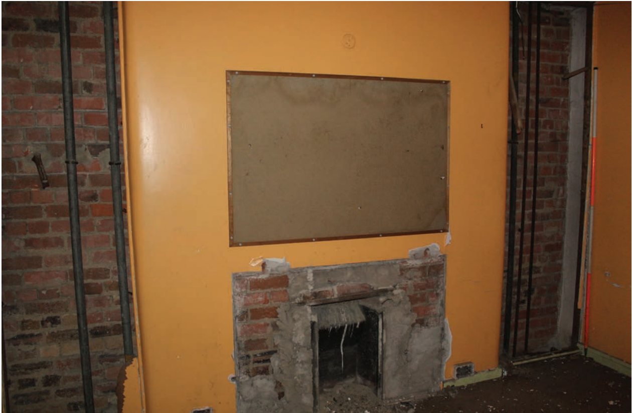
Figure 175 Room F19, looking north. Note brickwork construction. Scale 1x2 m
