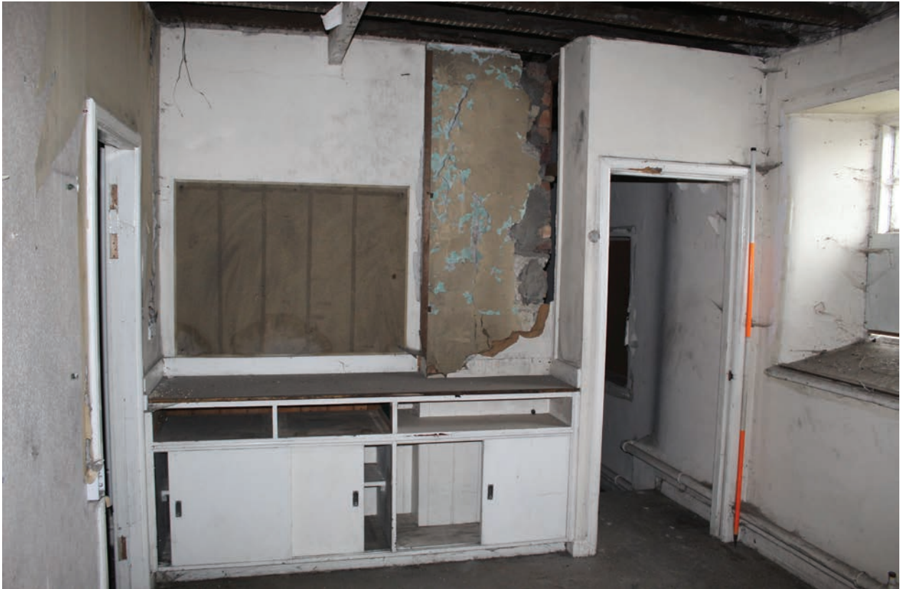
Figure 256 Room F20, facing west. Scale 1x2 m
