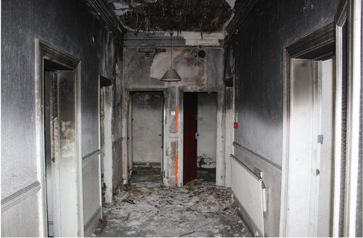
Figure 118 Room G3, facing east. Scale 1x2 m
