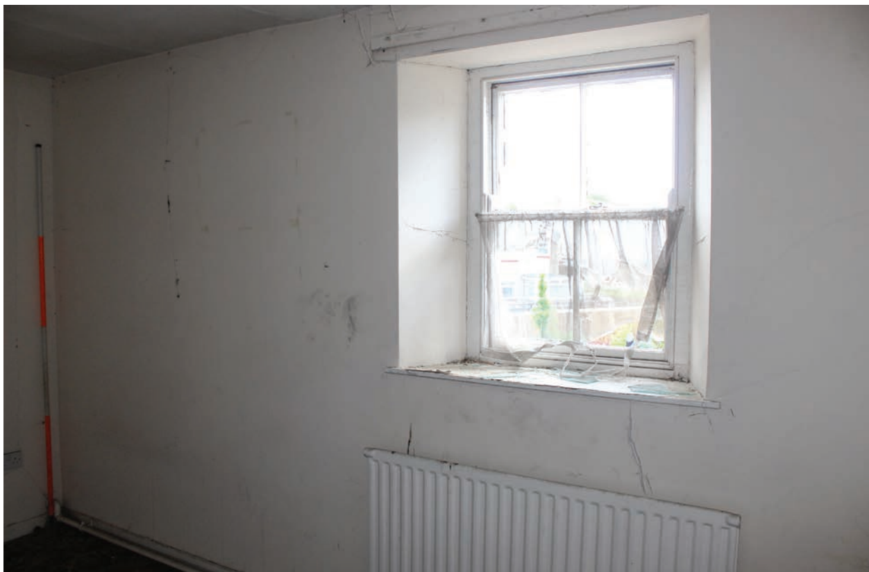
Figure 182 East wall of Room F25. Scale 1x2 m
