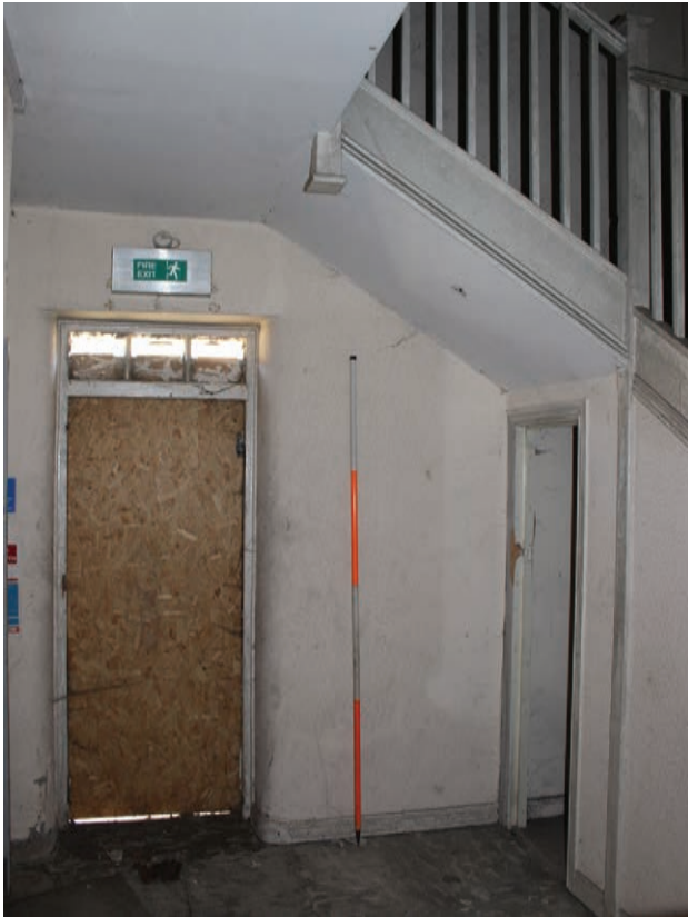
Figure 59 North wall of Room G41, facing north. Scale 1x2 m
