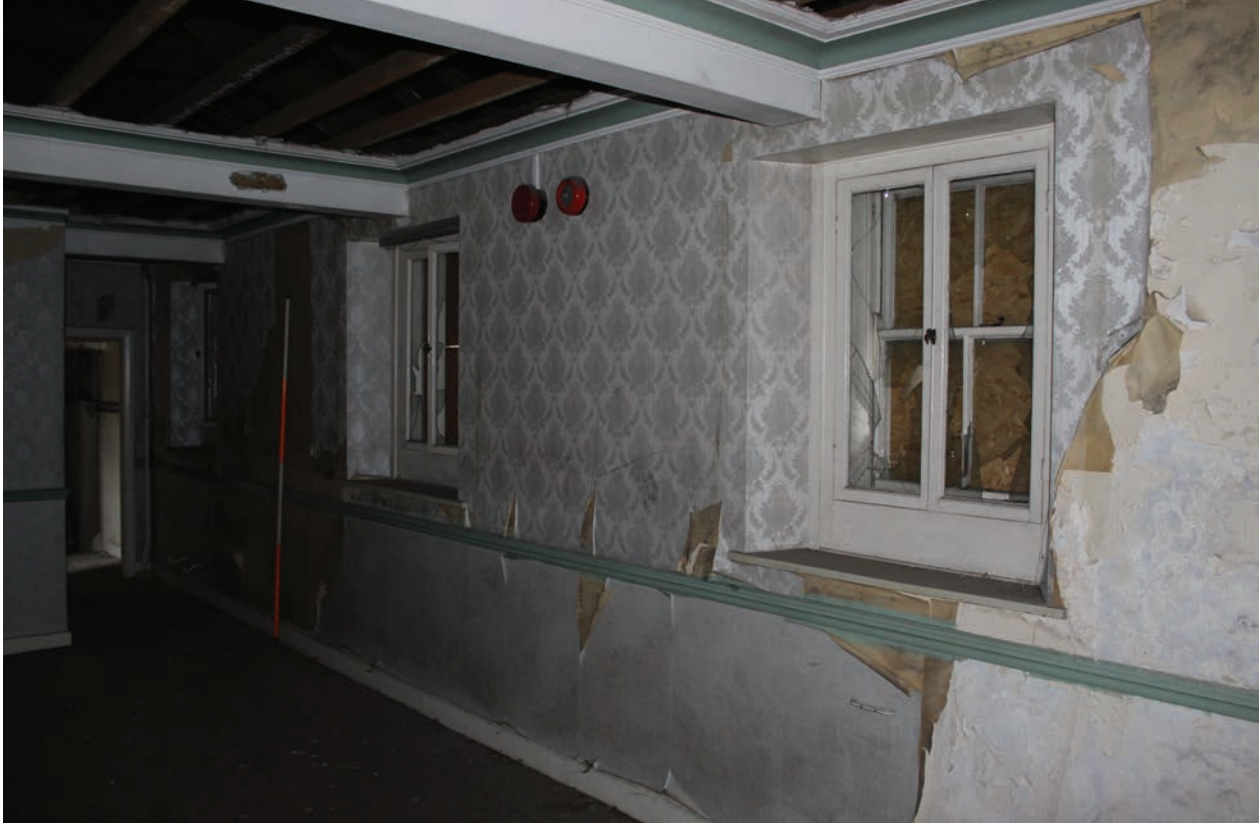
Figure 258 Room F22, facing north-west. Scale 1x2 m
