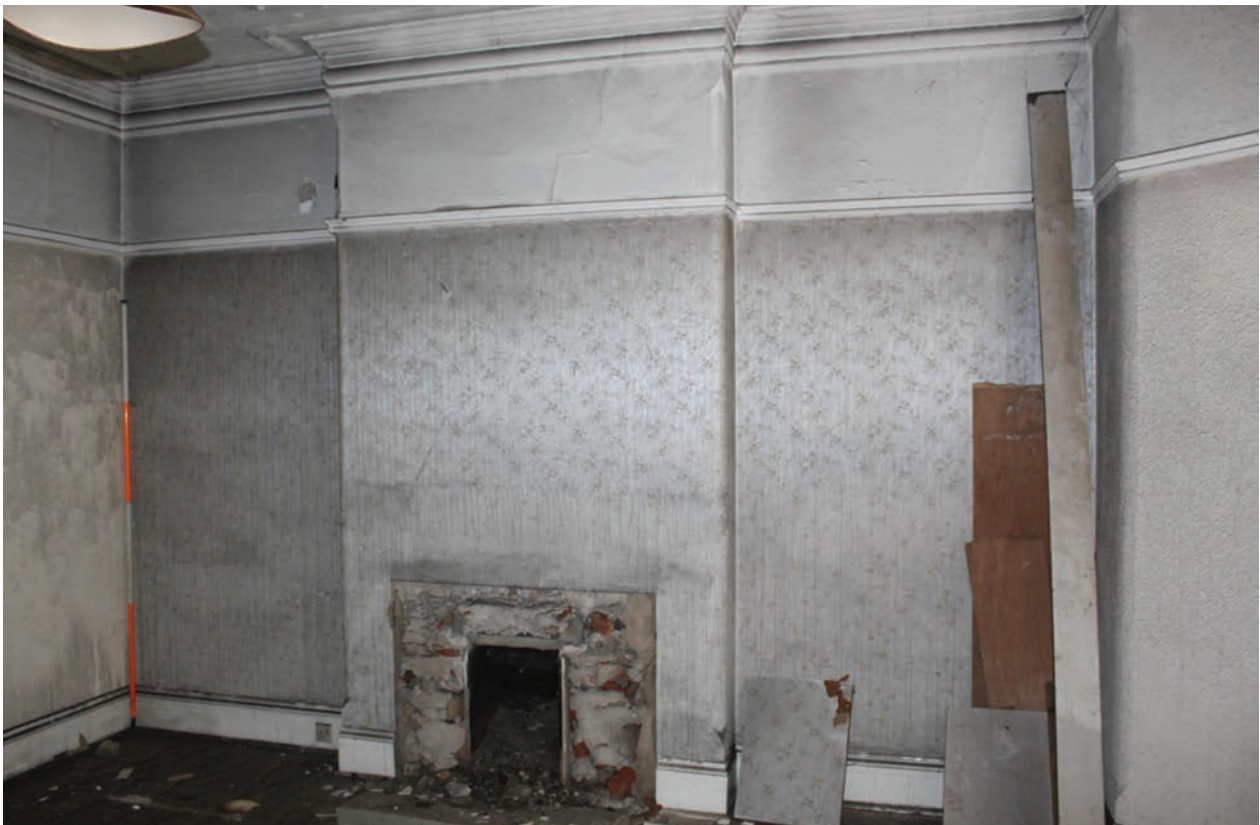
Figure 124 South wall of Room G9, facing south. Scale 1x2 m
