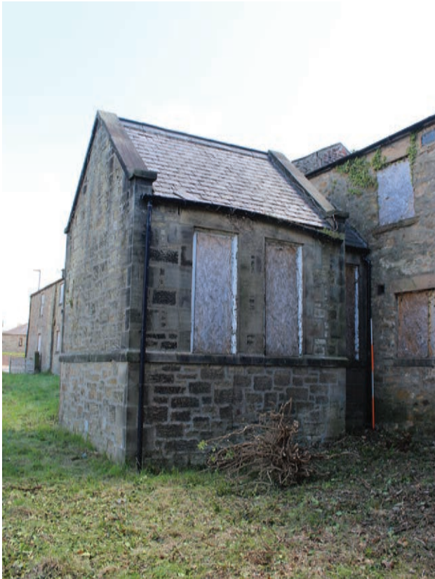
Figure 202 Detail of 1883 addition to the north elevation of Building C, facing south-east. Scale 1x2 m
