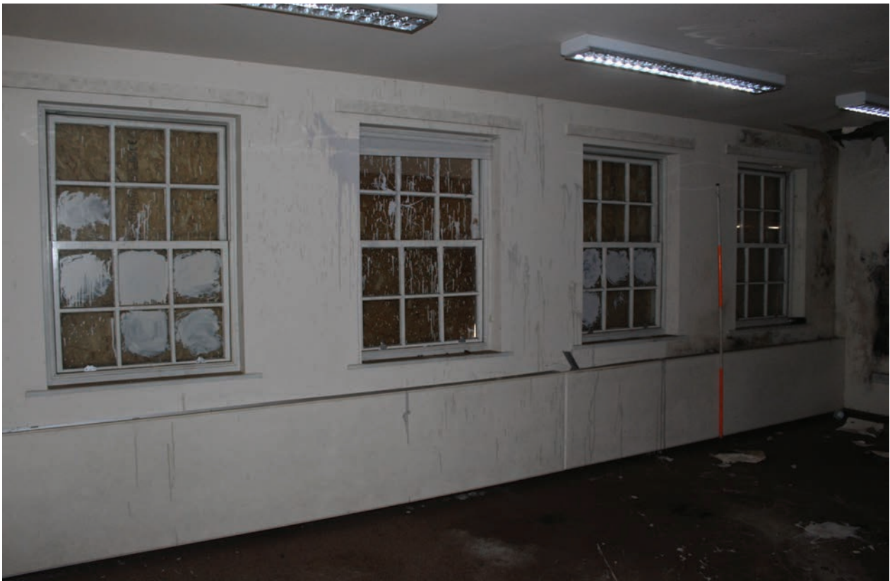
Figure 23 North wall of Room G10, facing north-east. Scale 1x2 m
