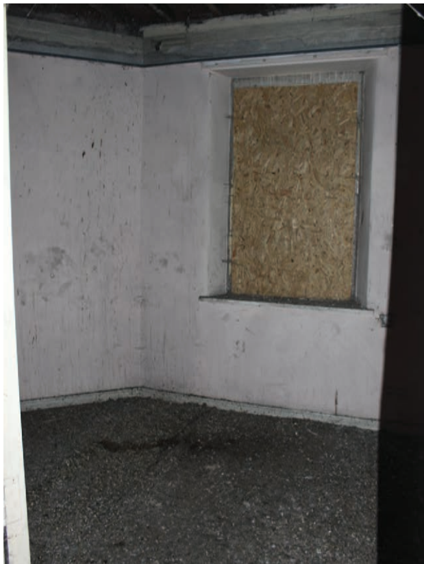
Figure 247 Room F11, facing north-west. No scale
