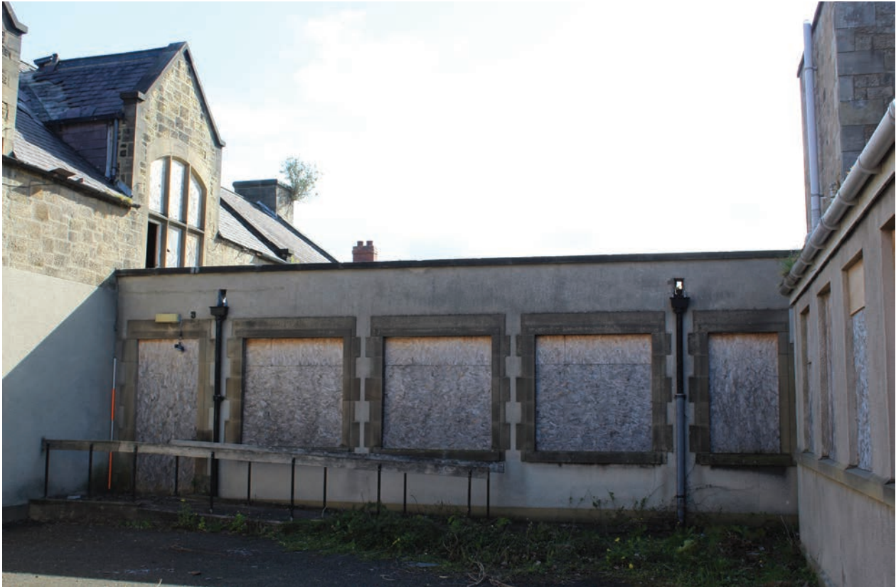
Figure 16 Western elevation of the north/south aligned corridor linking Building A to Building B, facing east. Scale 1x2 m
