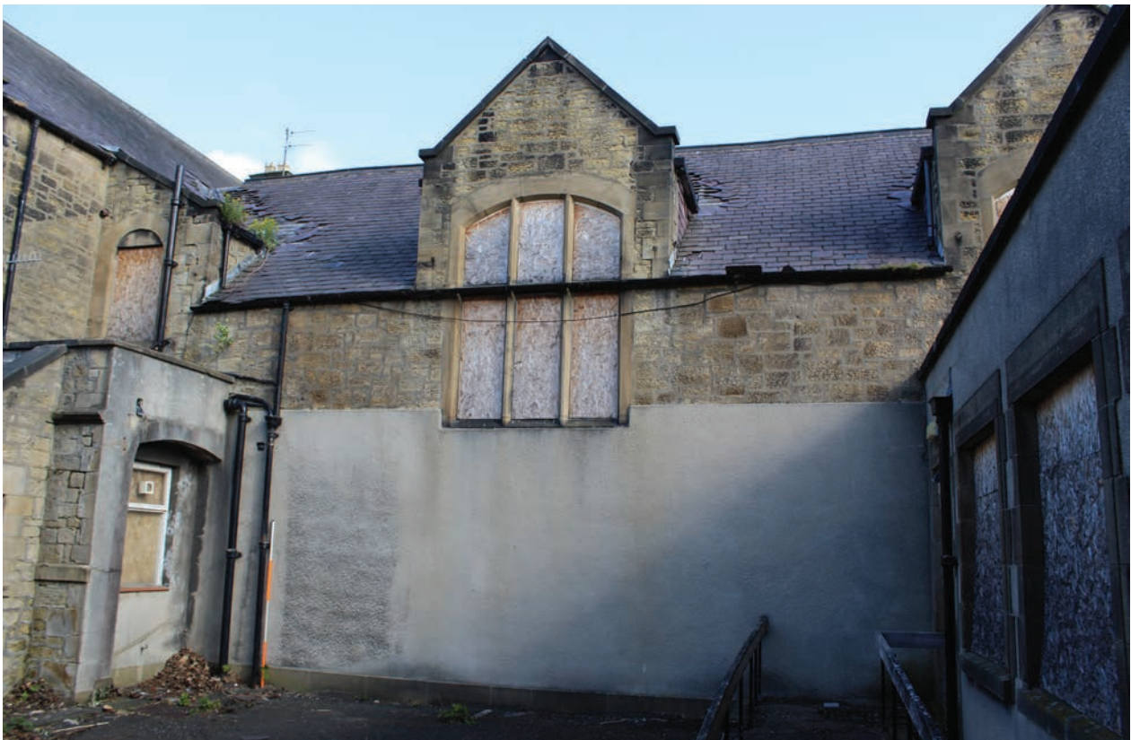
Figure 94 South elevation of the dining hall in Building B, facing north. Scale 1x2 m
