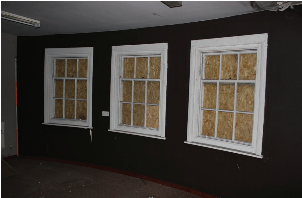
Figure 66 West wall of Room F1, looking south-west. Scale 1x2 m
