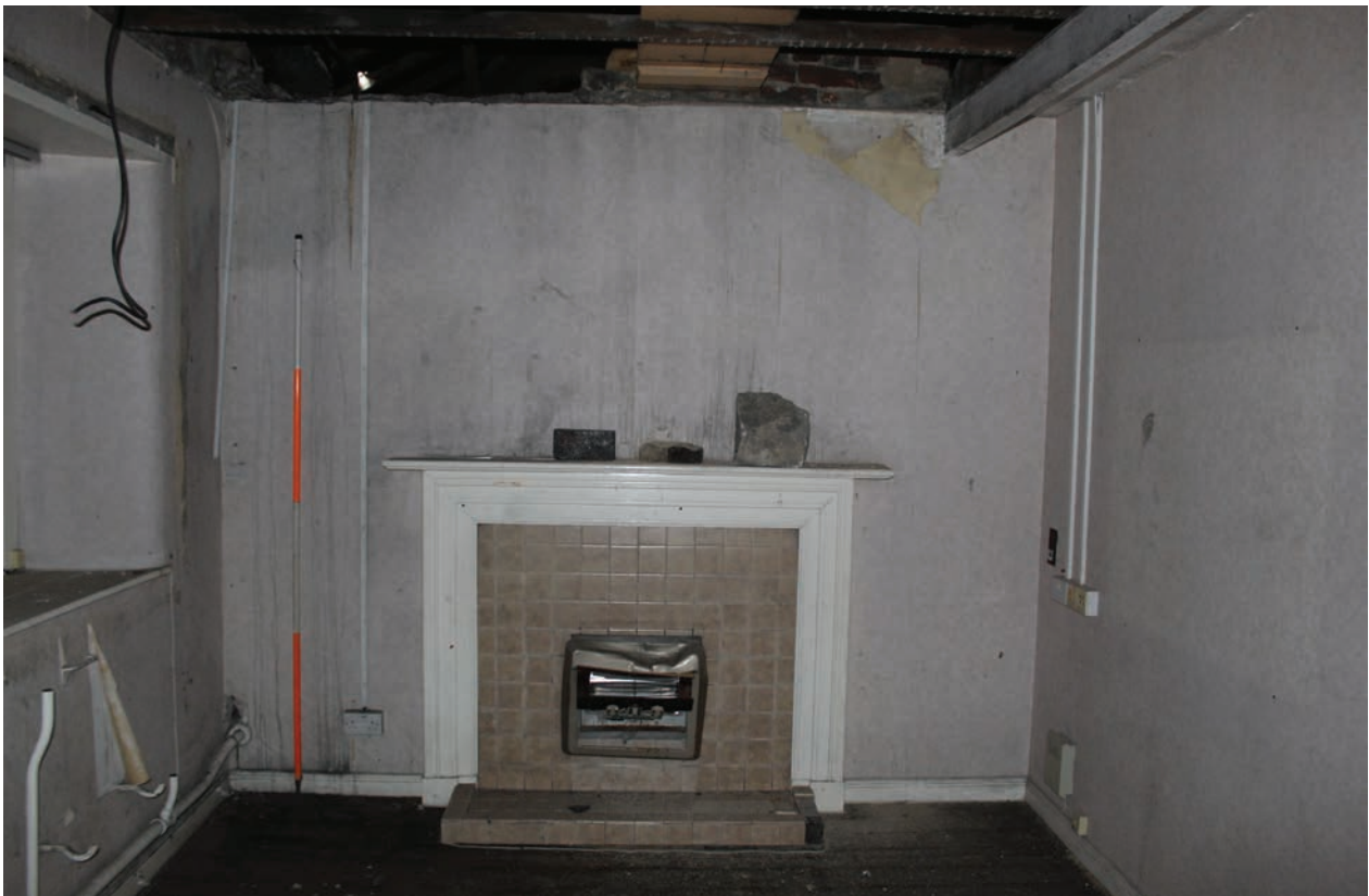
Figure 78 West wall of Room F26, facing west. Scale 1x2 m
