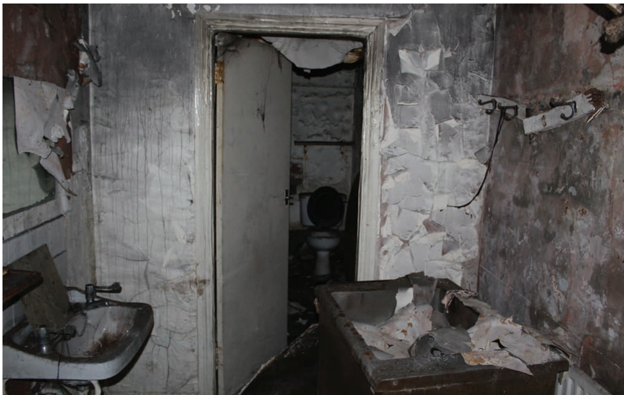
Figure 120 Room G5, facing south. No scale
