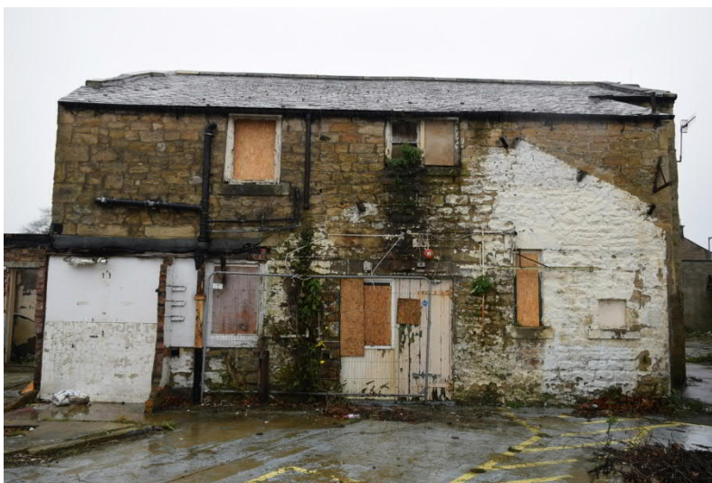
Figure 25. East elevation of the former fever wards in the stone breaking yard to the east of the workhouse.
