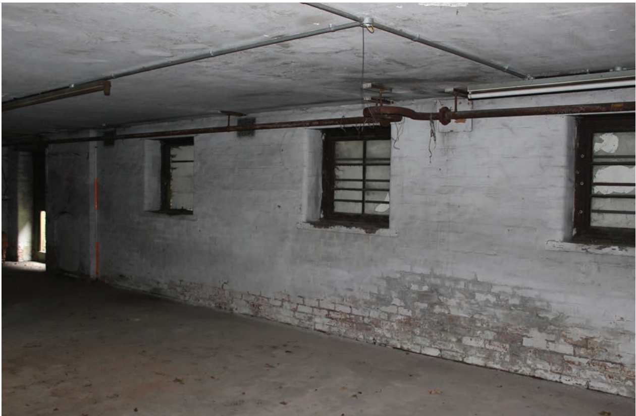
Figure 208 North wall of Room LG1, facing north-west. Scale 1x2 m
