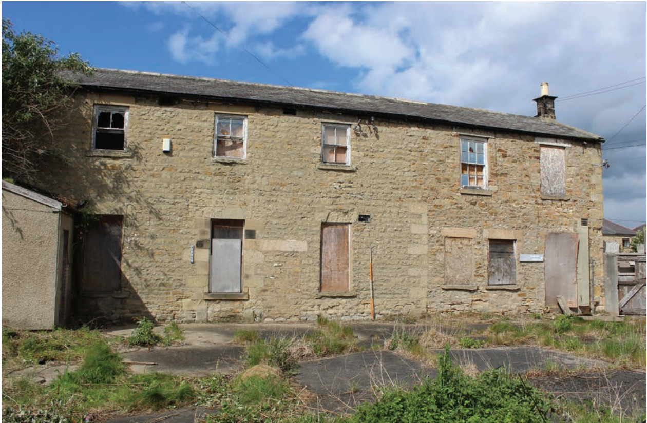
Figure 187 Eastern end of the south elevation of Building C, facing north-east. Scale 1x2 m
