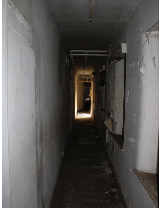
Figure 40 Room G28, facing west. Scale 1x2 m
