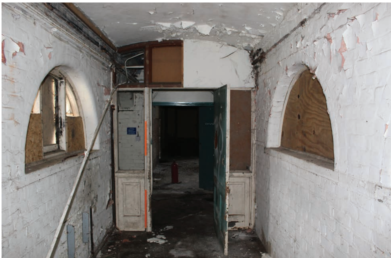
Figure 135 Room G14, facing south. Scale 1x2 m
