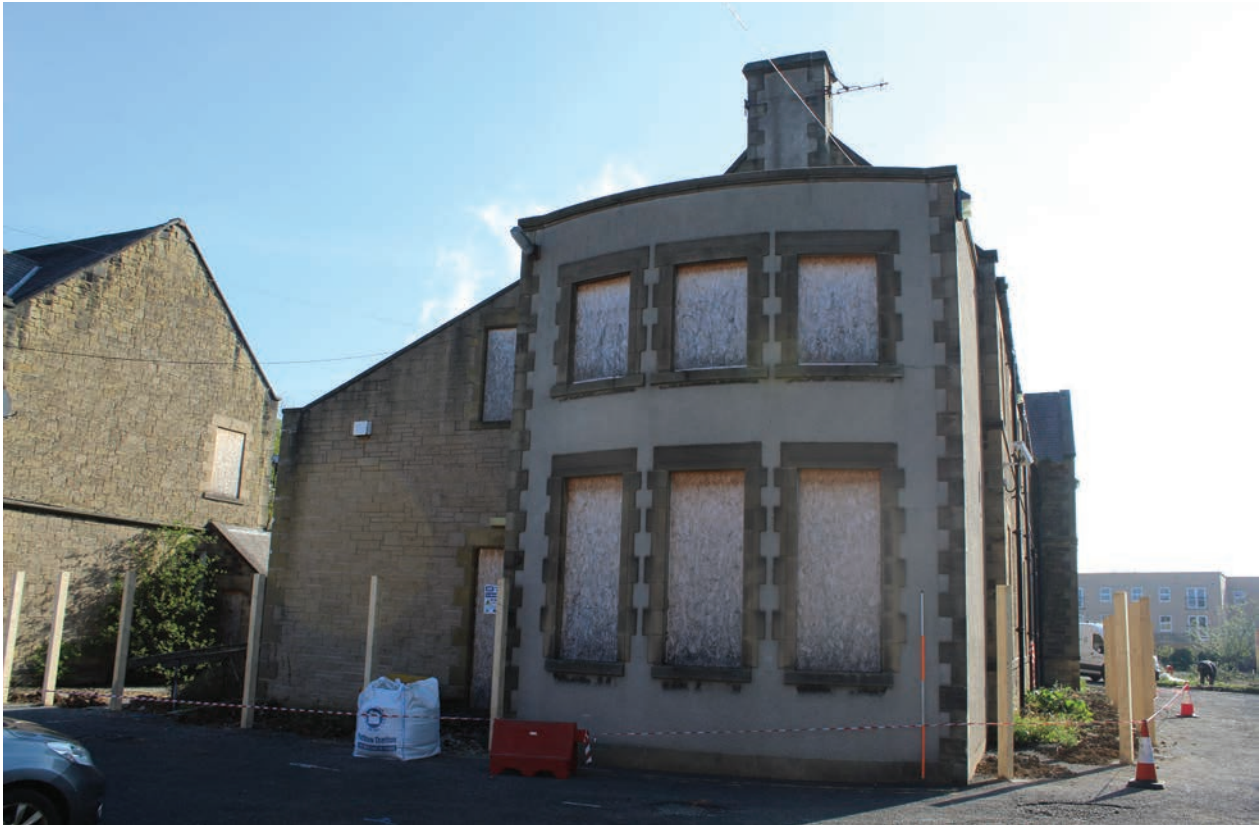
Figure 9 Western elevation of Building A, facing north-east. Scale 1x2 m
