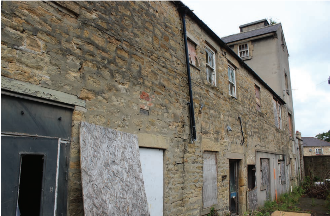
Figure 111 East elevation of Building B, facing north. Scale 1x2 m
