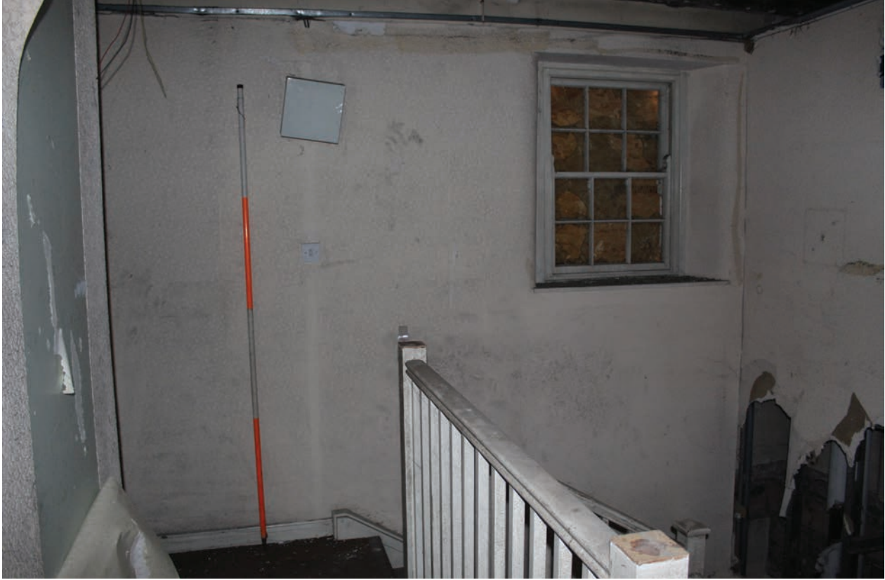
Figure 61 North wall of Room F37, facing north. Scale 1x2 m
