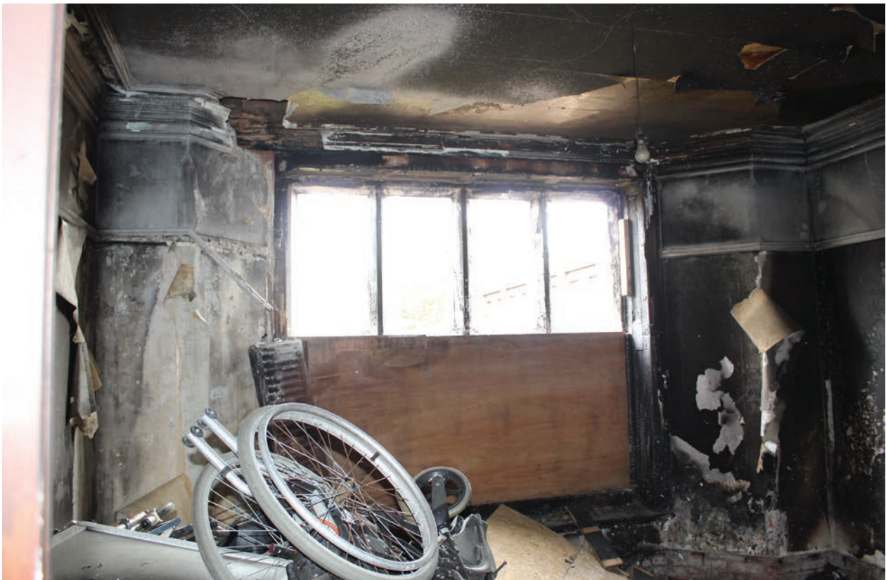
Figure 115 West wall of Room G1, facing west. No scale
