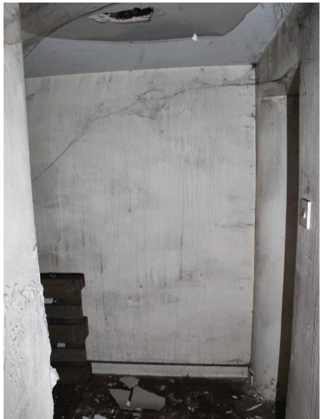
Figure 122 Room G8, looking south. No scale
