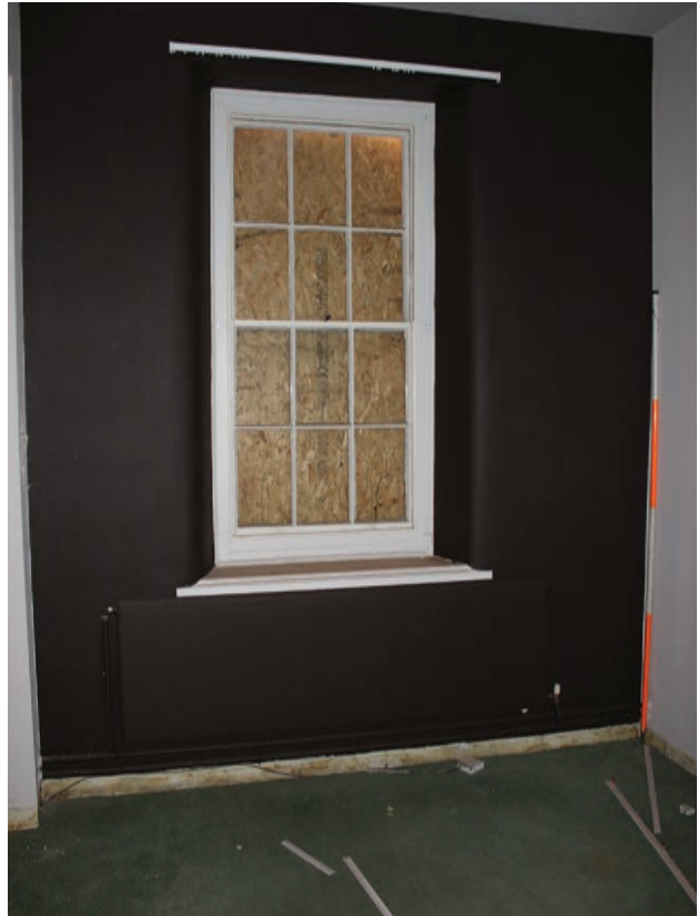
Figure 20 South wall of Room G5, facing south. Scale 1x2 m
