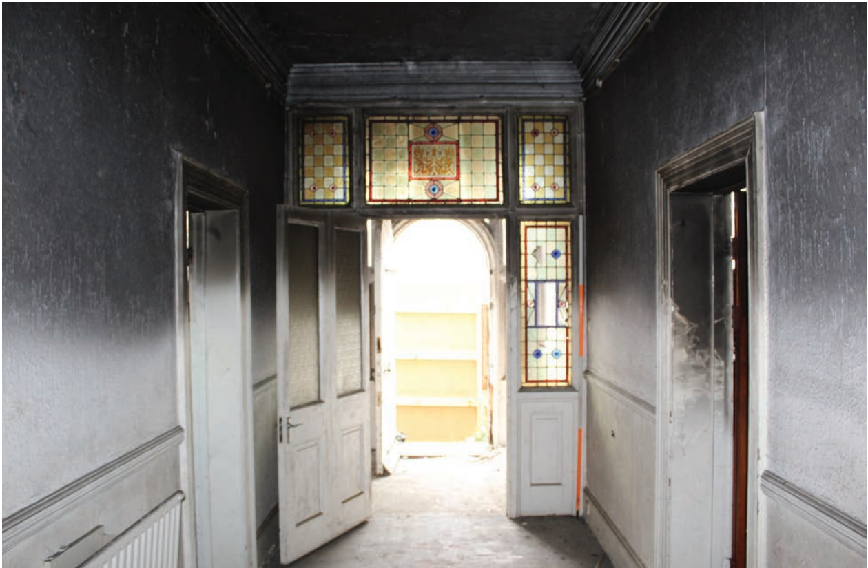
Figure 119 Room G3, facing west. Scale 1x2 m
