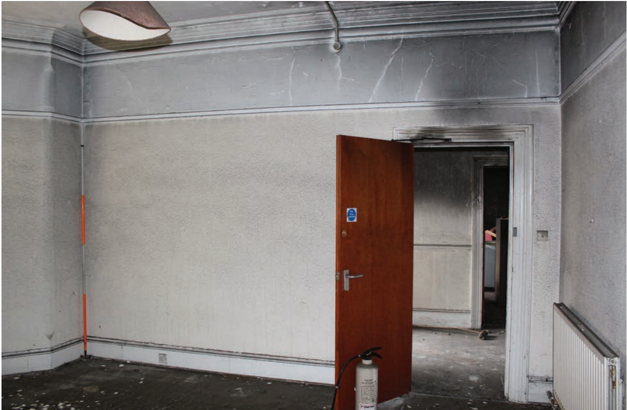
Figure 123 North wall of Room G9, facing north. Scale 1x2 m
