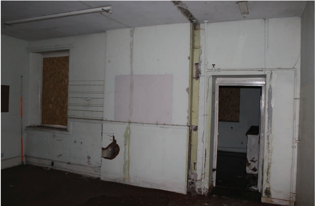
Figure 244 North wall of Room F8, facing north. Scale 1x2 m
