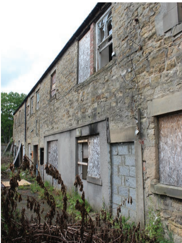
Figure 112 East elevation of Building B, facing south. Scale 1x2 m
