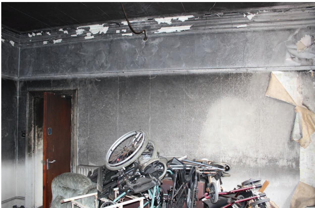
Figure 113 South wall of Room G1, facing south-east. No scale
