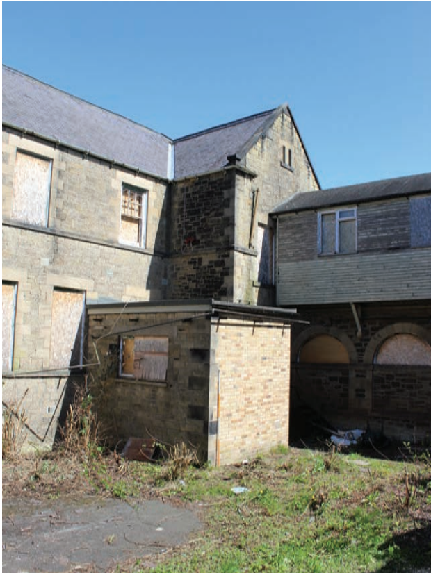
Figure 190 Detail of the gabled bay marking the junction between the older phases of the workhouse and the 1883 extension on Building C, facing north-east. Scale 1x2 m
