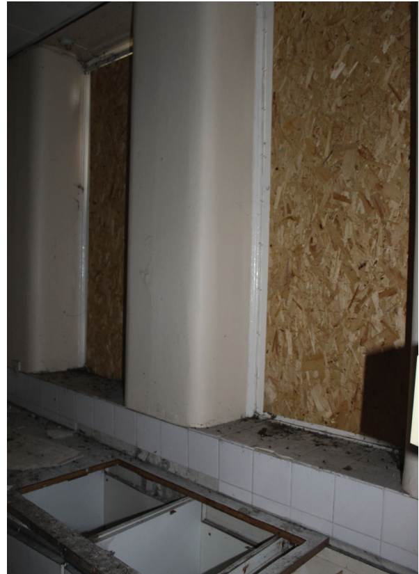
Figure 240 Paired windows in the north wall of Room F1, facing north-west. No scale
