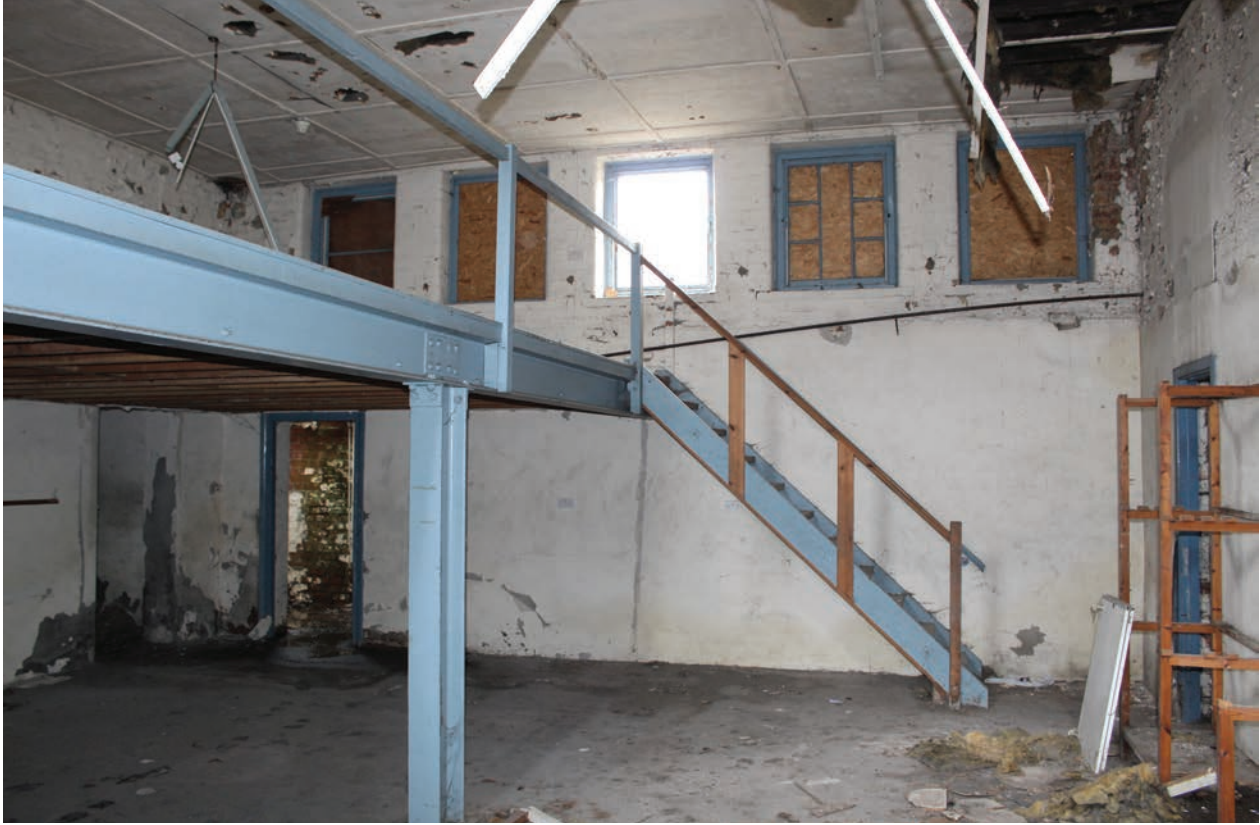
Figure 138 Room G16, looking south-east. No scale
