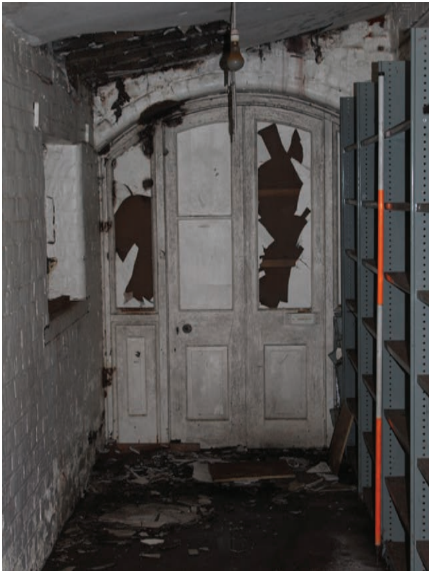
Figure 143 Room G21, looking west. Scale 1x2 m
