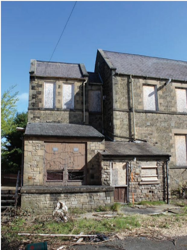
Figure 192 Western end of south elevation of Building C, facing north. Scale 1x2 m
