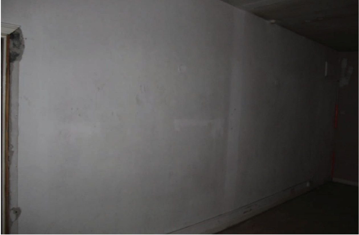
Figure 55 North wall of Room G40, facing north-east. Scale 1x2 m
