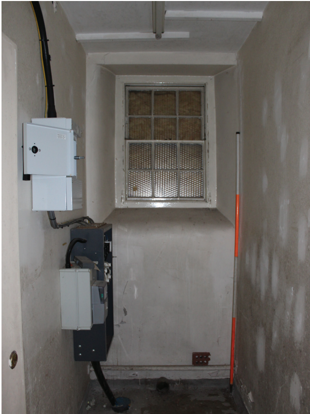
Figure 38 Room G26, facing south. Scale 1x2 m
