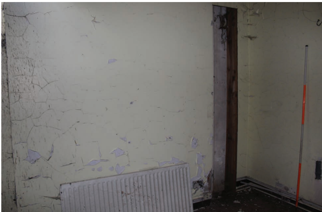
Figure 184 North and east walls of Room S1. Scale 1x2 m
