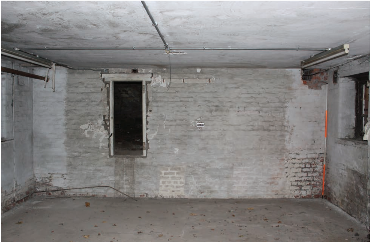
Figure 209 East wall of Room LG1, facing east. Scale 1x2 m
