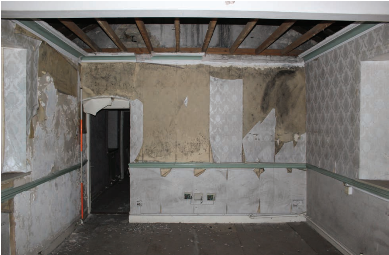
Figure 259 Room F22, facing east. Scale 1x2 m
