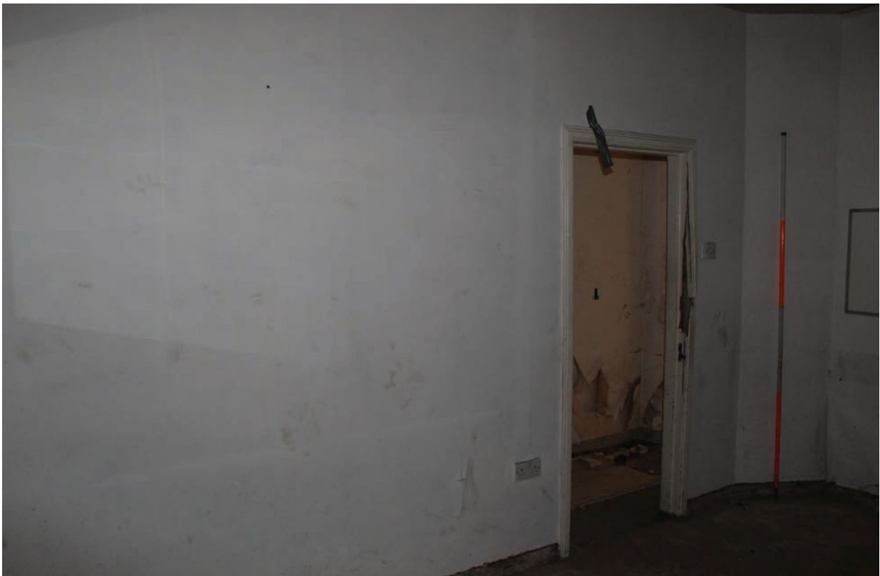
Figure 45 North wall of Room G33, facing north-east. Scale 1x2 m
