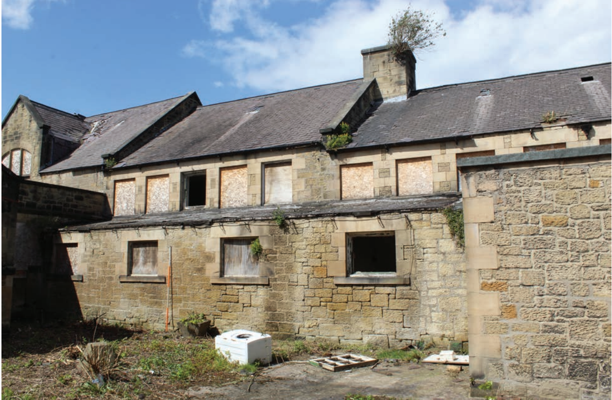
Figure 91 Detail of ranges with clerestory glazing in the 1883 portion of the south elevation of Building B, facing north-west. Scale 1x2 m
