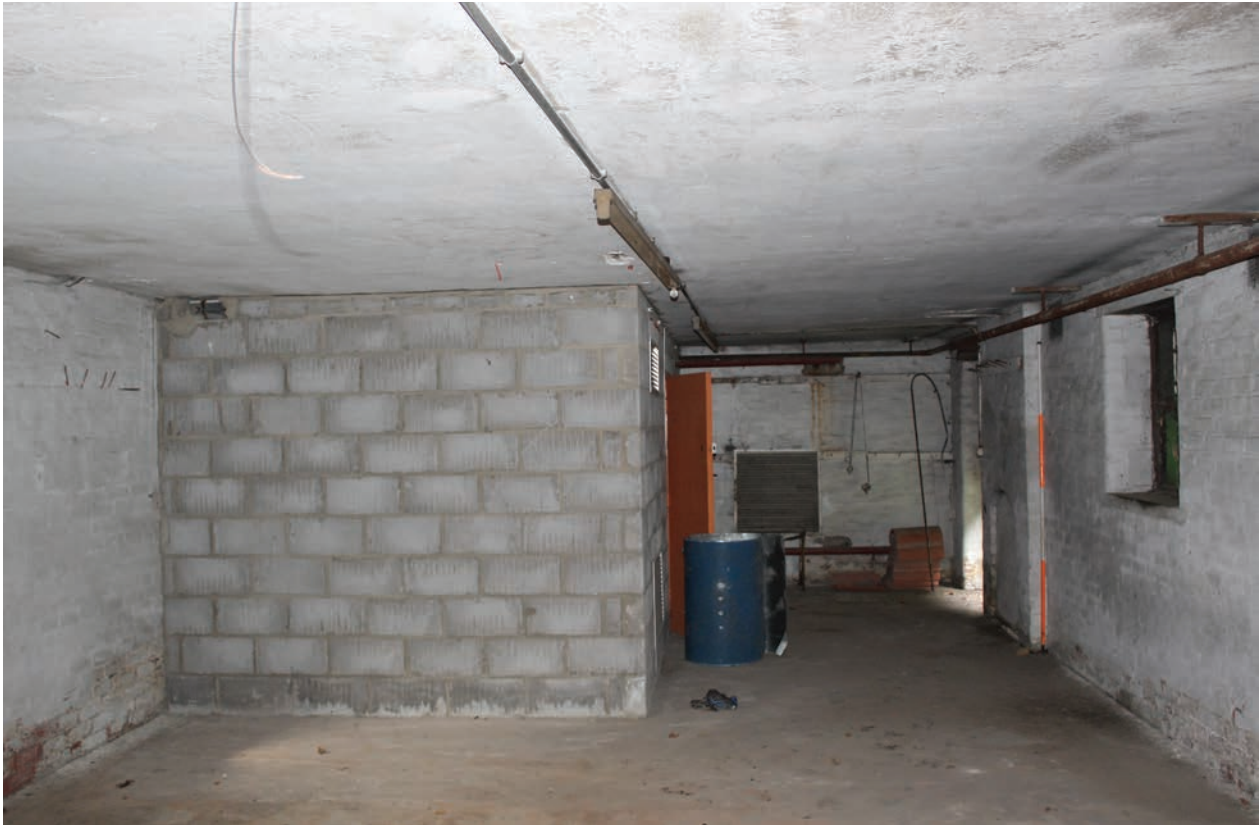
Figure 211 Room LG1, facing west. Scale 1x2 m
