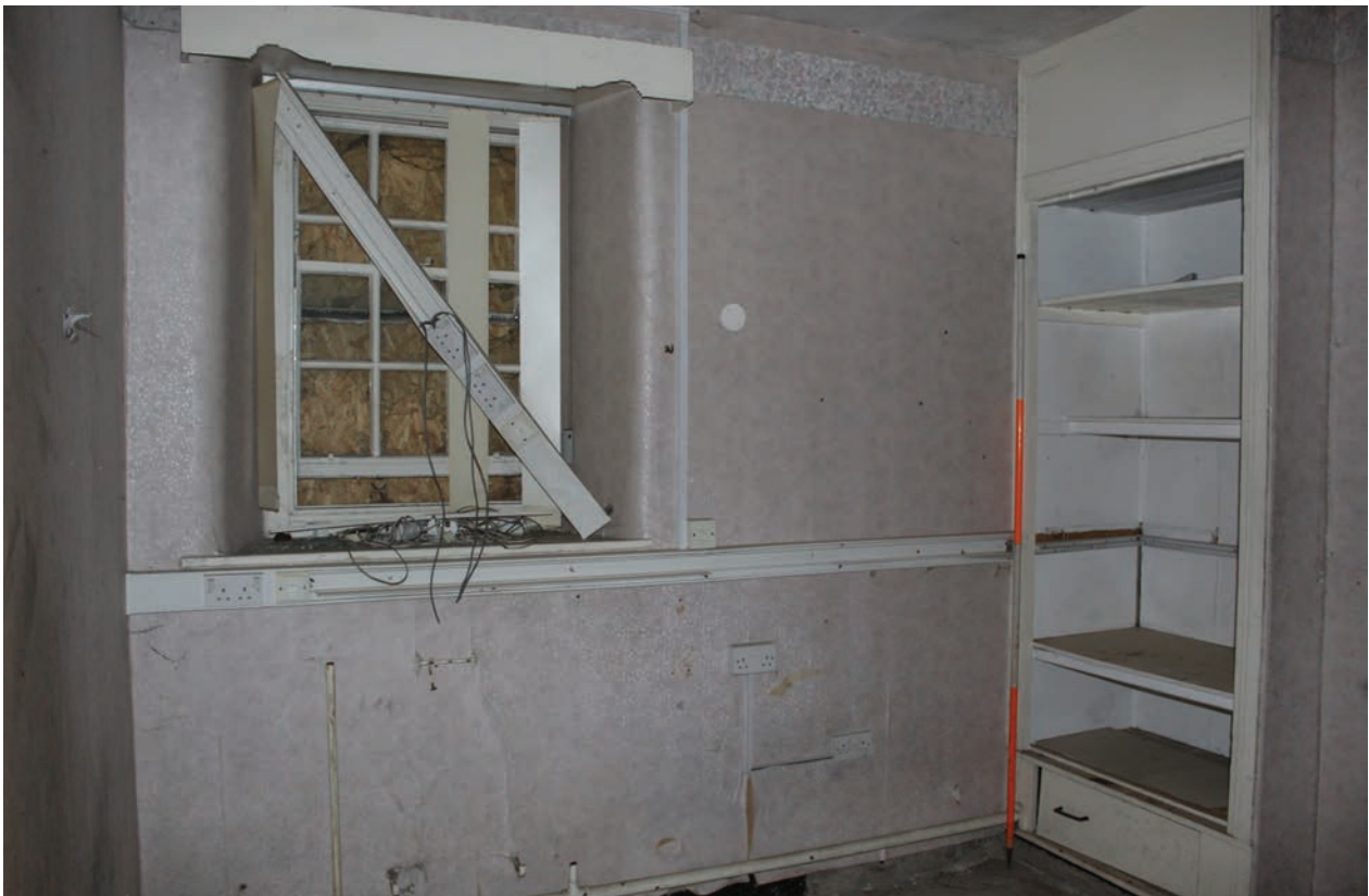
Figure 52 South wall of Room G38, facing south. Scale 1x2 m
