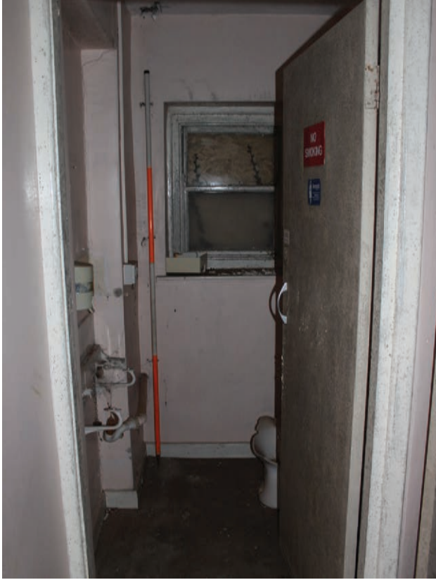
Figure 224 Facing north into Room G14. Scale 1x2 m
