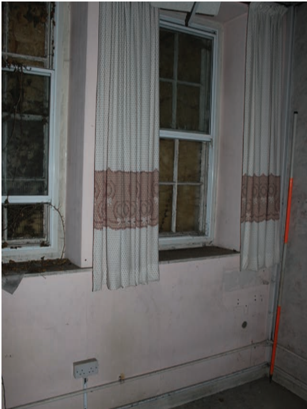
Figure 237 West wall of Room G27, facing north-west. Scale 1x2 m
