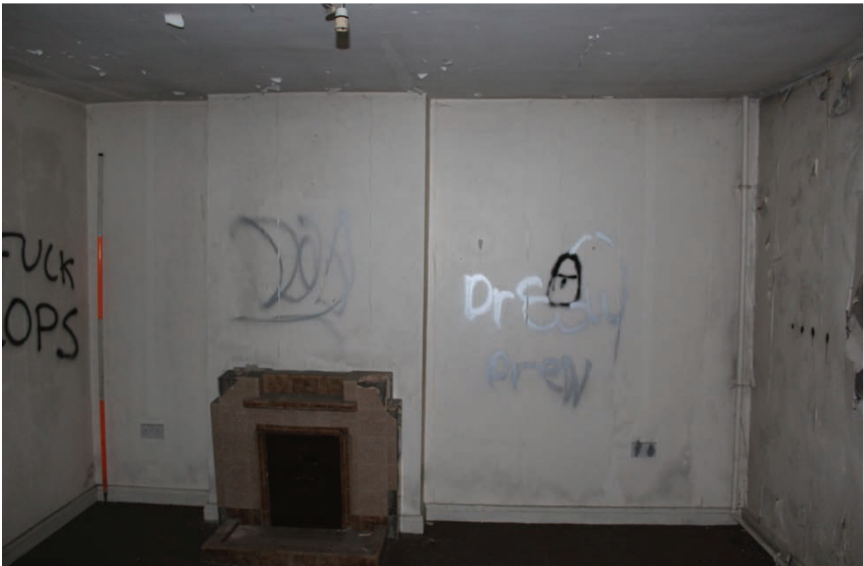
Figure 174 East wall of Room F17, facing east. Scale 1x2 m
