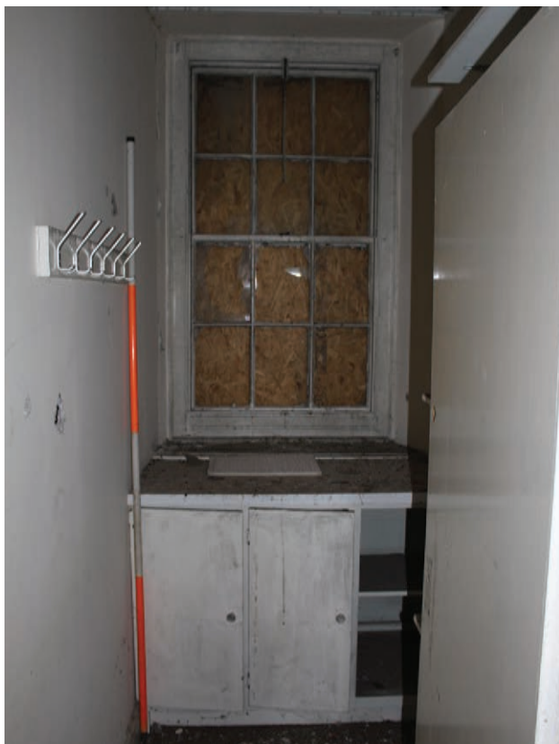
Figure 242 South wall of Room F5, facing north-west. Scale 1x2 m
