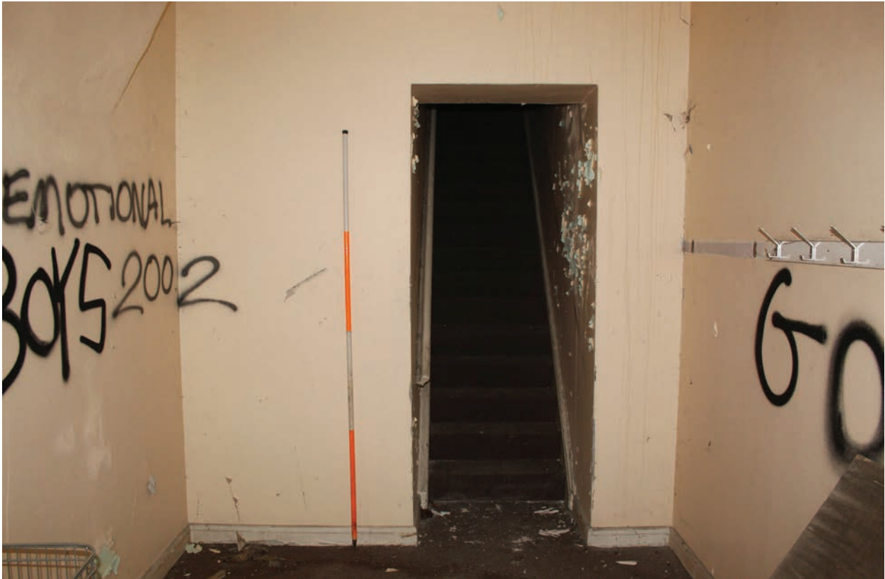
Figure 161 West wall of Room G39, showing inserted staircase mirrored in Room G41 to the south. Scale 1x2 m
