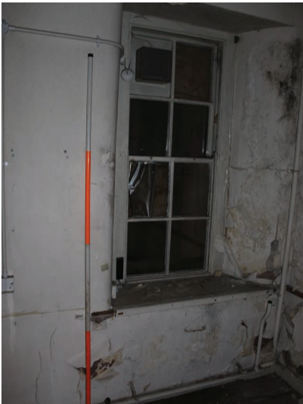
Figure 230 Facing south-west in Room G22. Scale 1 x 2 m
