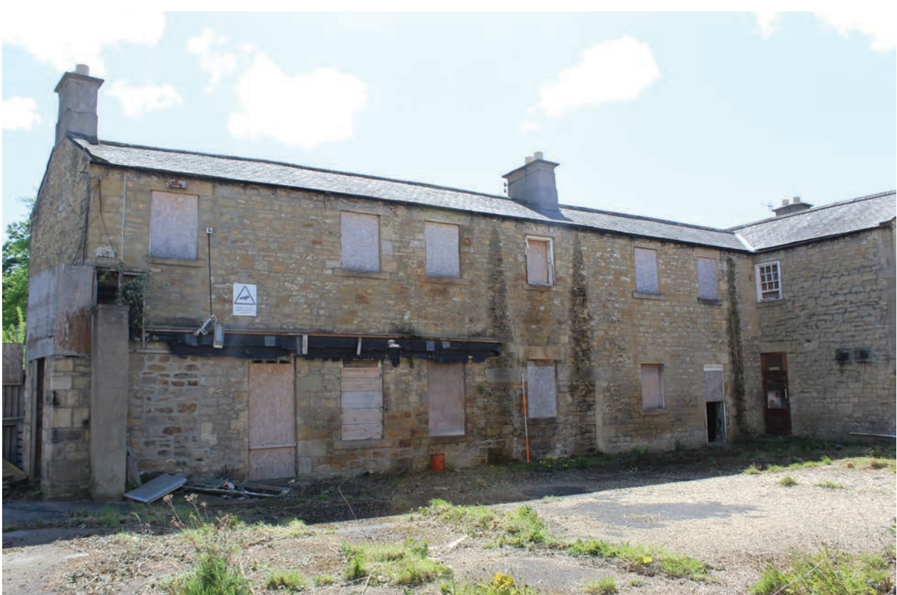
Figure 14 Eastern end of the north elevation of Building A, facing south. Scale 1x2 m
