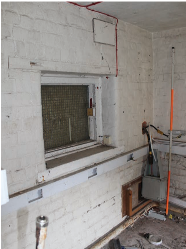
Figure 145 Room G23, facing south-east. Scale 1x2 m
