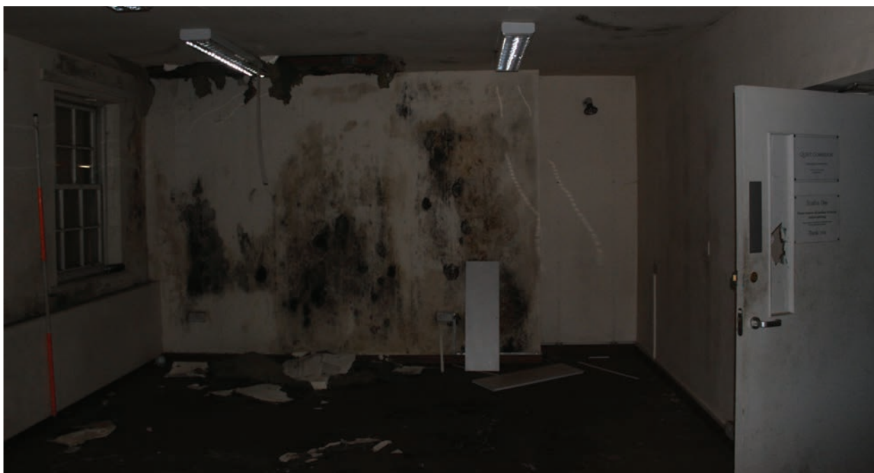
Figure 24 East wall of Room G10, facing east. Scale 1x2 m
