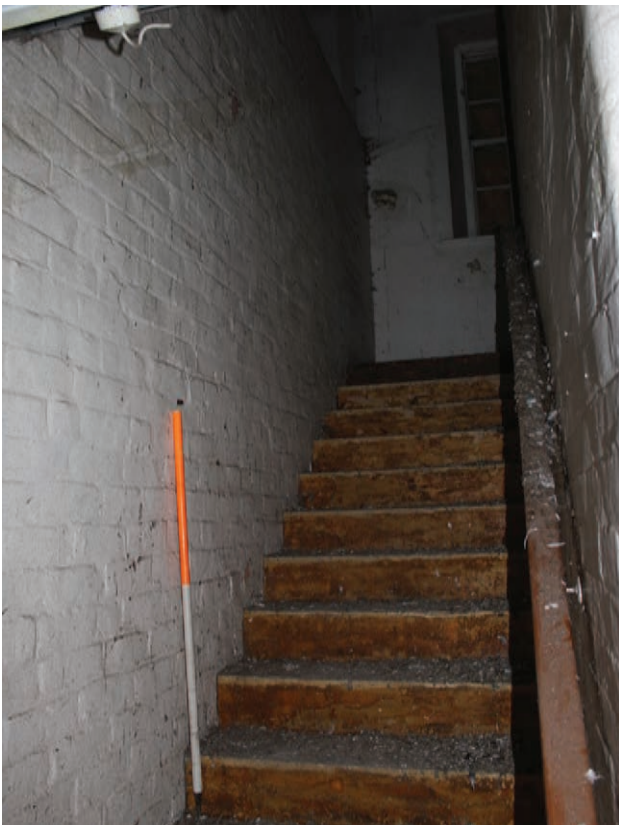
Figure 220 Looking south-east up the stairwell in Room G12. Scale 1 x 1 m
