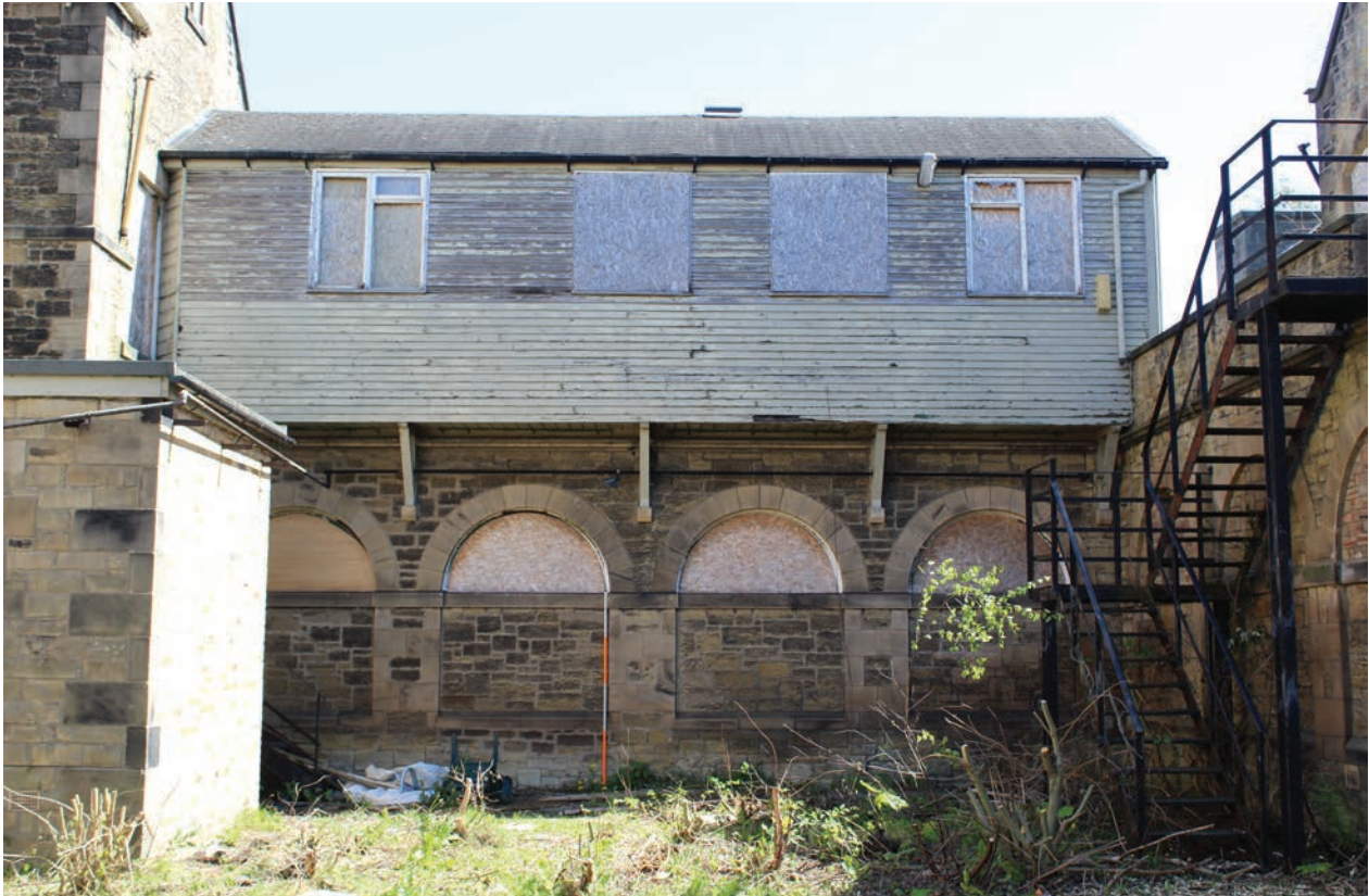
Figure 108 Detail of west elevation of the corridor linking Building B to Building C, facing east. Scale 1x2 m
