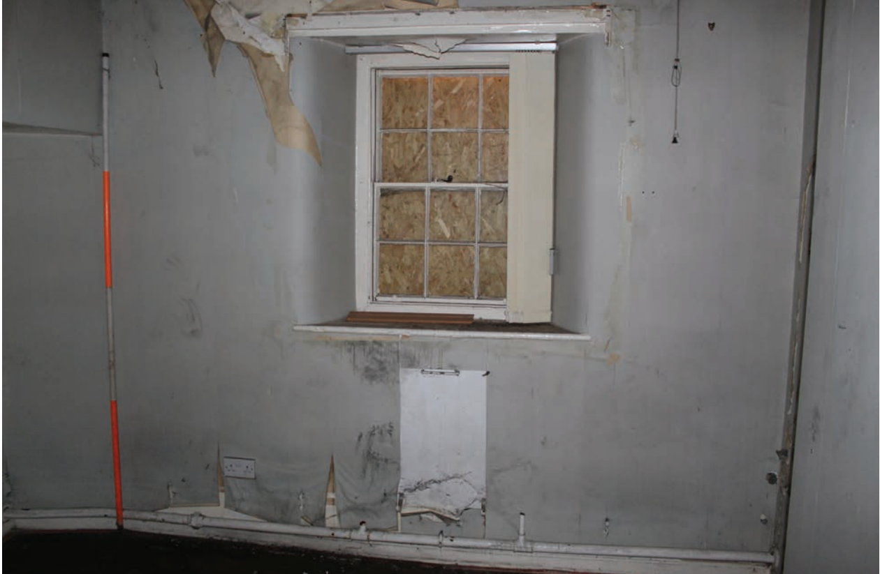
Figure 77 South wall of Room F25, facing south. Scale 1x2 m
