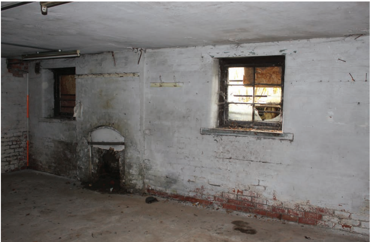
Figure 210 South wall of Room LG1, facing south-east. Scale 1x2 m
