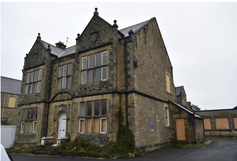
Figure 16. The master's house from the south-west (compare to Figure 7).
