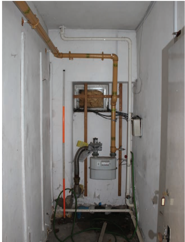
Figure 50 Room G37, facing south. Scale 1x2 m
