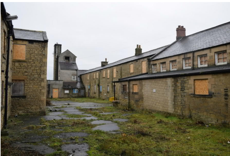
Figure 19. View south-east within the men's yard on the north side of the workhouse.
