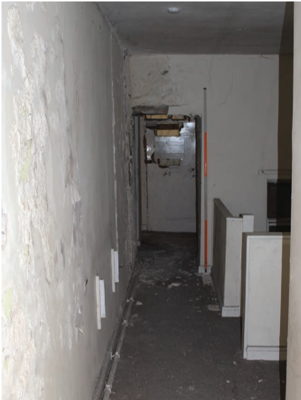
Figure 179 Looking south along the length of Room F22. Scale 1x2 m
