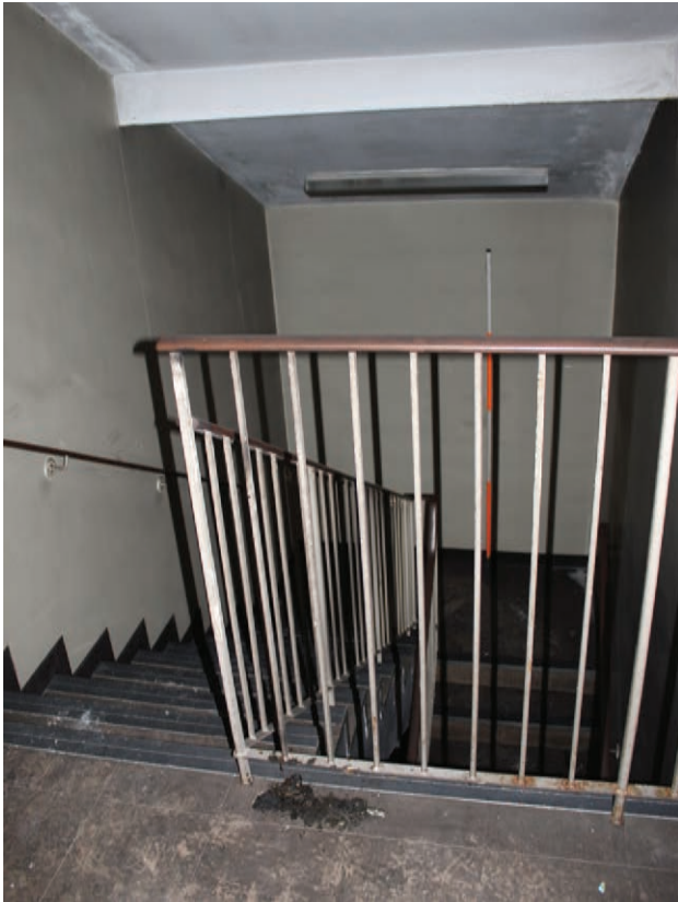
Figure 25 Stairwell Room G12/F38, looking north. Scale 1x2 m
