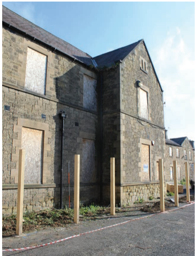
Figure 7 Detail of the western elevation of the southward projection of the 1883 extension on the south elevation of Building A, facing north-east. Scale 1x2 m
