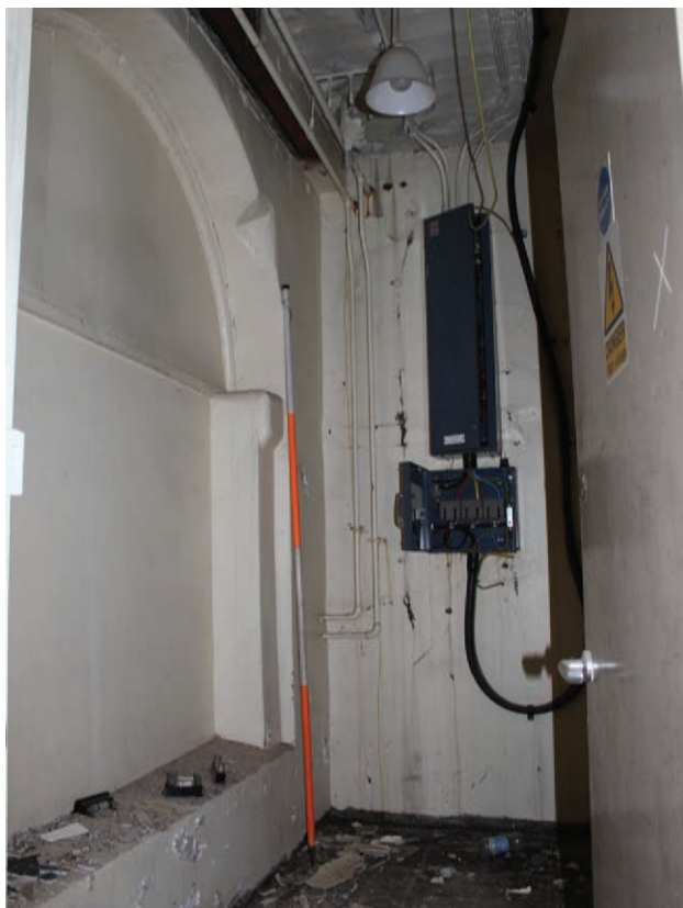
Figure 36 Room G23, facing north. Scale 1x2 m
