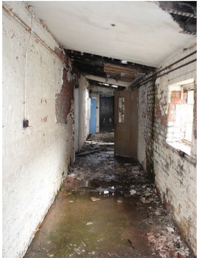
Figure 144 Room G22, facing west. Scale 1x2 m
