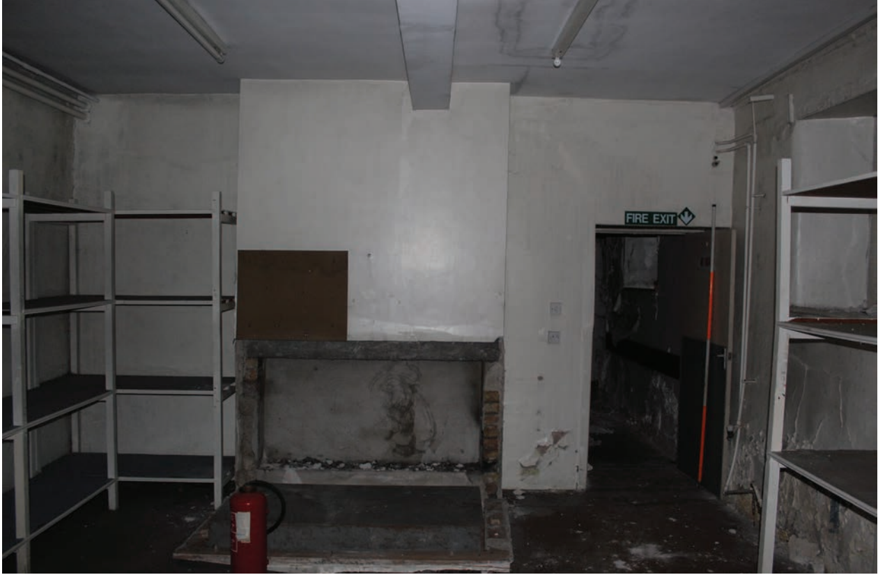
Figure 153 East wall of Room G29, facing east. Scale 1x2 m
