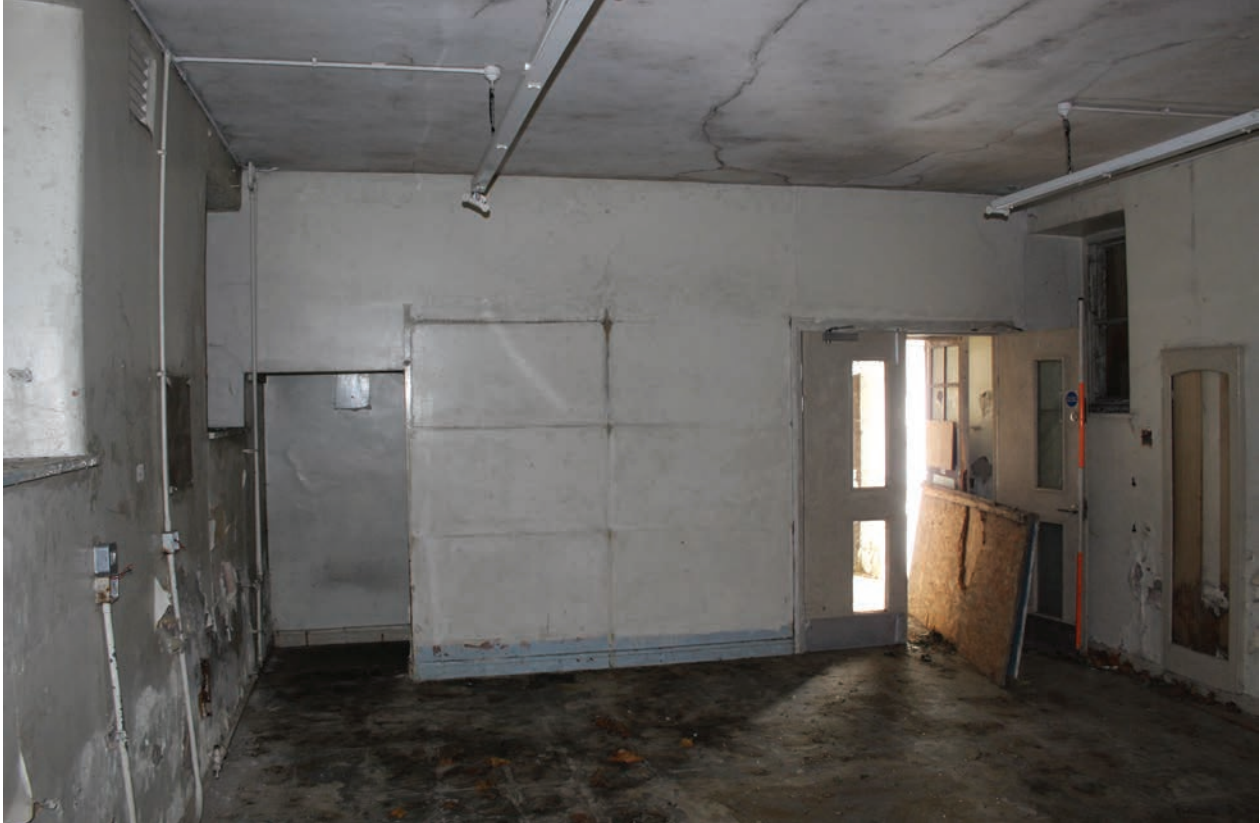
Figure 147 Room G24, facing east. Scale 1x2 m
