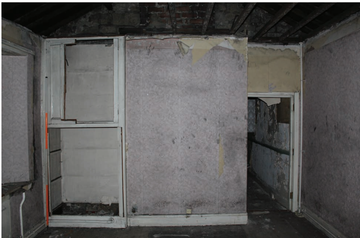
Figure 260 Room F23, facing east. Scale 1x2 m
