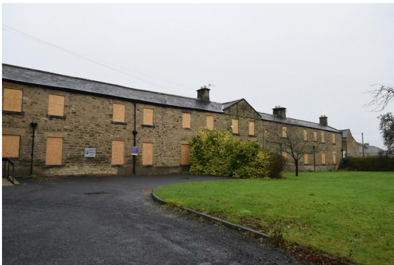
Figure 11. View across the eastern end of the south range showing the earlier phases of the workhouse.
