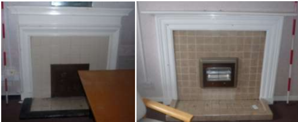
Plate 31. Surviving fireplaces in the Fairington Centre; these merit reuse to reference the Victorian character, but do not need to remain in situ
