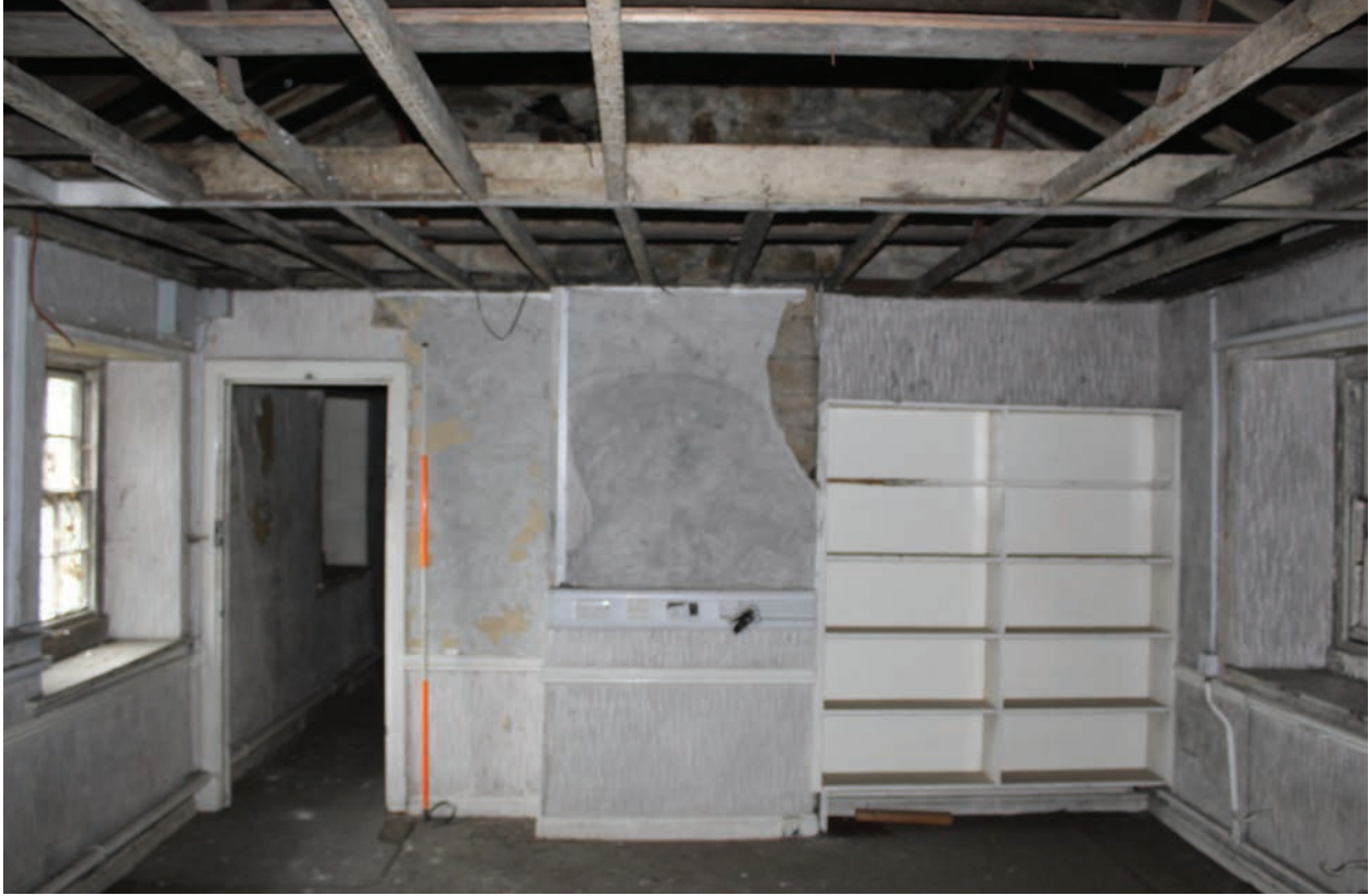
Figure 251 Room F14, facing east. Scale 1x2 m
