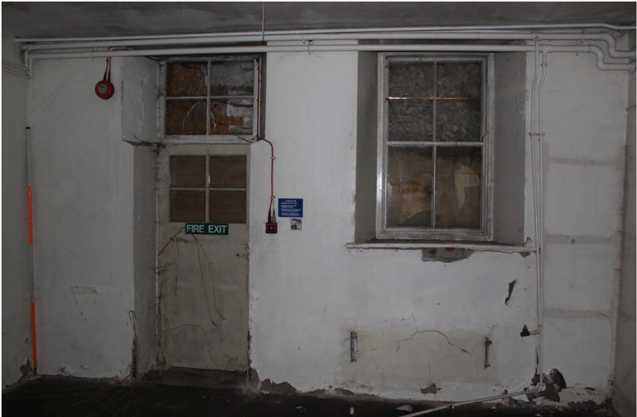
Figure 154 North wall of Room G30, facing north. Scale 1x2 m
