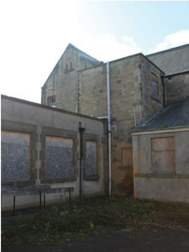
Figure 18 Detail of two-storey projection on the north elevation of the western end of Building A, facing south-east. Scale 1x2 m
