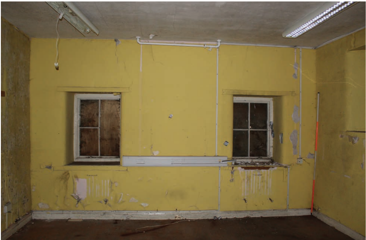
Figure 238 South wall of Room G30, facing south. Scale 1x2 m
