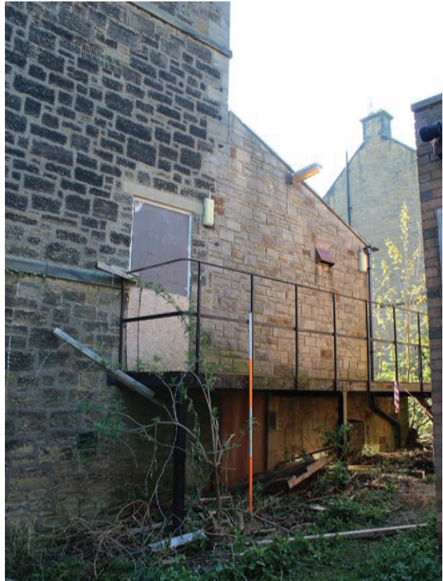
Figure 194 Western elevation of Building C, facing south-east. Scale 1x2 m
