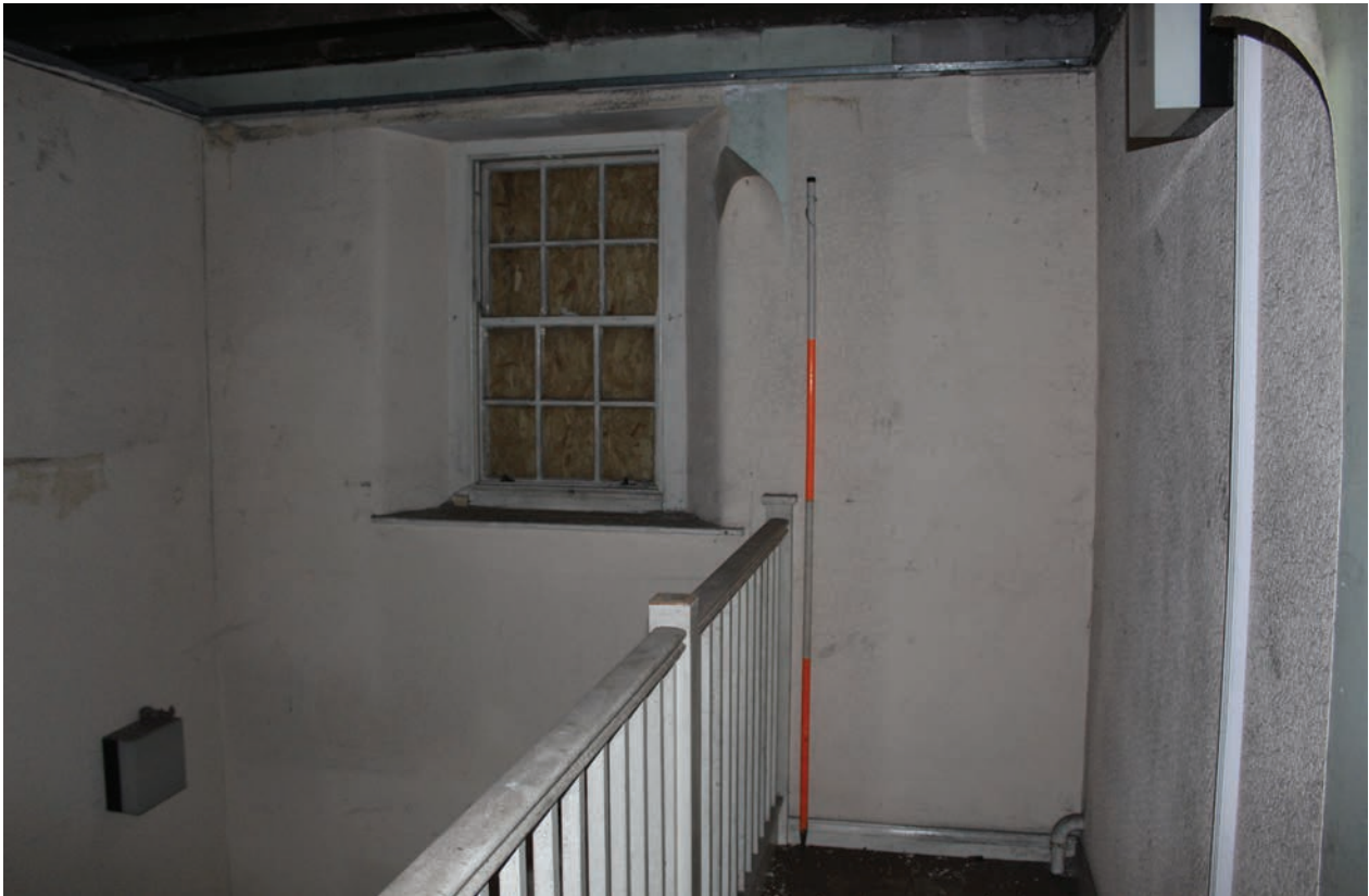
Figure 62 South wall of Room F37, facing south. Scale 1x2 m
