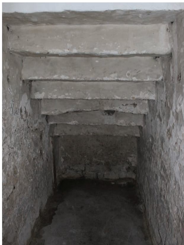
Figure 166 View of Room G49, looking south. No scale
