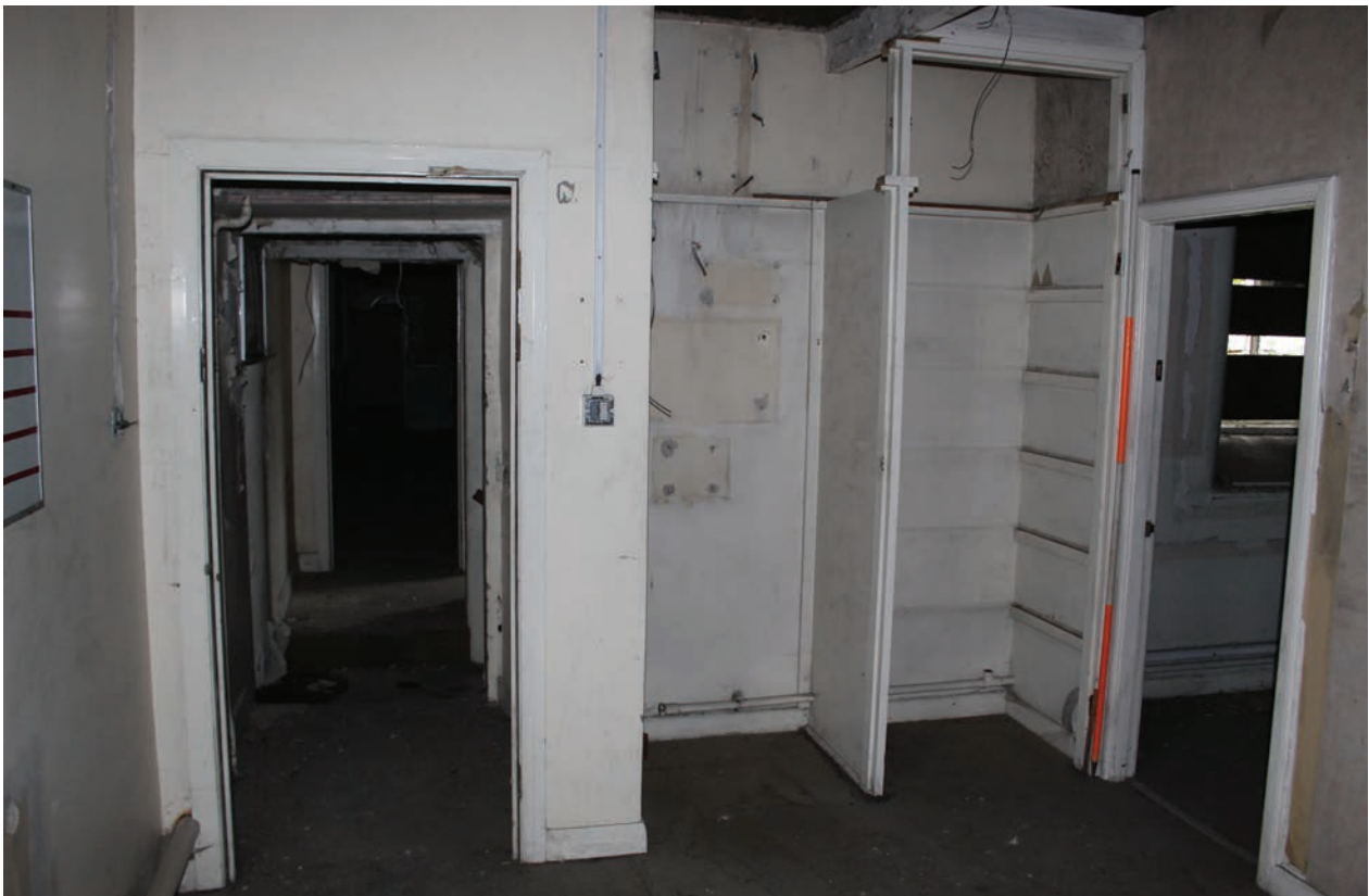
Figure 257 Room F20, facing east. Scale 1x2 m
