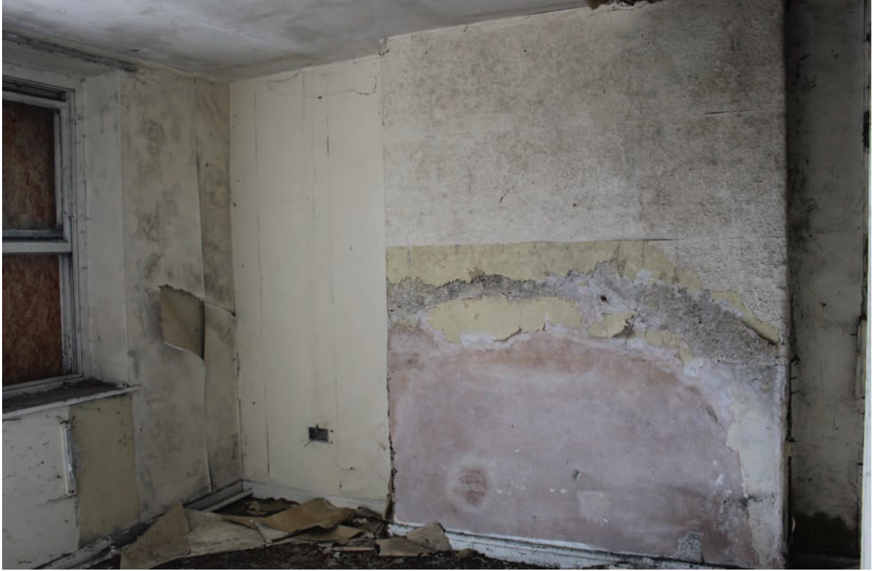
Figure 178 South wall of Room F20, facing south-east. Scale 1x2 m
