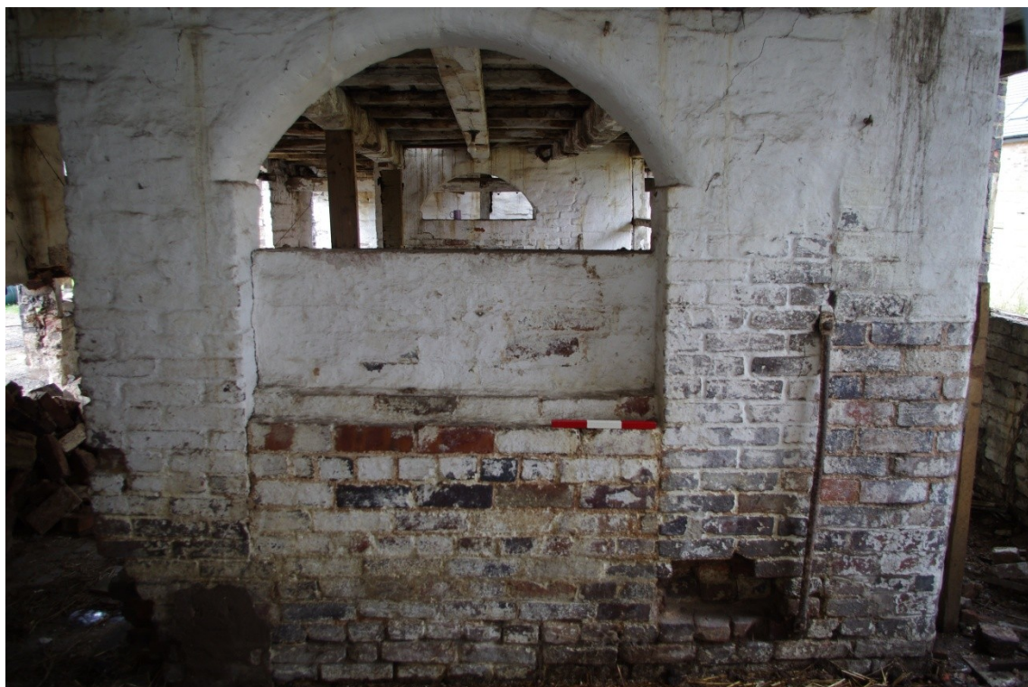
Figure 12 Cross Wall Between D & E Showing Multiple Building Phases.
