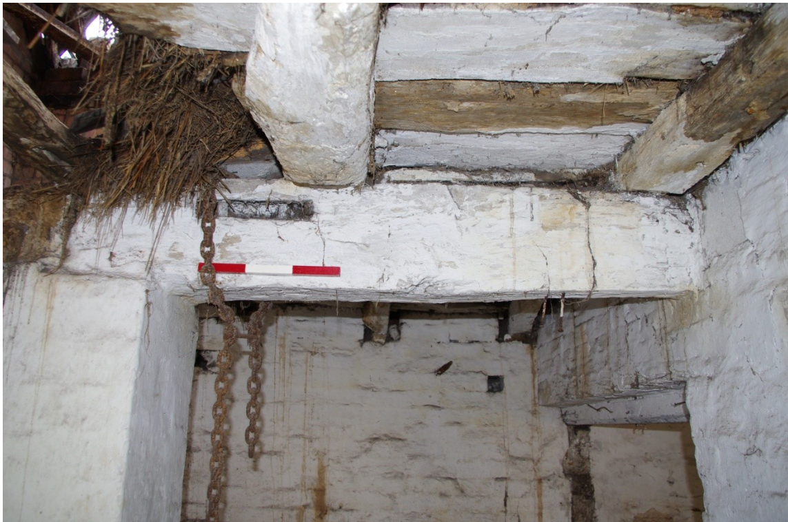
Figure 14 Re-used Bridging Beam E .
