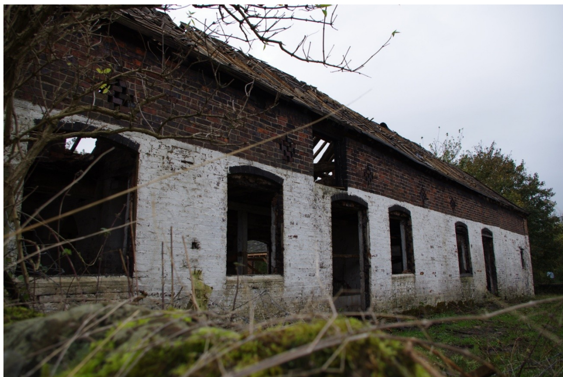
Figure 8 Rear Elevation (Oblique View looking South).
