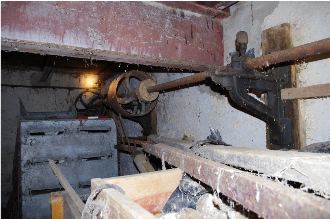
Figure 12 Line Shaft on Rear Wall of A (looking North West).
