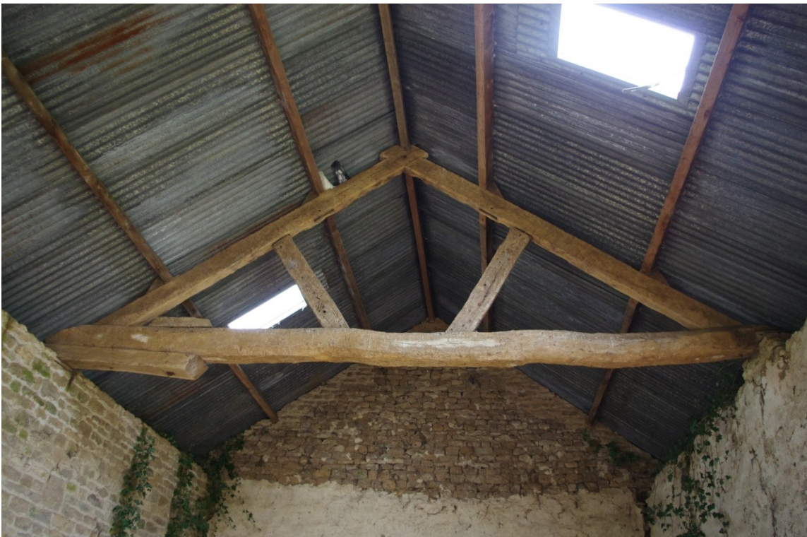
Figure 14 Truss Tr01 (looking East).
