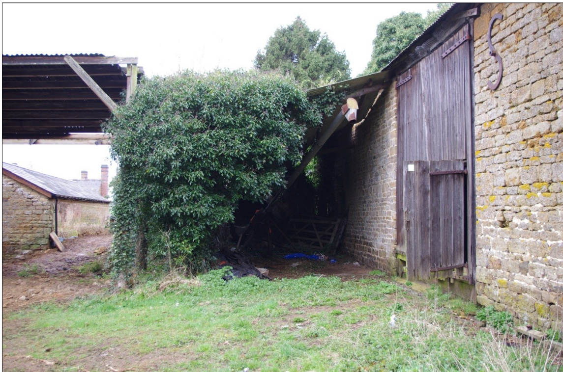
Figure 8 Lean To on Principal Elevation (looking West).
