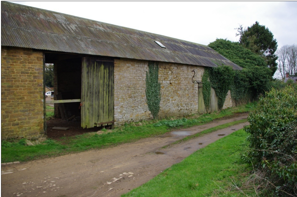
Figure 7 Rear, North Facing Elevation (looking South West).
