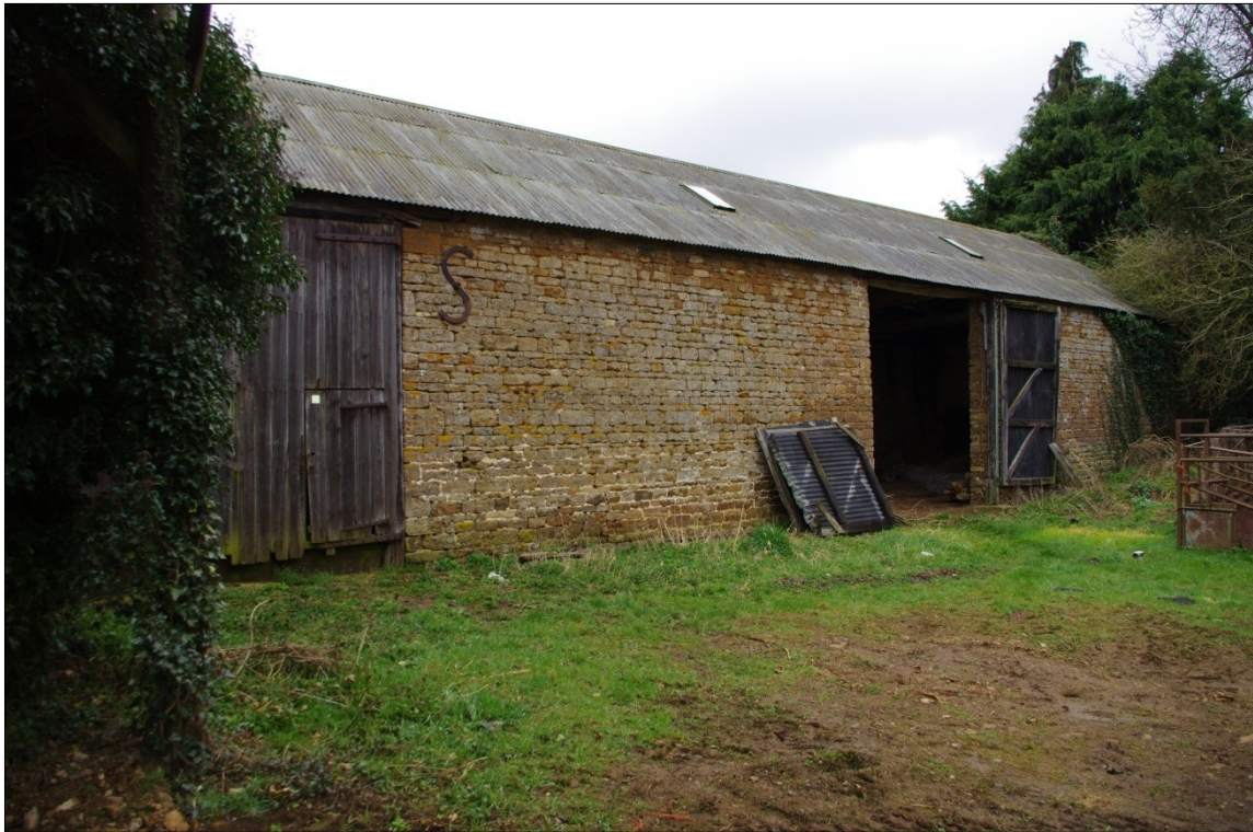
Figure 5 Principal Elevation (looking North East).
