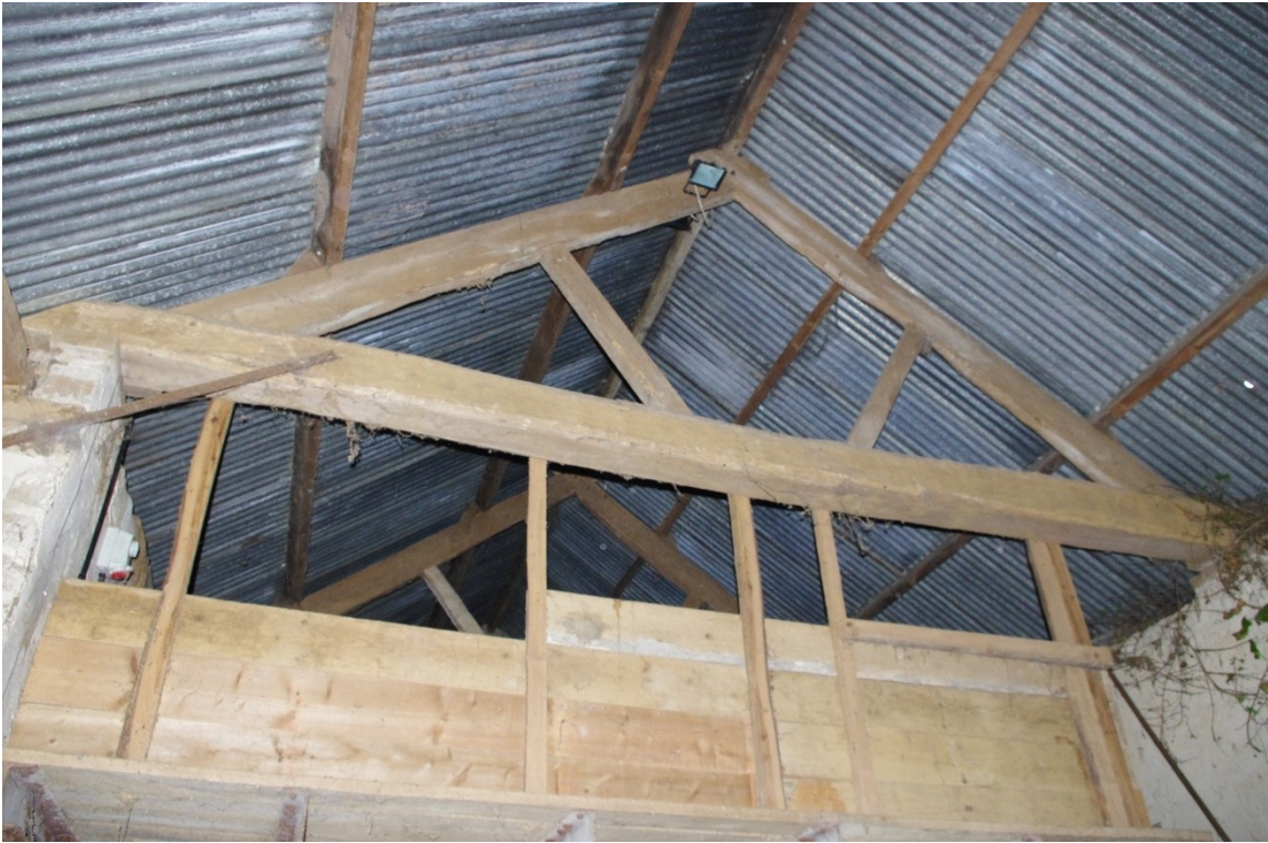
Figure 13 Truss Tr05 (looking West).
