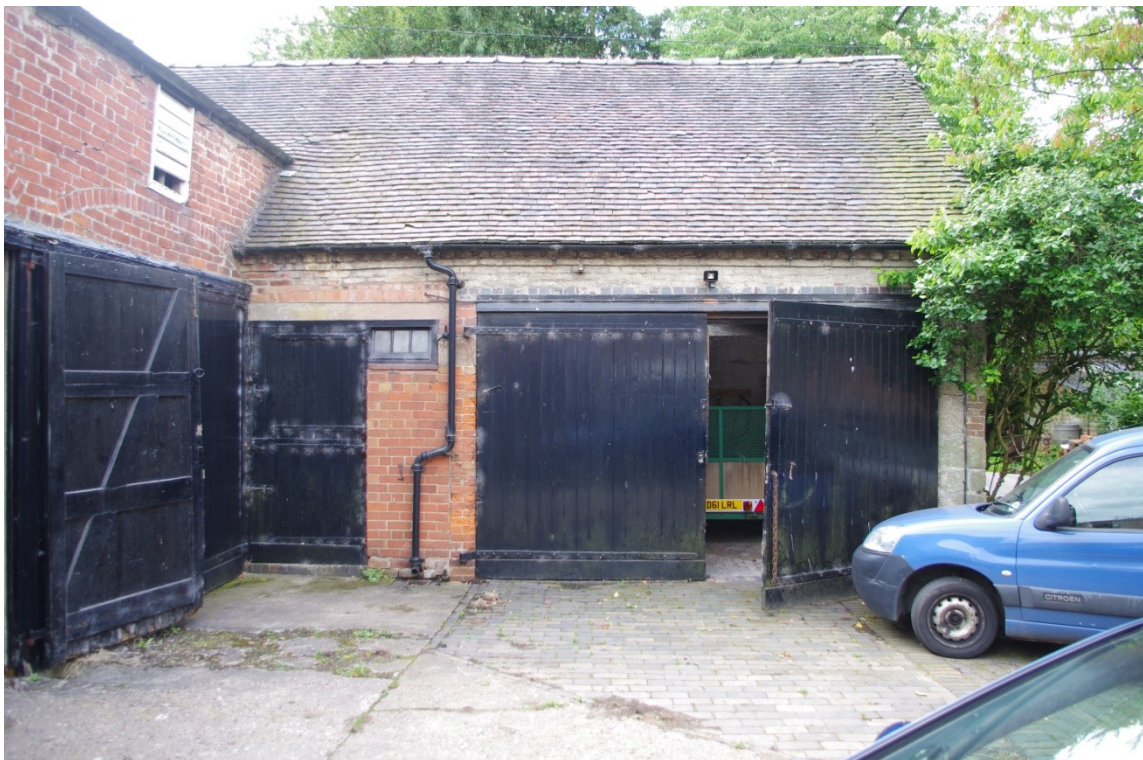
Figure 9 Principal Elevation D (looking South - South East).
