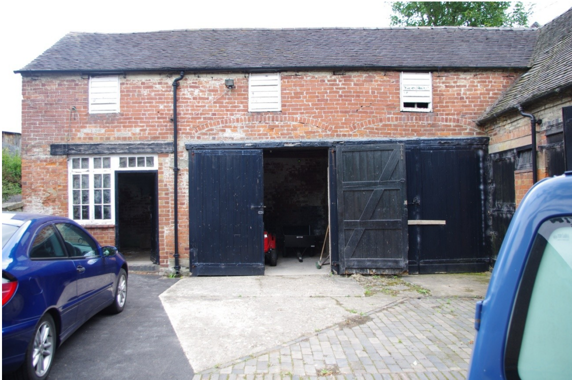
Figure 8 Principal Elevation A , B & C (looking West - North West).
