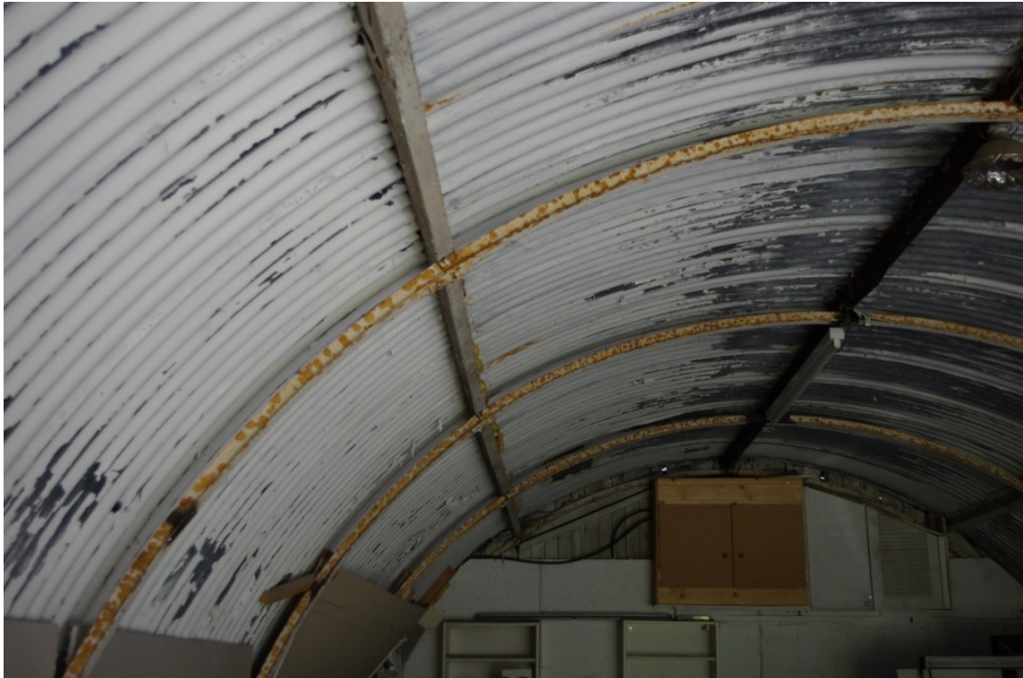
Figure 11 Visible Ribs & Purlins, Hut A .
