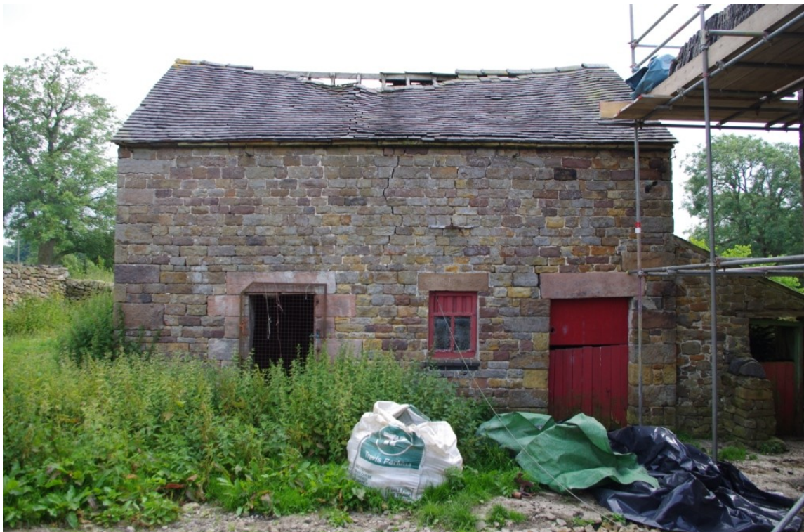
Figure 18 Building 02 Principal Elevation, General View (Looking East-South East).
