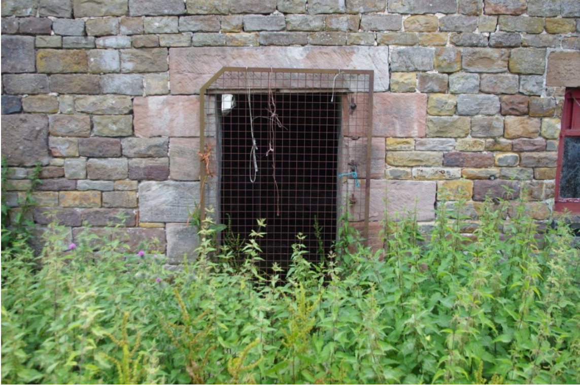
Figure 19 Building 02, Well Finished Quoins on Northernmost Door, Principal Elevation.
