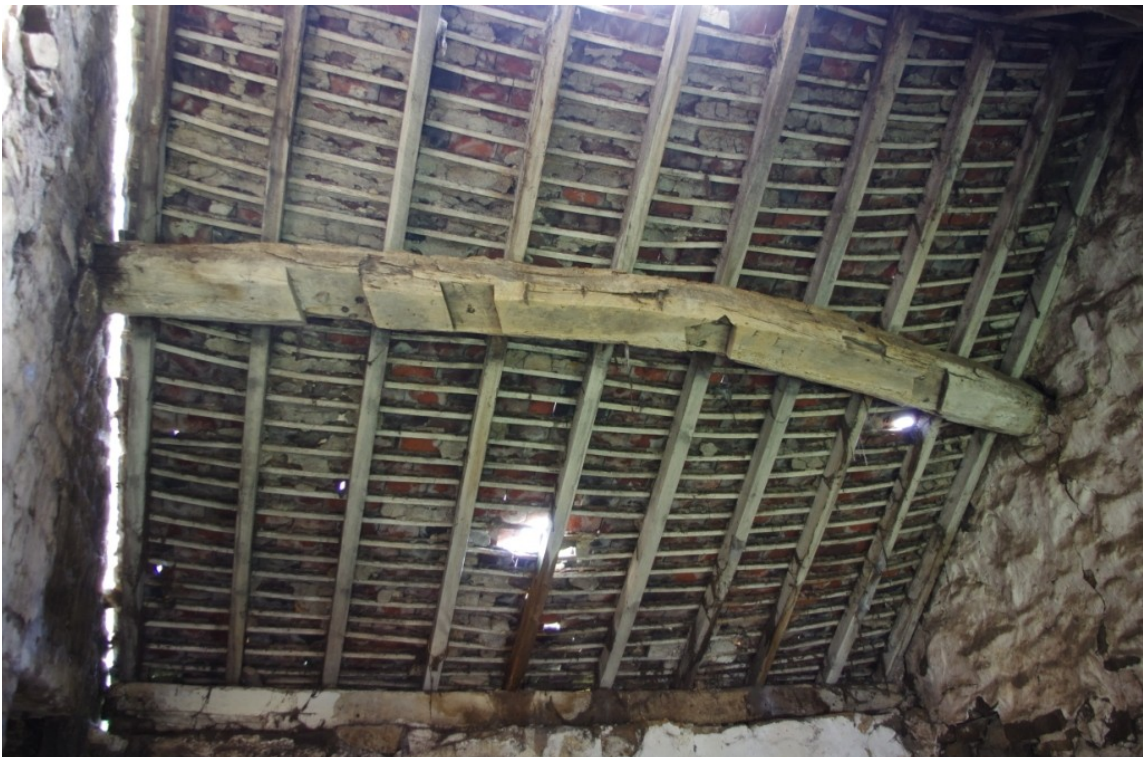
Figure 16 Building 01B, Possible Cruck Blade Re-used as a Purlin.
