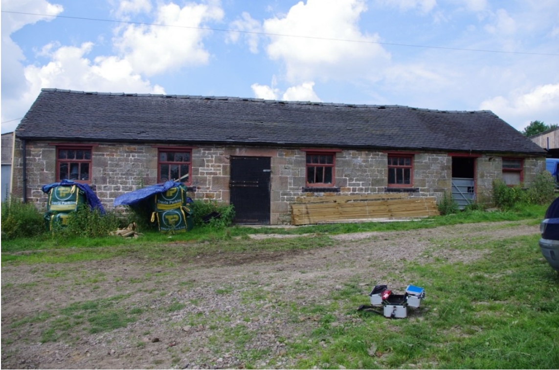
Figure 23 Building 03 Principal Elevation, General View (Looking West-North West).
