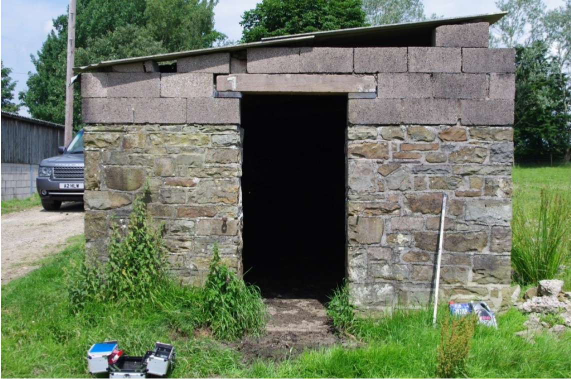
Figure 25 Building 04 General View of Southern Gable (Looking North).
