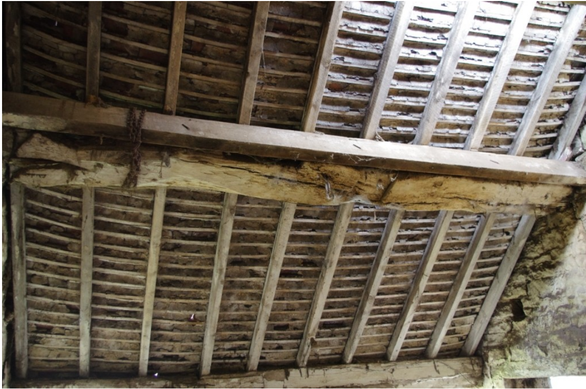
Figure 17 Building 01B, Bay Post Re-used as Purlin.
