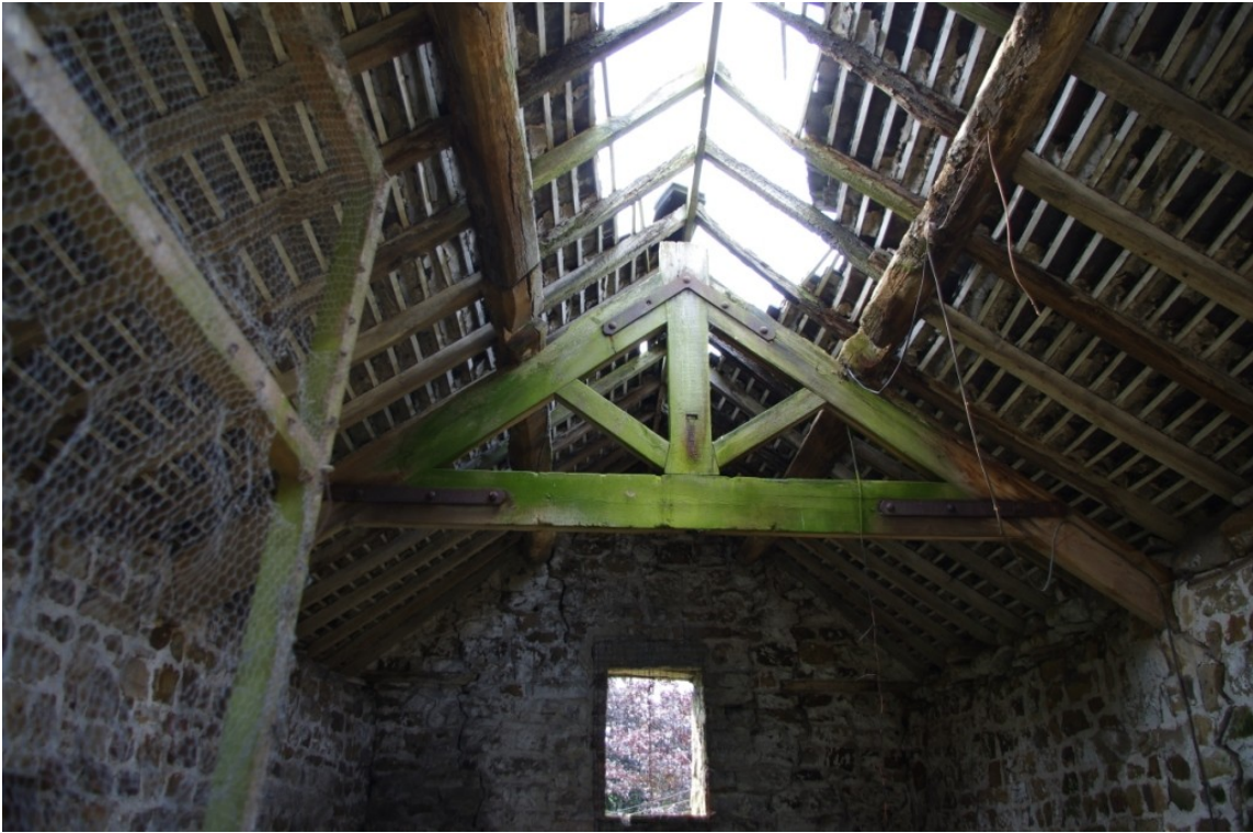
Figure 21 Building 02(A) Roof Truss.
