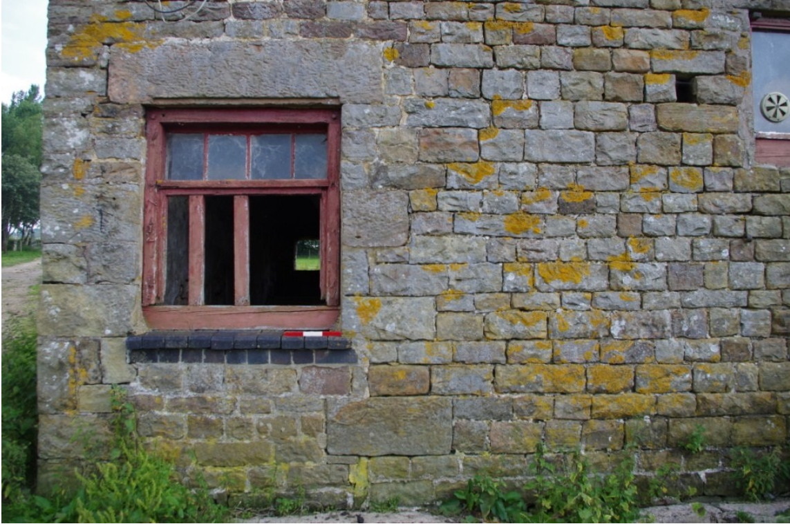
Figure 13 Building 01 Window Inserted into Blocked Doorway, Principal Elevation.
