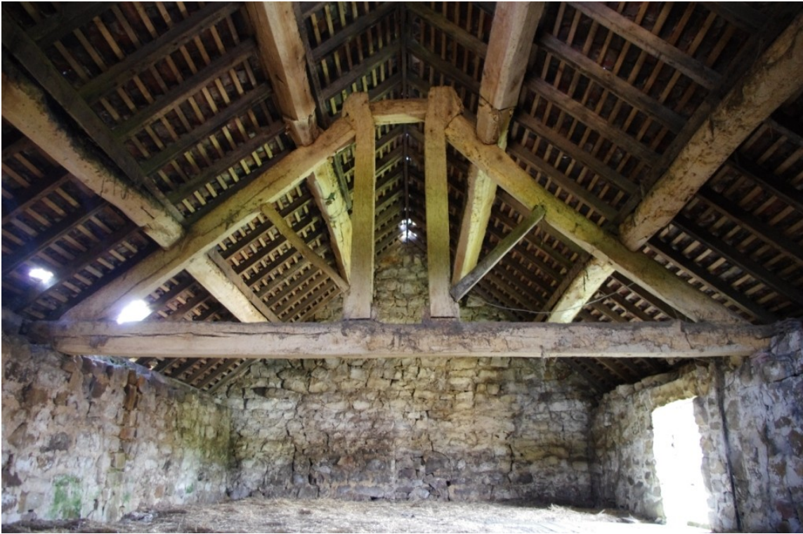
Figure 15 Building 01A Roof Truss.
