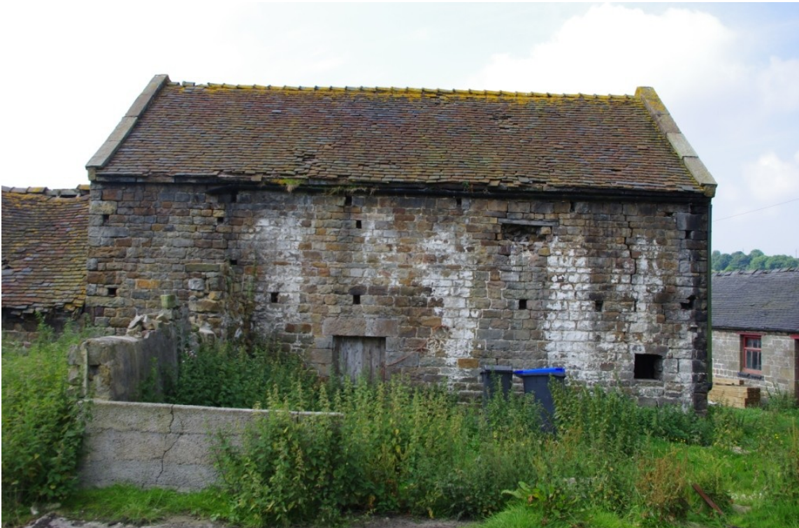
Figure 14 Building 01 Rear Elevation (Looking South-South West).
