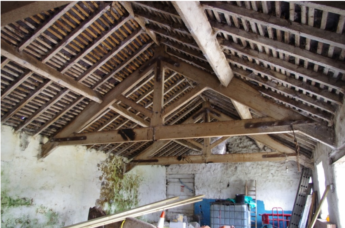
Figure 24 Building 03 Roof Truss.
