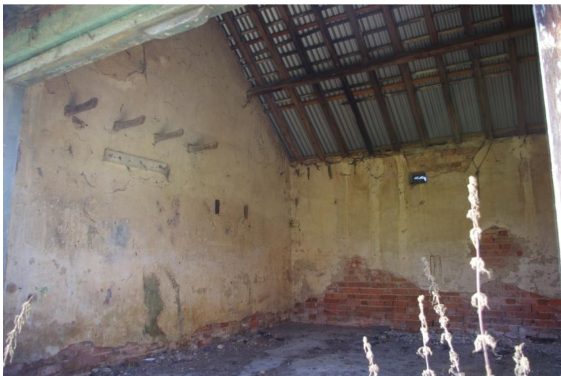
Figure 20 Building E (2) Rendered Finish & Saddle Tree on South Wall.
