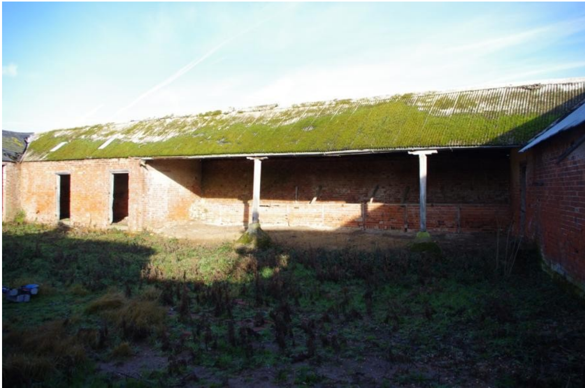
Figure 6 Building A Principal Elevation (looking North – North West).
