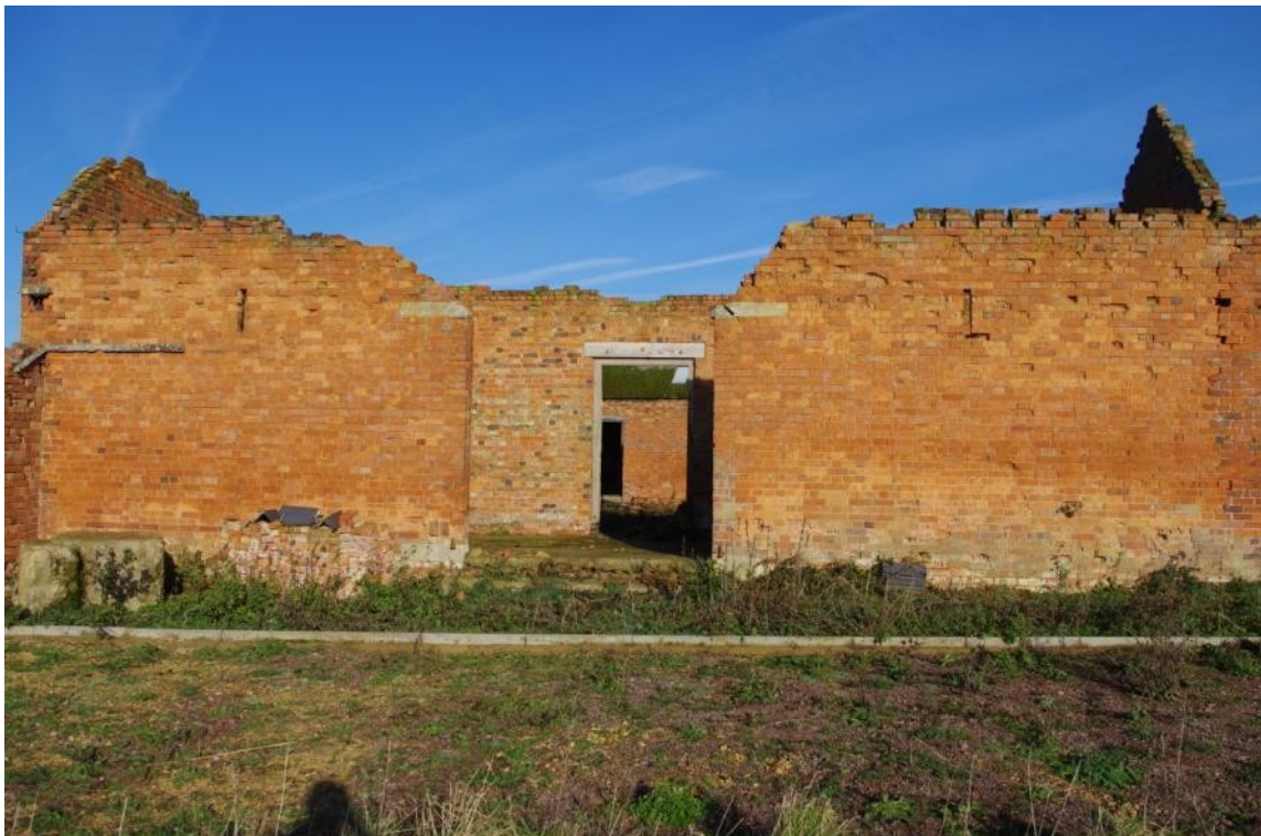
Figure 9 Building D South Facing Elevation (looking North East).
