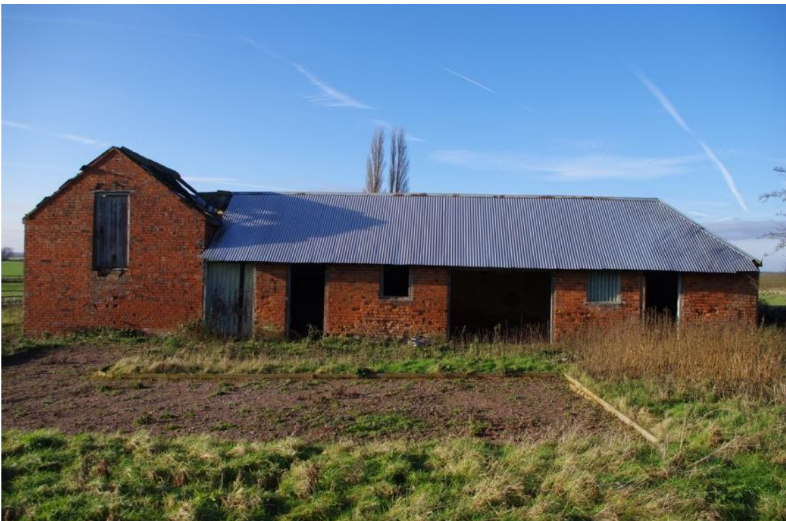
Figure 11 Building E Principal Elevation (looking West – North West).
