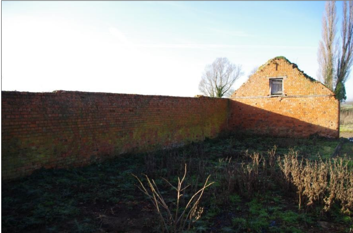
Figure 8 Building C General View (looking West – South West).
