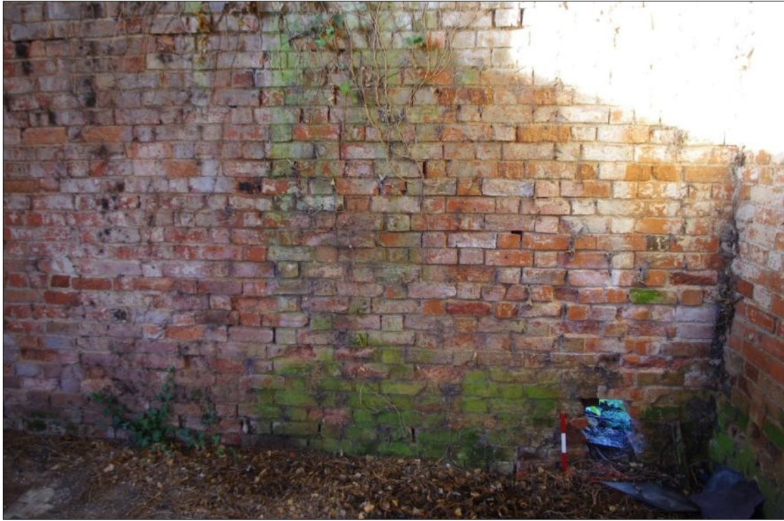
Figure 16 Building B (3) Inserted Opening for Poultry at Ground Level in Rear Wall.
