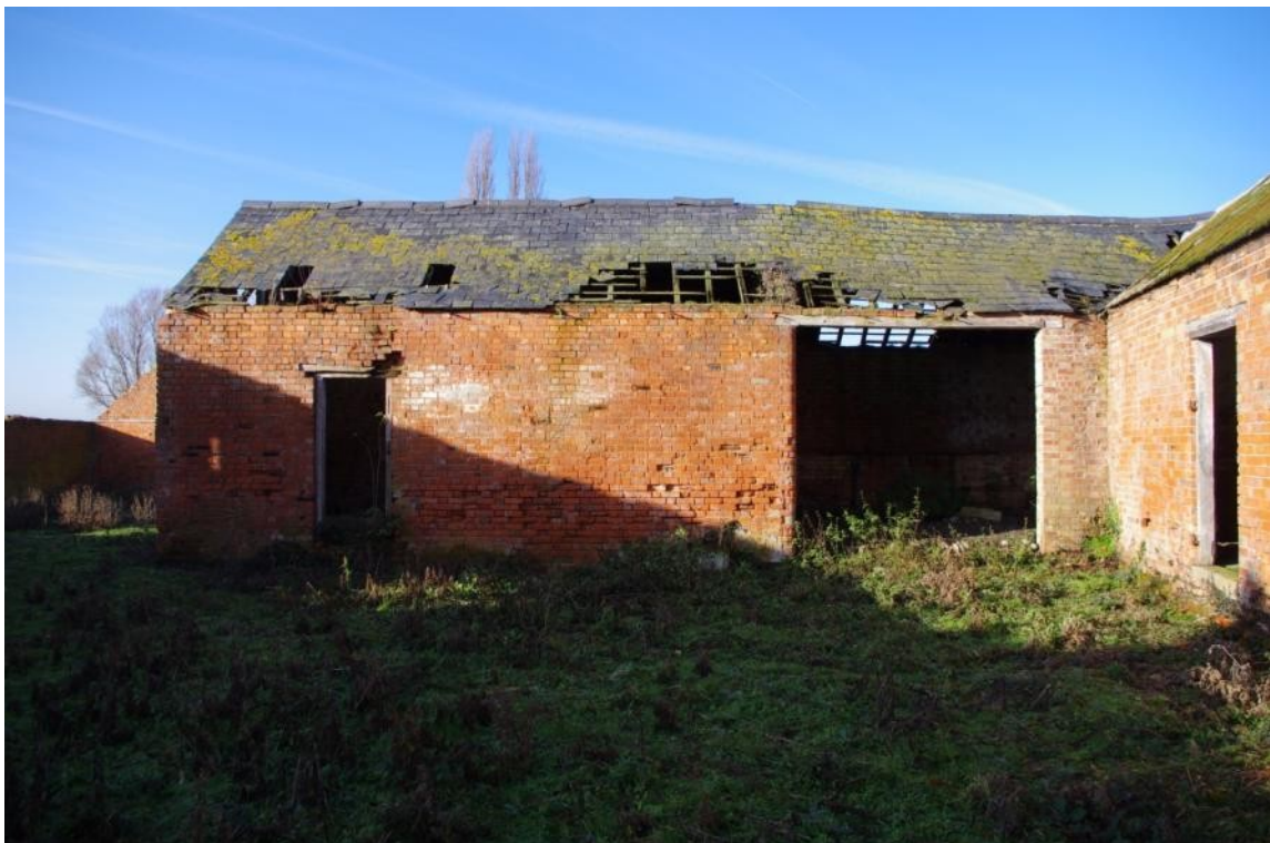
Figure 7 Building B Principal Elevation (looking West – North West).
