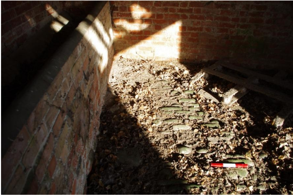
Figure 14 Building B (1) Pitched Stone Floor & Brick-Built Manger.
