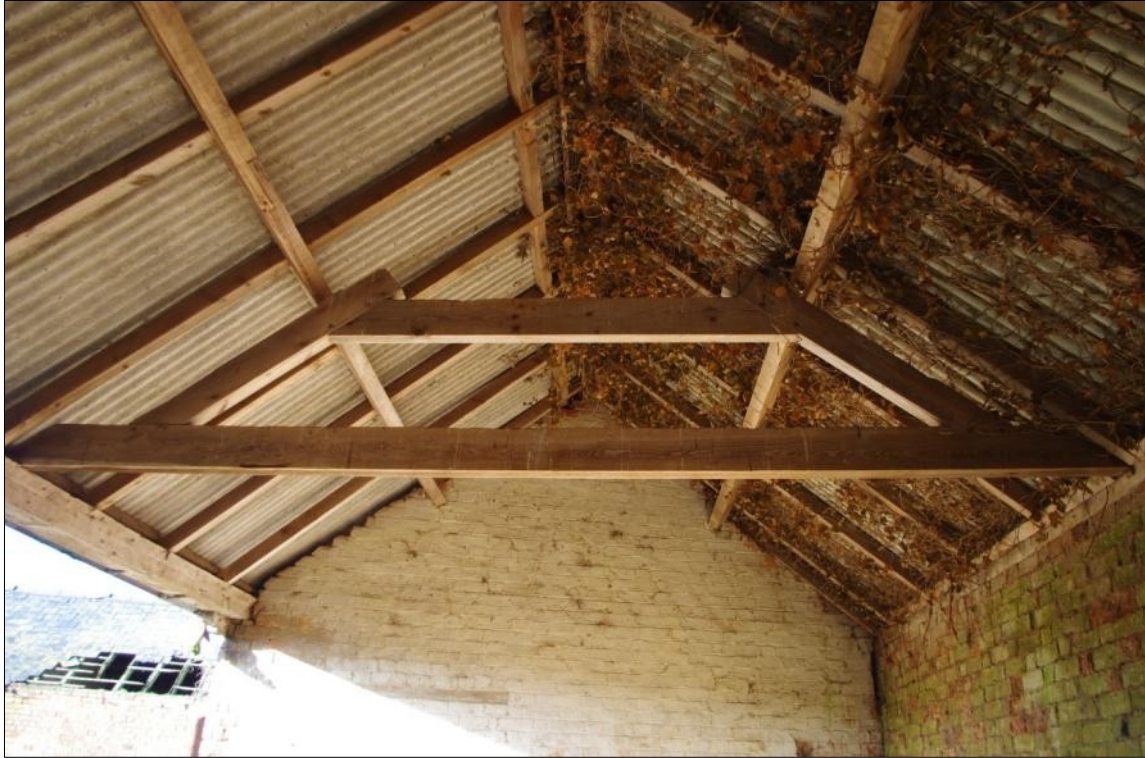
Figure 12 Building A Truncated Principal Rafter Truss.
