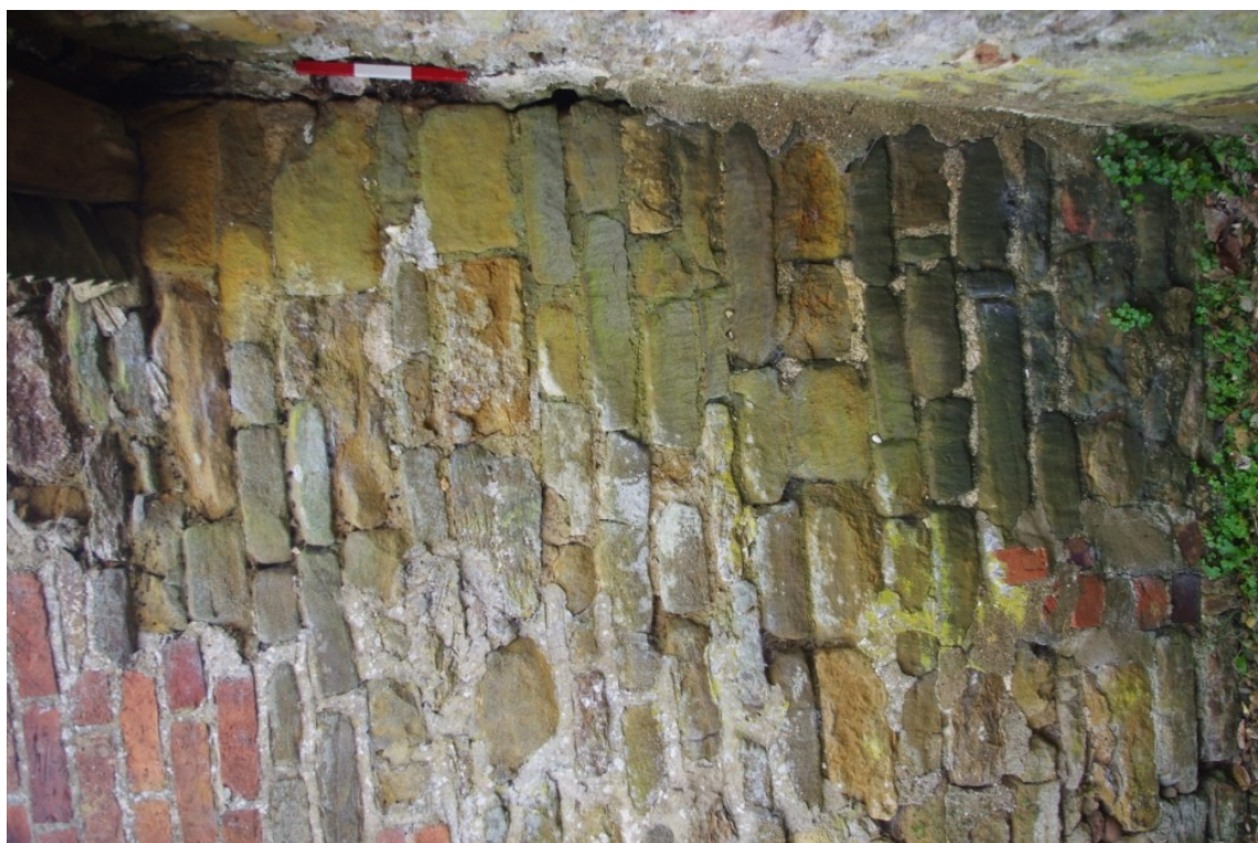
Figure 14 Building B Quoined South West Corner.
