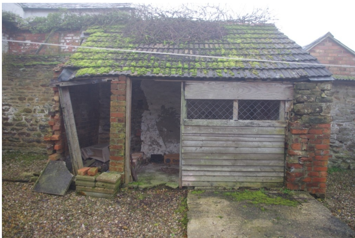
Figure 12 Building B North Facing Elevation, General View (Looking South).
