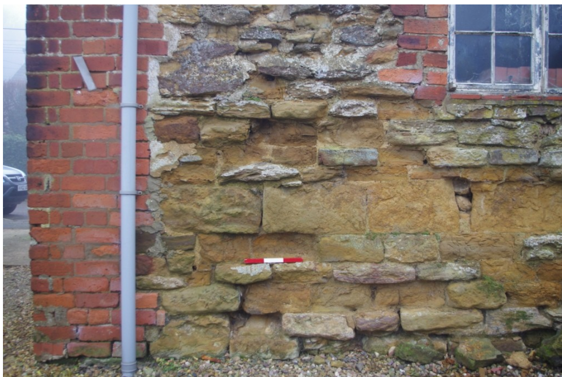
Figure 10 Building A Ashlar Blocks & Narrow Courses on West Facing Elevation.
