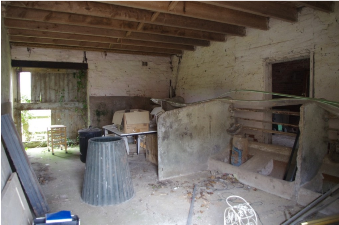
Figure 11 Building A (2) Concrete Stalls & Feed Passage on East Wall.
