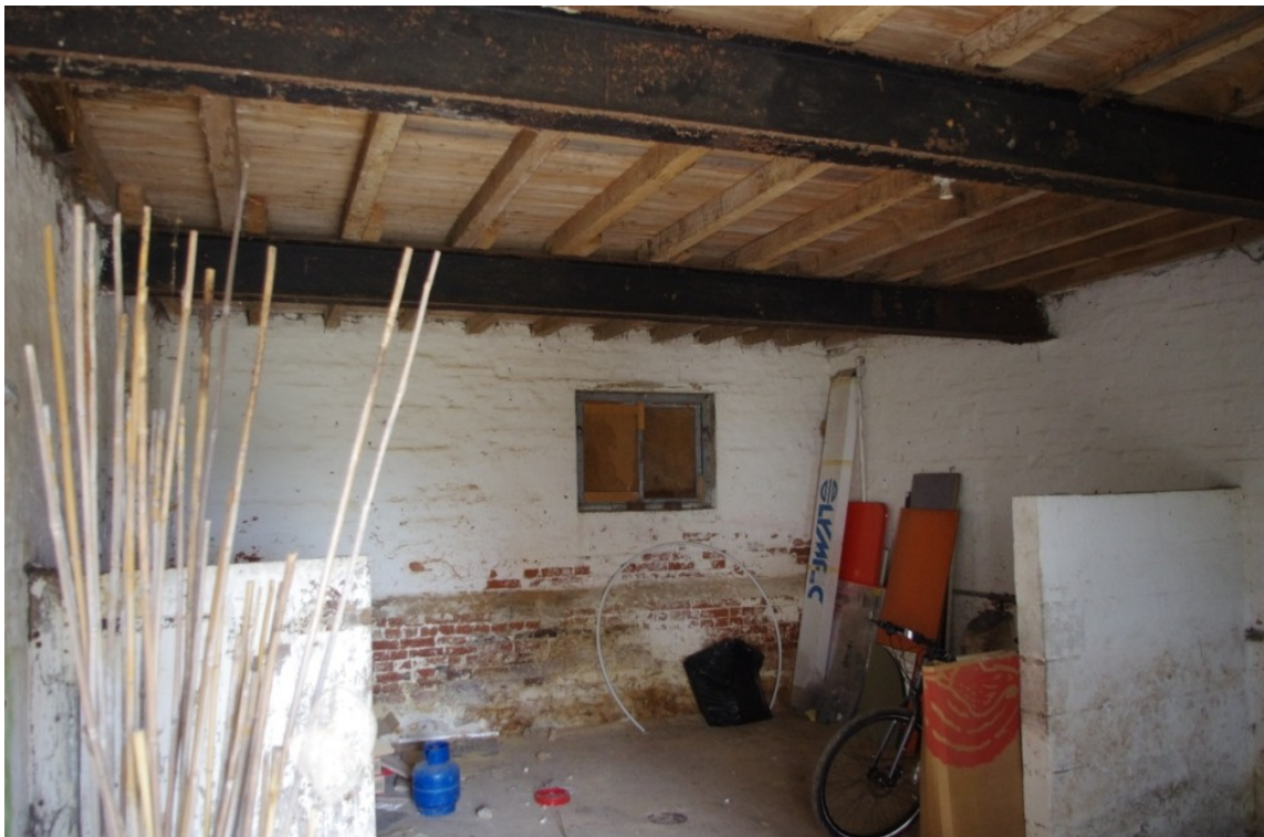
Figure 12 Building A (1) General View & RSJ Bridging Beams (Looking North-North East).
