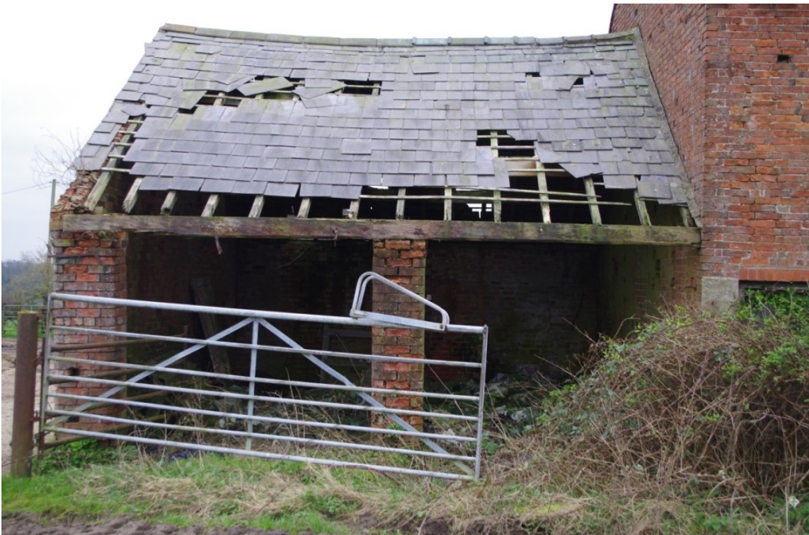
Figure 16 Building C Principal Elevation (Looking South).
