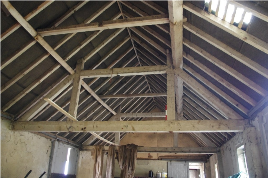
Figure 15 Building B (2) Queen Post Truss.
