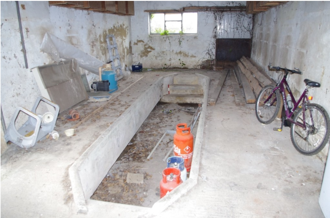
Figure 14 Building B (1) Sunken Milking Floor (Looking North West).
