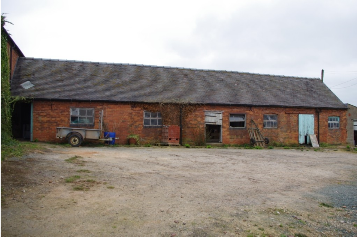
Figure 13 Building B Principal Elevation (Looking East).
