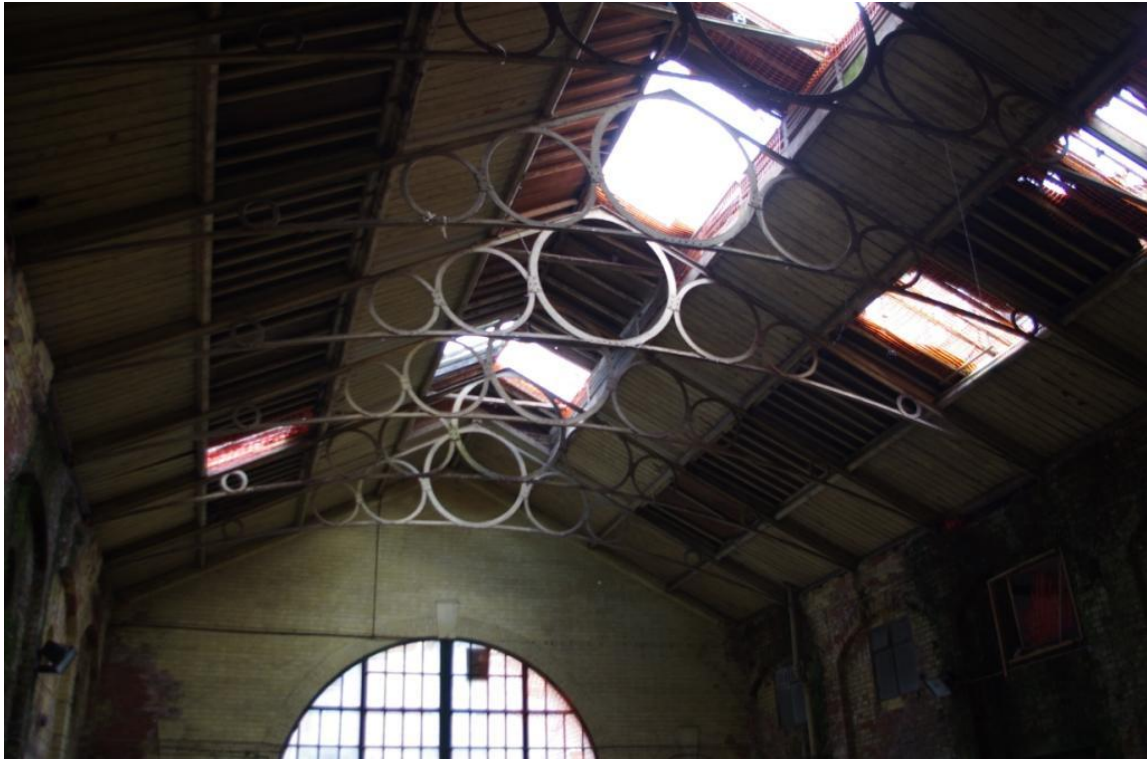
Figure 10 (1) Diminishing Hoop Cast Iron Truss.
