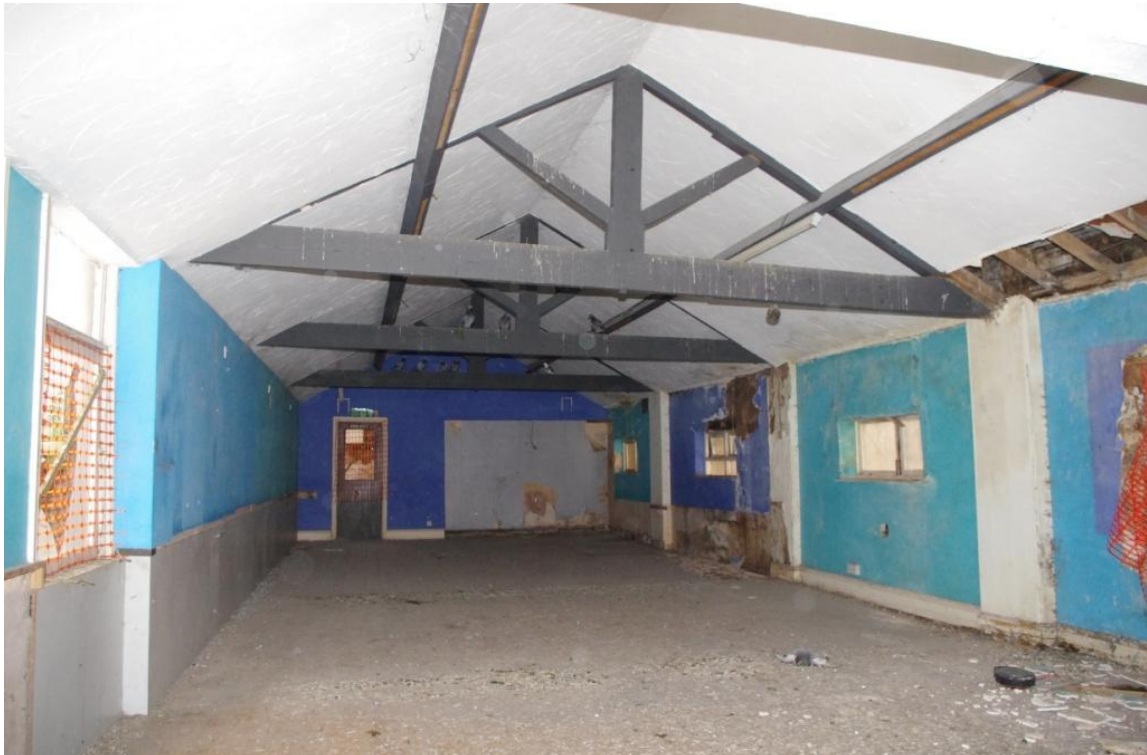
Figure 17 (3) First Floor, General View & King Post Roof Truss (Looking West).
