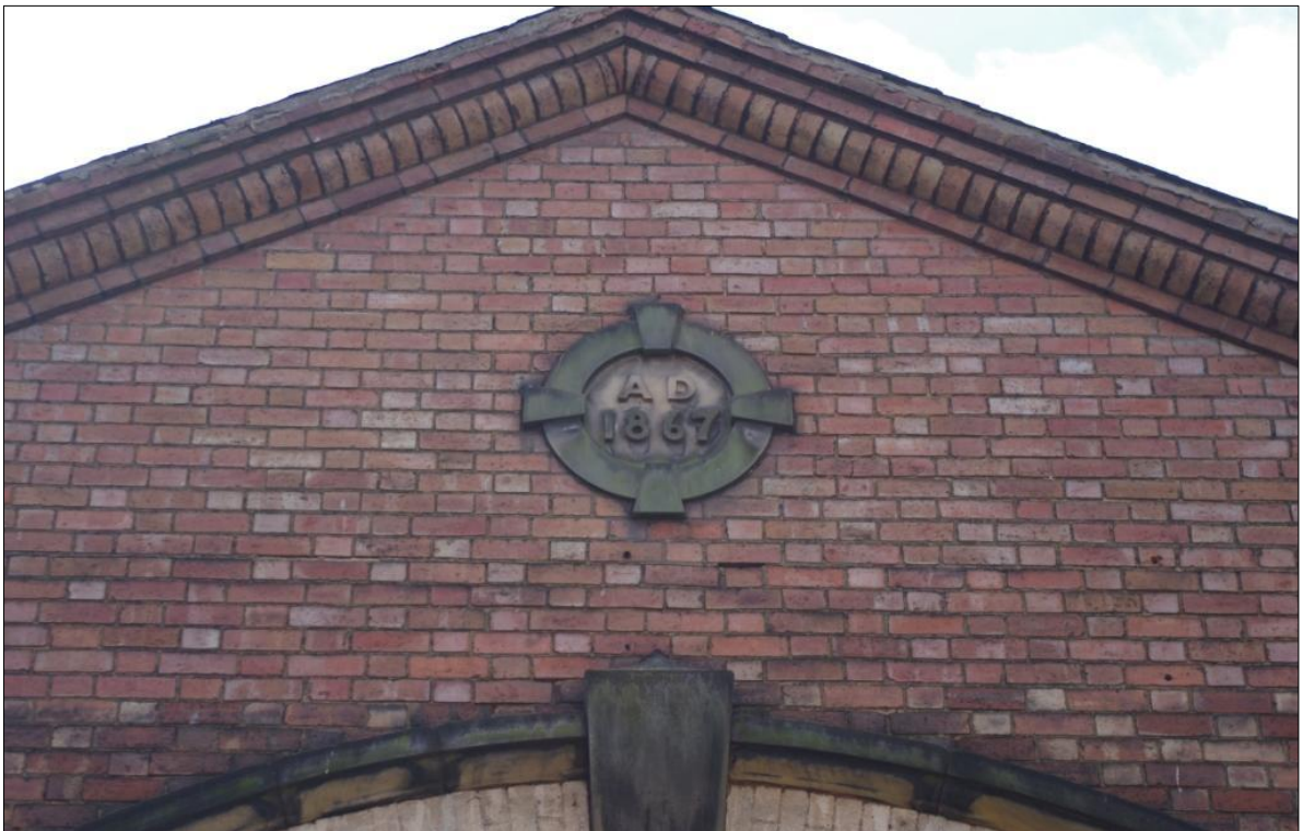
Figure 7 (1) Date Stone on Principal Elevation.
