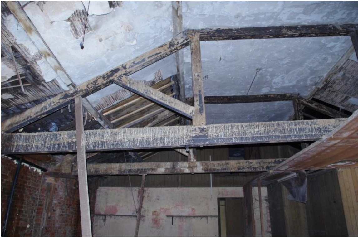
Figure 16 (2) Queen Post Roof Truss.
