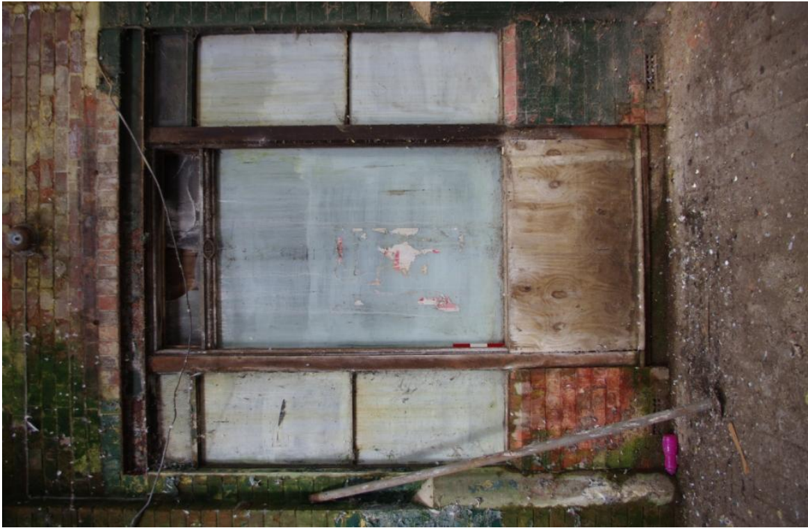
Figure 12 (1) Early Glazed Opening on North Wall (Looking North).
