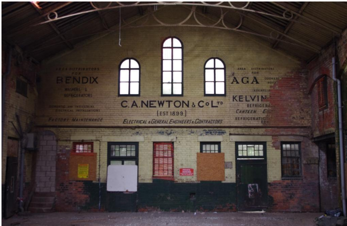
Figure 11 (1) East Facing Gable, Internal with Signage & Windows.
