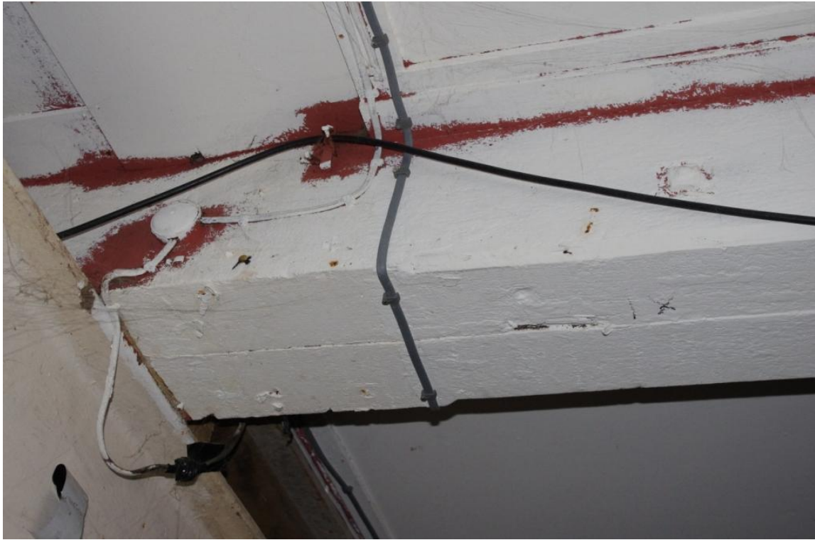
Figure 14 (2) Chamfered & Stopped Joist.
