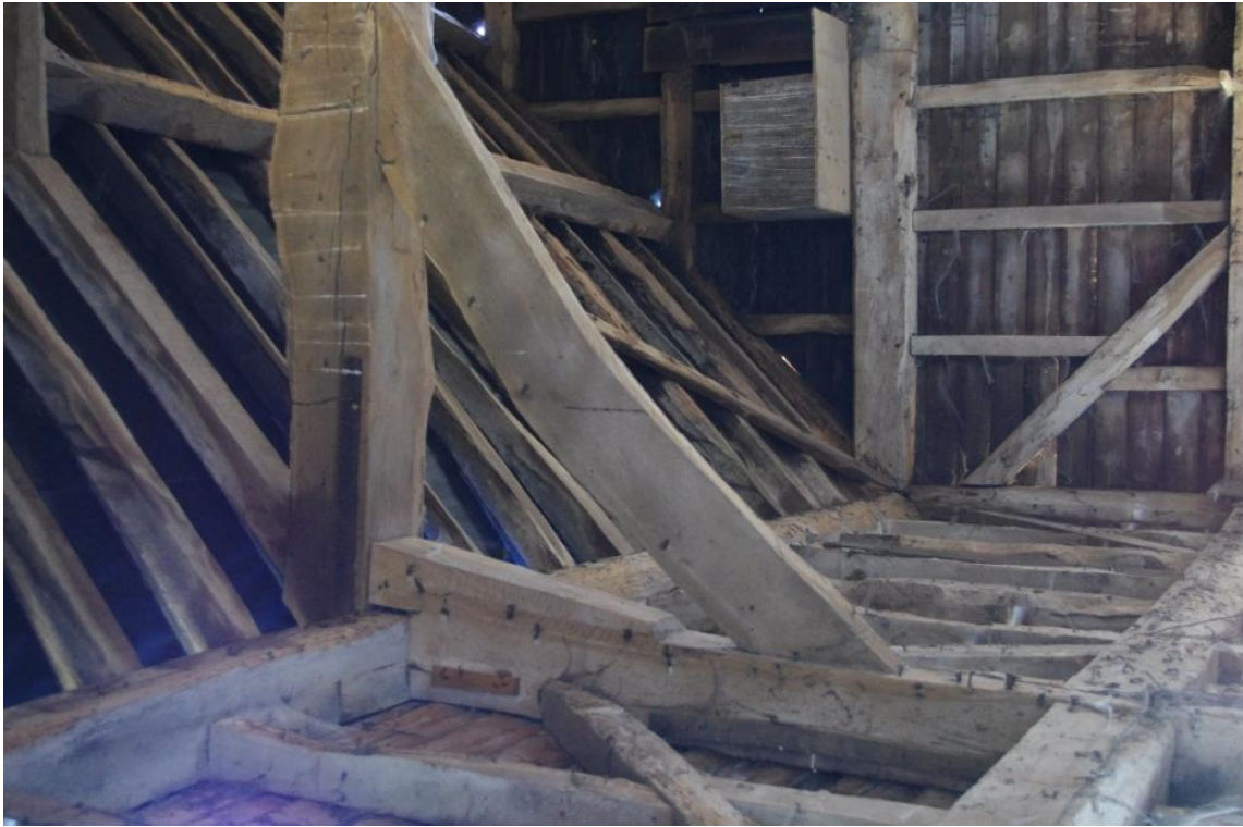
Figure 11 Concave Brace Between Bay Post & Tie Beam.
