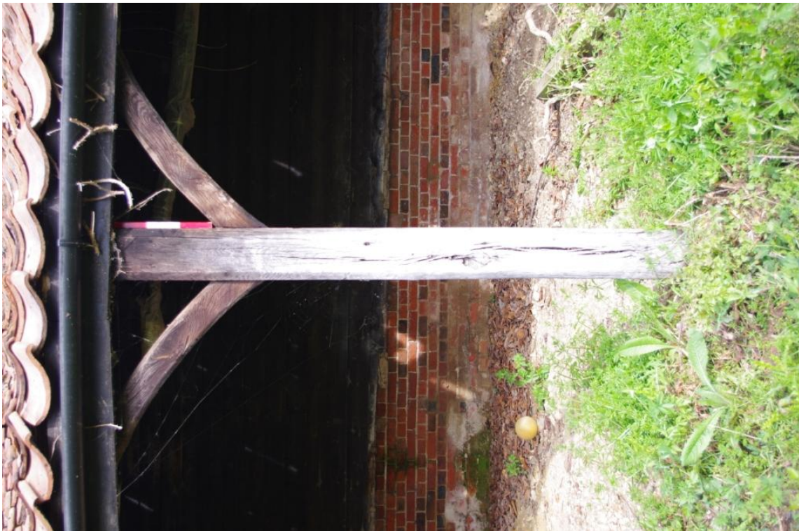
Figure 10 Concave Braces on Shelter Shed, South East Facing Elevation.
