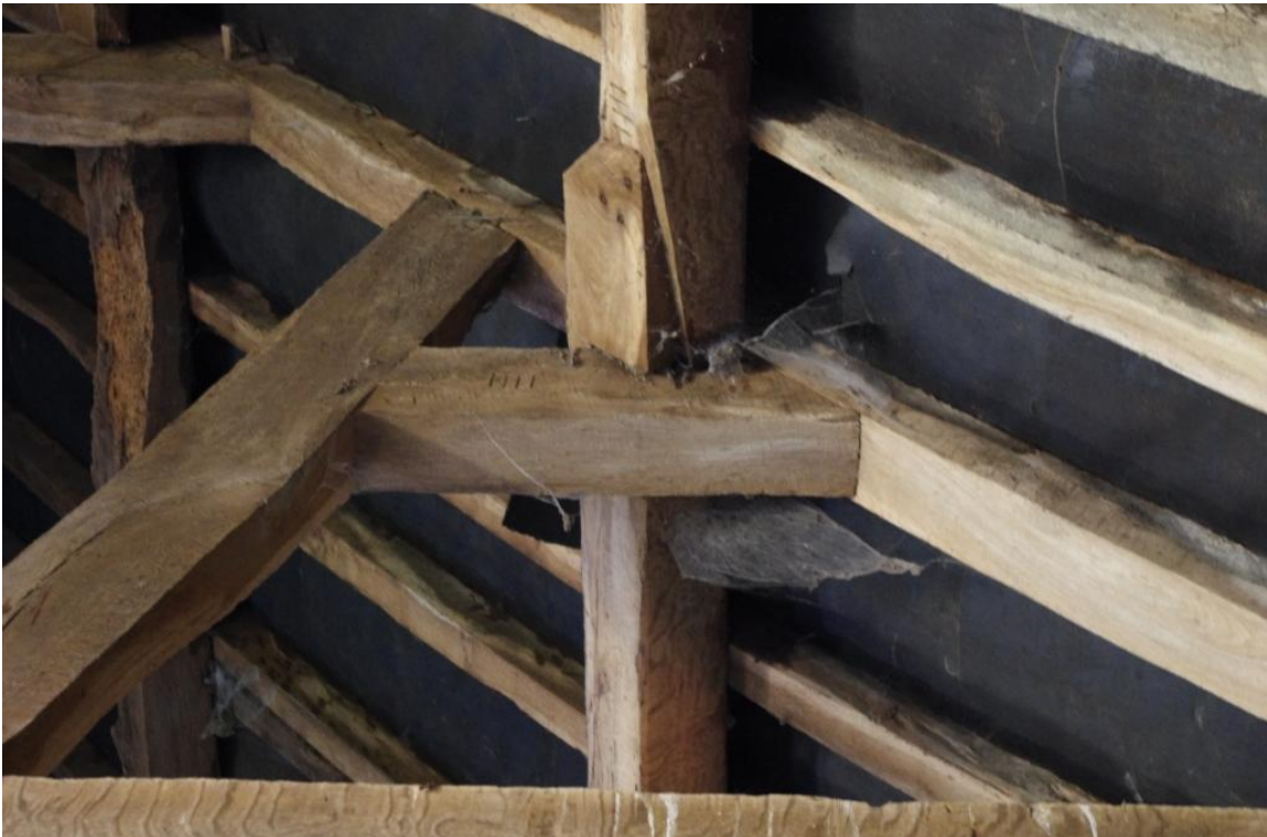
Figure 16 Interrupted Collar Beam & Clasped Purlin.
