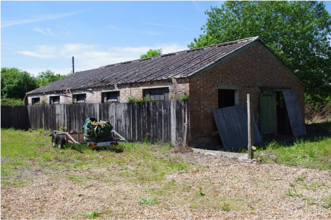
Figure 19 Building B , General View (Looking West – South West).
