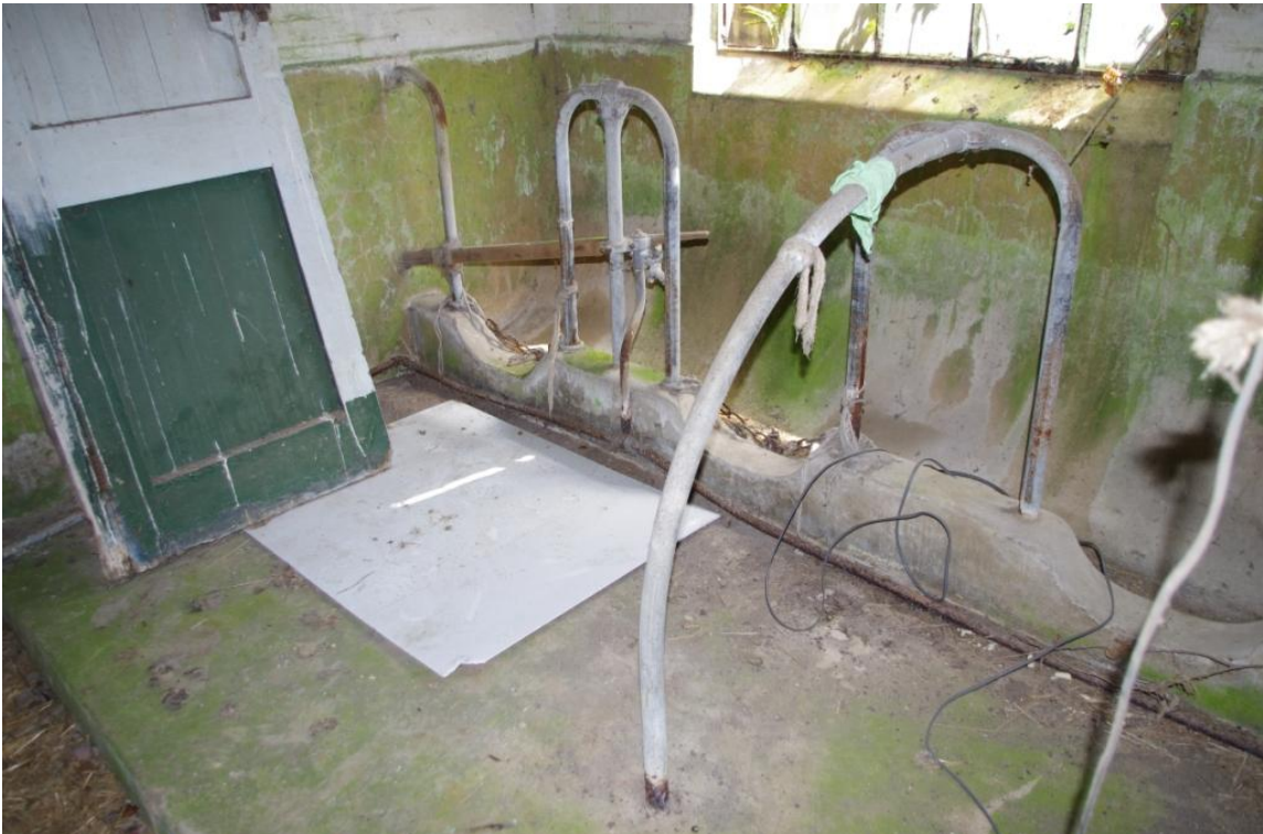
Figure 20 Building B Concrete & Steel Stalls.
