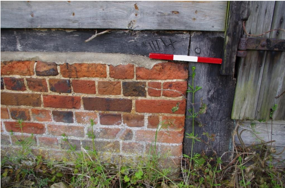
Figure 14 Assembly Marks on Sill Beam, External View.
