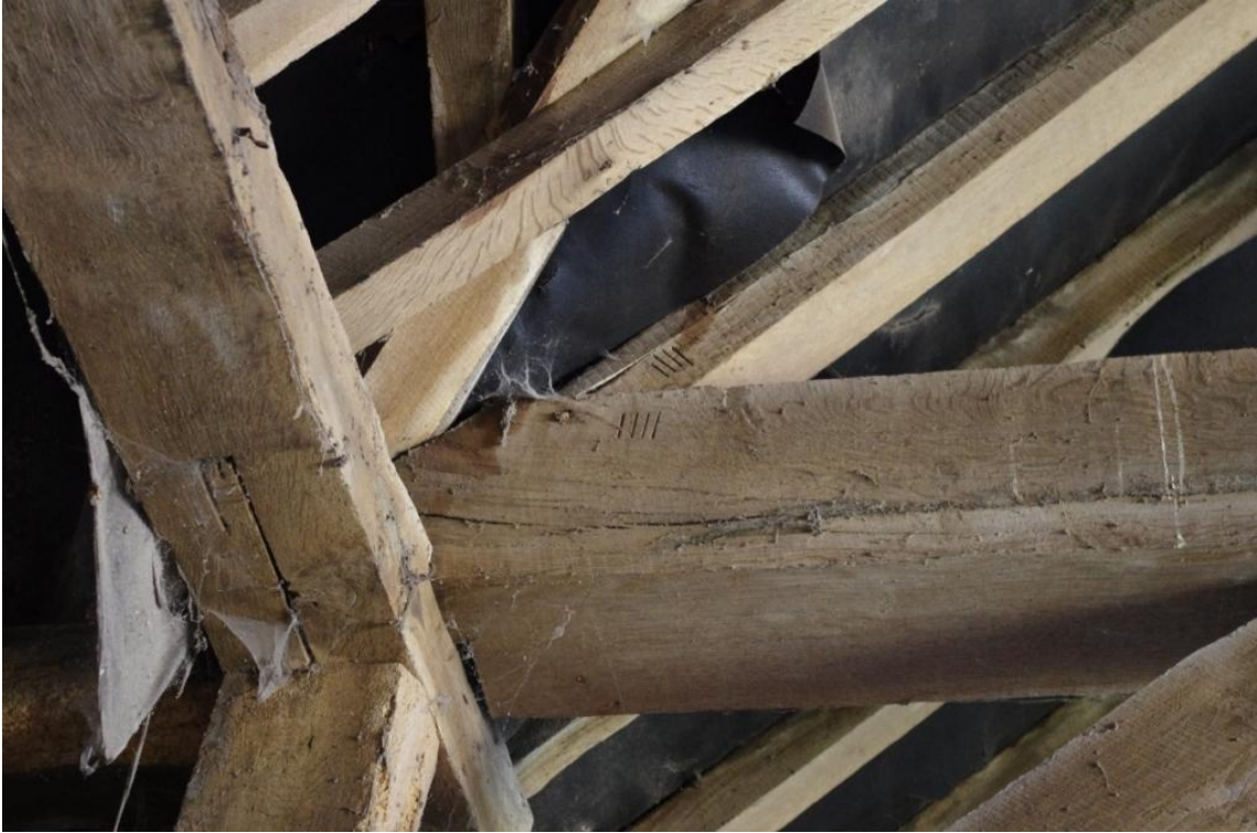
Figure 17 Assembly Marks on Truss.
