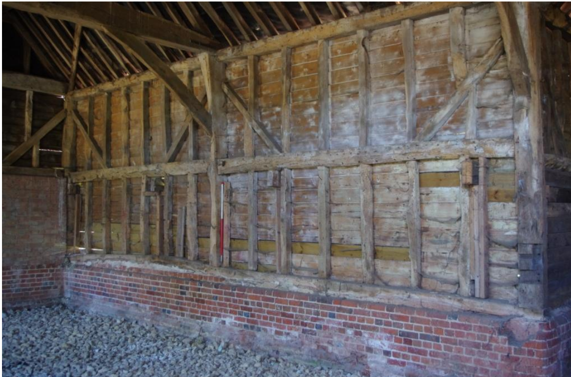
Figure 12 Wall Studding, Internal Wall (Looking East).
