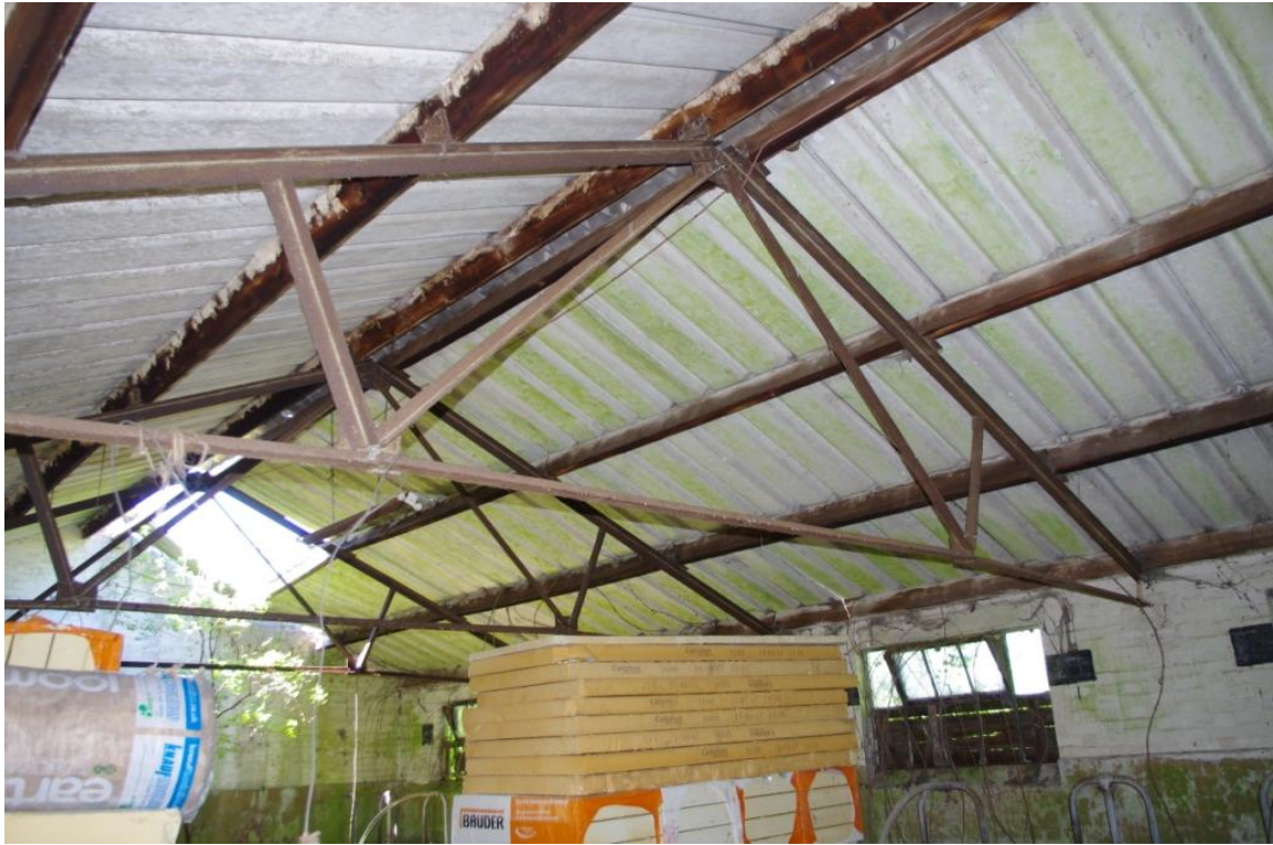
Figure 21 Building B Roof Trusses.
