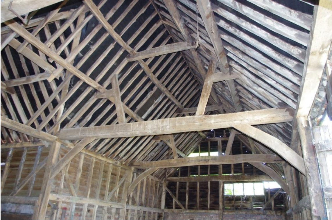
Figure 15 Truss, General View (Looking South West).
