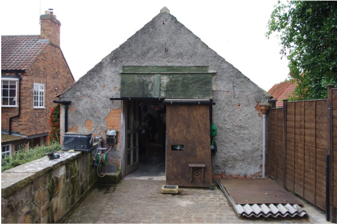
Figure 11 Building A (2) East Facing Gable Showing Modified Cart Door.
