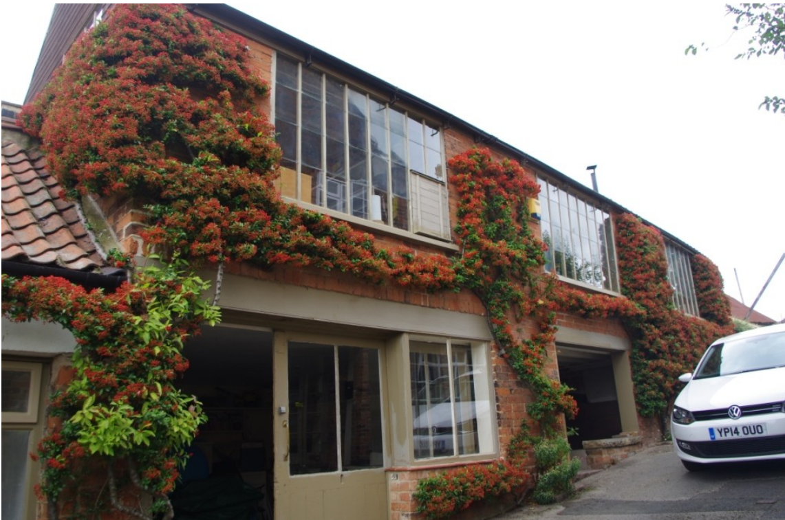
Figure 10 Building A (2) Principal Elevation, Showing Weavers Windows at First Floor Level (Looking North East).
