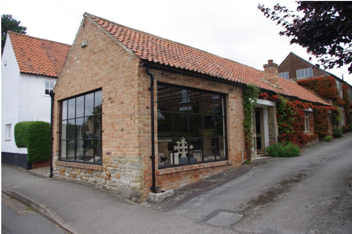
Figure 7 Building A (1) General View (Looking North-North East).
