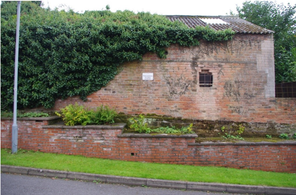
Figure 20 Building B (1) Rear Elevation, Showing Early/Original Brickwork (Looking South-South East).
