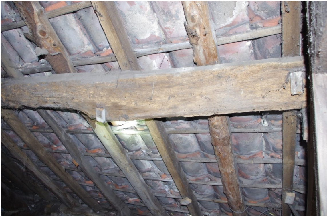
Figure 18 Building A (1) Hardwood Purlin and Wood & Deal Common Rafters (Looking South).
