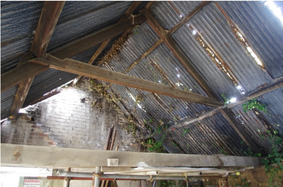
Figure 22 Building B (2) Roof Truss.
