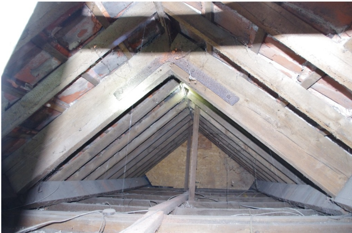
Figure 14 Building A (2) Roof Structure (Looking West-South West).
