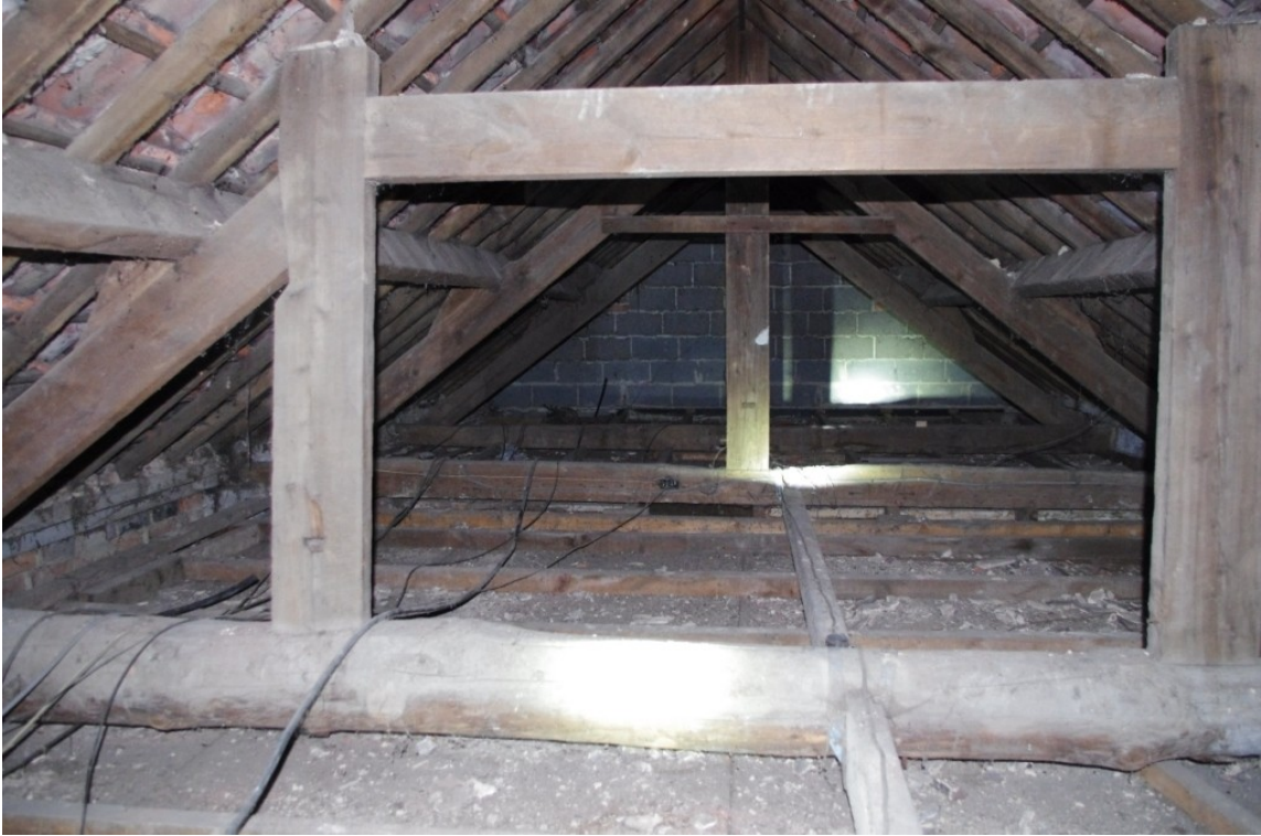
Figure 15 Building A (1) Tr02 King Post Truss (Looking West-South West).
