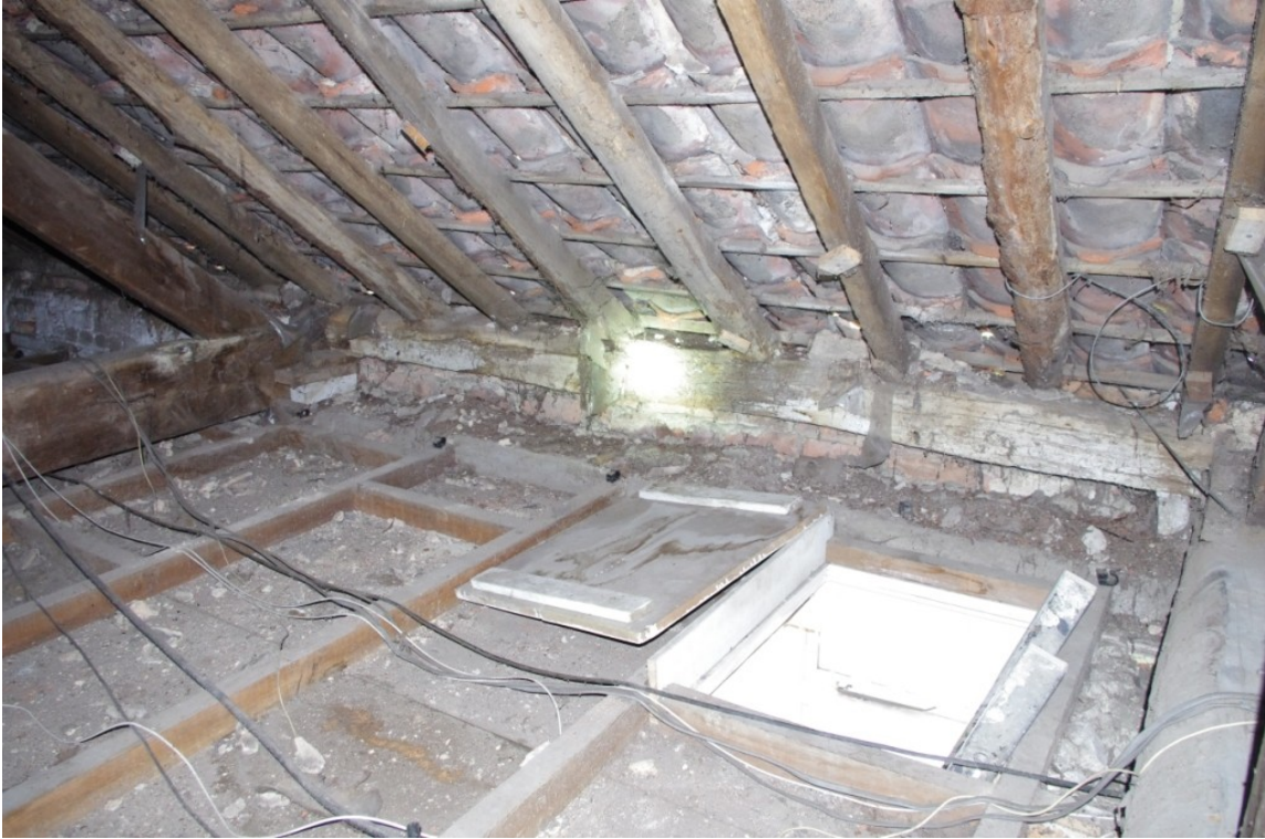
Figure 19 Building A (1) Wall Plate Visible Internally on Principal Elevation (Looking South).
