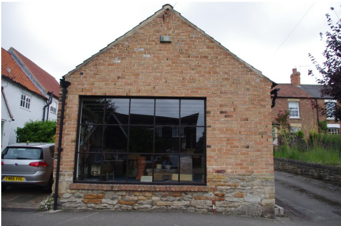
Figure 8 Building A (1) Main Street Gable Showing Stone Courses.
