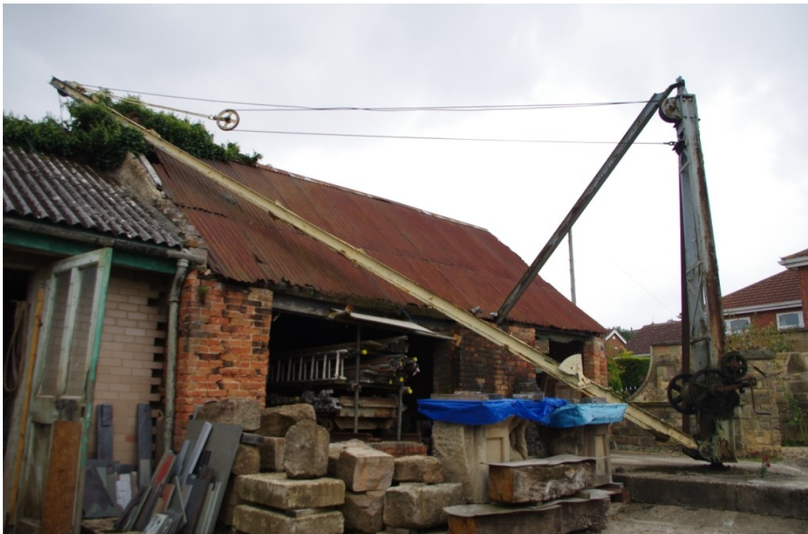
Figure 24 Crane, Building B (2) in the Background (Looking North East).
