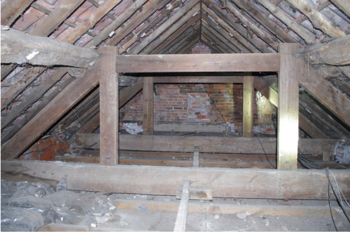
Figure 17 Building A (1) Tr05 Queen Post Truss with Deal Tie Beam (Looking East-North East).
