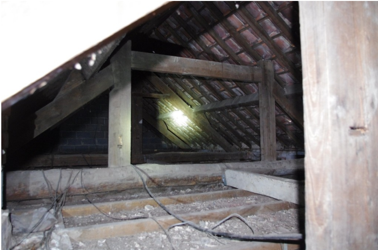
Figure 16 Building A (1) Tr03 Queen Post Truss with Poorly Finished Tie Beam (Looking West).
