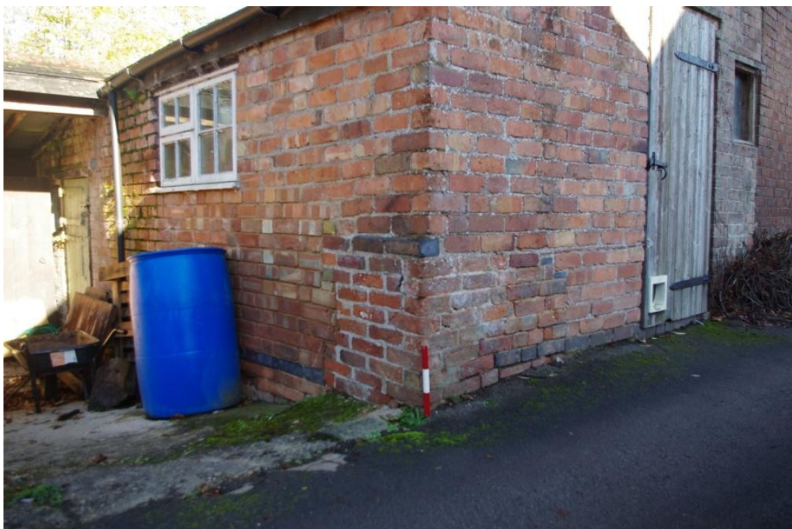
Figure 15 Building D Multiple Brickwork Phases on South & West Facing Elevations.
