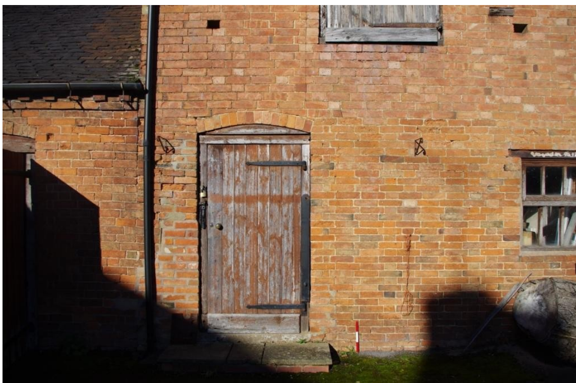
Figure 10 Building A Multiple Brickwork Phases on Principal Elevation.
