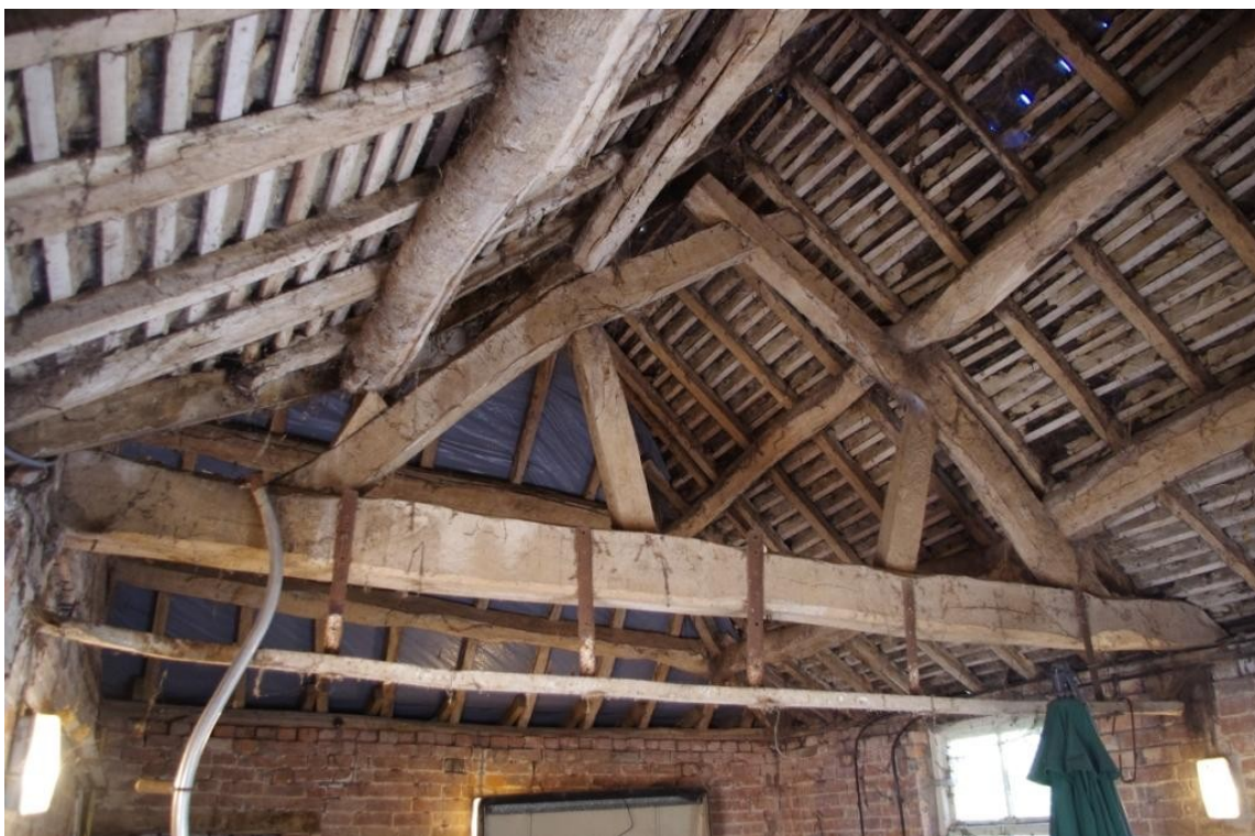
Figure 14 Building B (2) Roof Truss.
