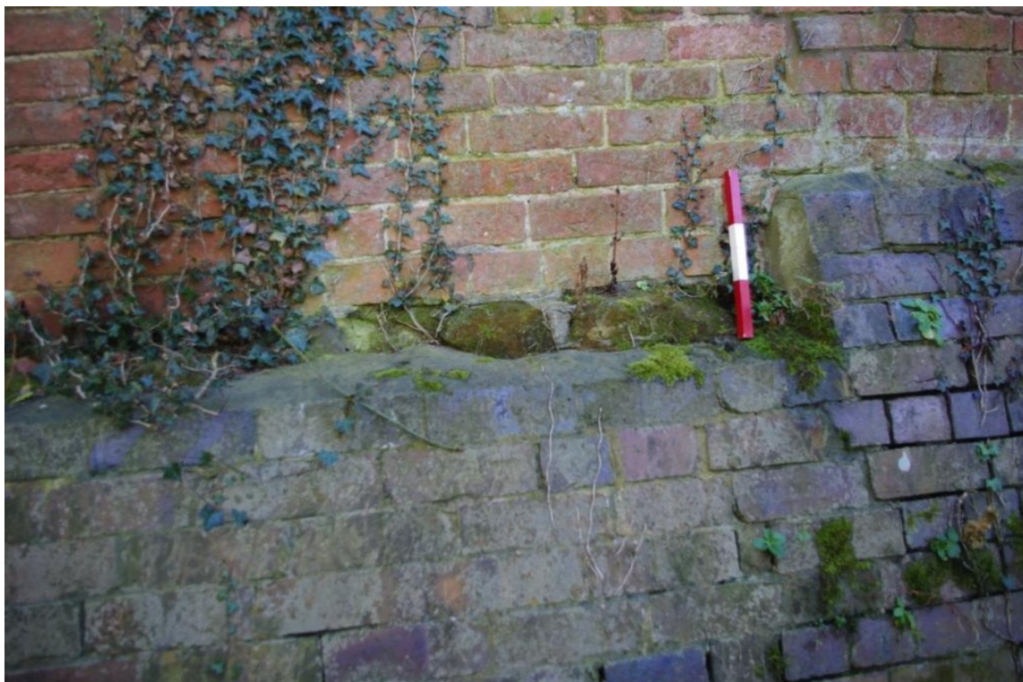
Figure 9 Building A Blue Brick Revetment & Earlier Stone Footing.
