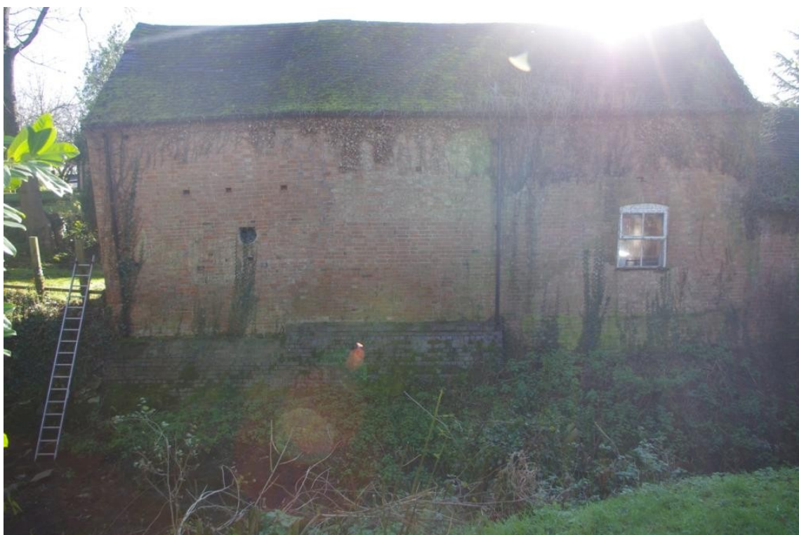
Figure 8 Building A Rear Elevation (Looking South – South East).
