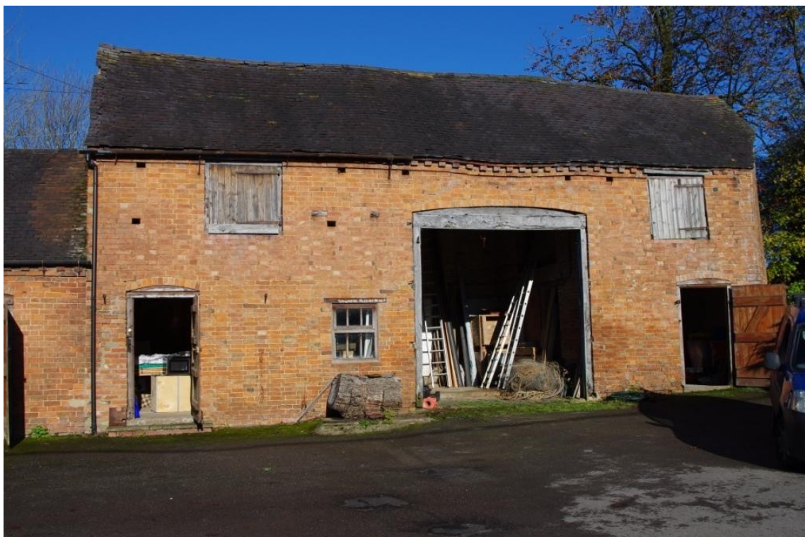
Figure 7 Building A Principal Elevation (Looking North – North West).
