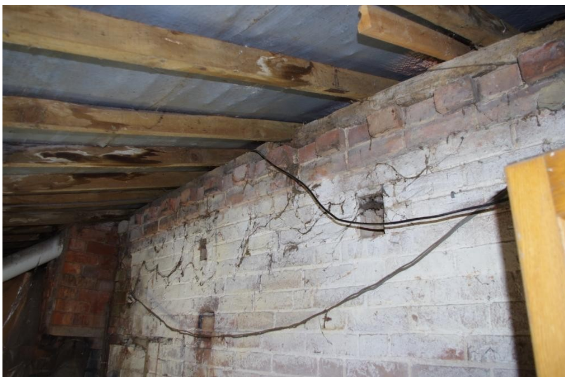
Figure 16 Building D Corbelling on Easternmost Wall.
