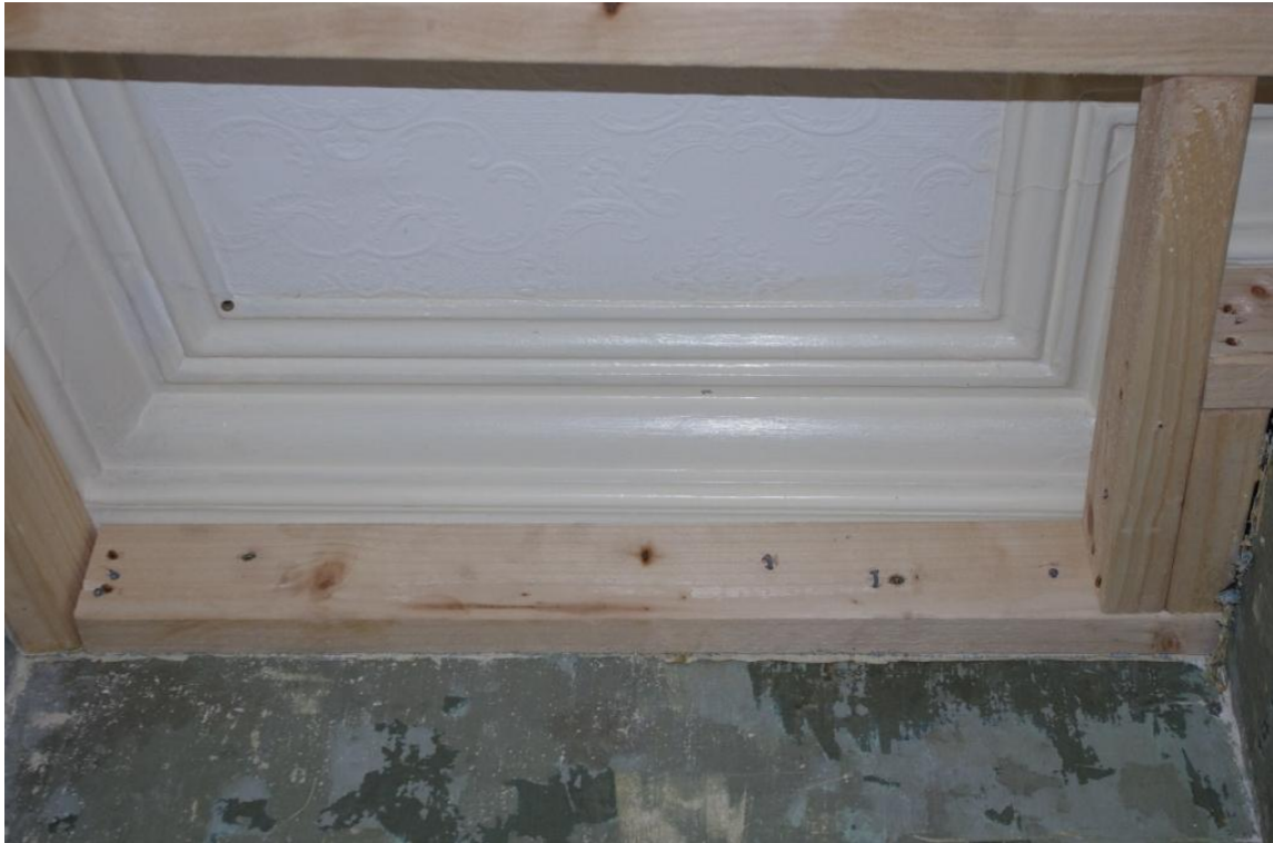
Figure 14 (F) Plaster Ceiling Cornice Adjacent to Chimney Breast.
