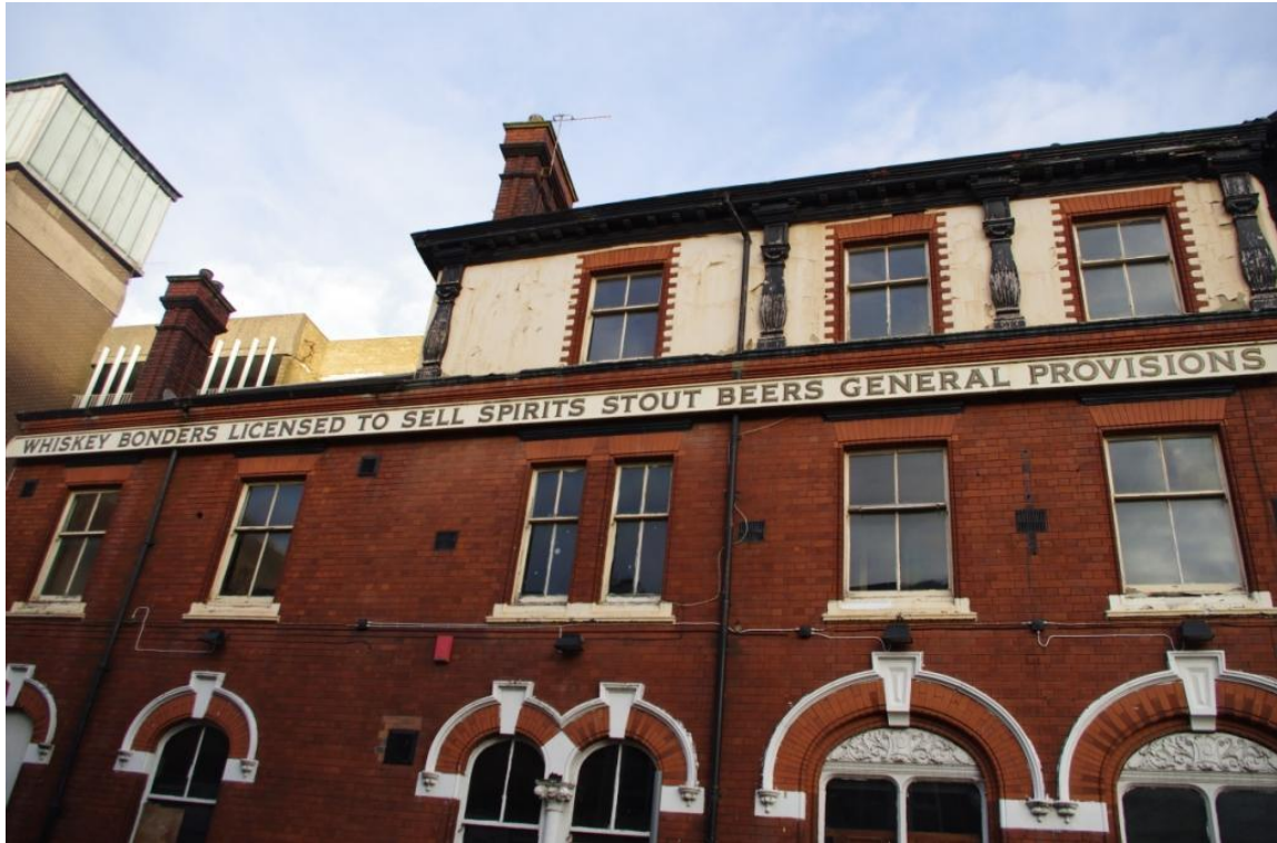
Figure 10 Signage on Goodson Street Elevation (Looking North East).
