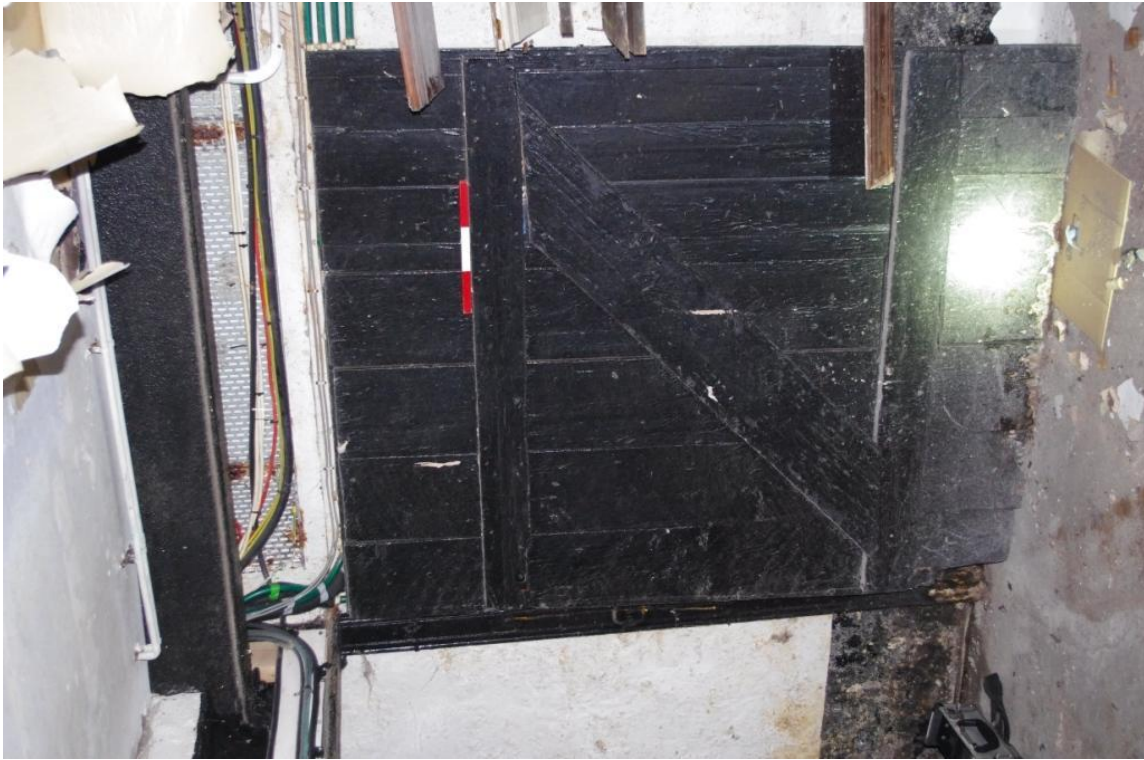
Figure 12 Original Plank & Batten Door in Cellar.
