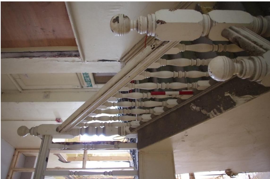
Figure 13 Stair Detail, Second Floor (Looking West).
