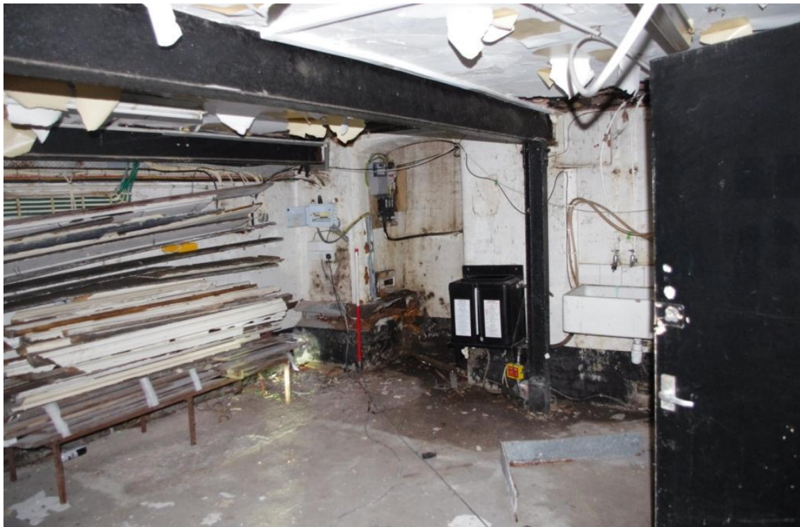
Figure 11 Cellar (B), General View (Looking East).
