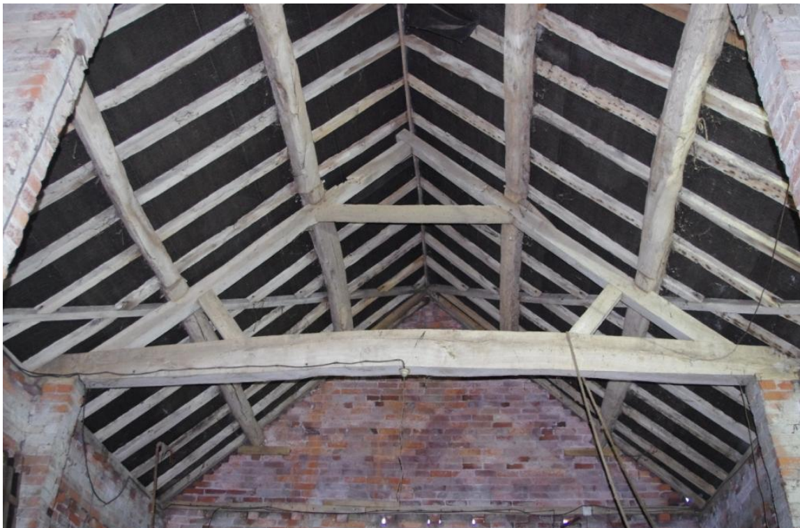
Figure 13 Truss 01 (Looking South West).
