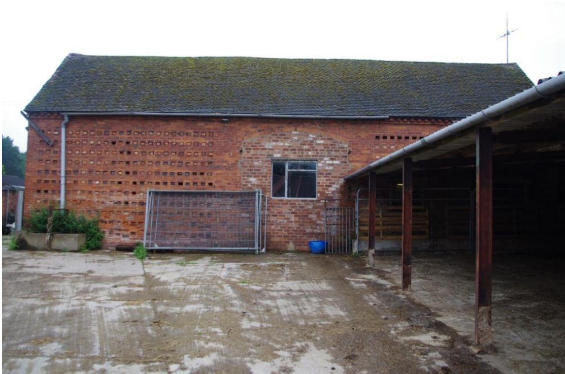
Figure 6 Principal Elevation (Looking North West).
