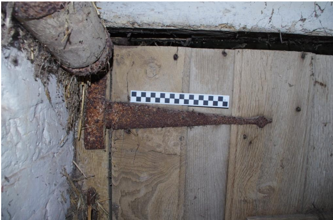
Figure 11 Potentially 17th Century Strap Hinge on Corn Hole Door.
