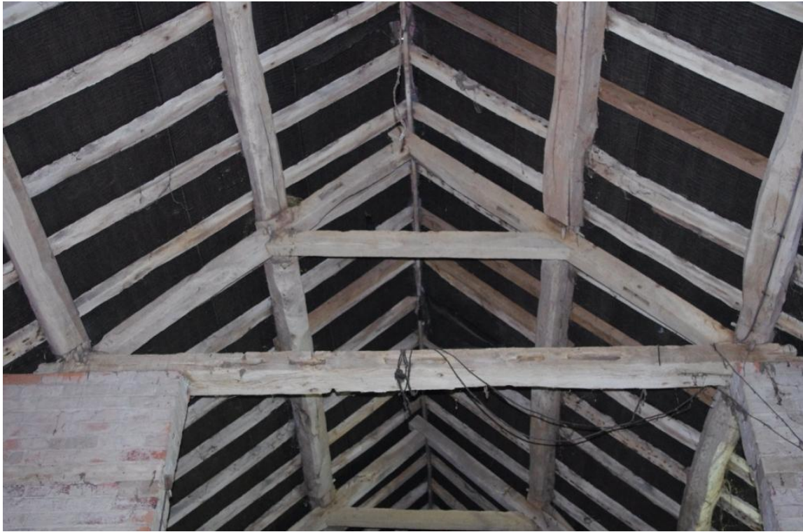
Figure 12 Truss 02 (Looking South West).
