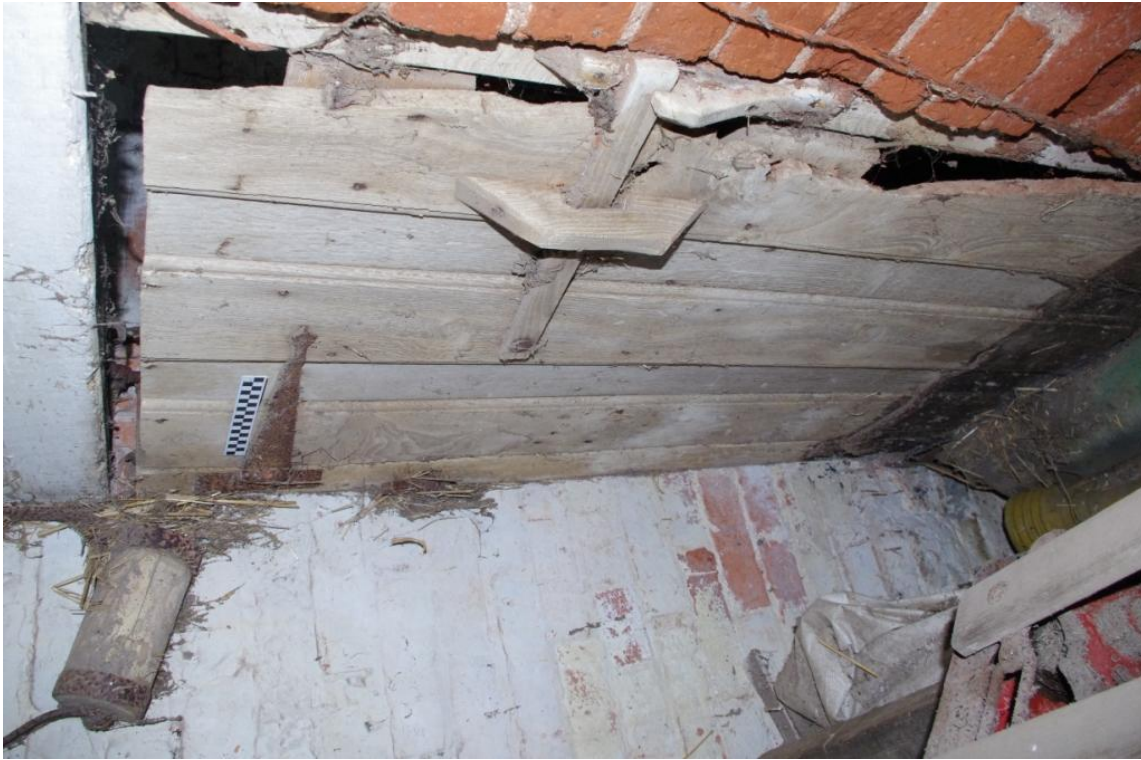
Figure 10 Potentially 17th Century Door to Corn Hole.
