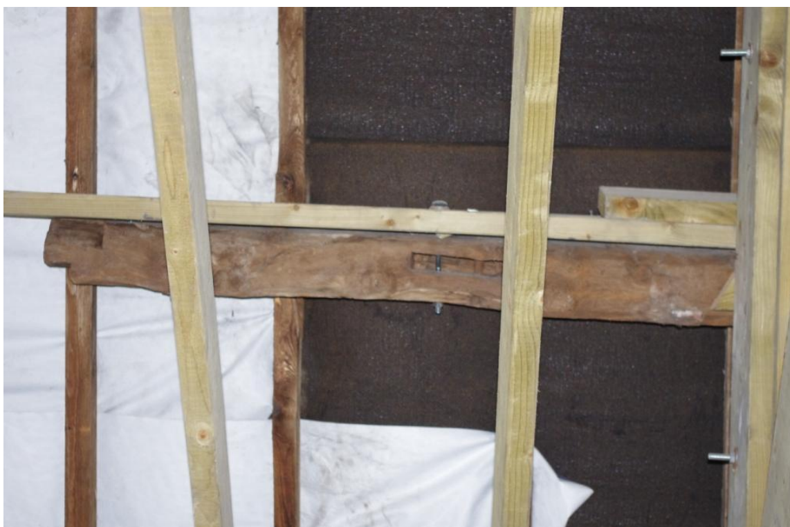
Figure 12 ▲ Re-used Purlin on Front Roof.
