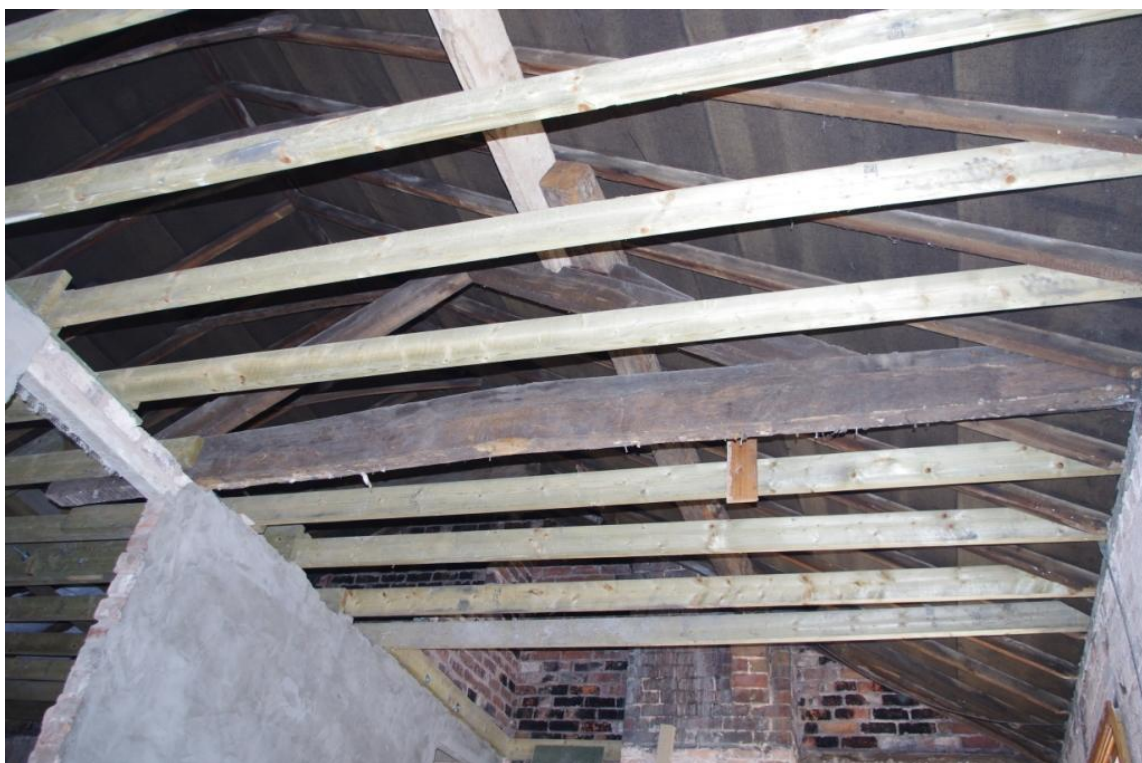
Figure 11 ▲ Partial Roof Truss.
