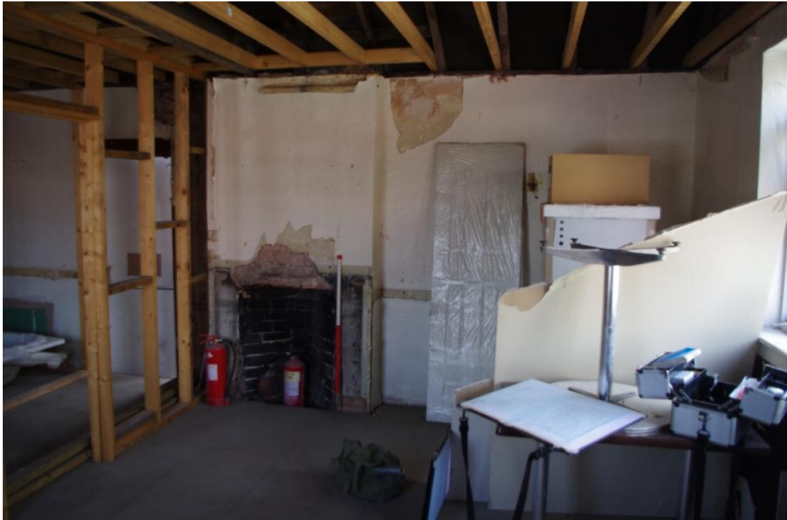
Figure 15 B (07) Smaller Chimney Breast (Looking South – South West).
