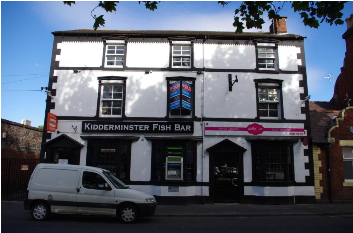
Figure 7 Principal Elevation (Looking West – North West).
