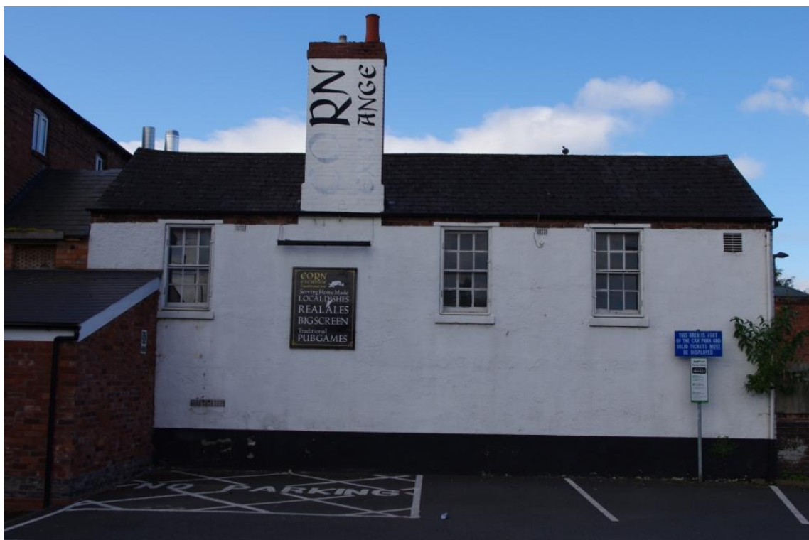
Figure 9 North – North East Facing Elevation of B (Looking South – South West).
