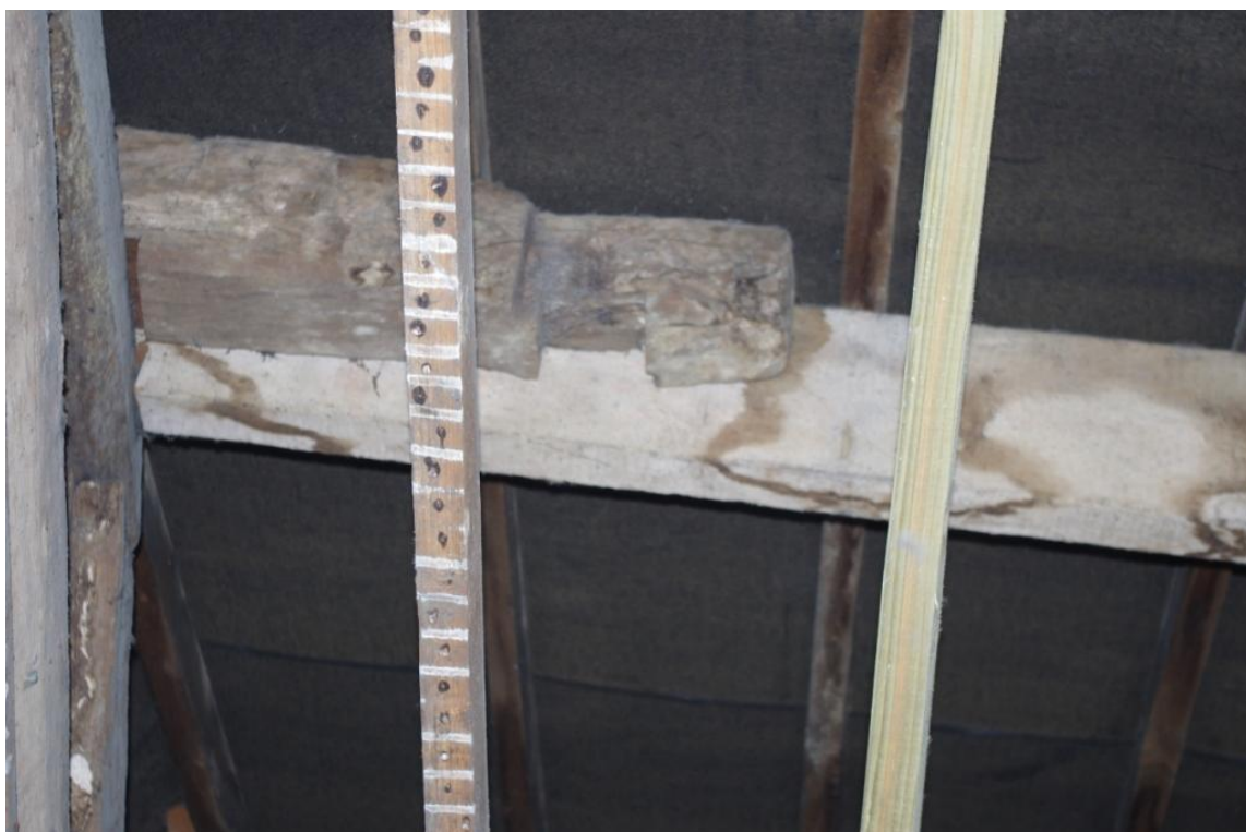
Figure 13 ▲ Re-used Purlin on Front Roof.
