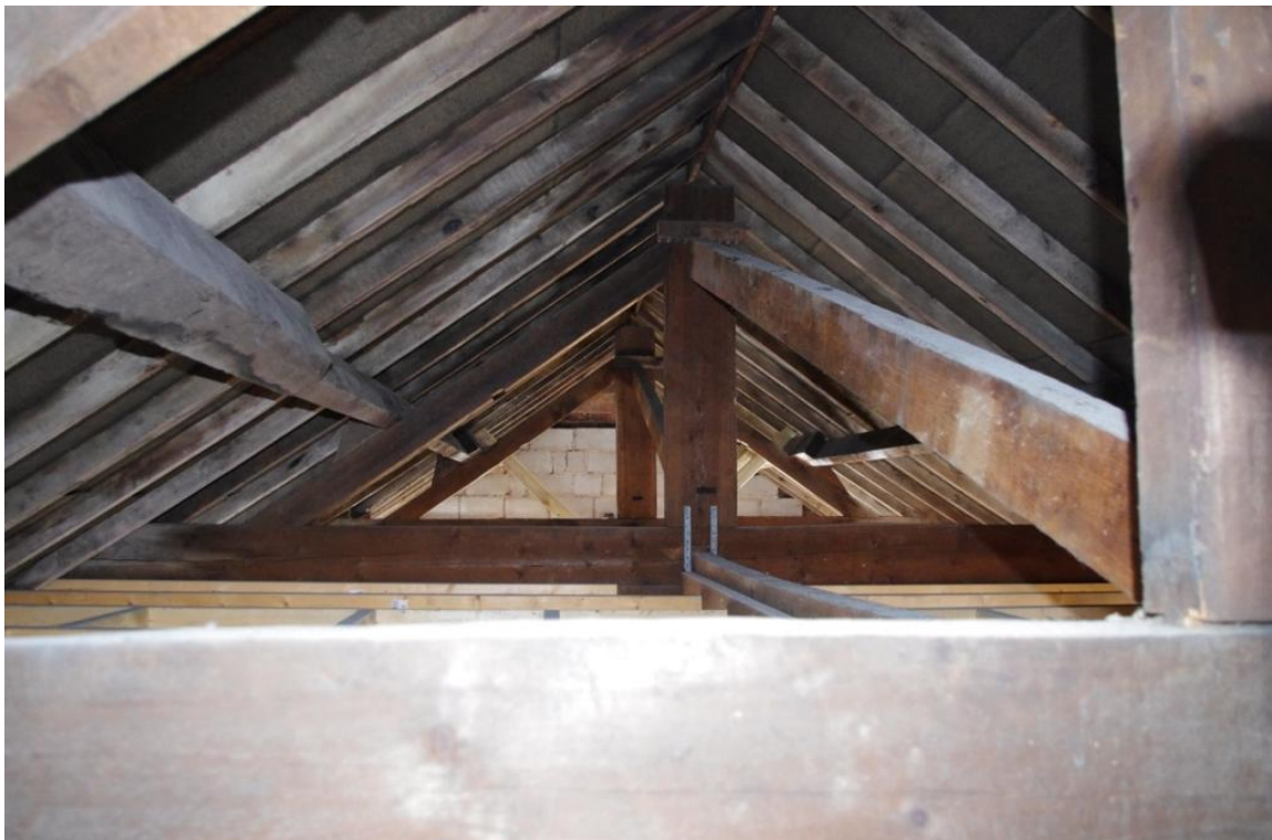
Figure 16 B King Post Truss (Looking West – North West).
