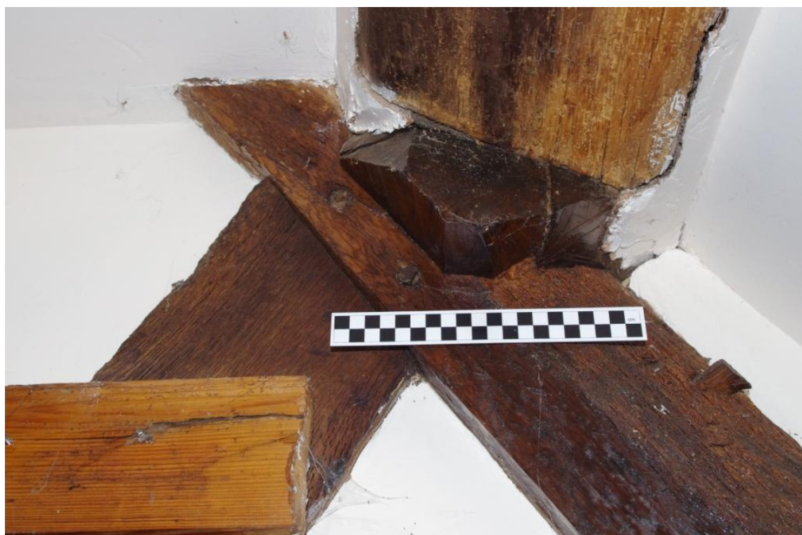
Figure 21 (4) Butt Purlin with Bolted Principal & Raking Strut.
