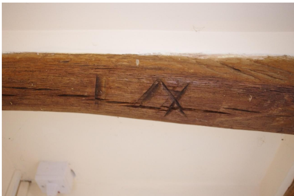
Figure 25 Incised Assembly Marks on Underside of Collar Beam in (5).
