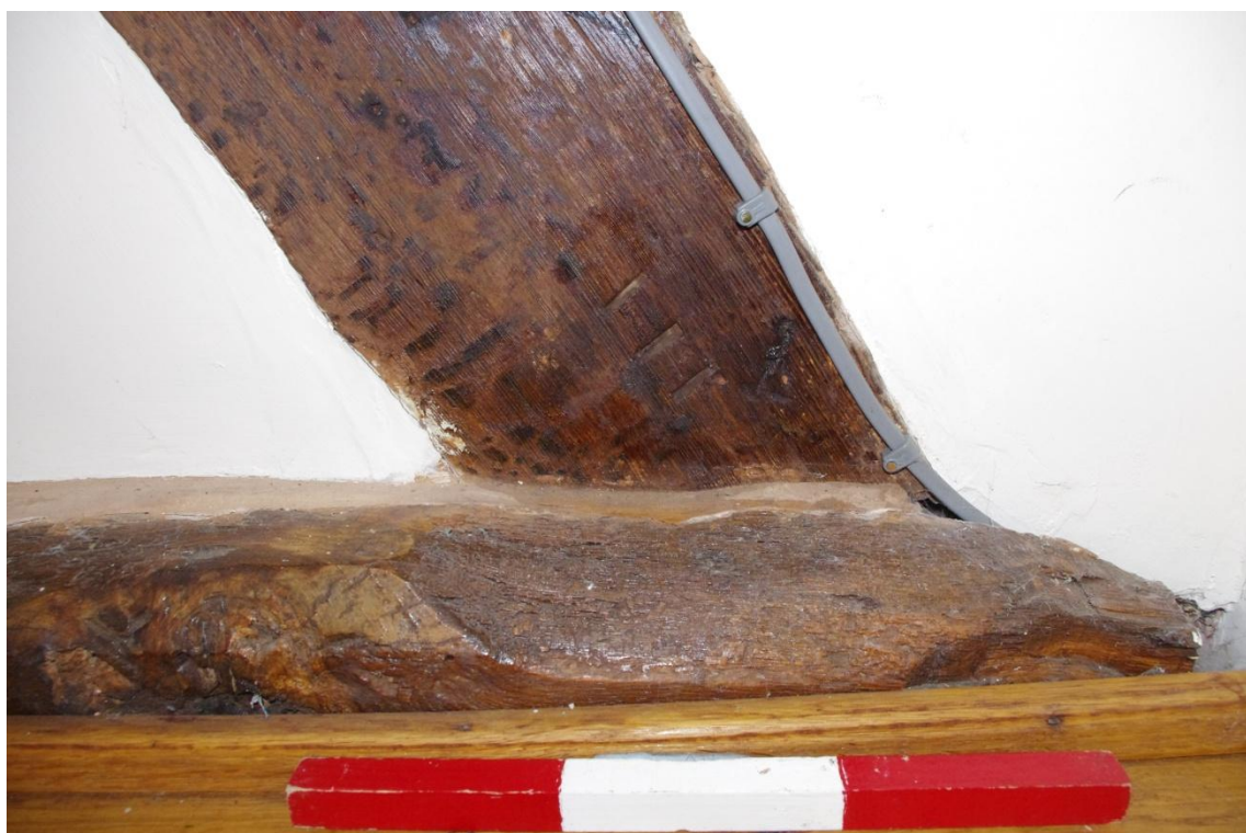
Figure 23 Incised Assembly Marks on South East Face of Tie Beam in (6).
