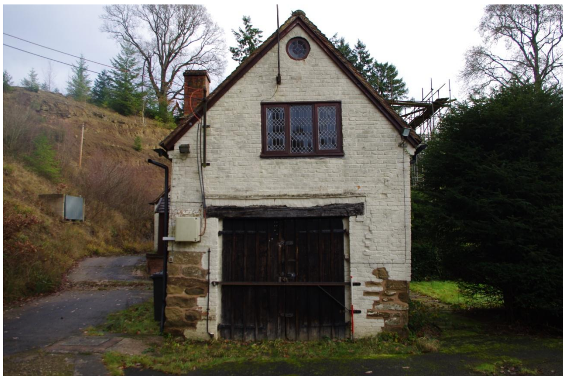
Figure 14 The Lodge, North West Facing Gable Showing Re-building.
