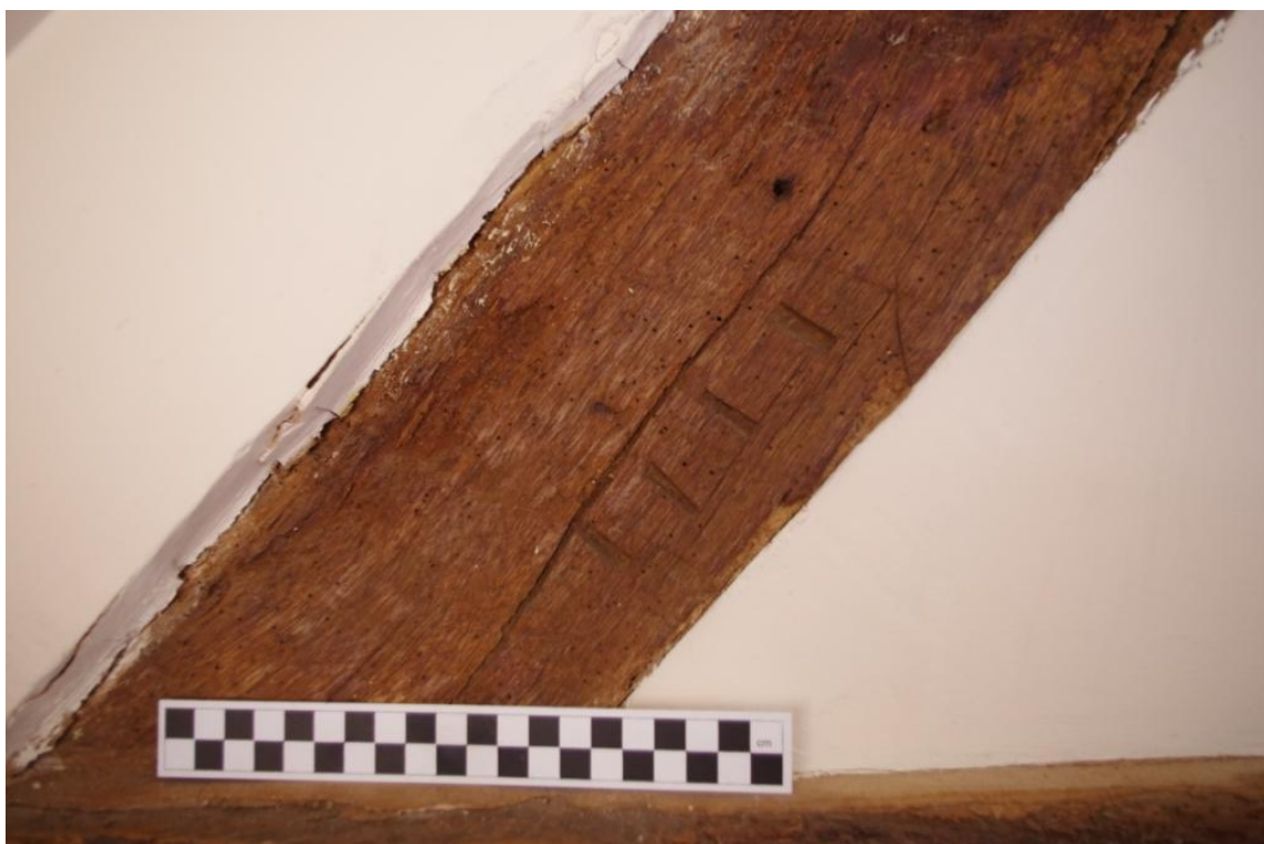
Figure 24 Incised Assembly Marks on South East Face of Tie Beam in (5).
