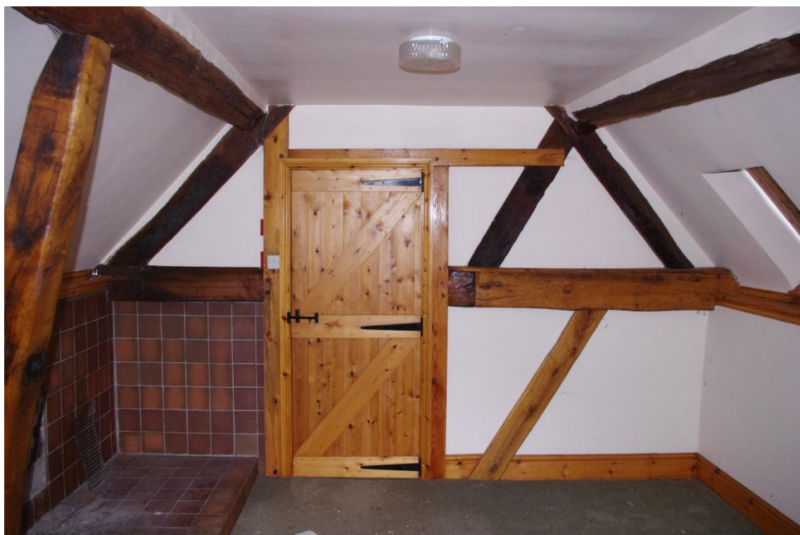
Figure 20 Central Roof Truss (Looking South East).
