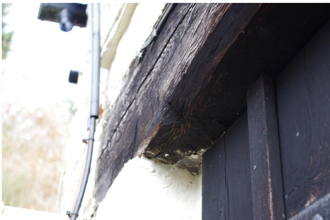
Figure 15 Stopped & Chamfered Beam on North West Facing Gable.
