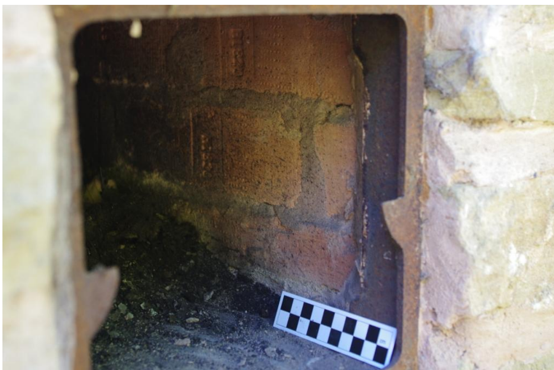
Figure 17 Modern Brickwork within the Chimney.
