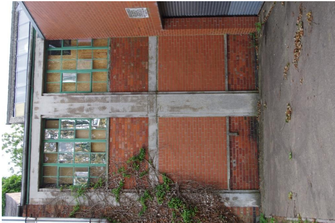
Figure 8 Southern Concrete Framed Extension (Looking South East).
