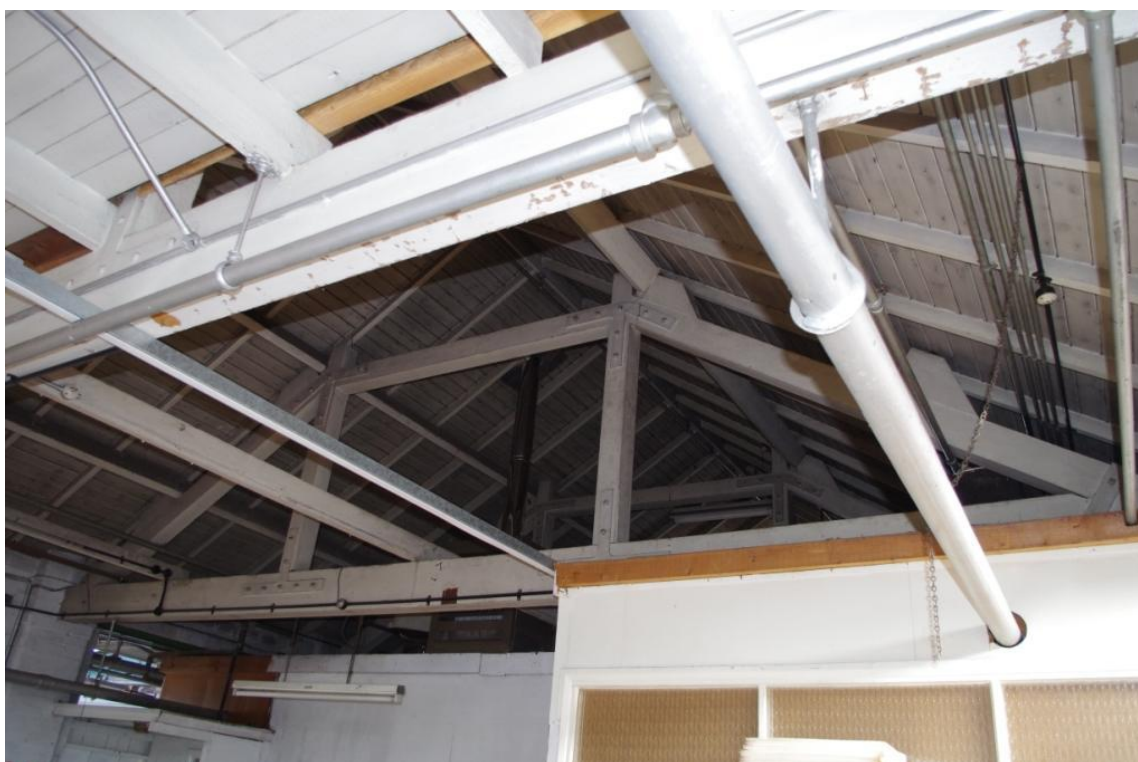
Figure 6 Queen Post Truss in Original Building.
