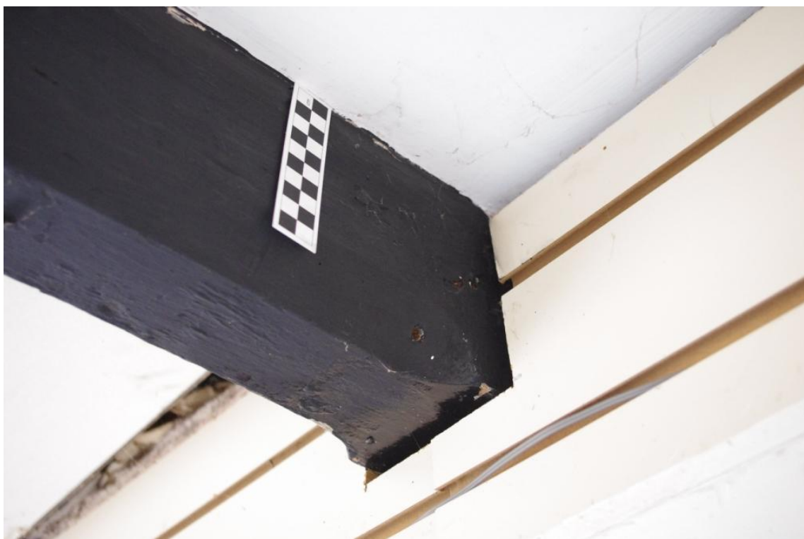
Figure 10 Room (1), Chamfered and Stopped Bridging Beam.
