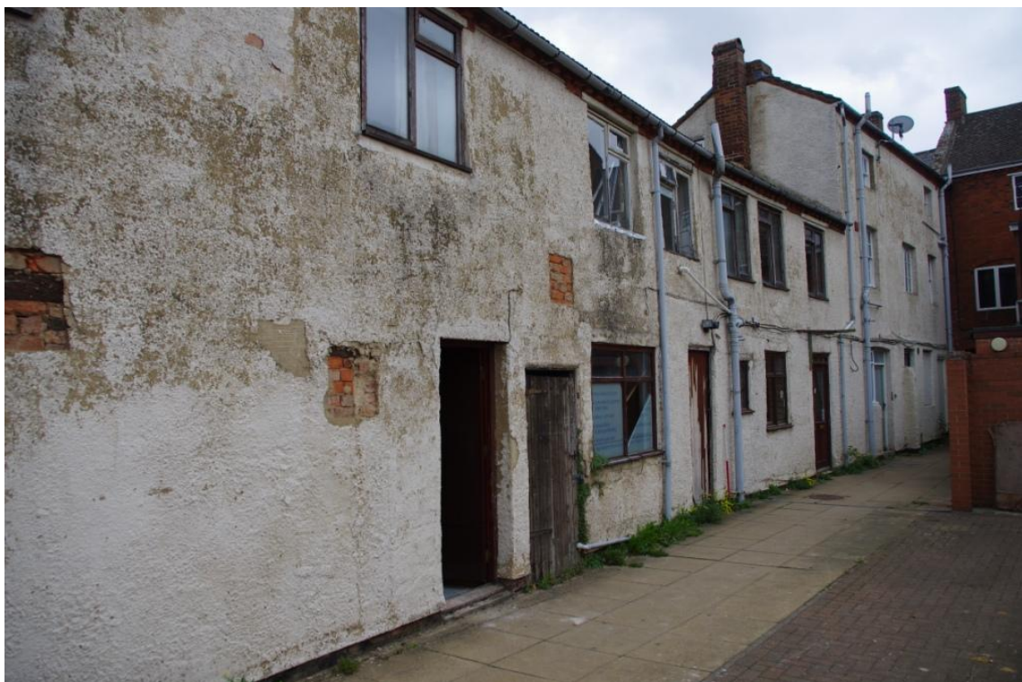
Figure 7 Principal Elevation (Looking South East).
