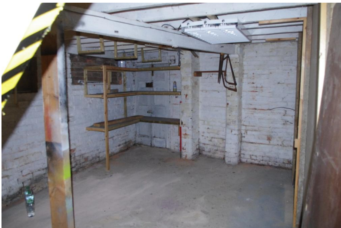
Figure 12 Room (2) South Facing Gable Showing Earlier Door (Left) and Brick Columns Supporting First Floor Chimney (Looking North – North West).
