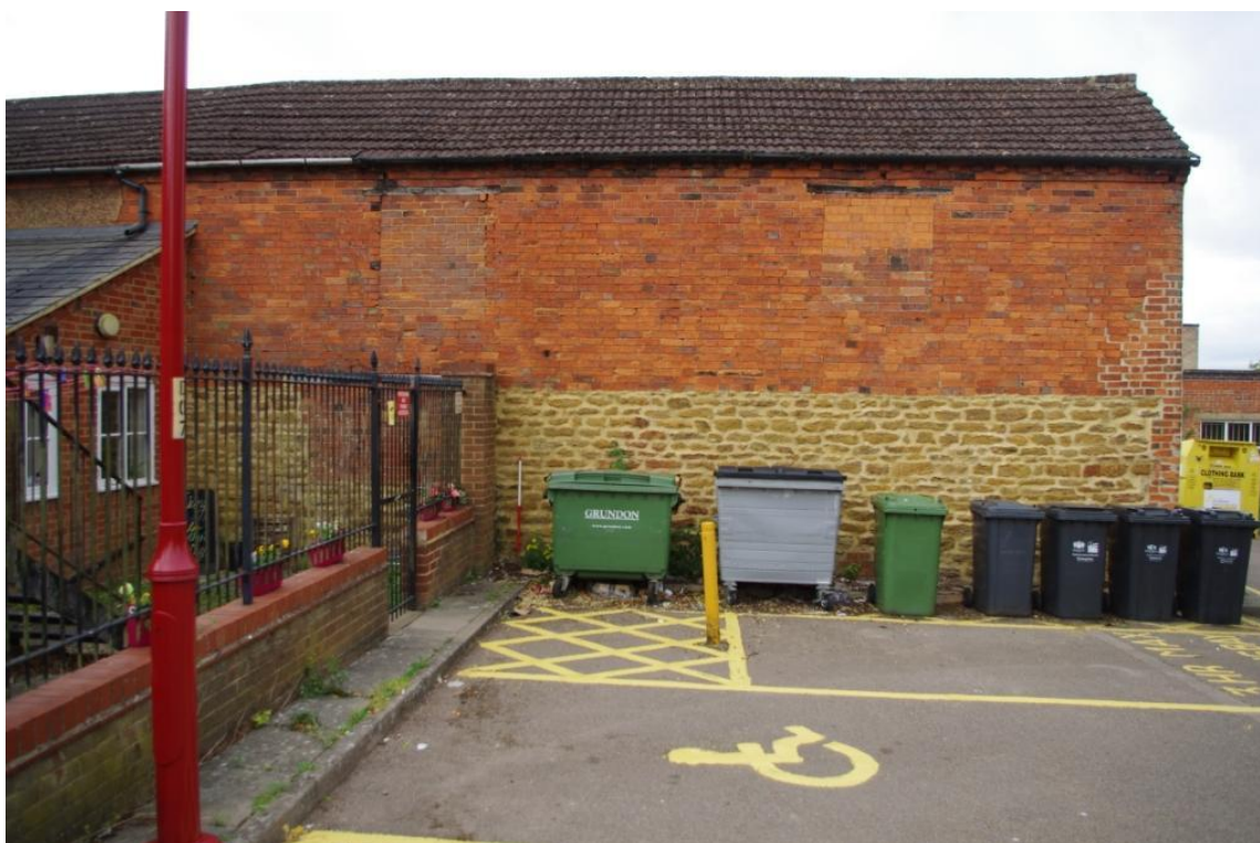
Figure 6 East – North East Facing Long Elevation (Looking West – South West).
