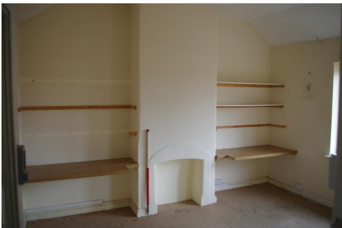
Figure 13 Room (3) Chimney Breast (Looking South).
