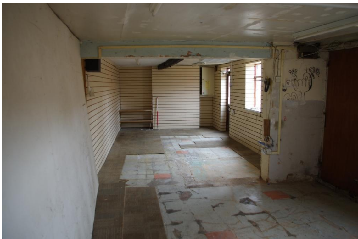
Figure 9 Room (1), General View (Looking South – South East).
