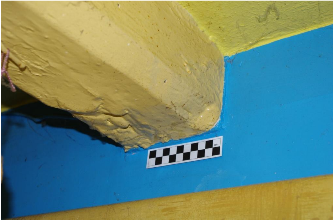
Figure 18 A(9) Chamfered and Stopped Bridging Beam.
