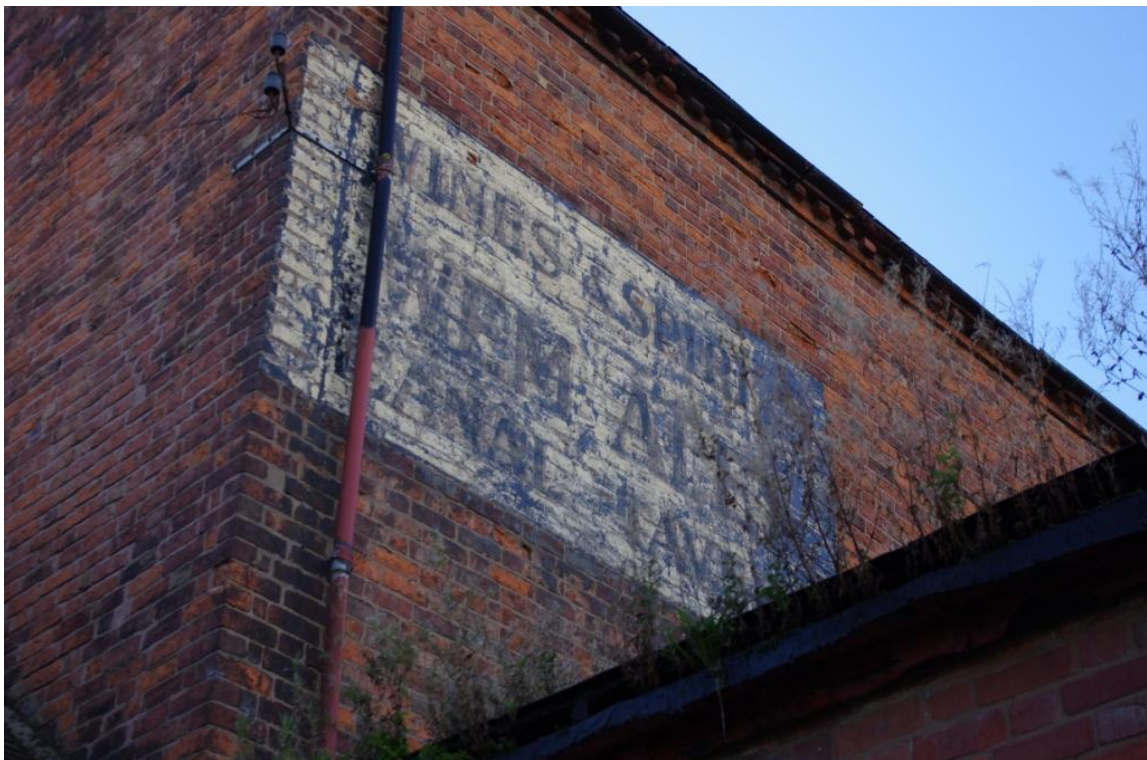
Figure 15 Signage on Rear (Canalside) Elevation.
