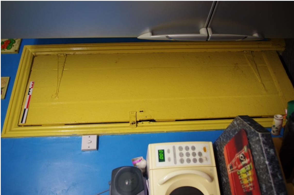
Figure 18 A(9) Chamfered and Stopped Bridging Beam.
