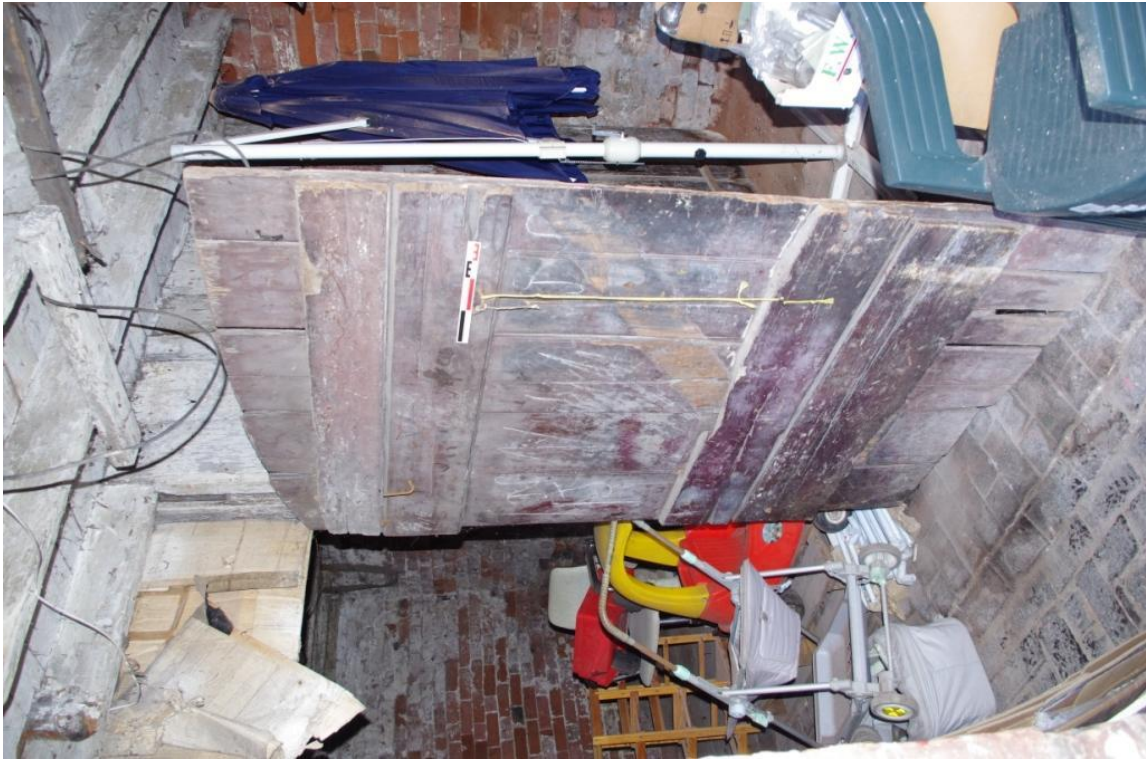
Figure 20 B (12) 19th Century Plank Door.
