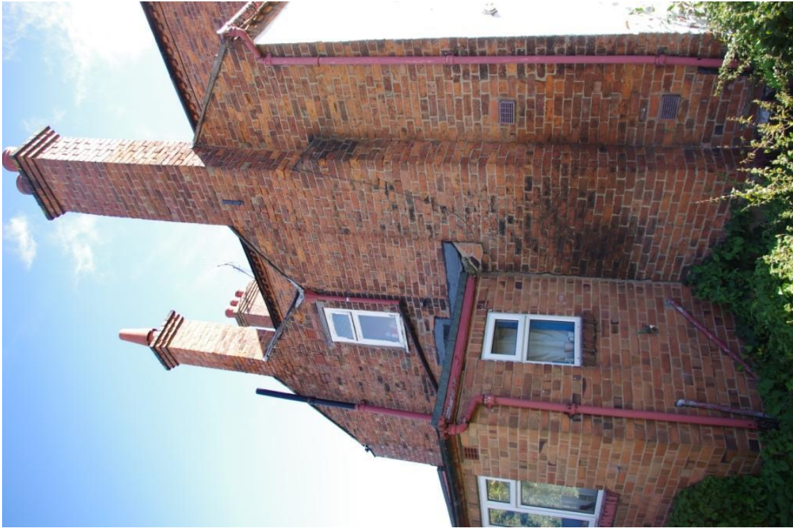
Figure 14 Rear Elevation (Looking South-South East).
