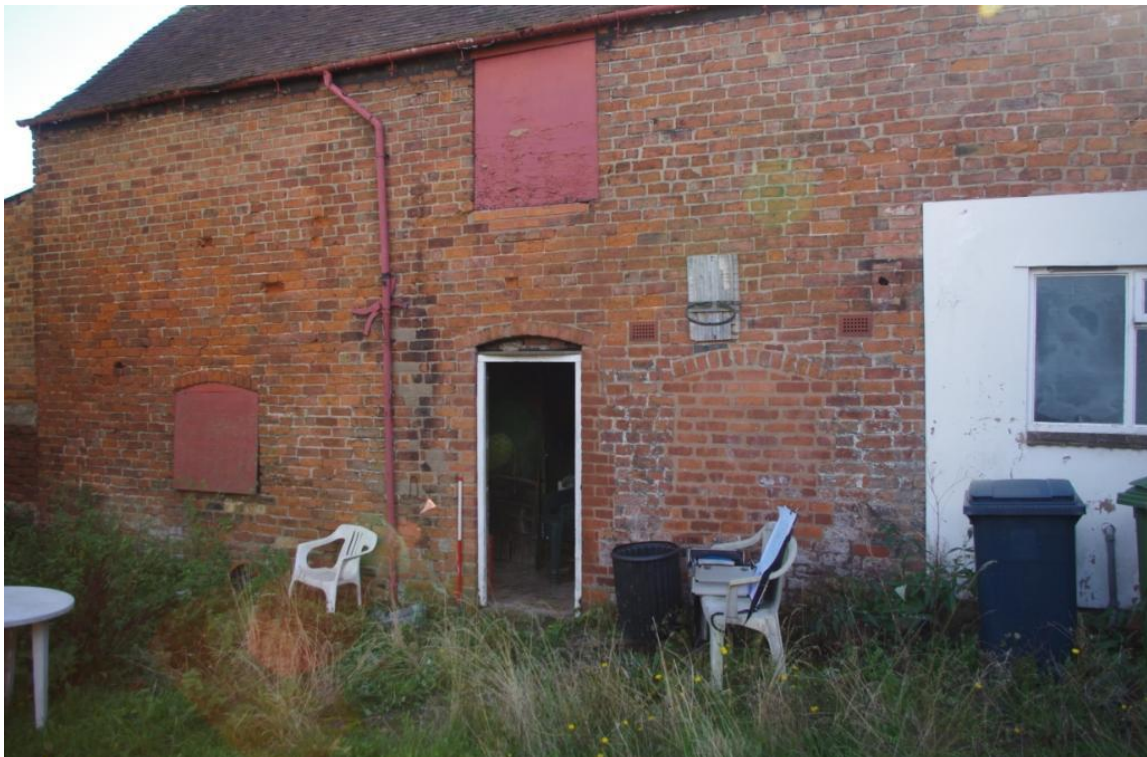
Figure 17 B(12) Rear Elevation (Looking South East).
