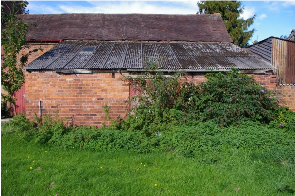
Figure 16 B(13) Principal Elevation (Looking North West).
