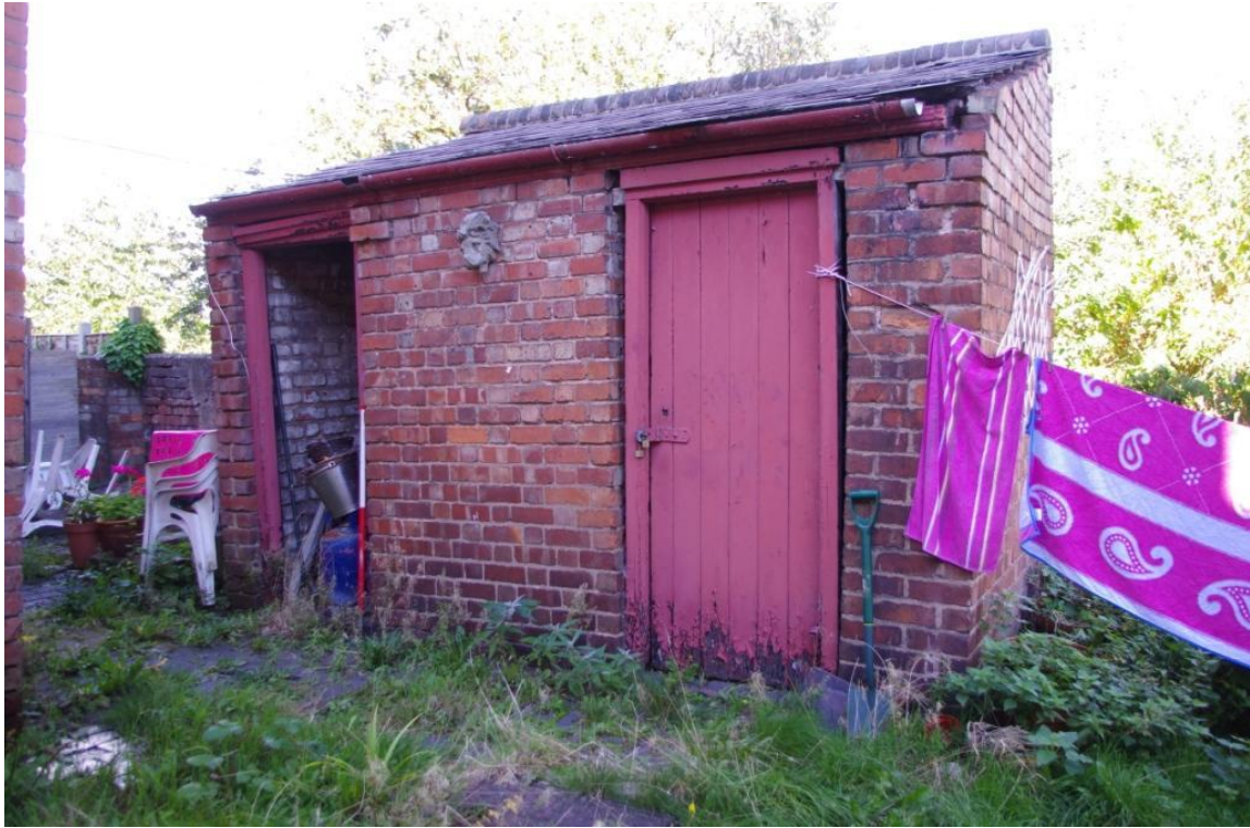
Figure 24 C Principal Elevation (Looking West-North West).
