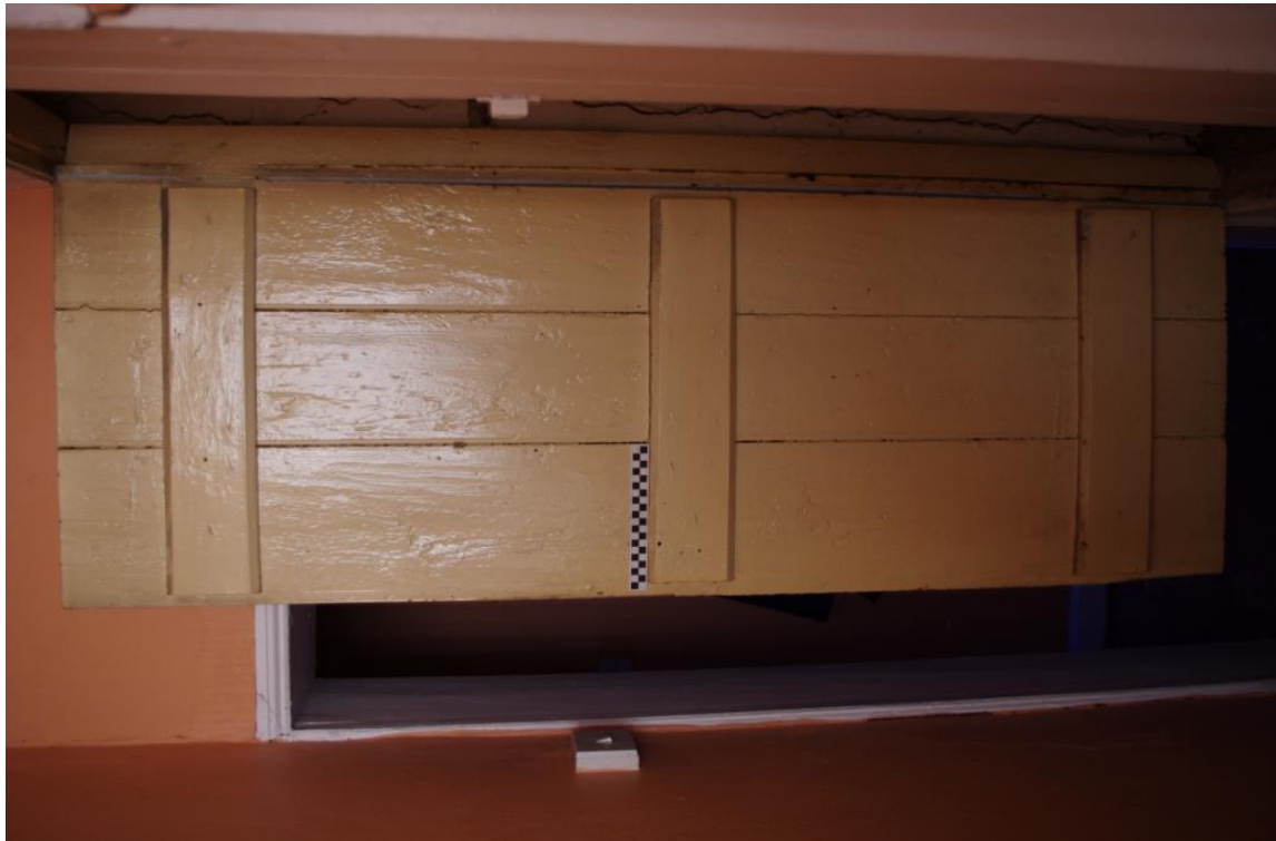
Figure 21 A (5) Plank and Batten Door.
