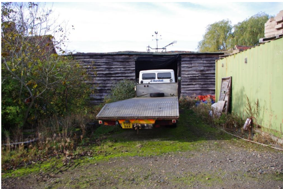
Figure 6 Rear Elevation (Looking West – South West).
