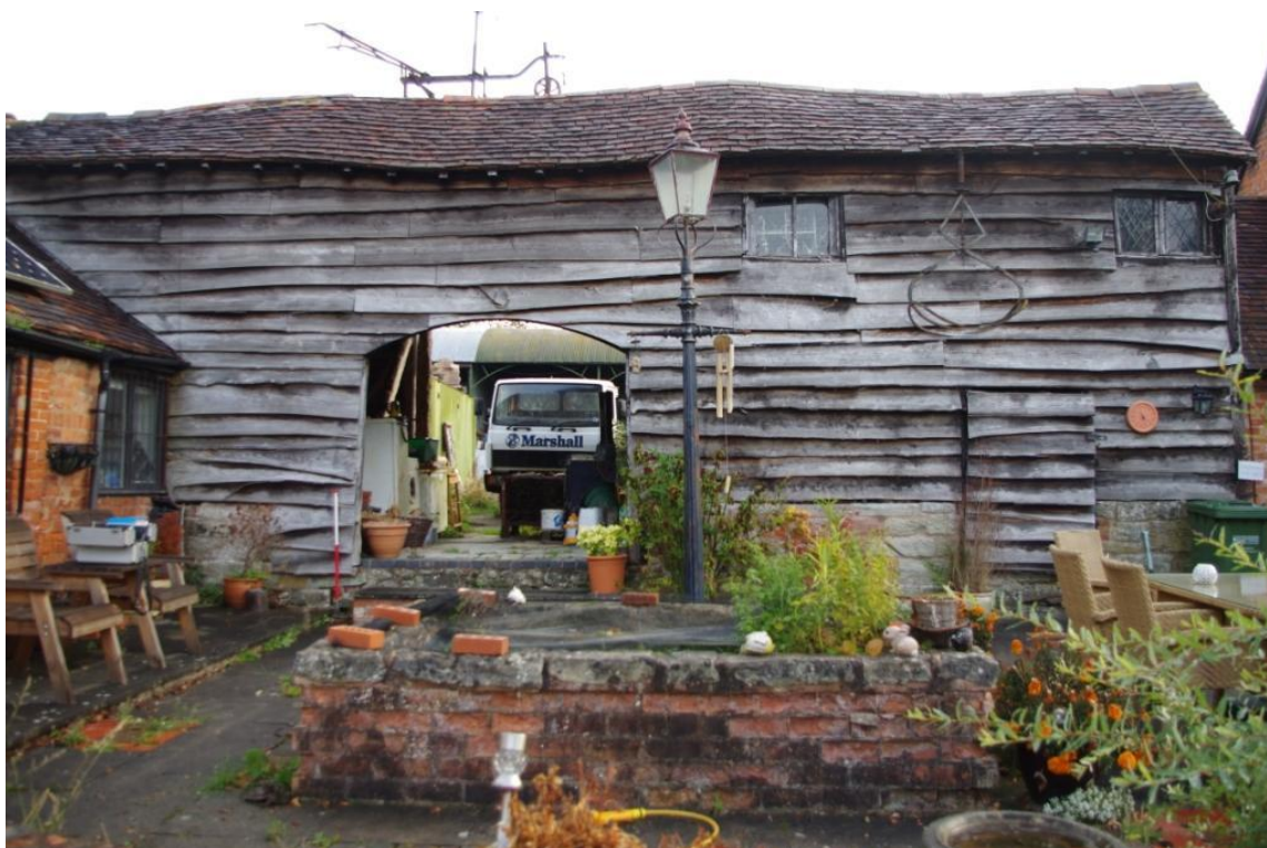
Figure 5 Principal Elevation (Looking East – North East).
