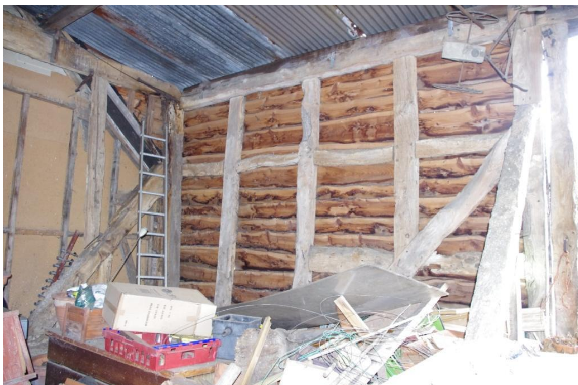
Figure 8 Square Framing on East Facing Elevation (Looking North – North East).
