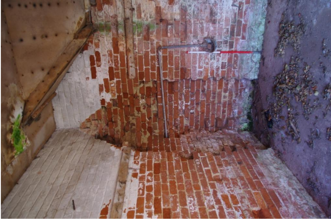
Figure 12 (16), Outline of Kiln/Furnace Structure in South West Corner.
