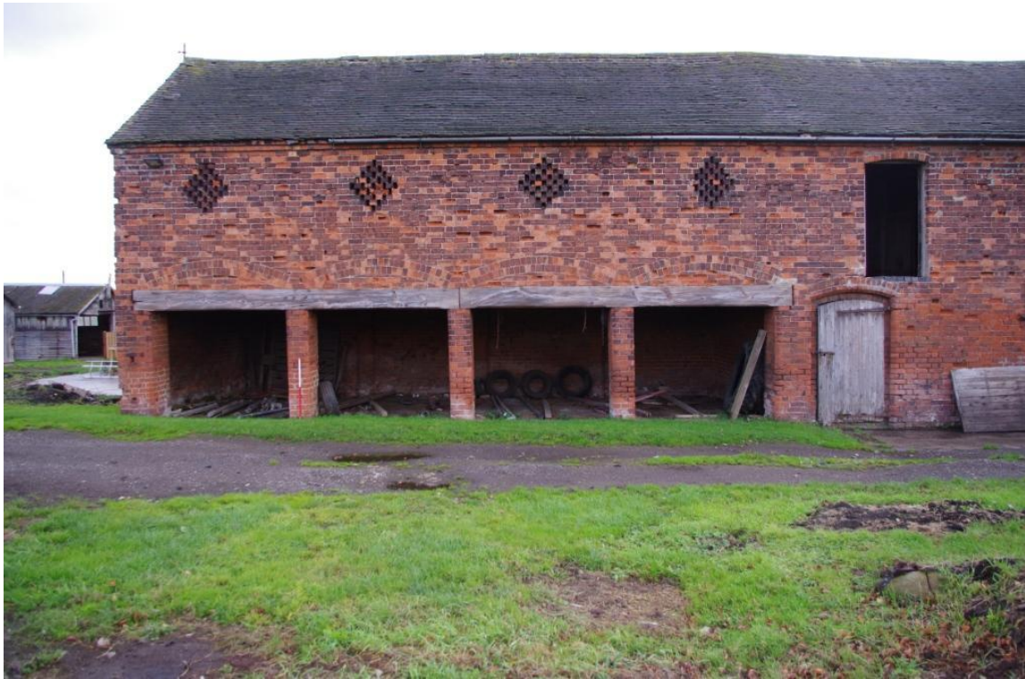
Figure 8 (6), West – North West Facing Elevation (Looking East – South East).
