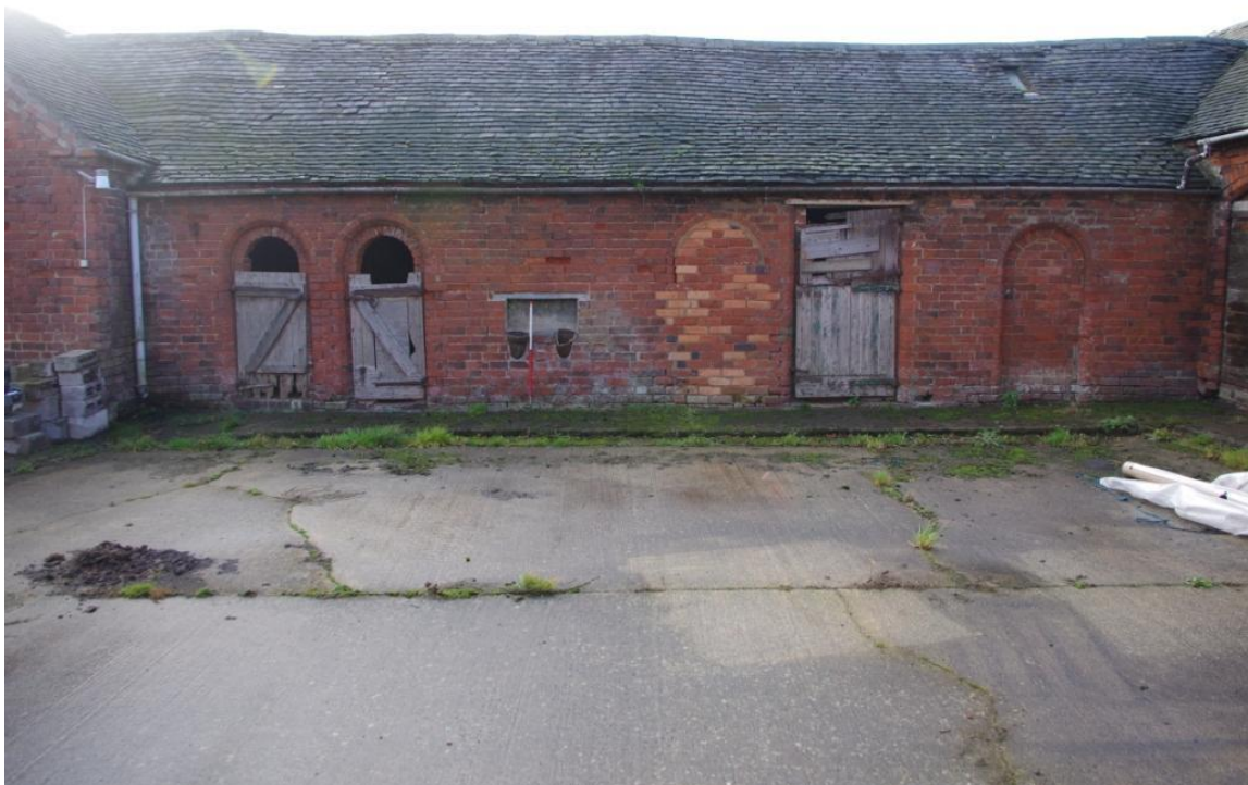
Figure 11 B(20), (21) & (22), North – North East Facing Elevation (Looking South – South West).
