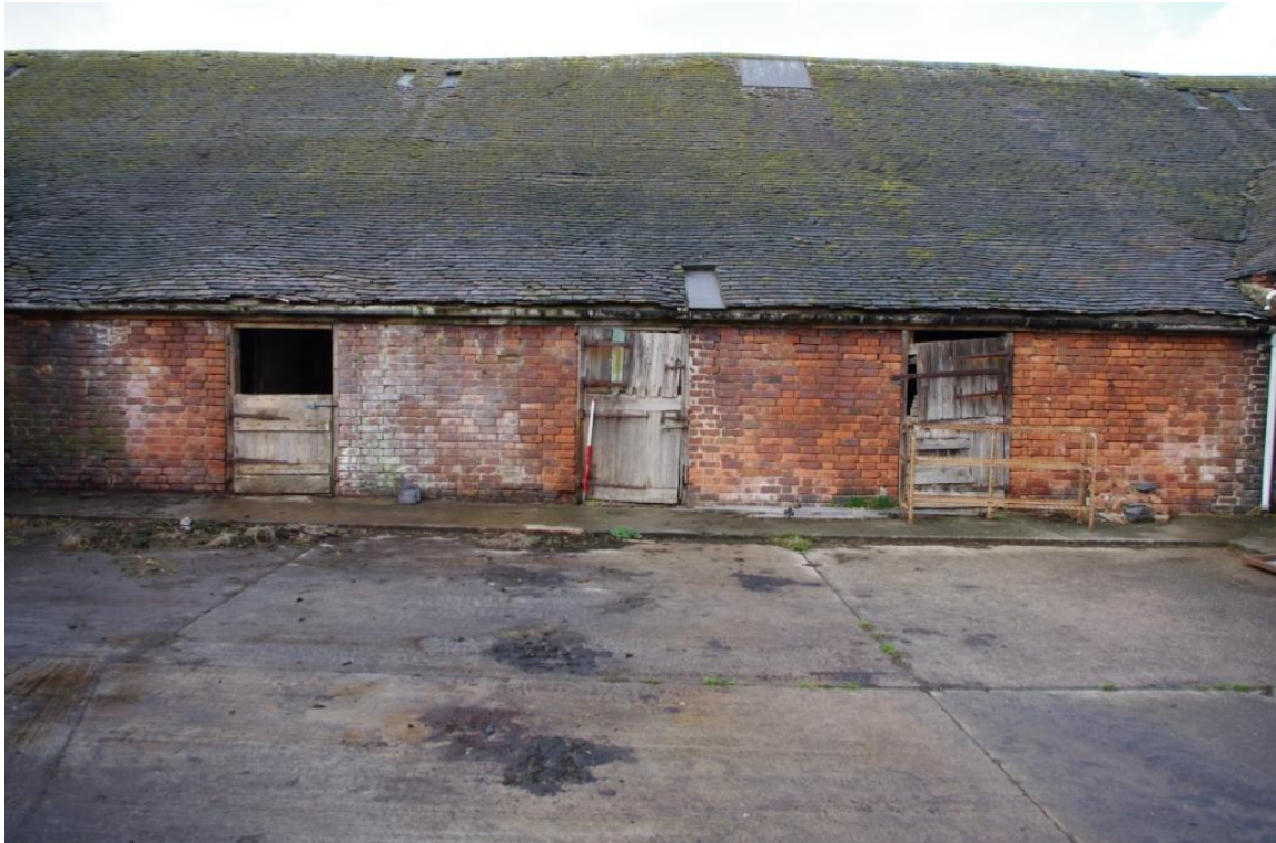
Figure 20 (10), (11), (12) & (13), East – South East Facing Elevation (Looking West – North West).
