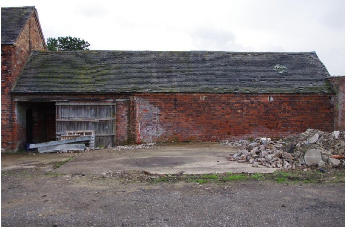
Figure 10 (1) & (2) West – North West Facing Elevation (Looking East – South East).
