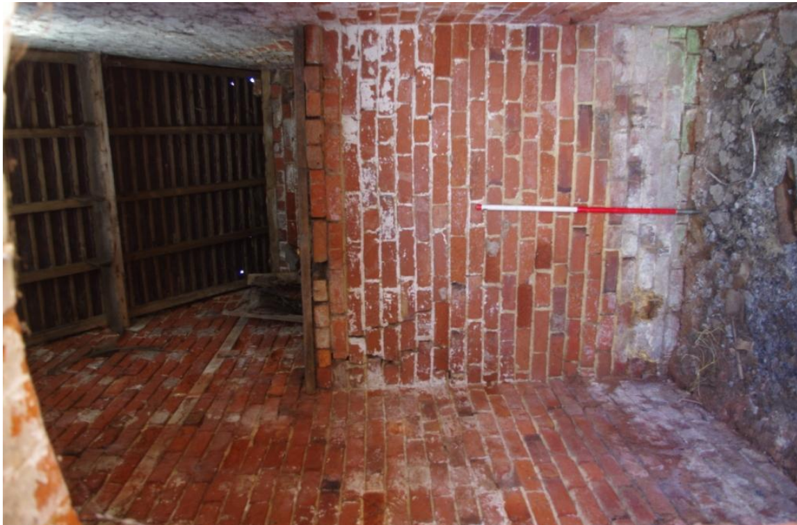
Figure 13 (18), Possible Poultry House (Looking East - North East).
