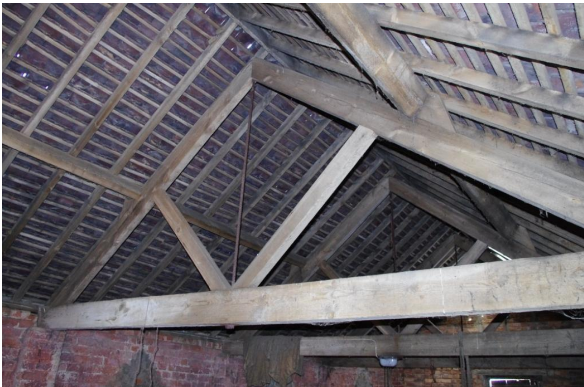
Figure 9 Roof Truss in Granary.
