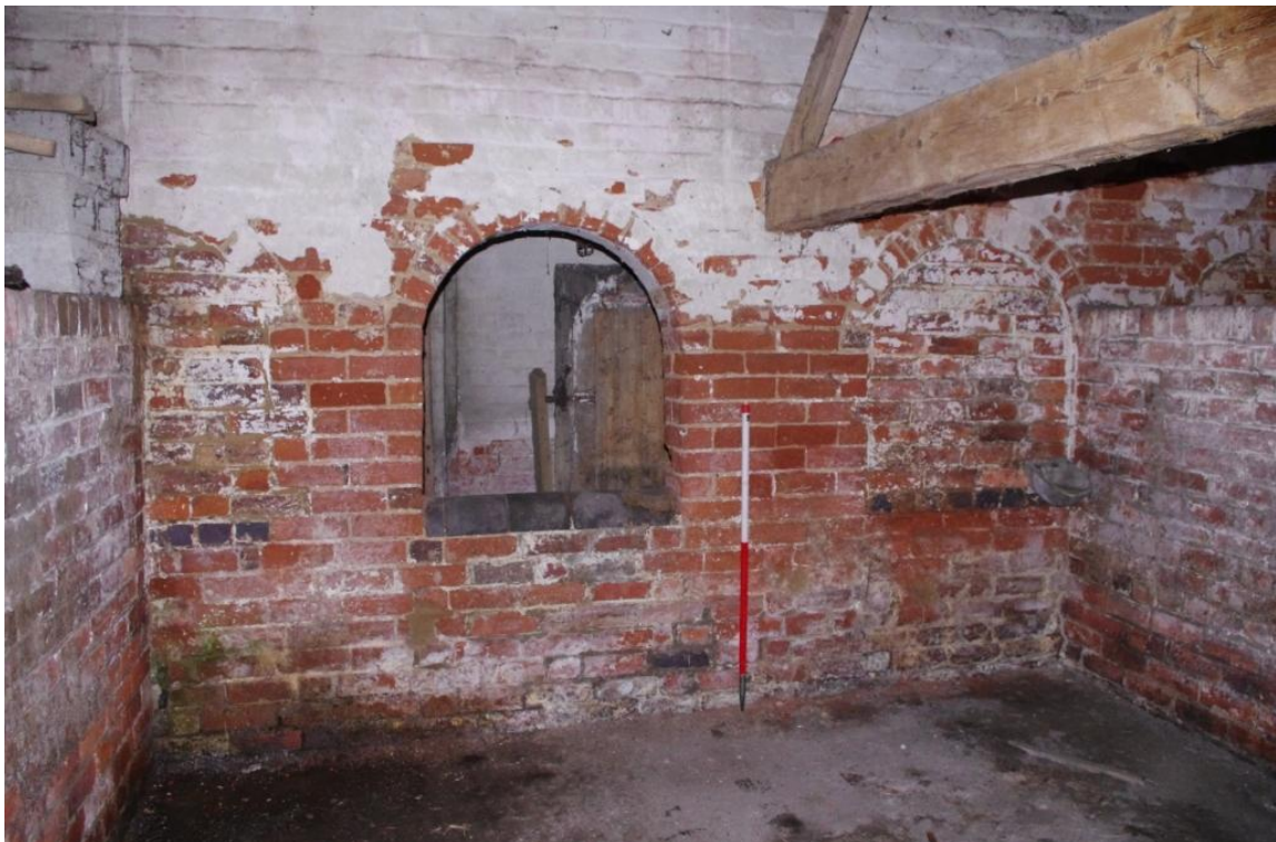
Figure 21 (11), Arched Feeding Holes from Feeding Passage (Looking North West).
