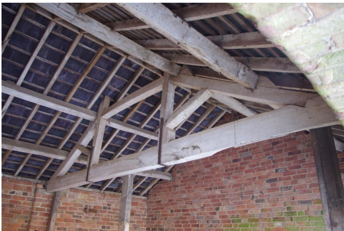
Figure 15 Building D (13) Queen Post Roof Truss.
