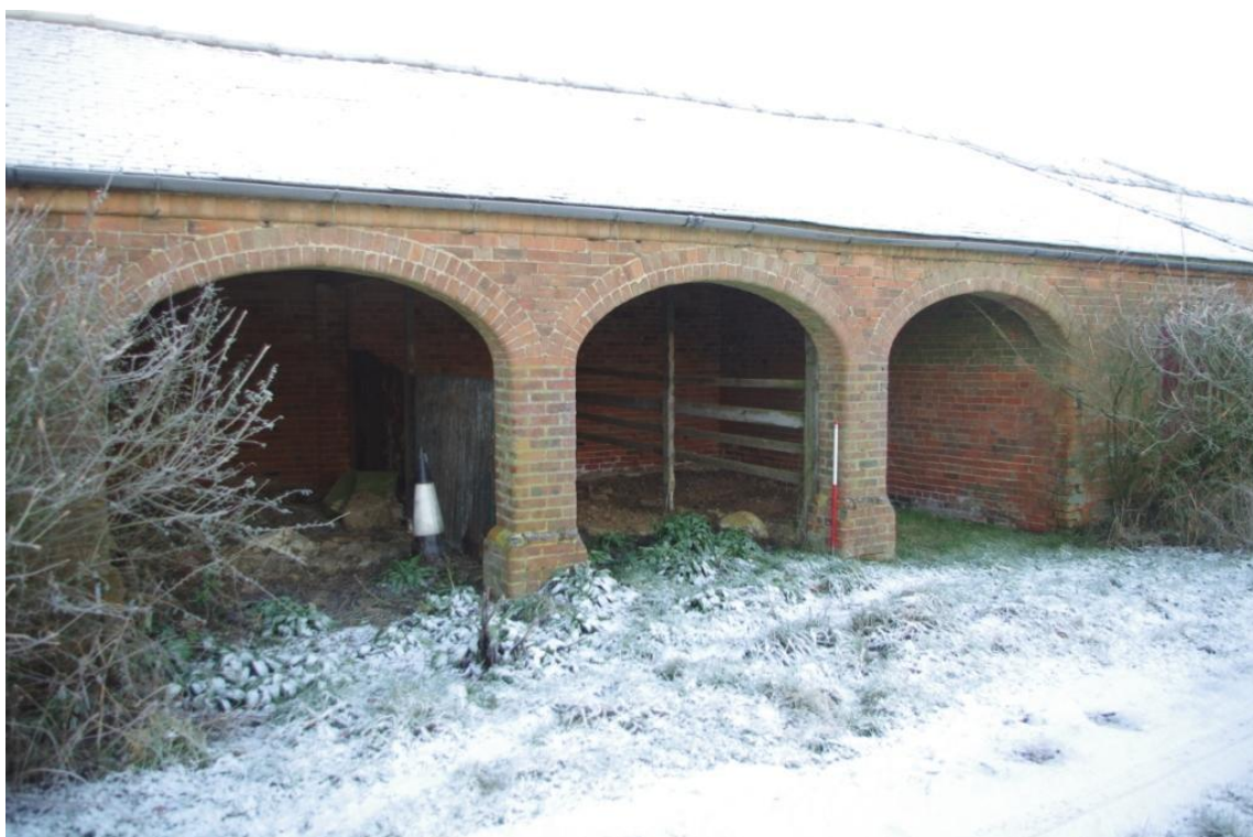
Figure 13 Building D (13) North West Facing Elevation (Looking South).
