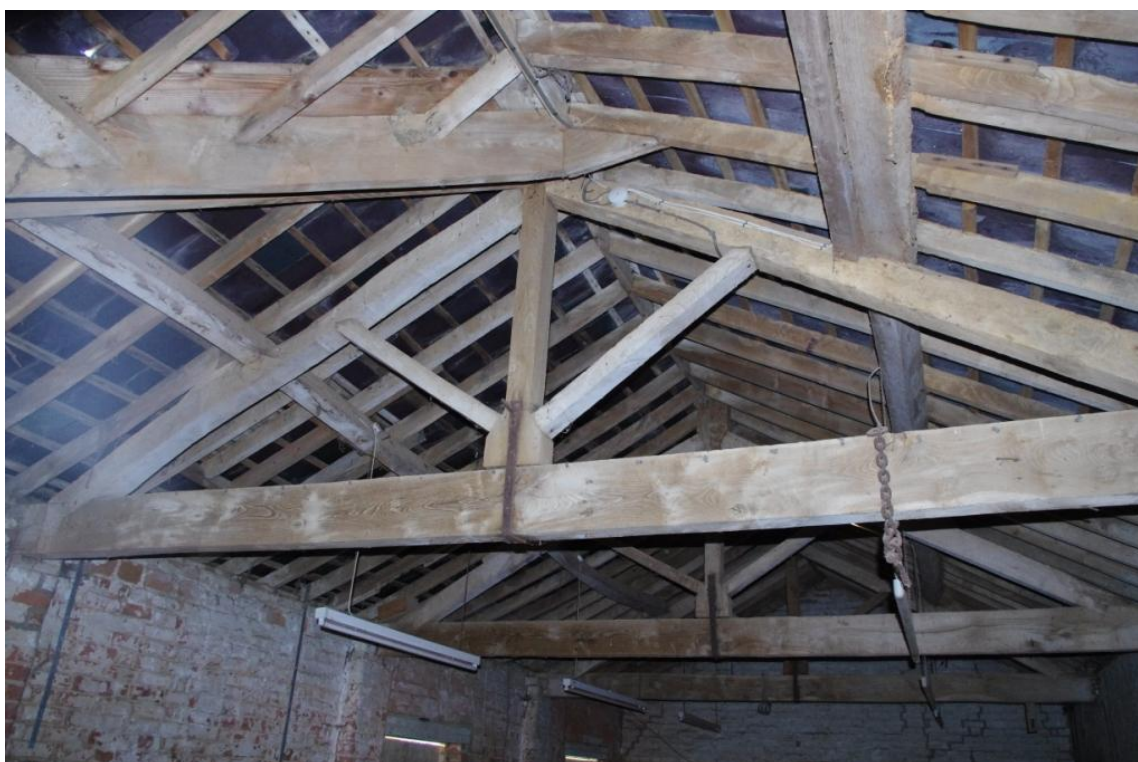
Figure 10 Building B (5) King Post Truss.
