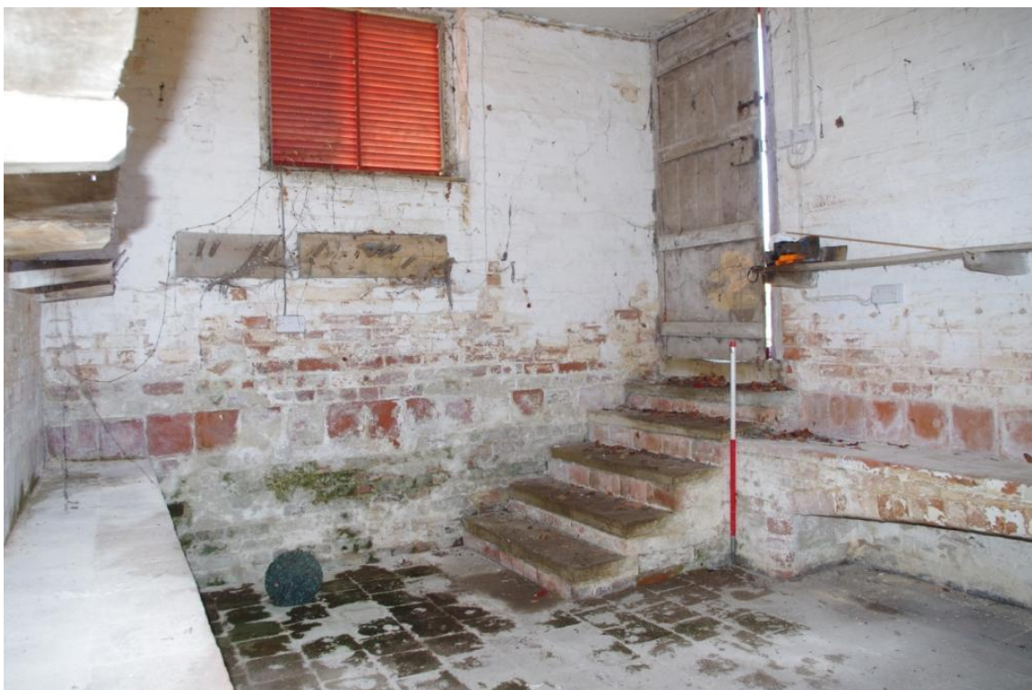
Figure 8 Building A(1) Sunken Dairy (Looking West).
