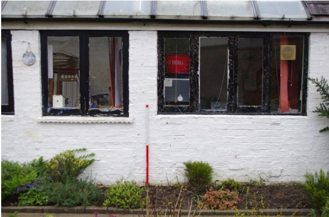
Figure 8 Principal Elevation Showing Extensive Glazing & Blocked Opening (Left) (Looking South East).
