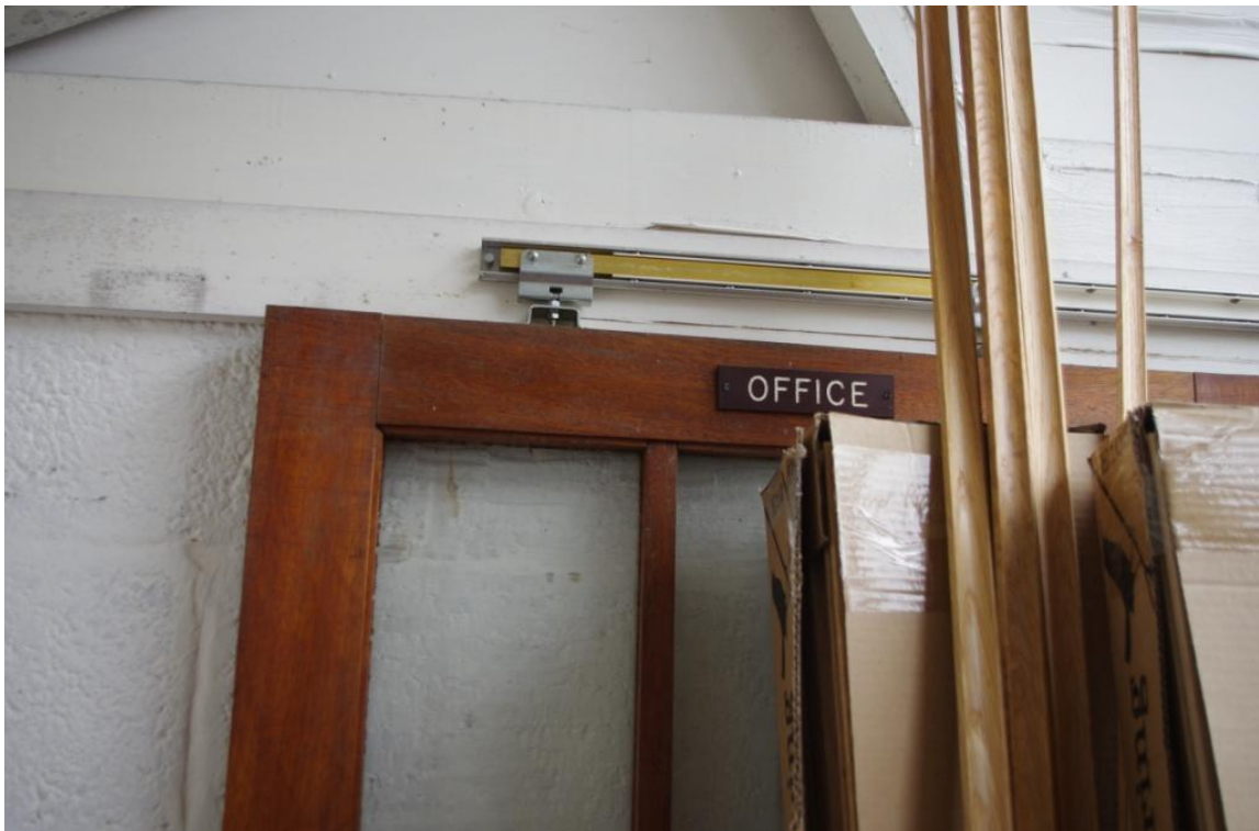
Figure 11 (3) Signage on Cross Wall Door.
