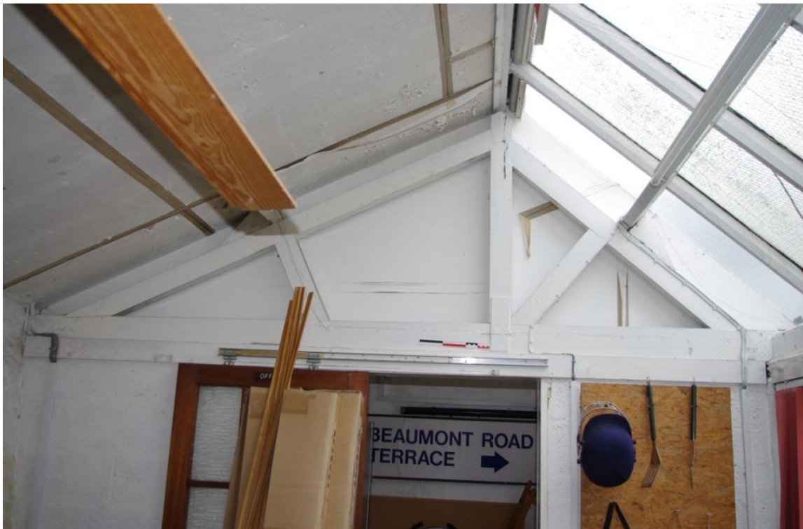
Figure 15 (3) Roof Truss (Looking South West).
