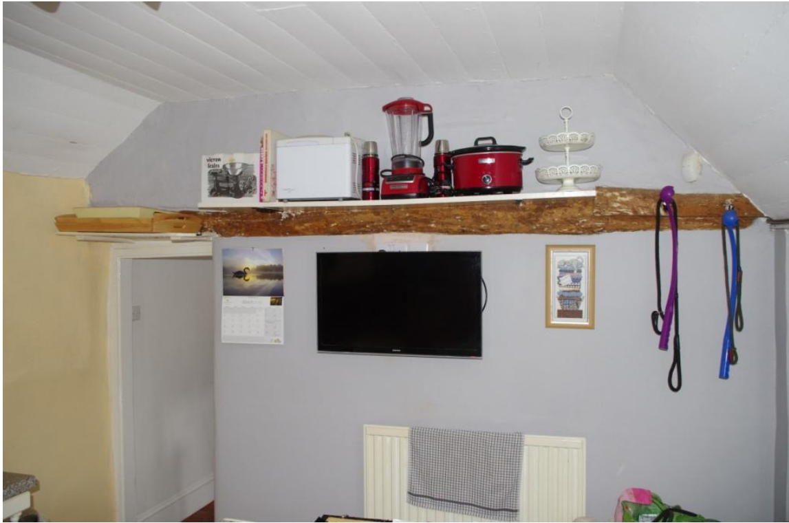
Figure 10 (1) Exposed Tie Beam in Westernmost Wall (Looking South West).
