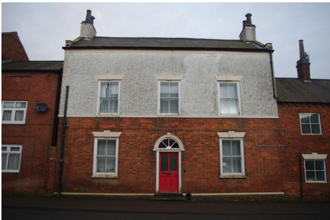
Figure 8 No. 31 Principal Elevation, General View (Looking North – North West).
