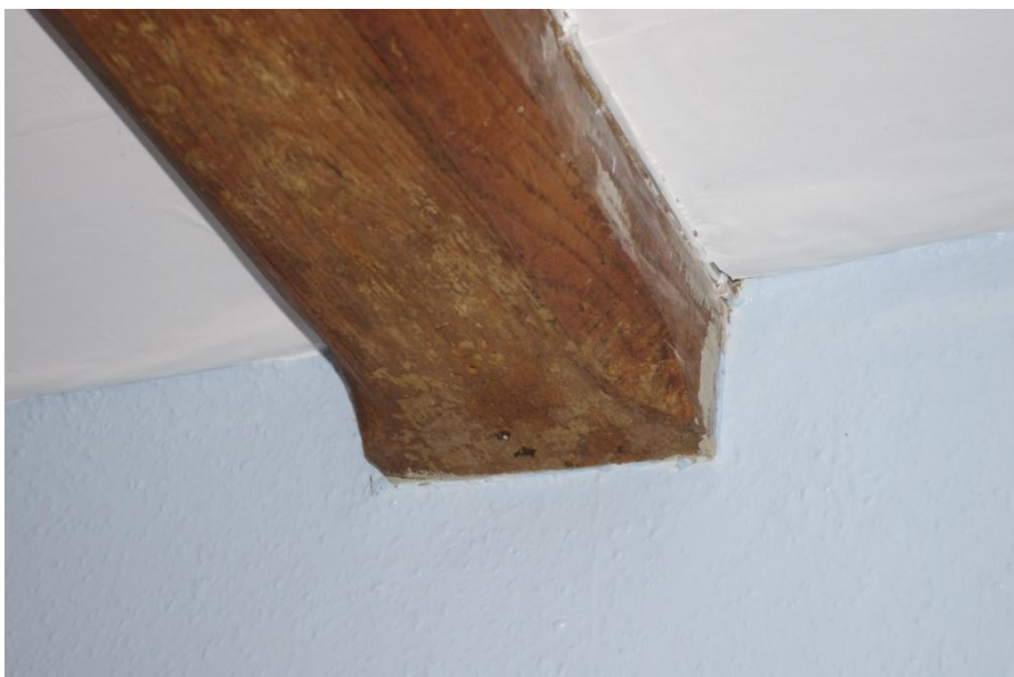
Figure 16 (8), Chamfered & Stopped Bridging Beam (Looking North East).
