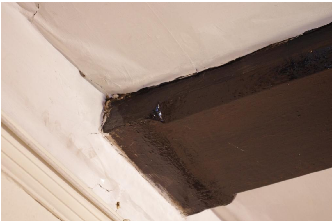
Figure 14 (4), Chamfered & Stopped Bridging Beam (Looking East).
