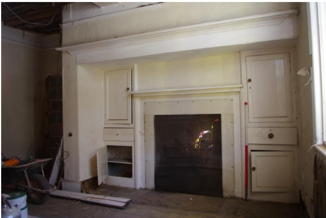
Figure 13 (3) Gable Fireplace (Looking North East).
