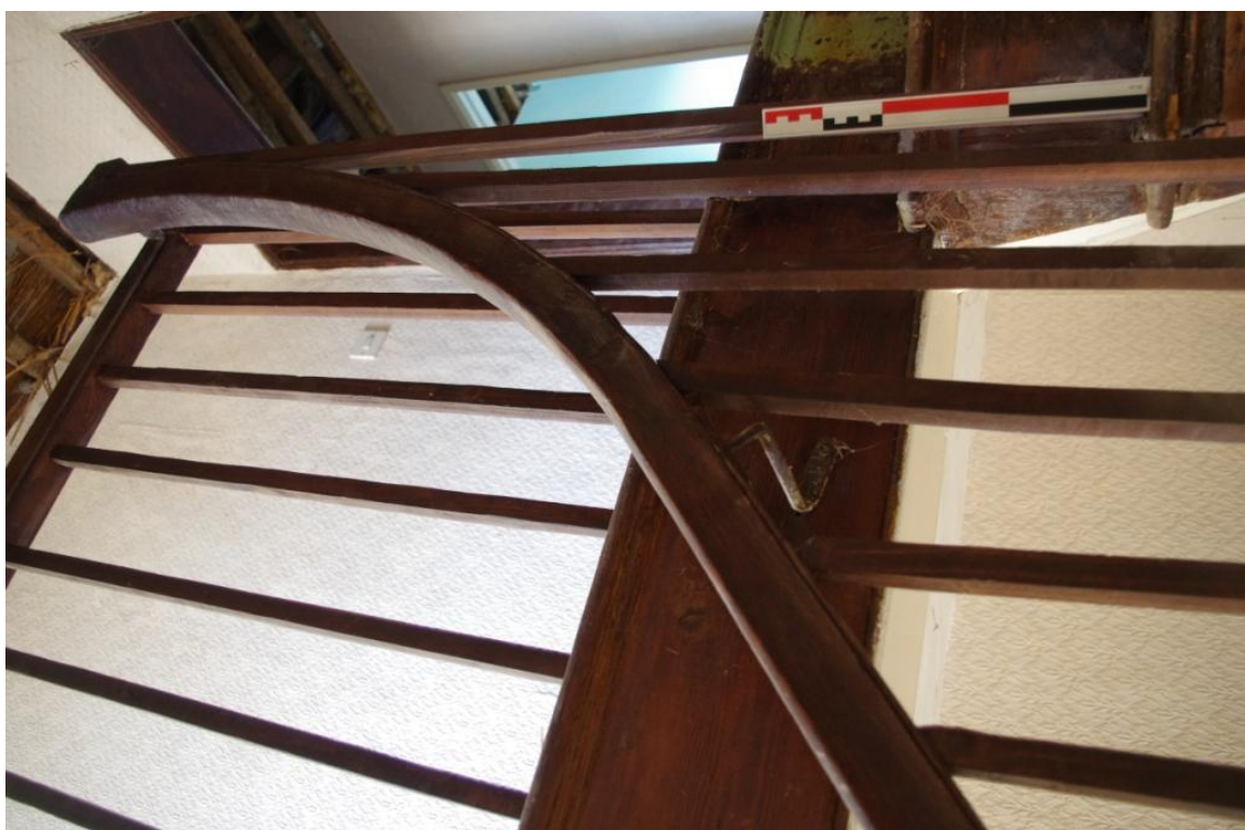
Figure 18 Ramped Handrail on First Floor (Looking West).
