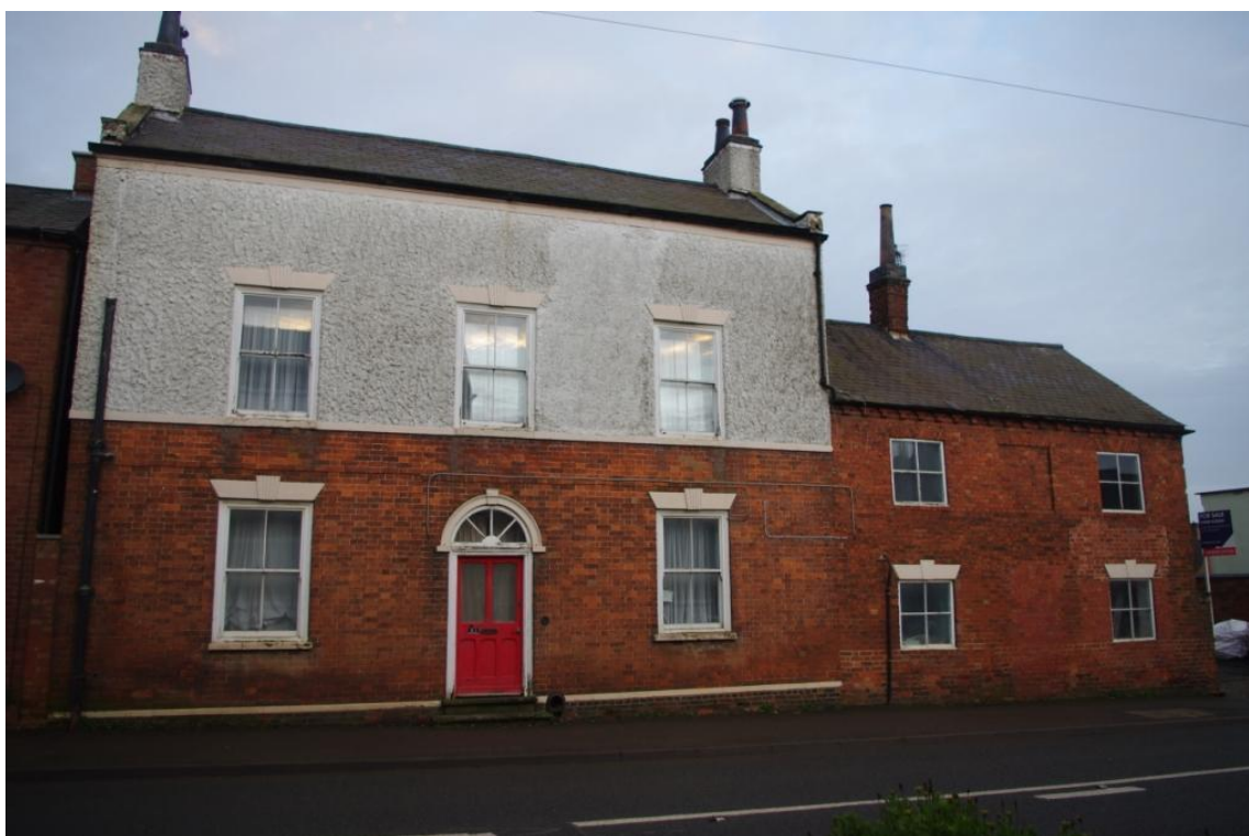
Figure 7 Principal Elevation, General View (No. 31 Left (Looking North)).
