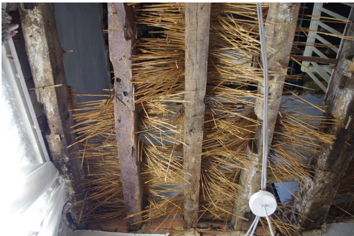
Figure 20 (13), Exposed Water Reed Floor & Reused Joists (Looking South West).
