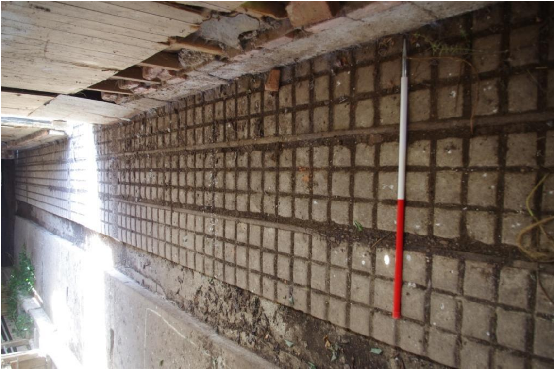
Figure 7 (5) Rails (Looking North East).
