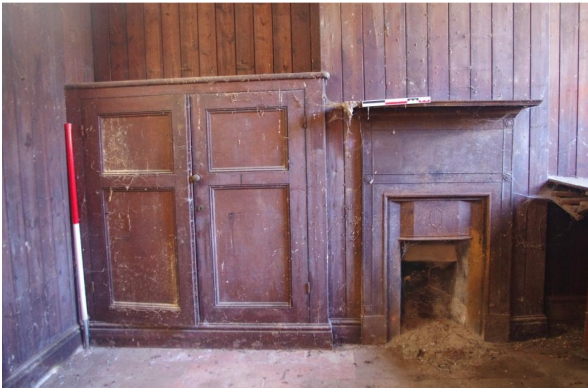
Figure 8 (1), Fireplace & Fitted Cupboard on South East Gable (Looking South East).
