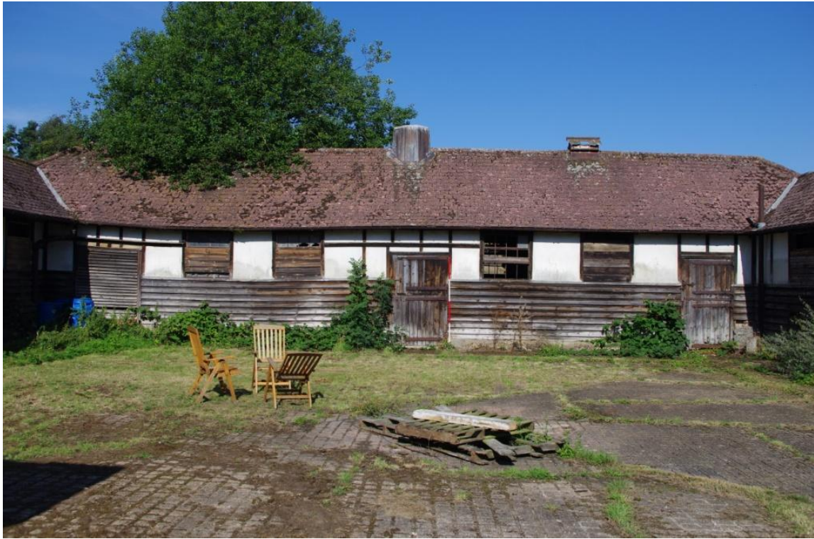
Figure 5 North West Range Principal Elevation, General View (Looking North West).
