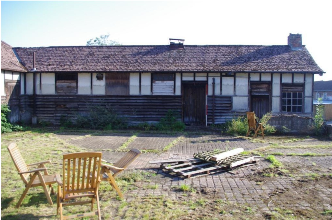
Figure 3 North East Range Principal Elevation, General View (Looking North East).
