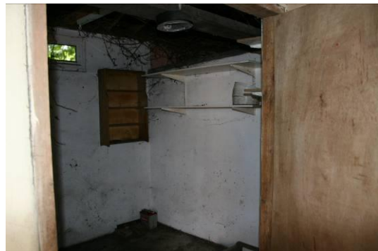
Stalls 1 and 2 (from the west). Windows in Stall 2 define an earlier mono-pitched building.
