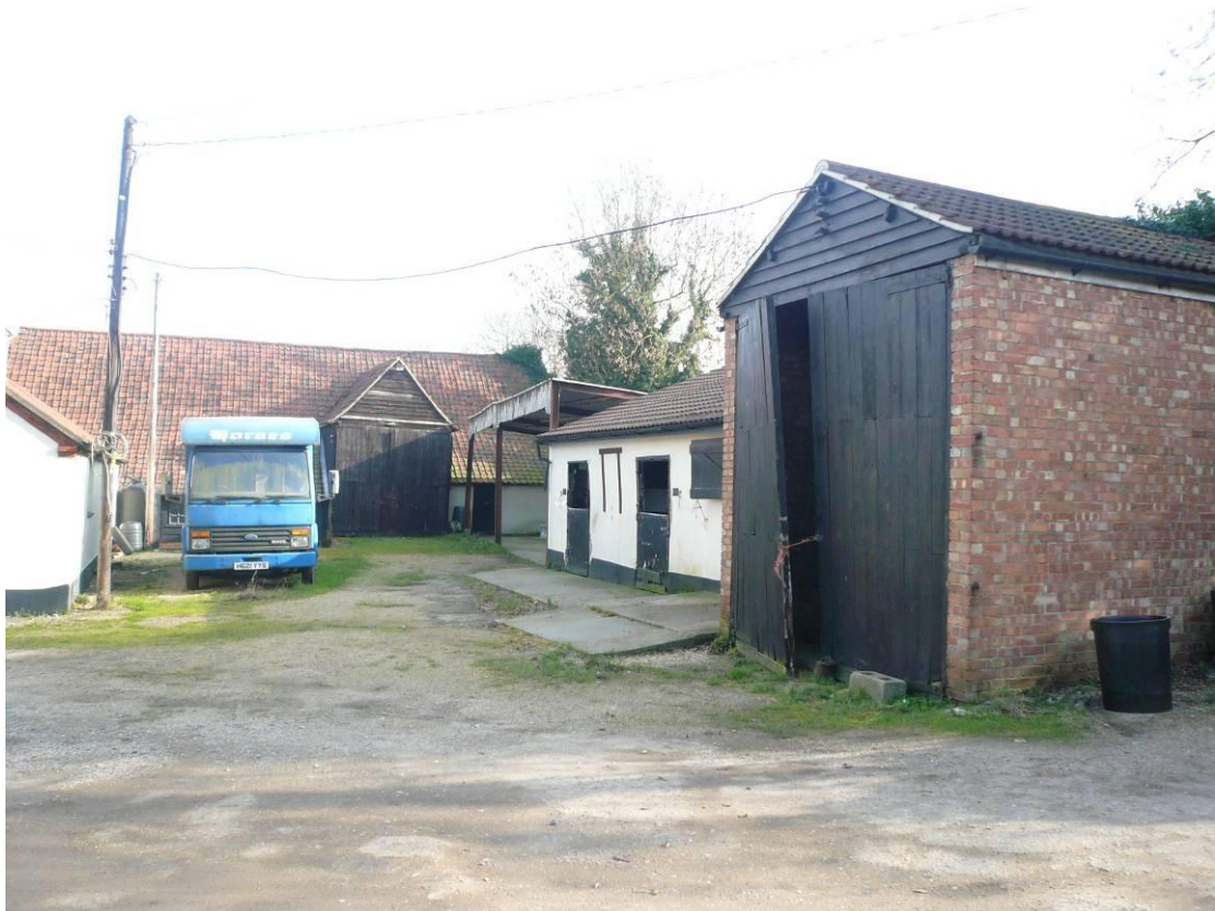
The west side of the Barn in 2011.
