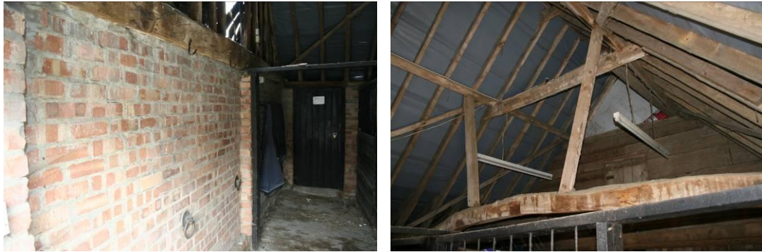
Corridor leads to northern outshut. Side purlin roof similar to the eastern bays.
