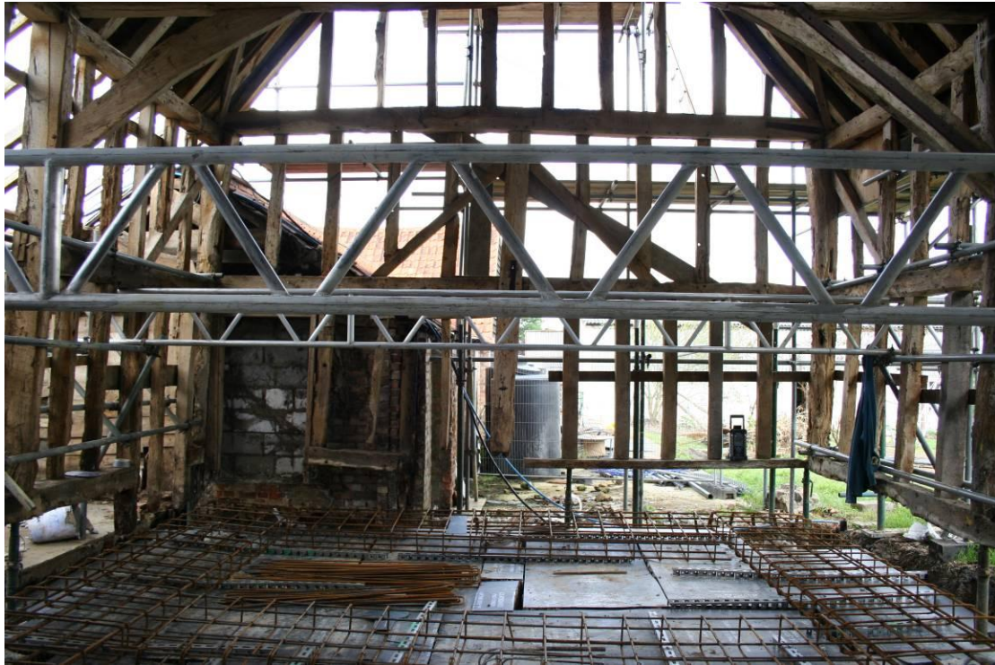
The northern elevation. Note opening for door into East Stables.
