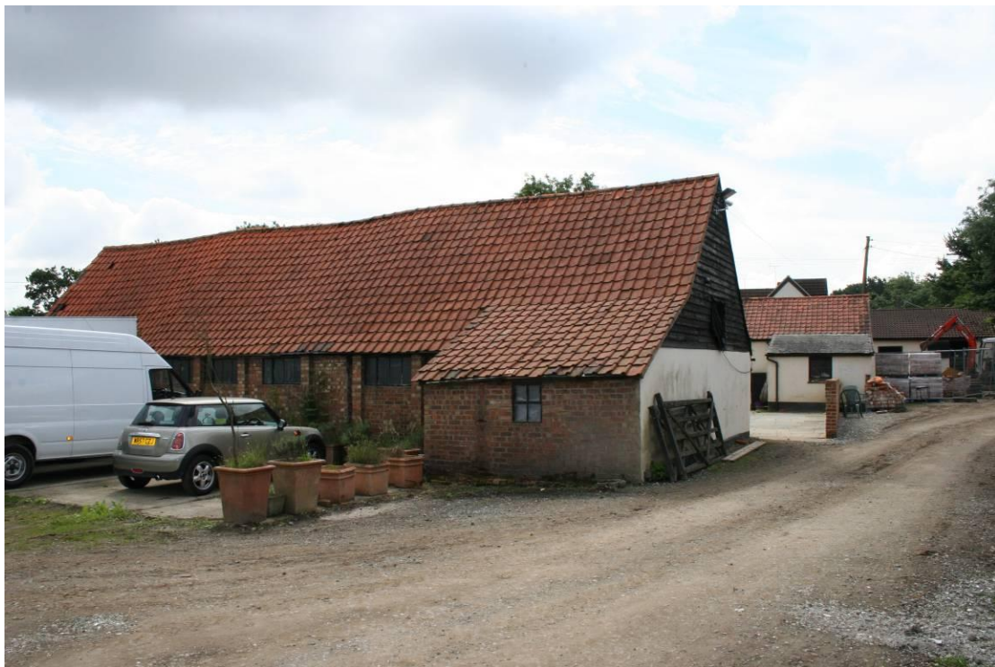
The North Stables from the NW.
