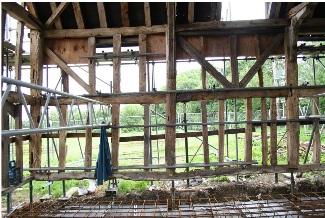
Bays 1 and 2 looking east.
