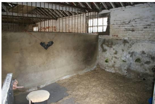
Stalls 1 and 2 (from the west) have blockwork partitions.
