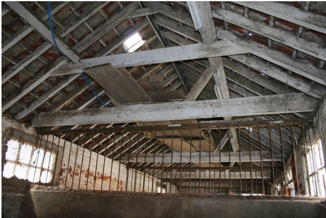
Roof structure looking west. Oak planks are stored on the tie-beams.
