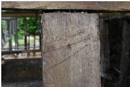
Variety of carpenter's marks on the Barn frame.
