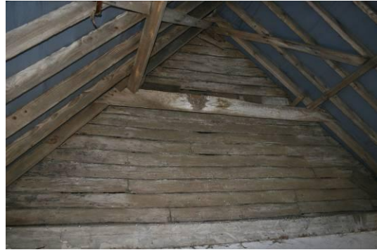
The eastern bay showing the stalls and the weather-boards on the partition. Looking NW.
