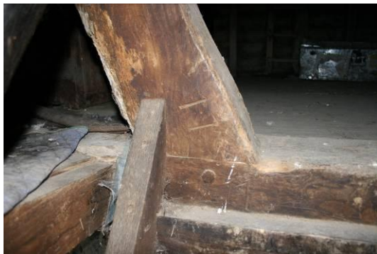
Carpenter's mark on the raking strut. Birds-mouthed struts reinforce the roof structure.
