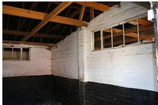
Stalls 1 and 2 (from the west). Windows in Stall 2 define an earlier mono-pitched building.
