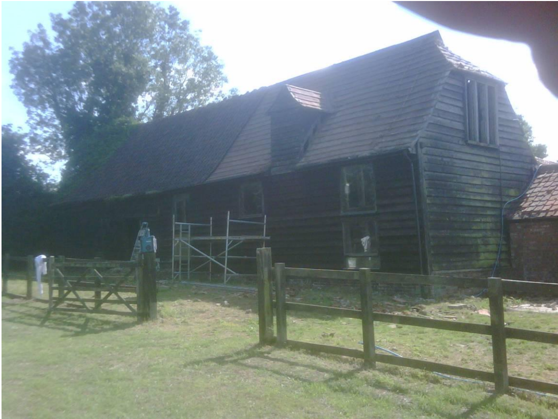
The east side of the Barn in 2011.
