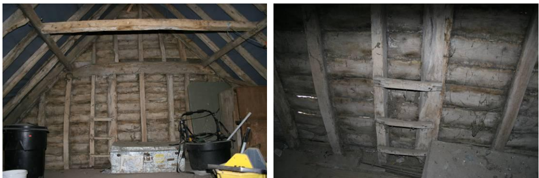
Timber framed eastern wall and C19th batten loft ladder.
