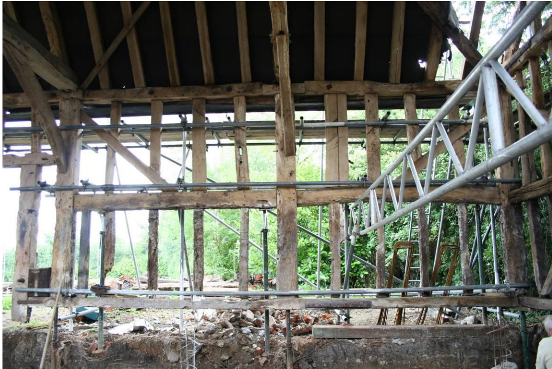
Bays 6 and 7 looking east.
