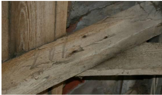
Merchants mark in the East Stables. C19th and C20th race knives and circle scribes.
