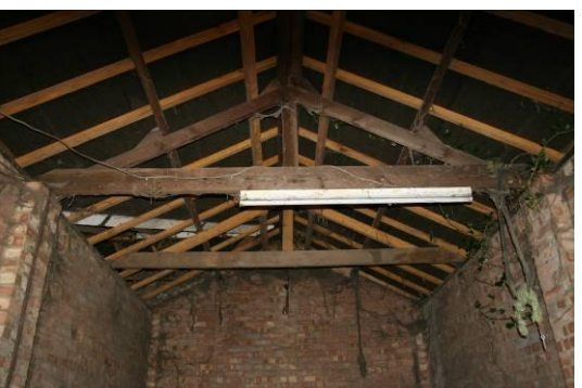
Blank interior and repaired roof using a C19th machined timber truss.
