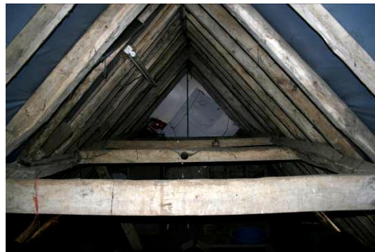
Carpenter's mark on the raking strut. Birds-mouthed struts reinforce the roof structure.
