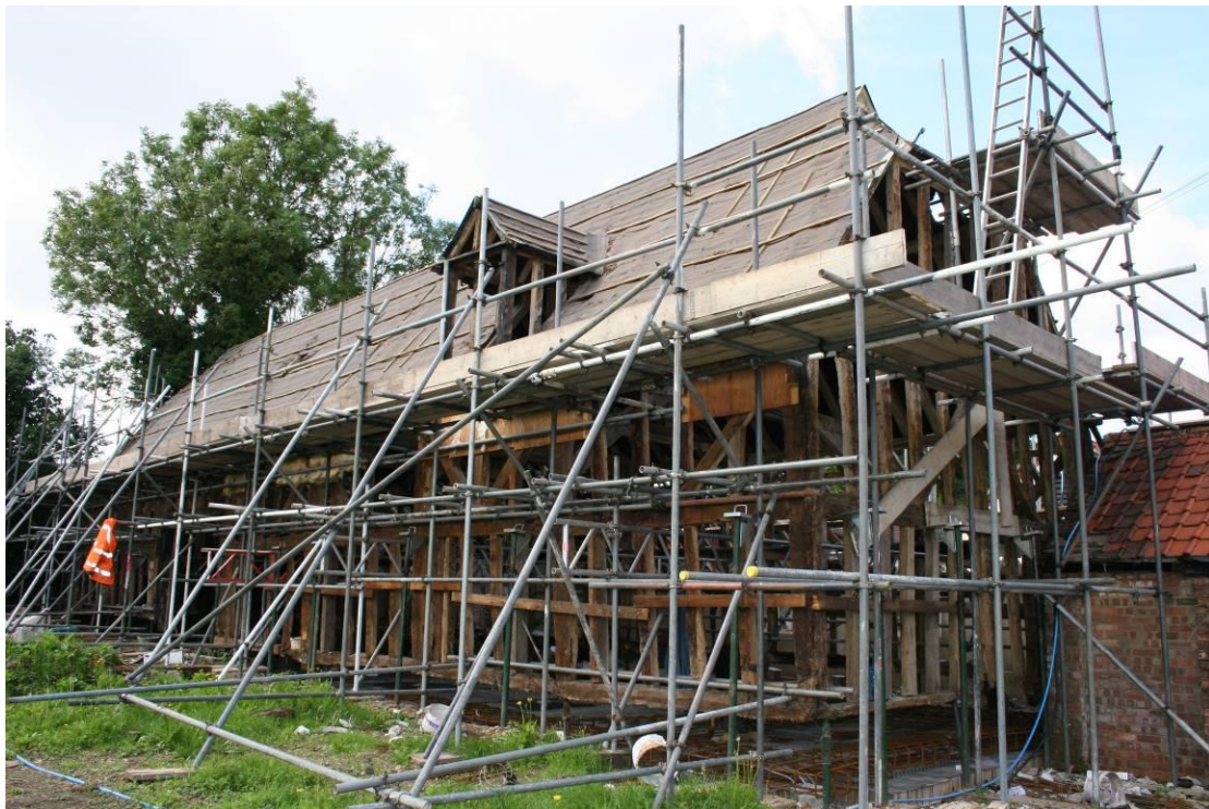
North and eastern elevations.
