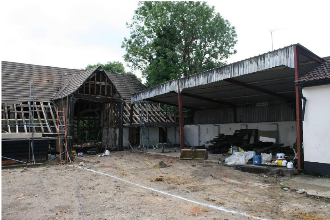
Asbestos roofed shelter. Looking SE.
