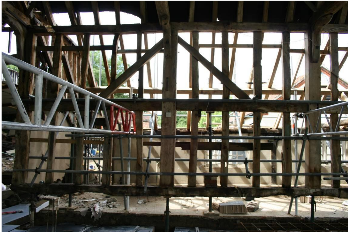
Bays 3 and 4 looking west.
