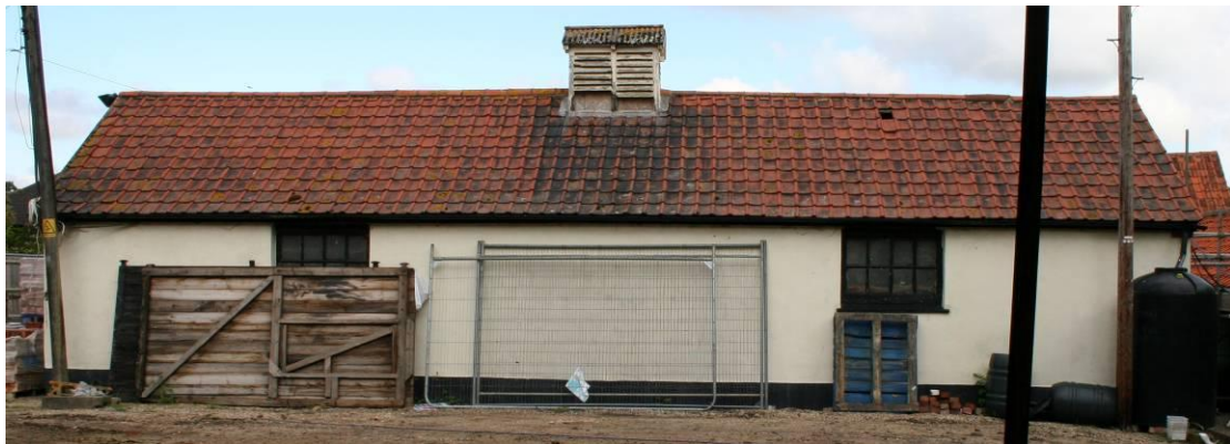
South elevation of the Central Stables.
