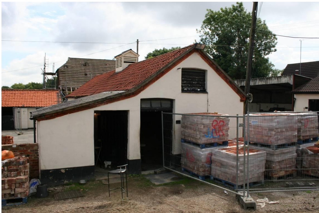
The Central Stables from the west.
