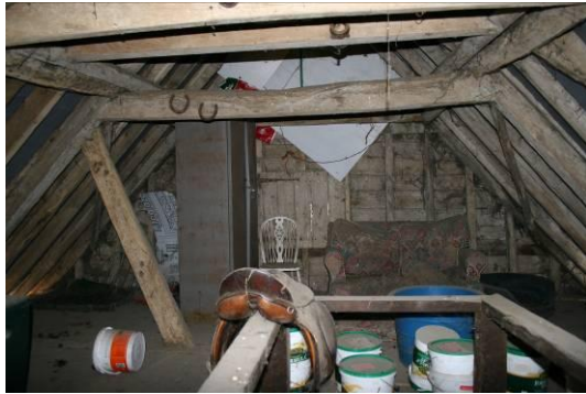
Loft looking west at the central hatch door.
