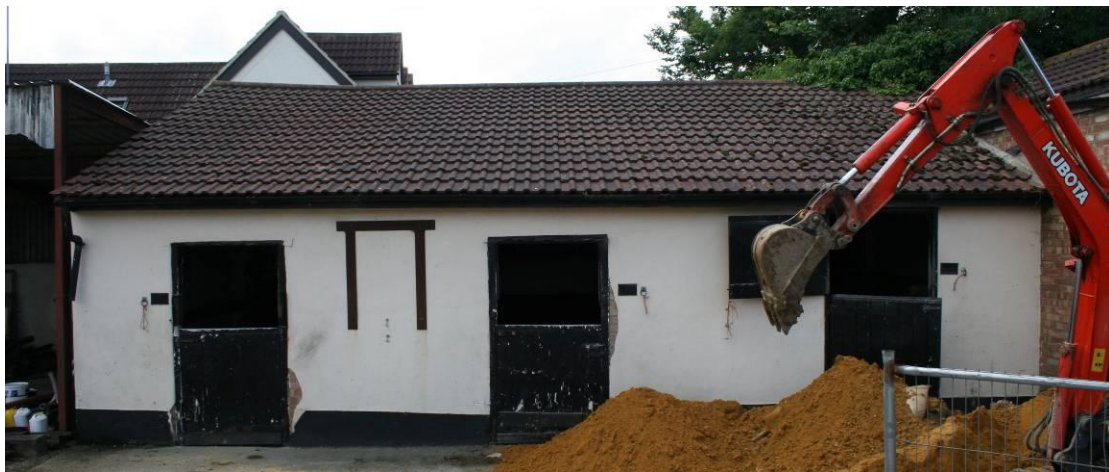
Northern elevation of the South Stables.
