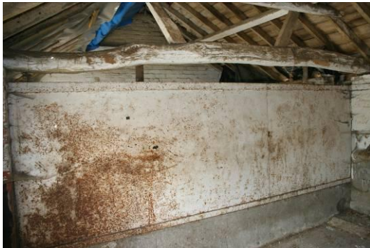
Stalls 1 and 2 (from the N) are separated with a steel sheet.
