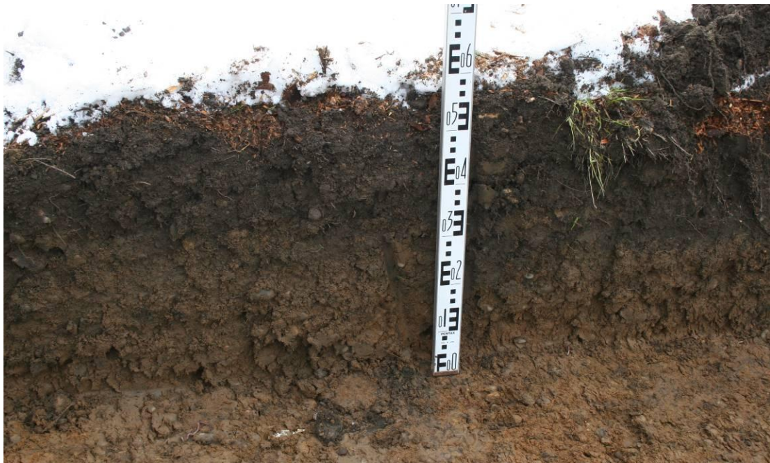
Typical section. 250mm of modern topsoil. A 250 -300mm deep spit was cut into the subsoil.
