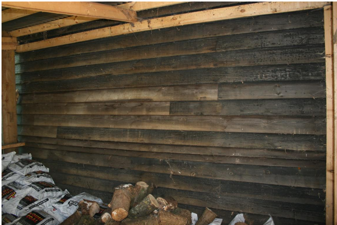
The western elevation inside the Shed.
