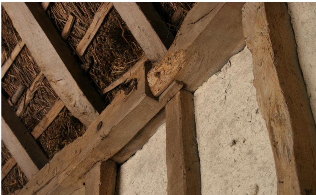
Detail of the forelocked scarf joint.
