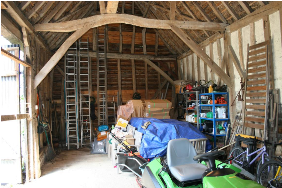
Looking W inside the Barn.
