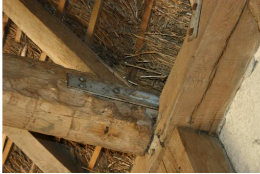
LC20th metal work repairs.
