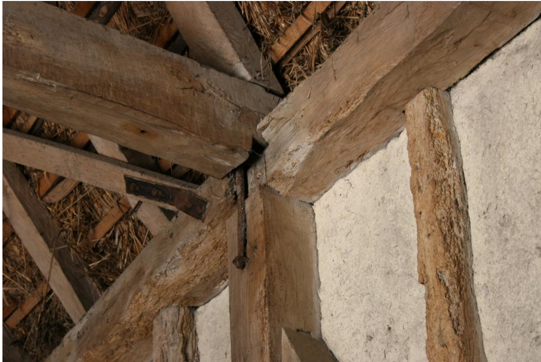
Detail of the principal post in Truss 2 (from W).
