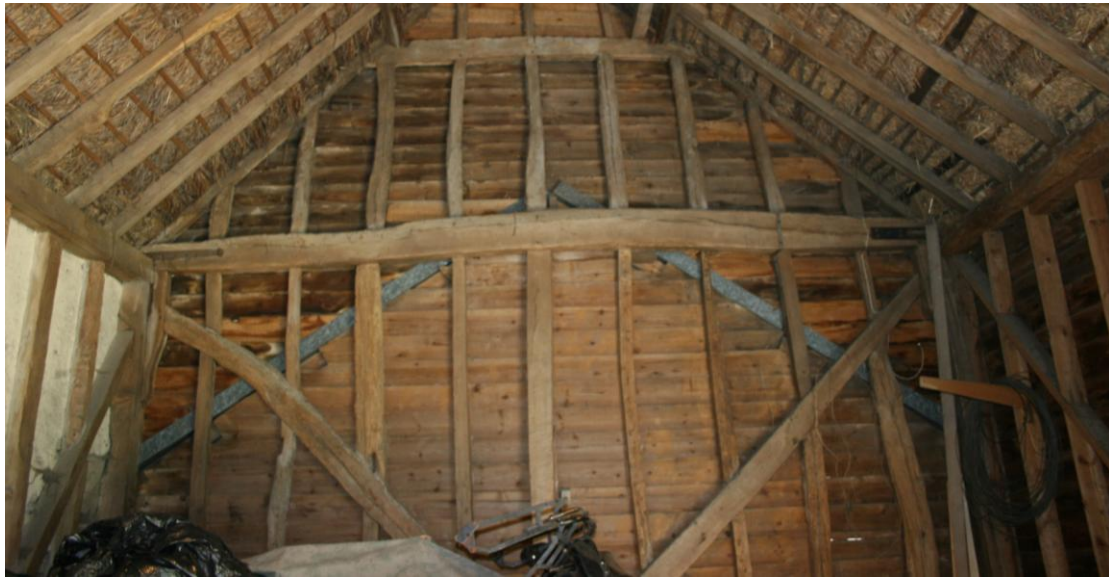
Detail of the eastern wall.
