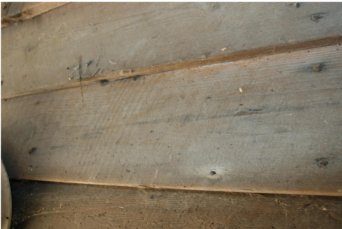
Detail of the weather-boards showing the circular saw marks and wrought iron nails.
