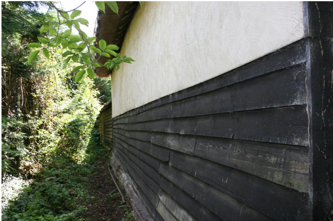
The northern elevation looking E.
