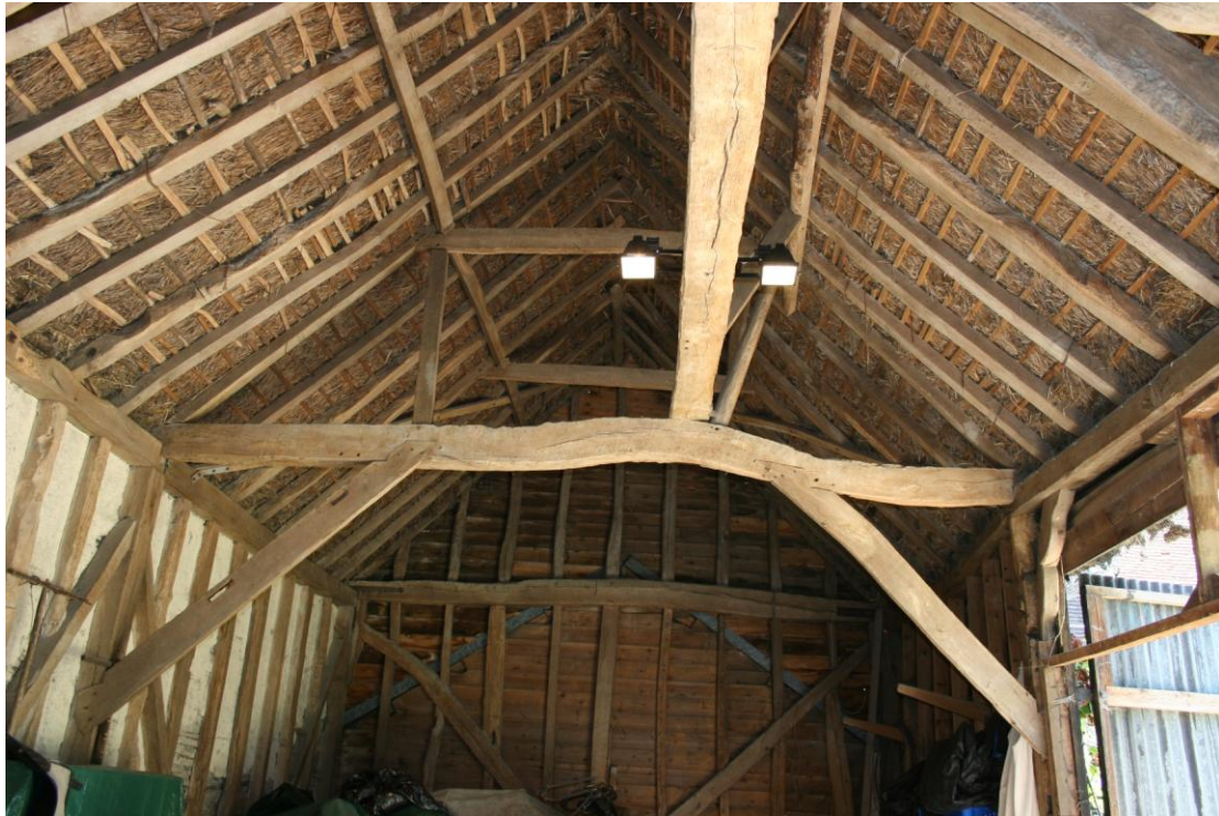
The tie beam in Truss 2 (from W).
