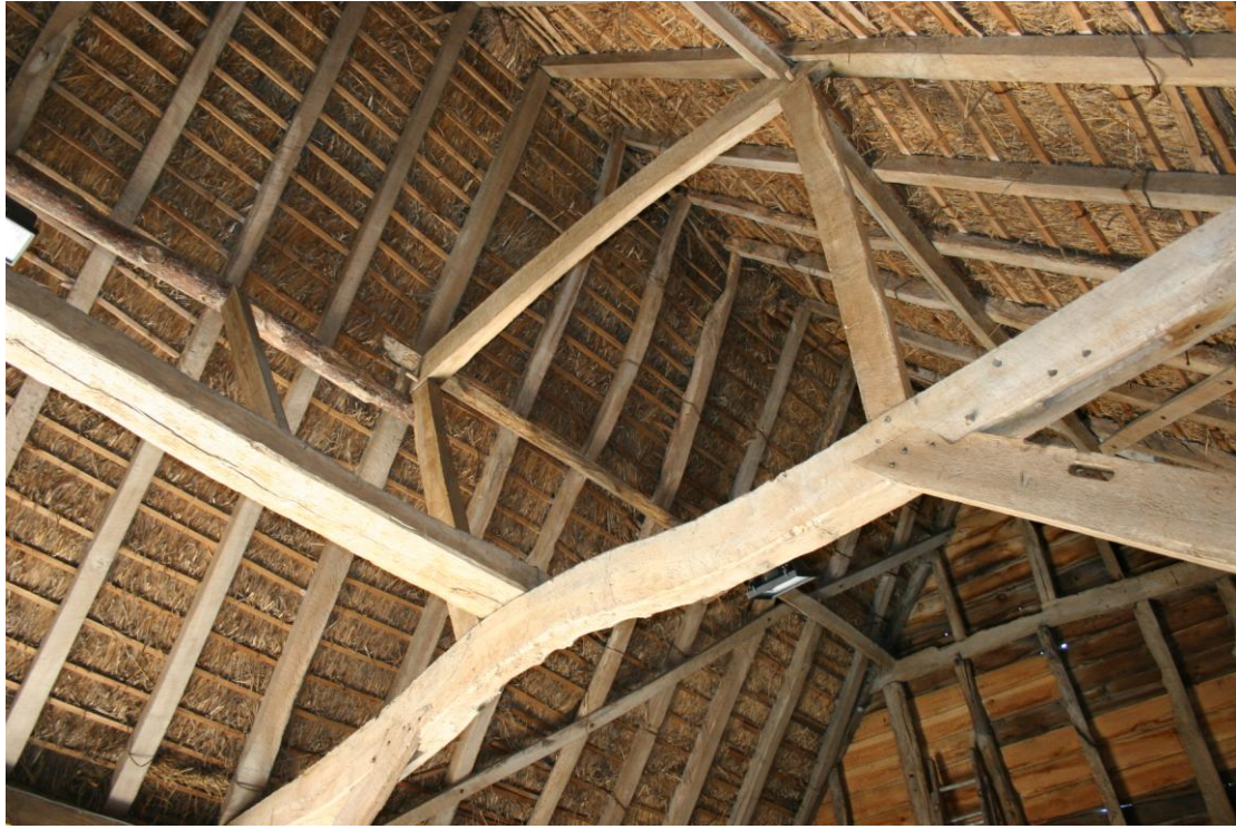
Looking upwards to the SW at the queen post roof.
