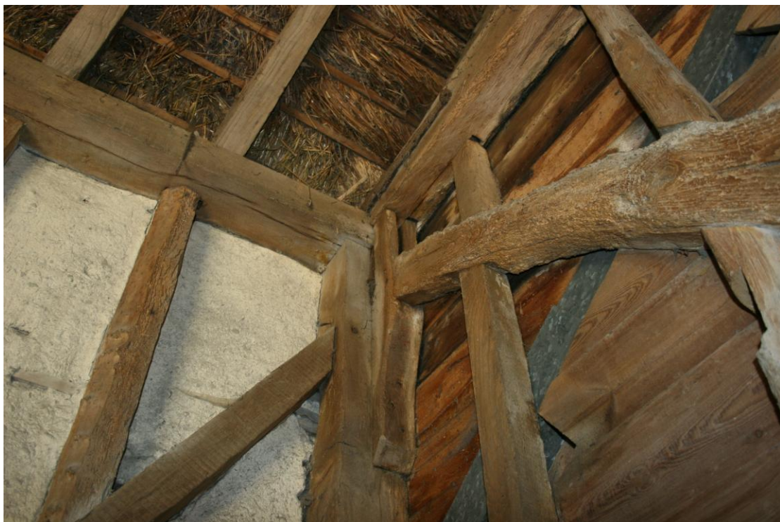
Detail of the NE corner post. Note the applied jowl piece.
