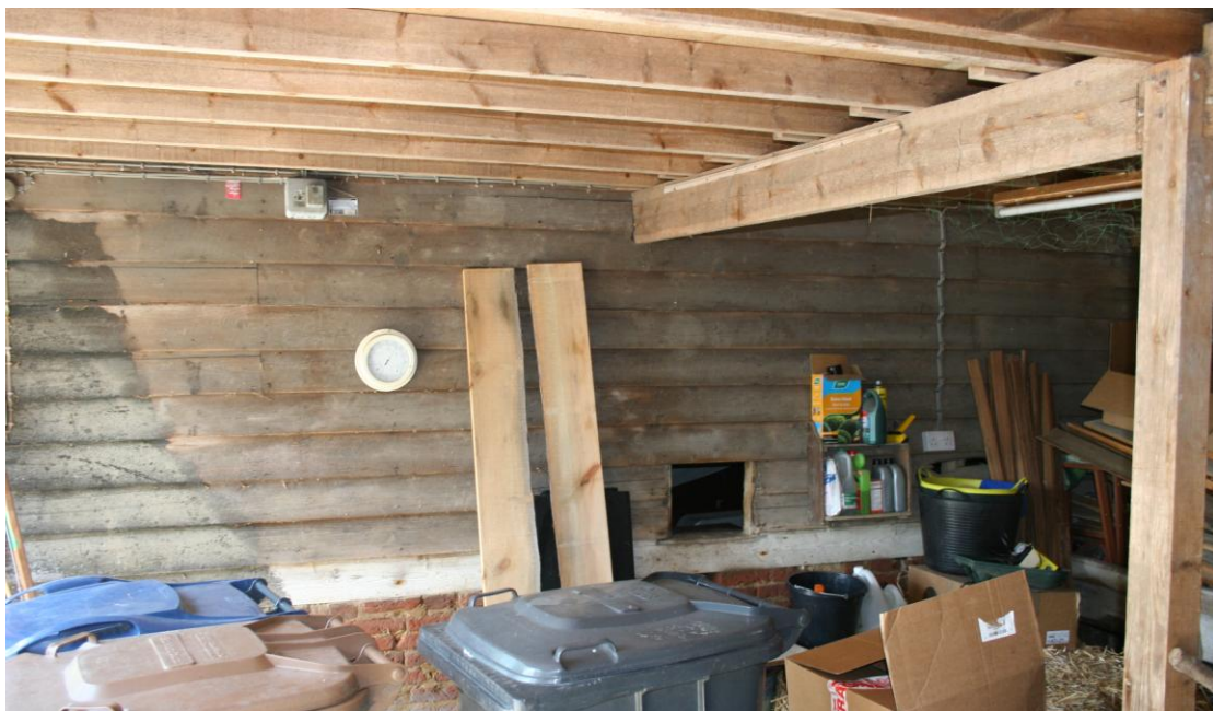
The eastern elevation inside the Shelter.
