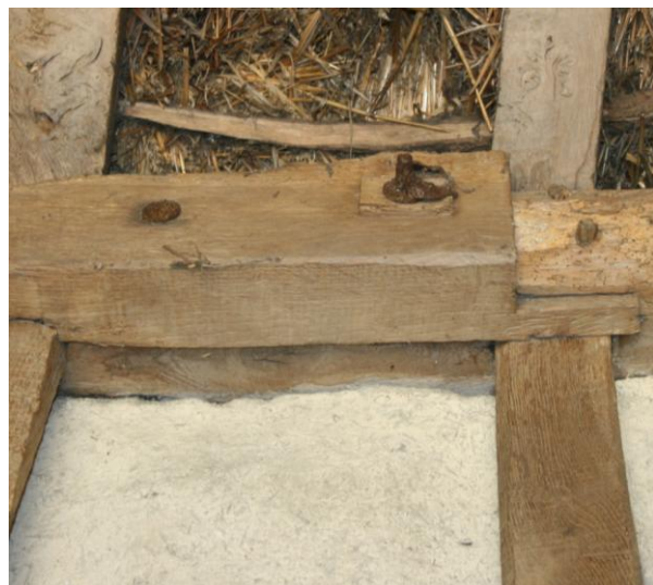
Pair of forelock bolts securing the scarf joint.
