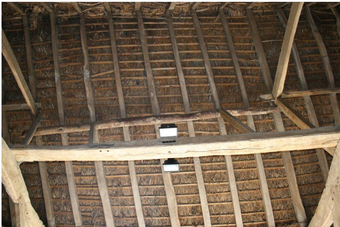
Detail of the thatch over the central bay/ Looking S.
