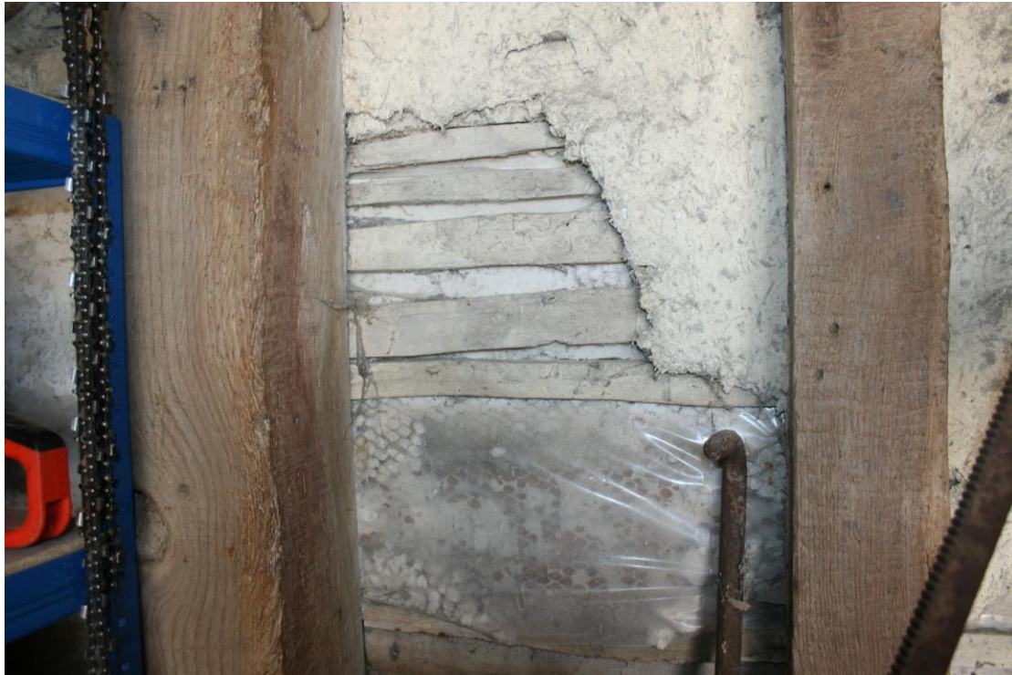
Detail of the north wall showing the layers of EML and lath and daub.
