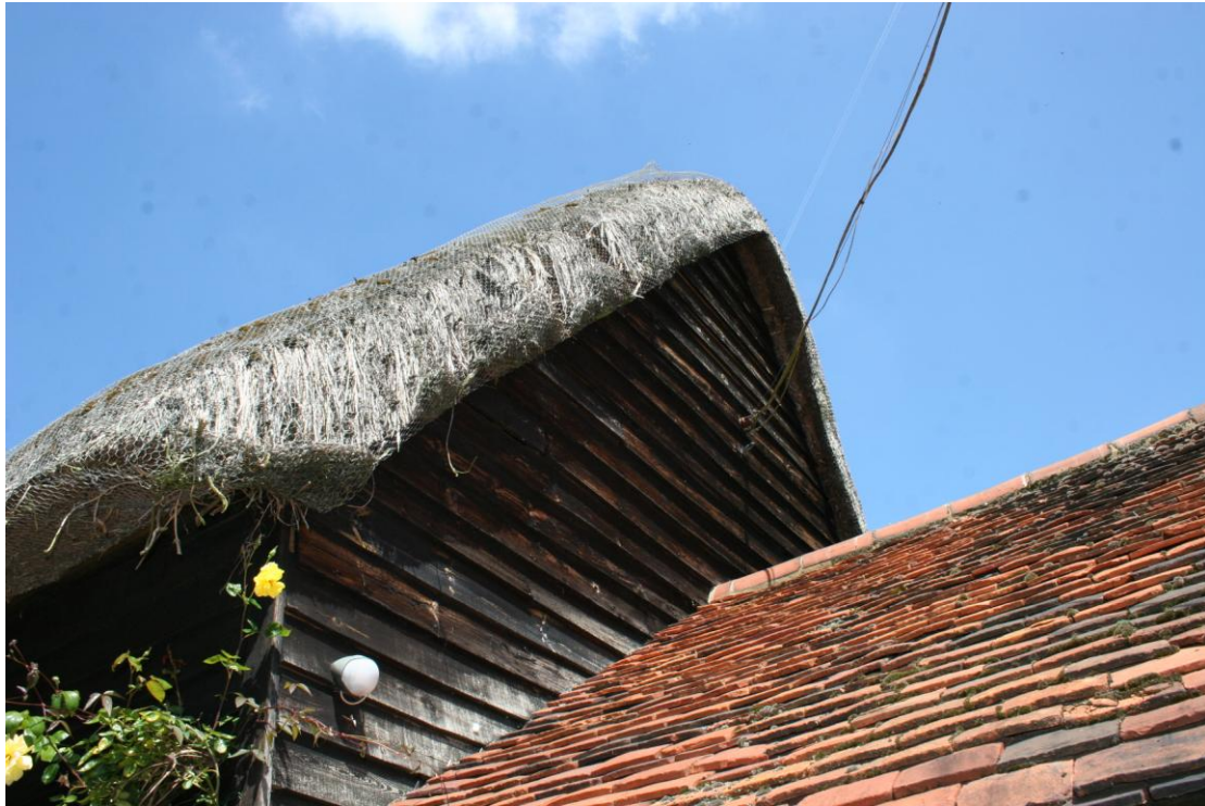
The eastern elevation. The exposed section has LC20th boards clearly bandsawn.
