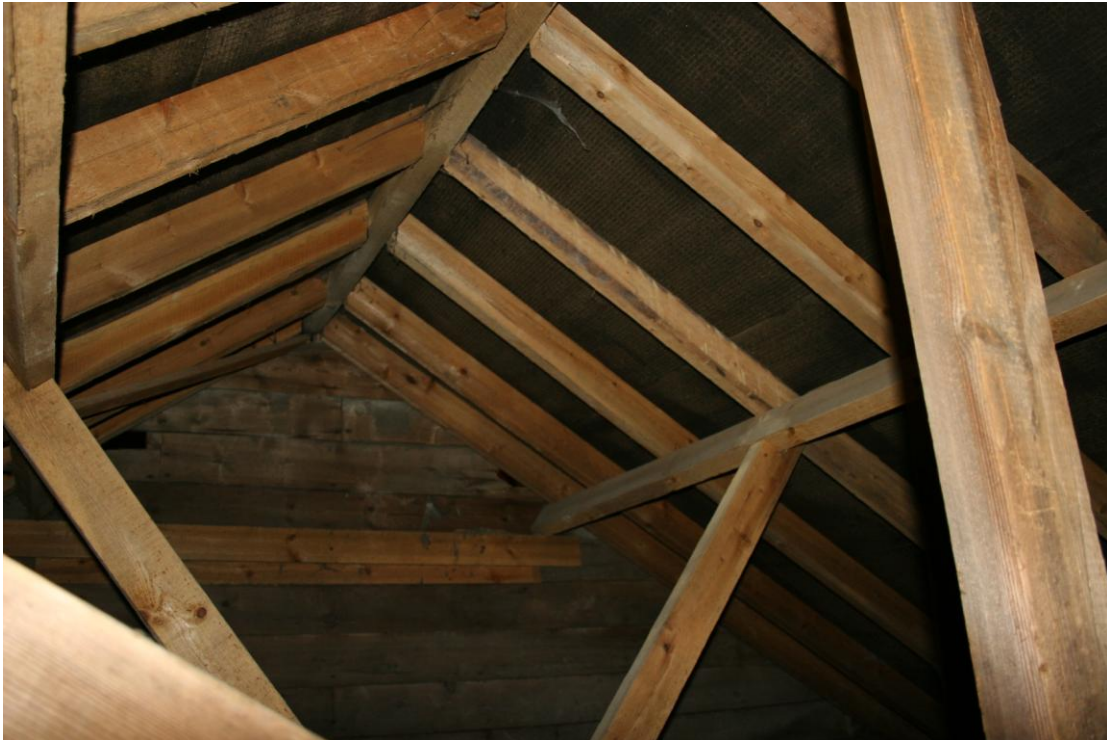
Looking at the eastern elevation through the recent structure.
