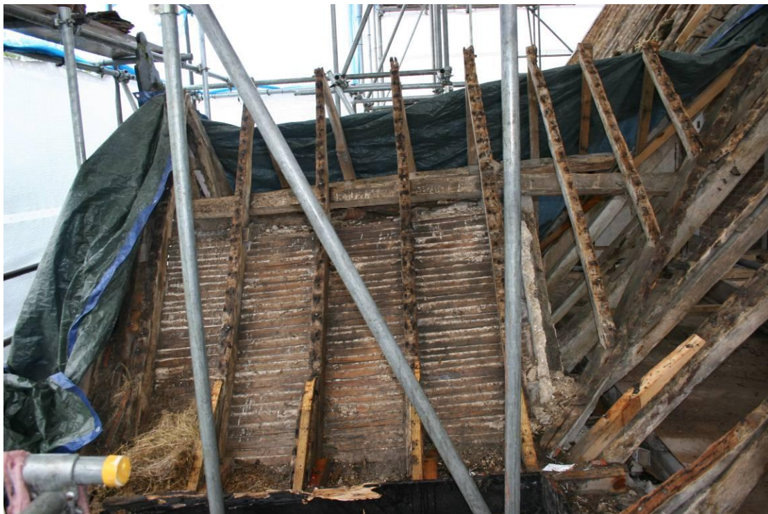
The porch roof looking W.
