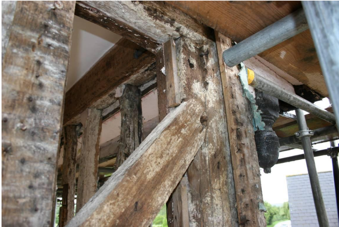
Reused primary brace nailed in position.
