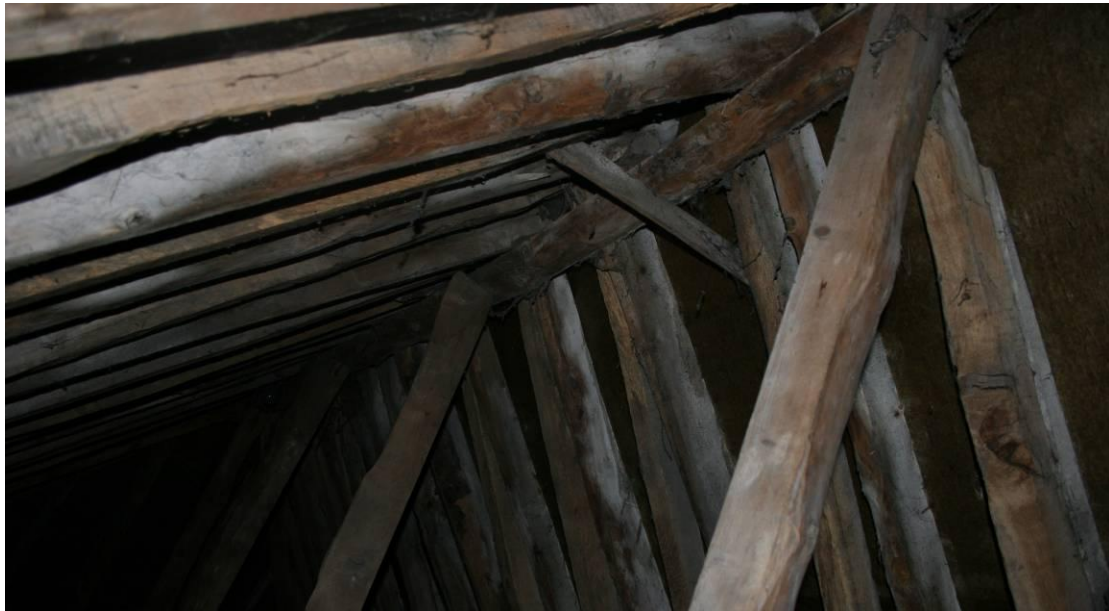
The apex of the rafters over the Rear Range looking N.
