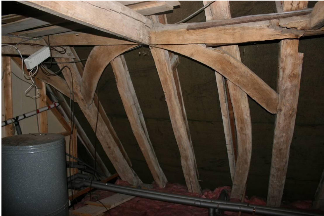
The windbraces seen in the eastern attic. Looking NW.
