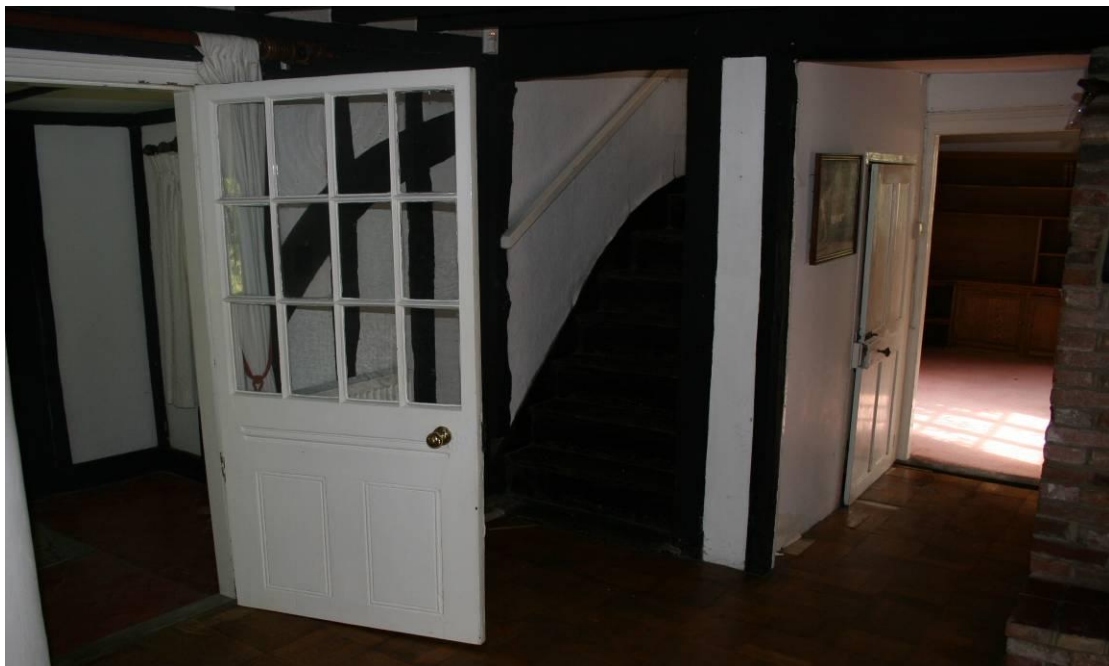
Looking SW towards the stairs and doorway down to the Cellar.
