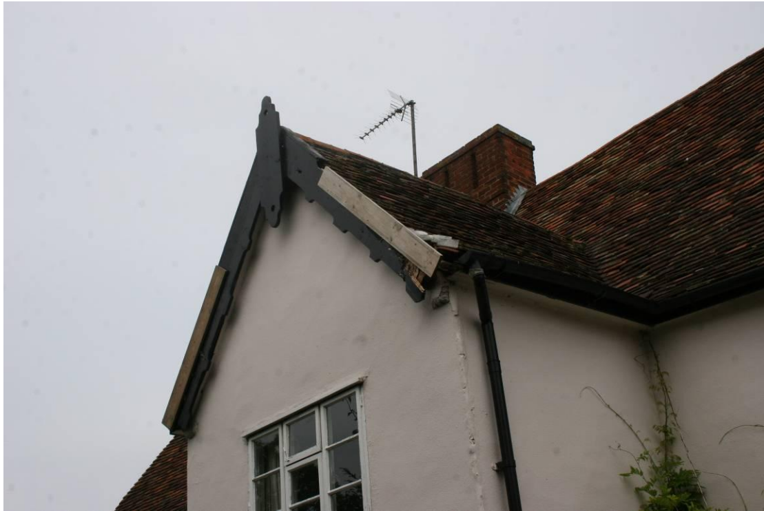
Detail of the porch. The crude boards are likely C20th.
