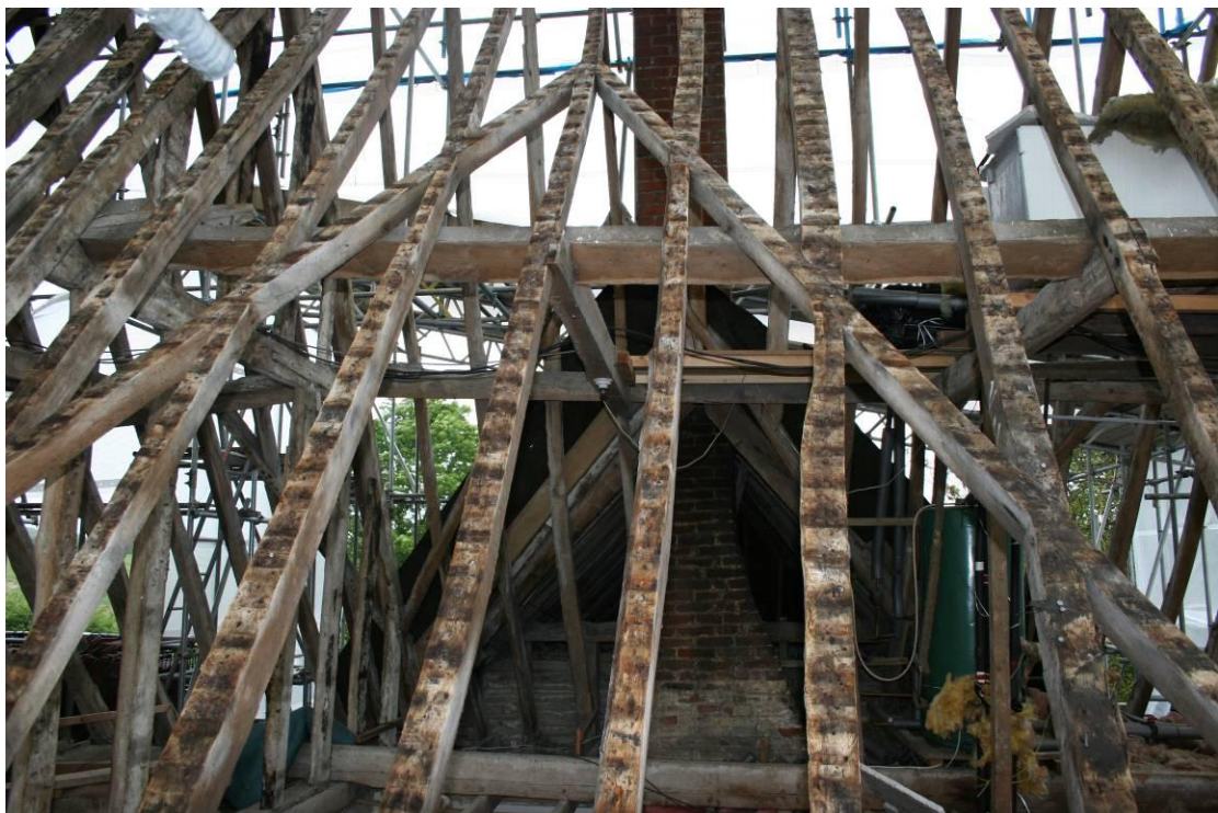
Detail of the primary bracing.
