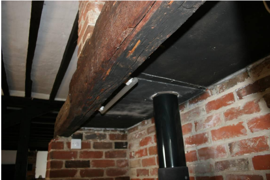
Detail of the bressummer and modern brickwork.
