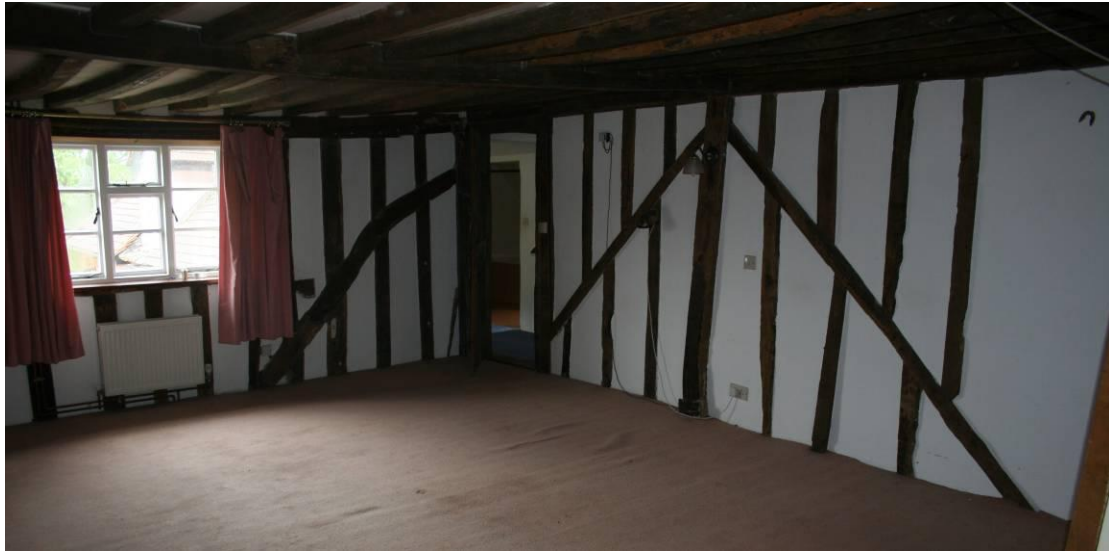
Master bedroom looking NE.
