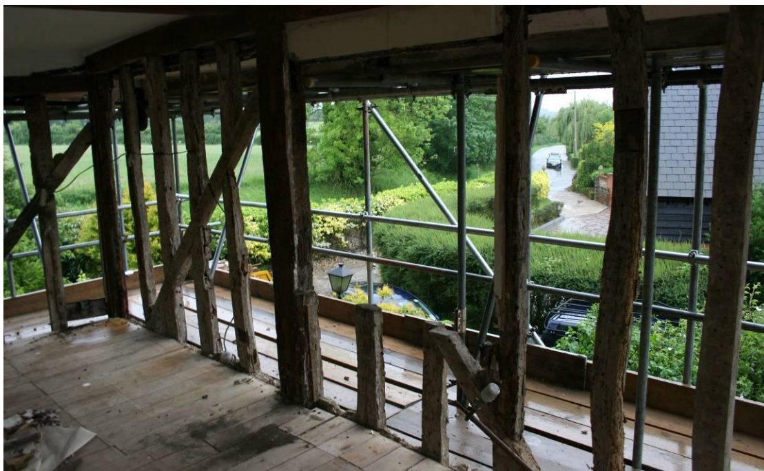
The western wall on the first floor looking SW.
