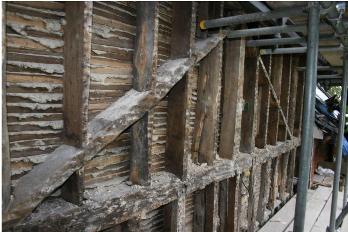
The frame of the eastern wall just below the jettied gable.
