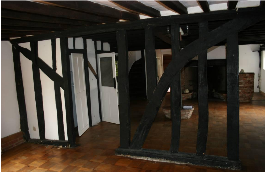
The frame of the wall common with the Living Room.
