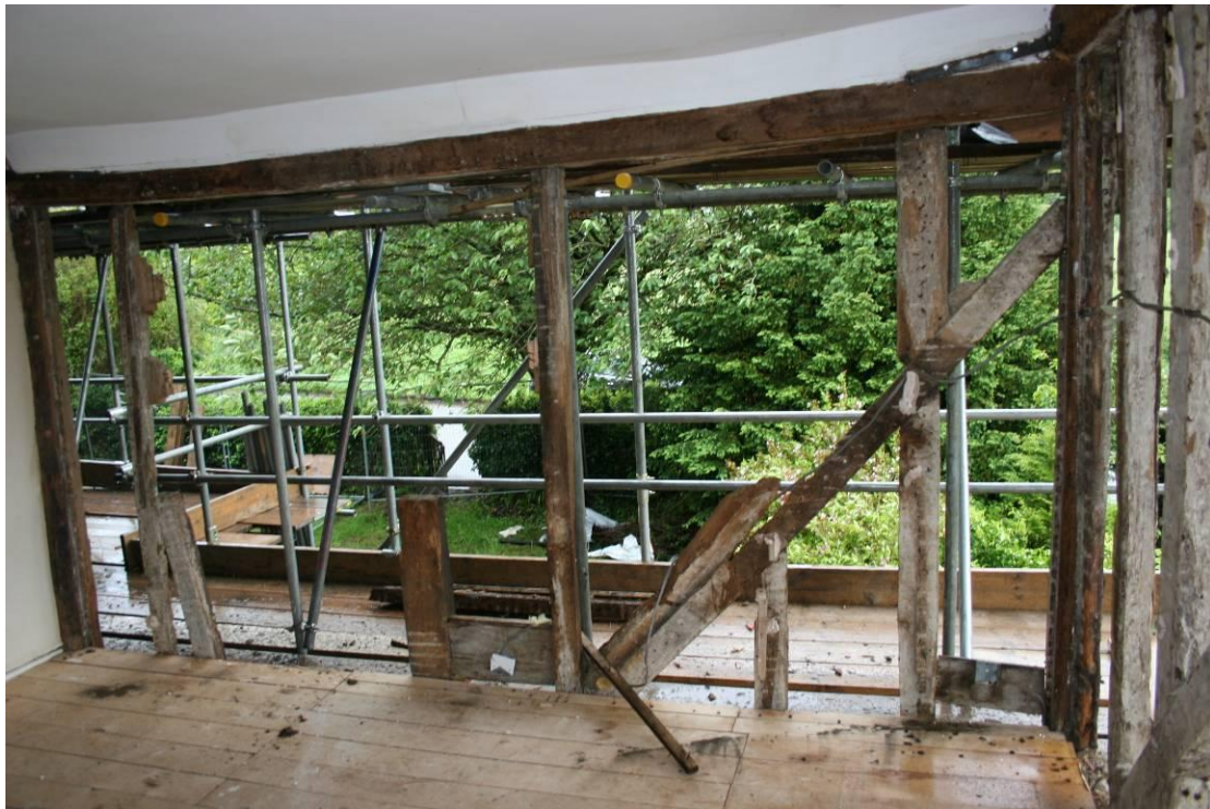
Looking S out of the front of the house.
