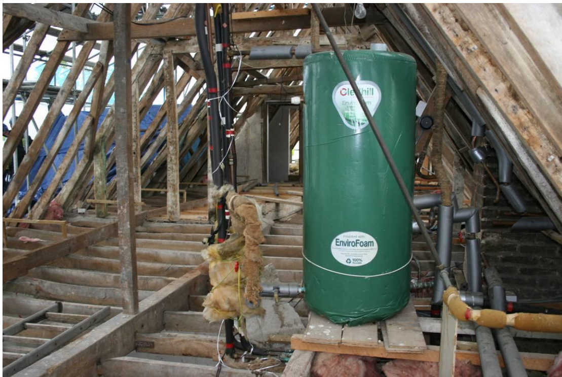
Looking W across the frame above Bedroom 2.
