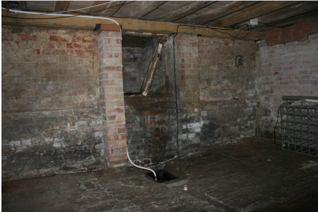
Looking NW in the Cellar.
