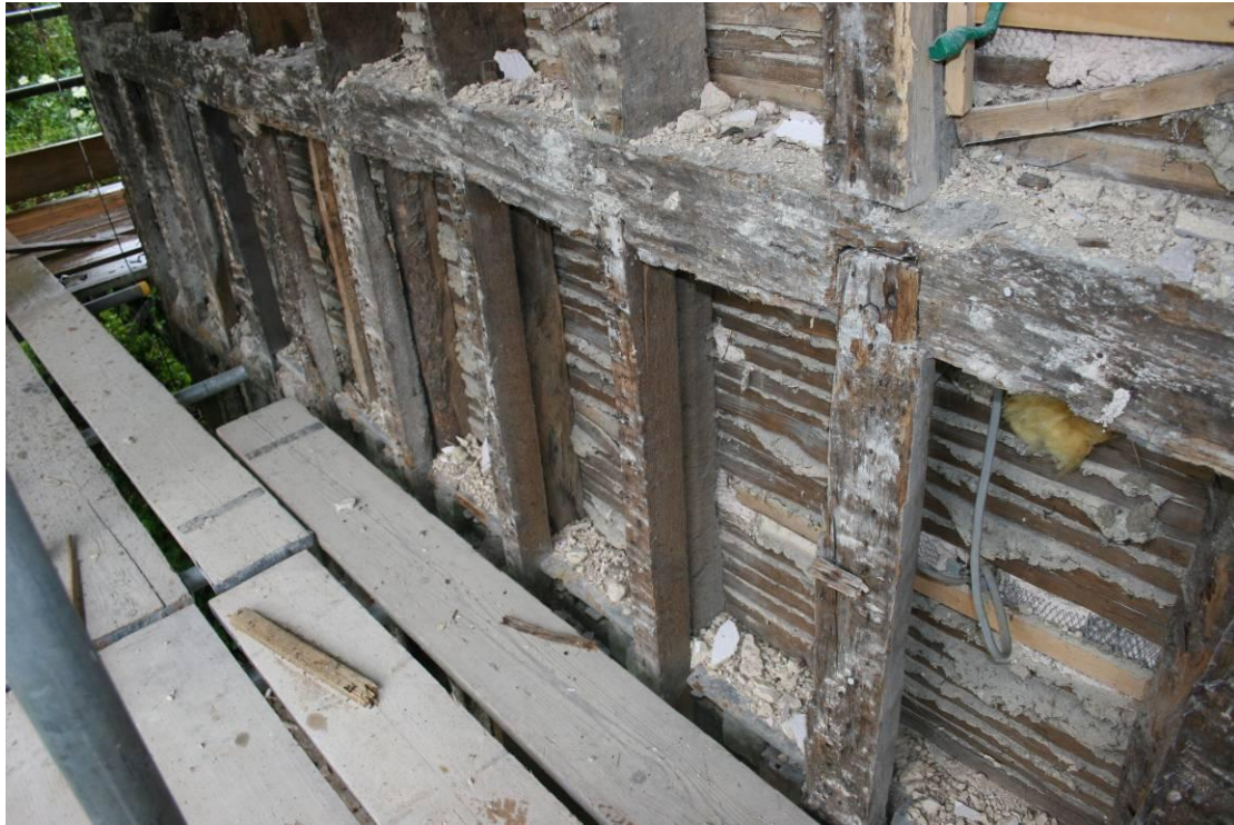
Skew nailed studs.
