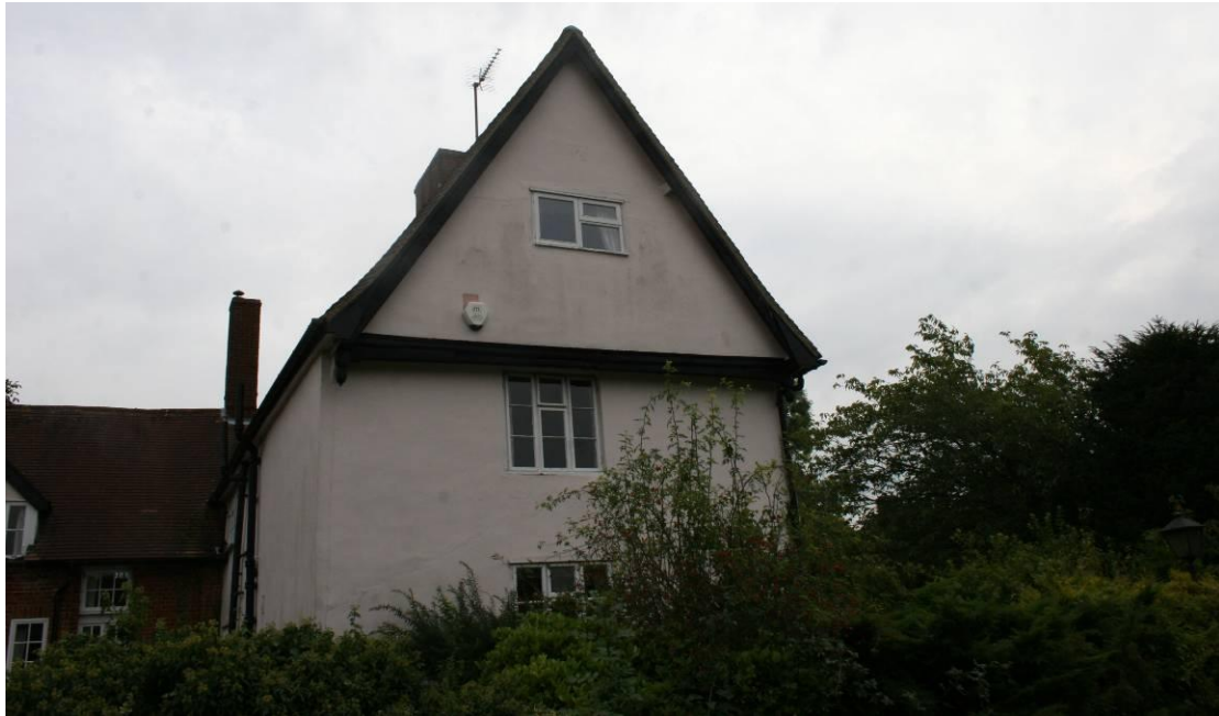
The western elevation of the timber-framed house.
