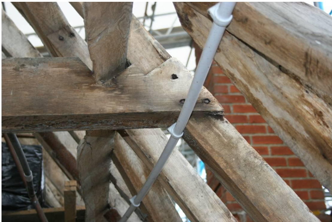
Detail of lapped and side nailed collar.
