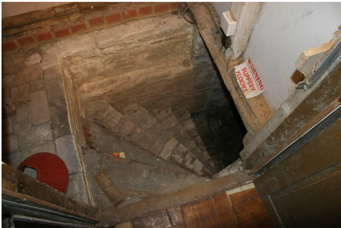
The brick steps down to the Cellar.
