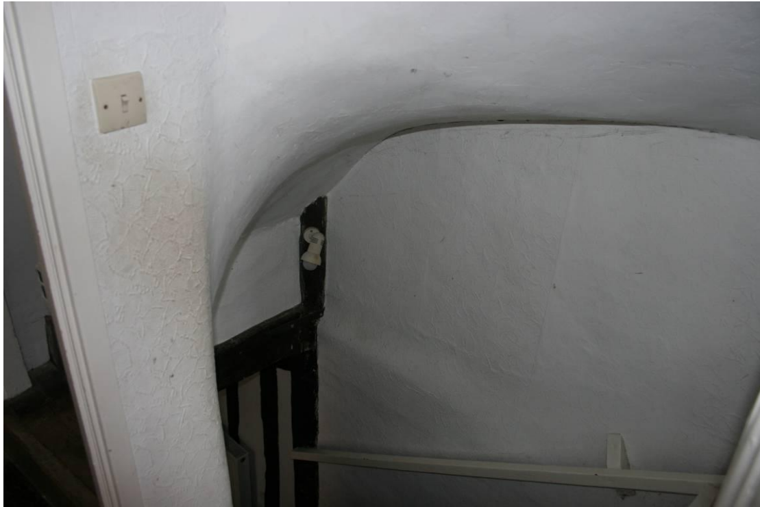
The soffit of the winder stair up to the attics.
