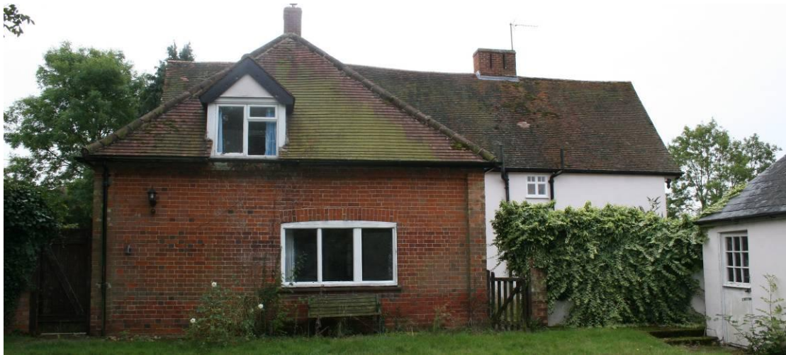
The northern elevation of the Rear Range.
