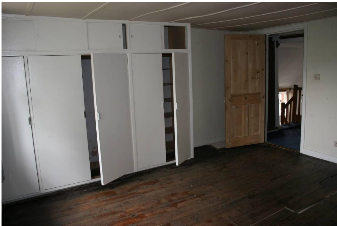
Looking NE in Bedroom 2.
