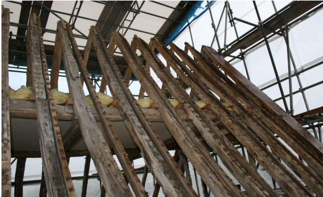
The roof over the Western Attic Room. Bedroom 4.
