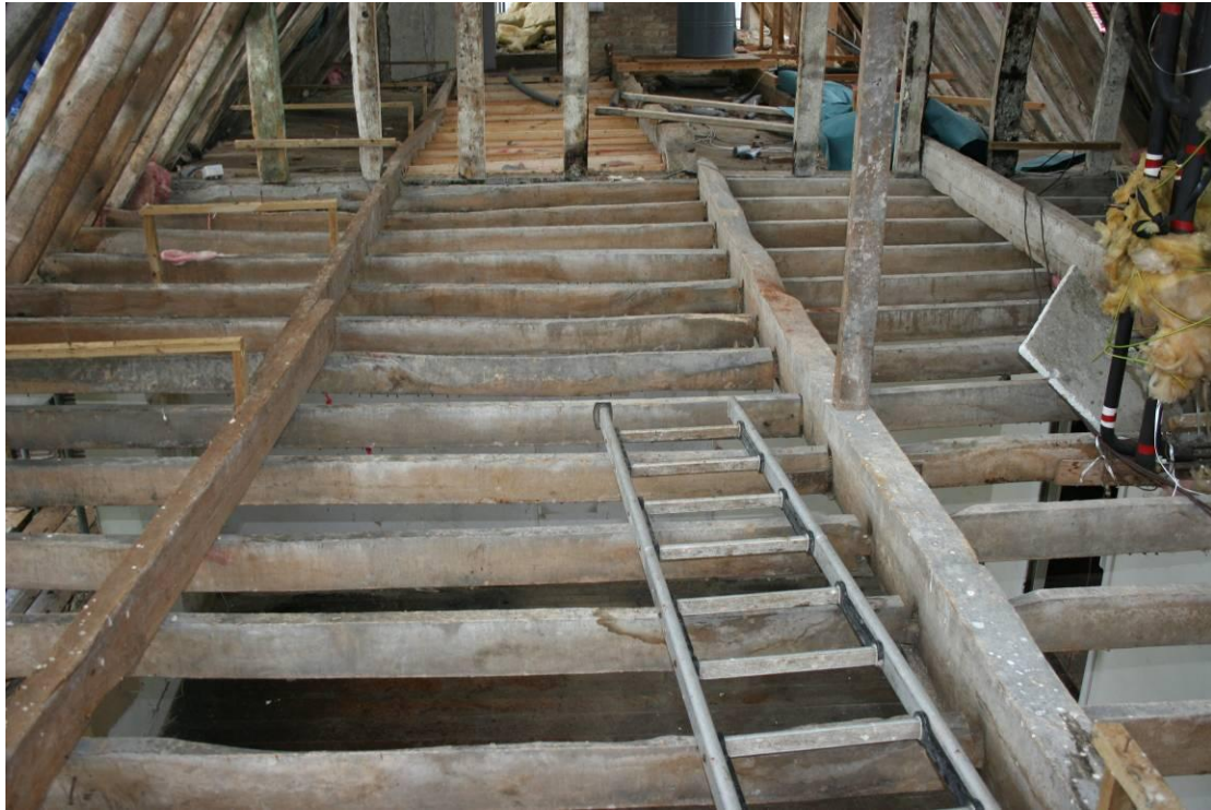
The frame over Bedroom 2. Looking W
