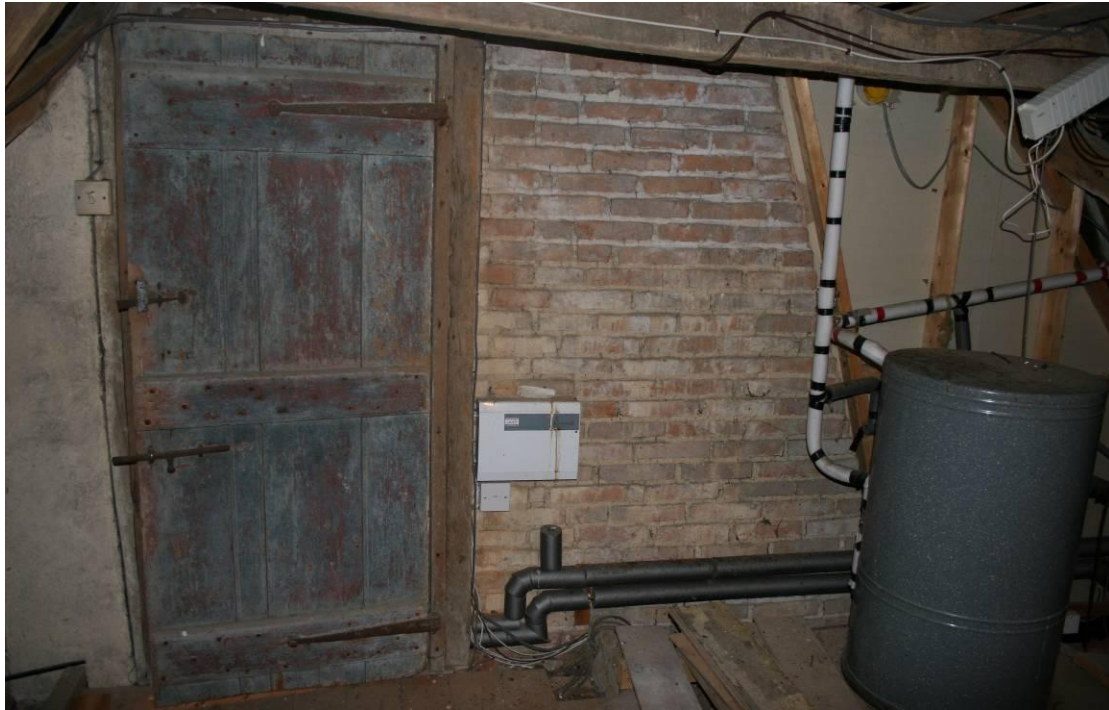
The EC19th door into the Eastern Attic.
