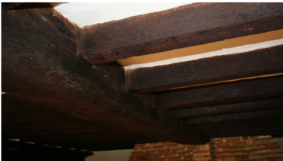
Detail of the main and common joists.
