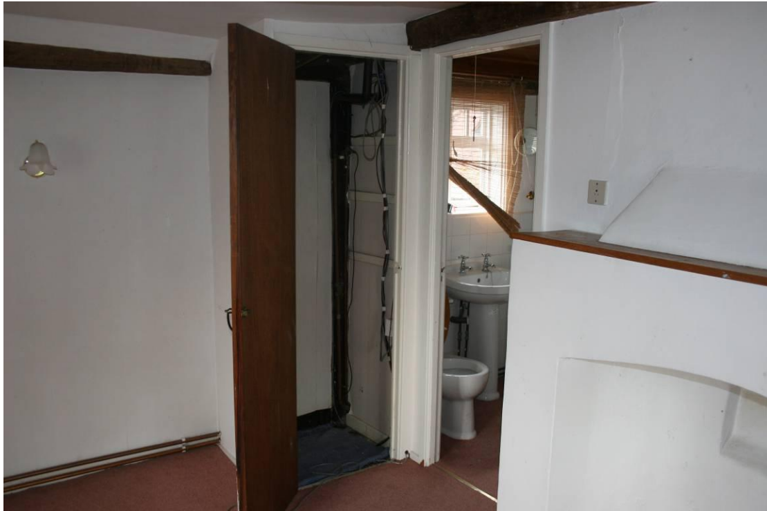
Airing cupboard in Bedroom 1.
