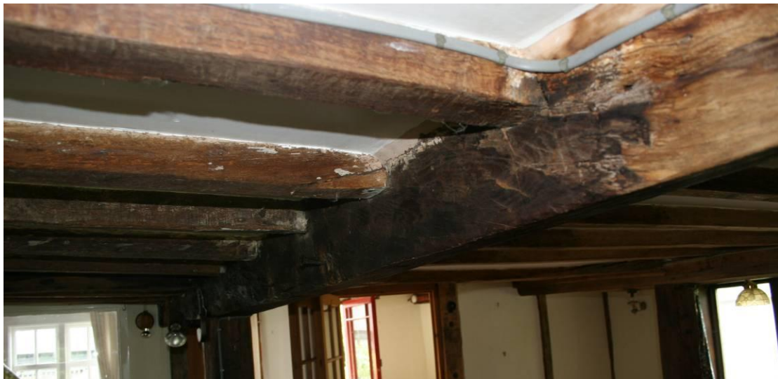
Detail of the frame over the Kitcehn.
