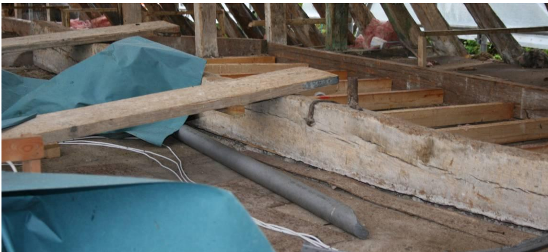
Detail of the forelock bolt and strapping. Looking SE.
