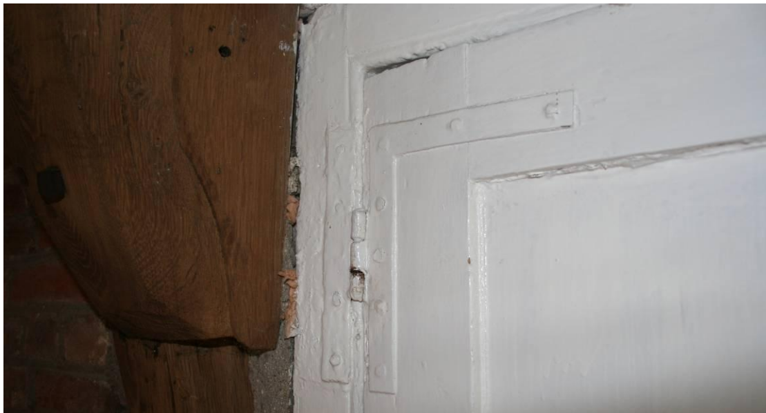
Detail of the door hinge.
