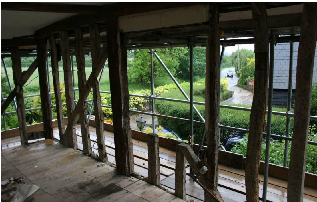
The stripped frame in Bedroom 1 looking SW.
