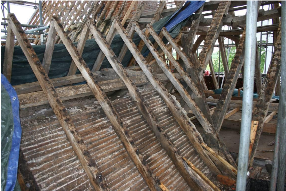
The porch roof looking NW.
