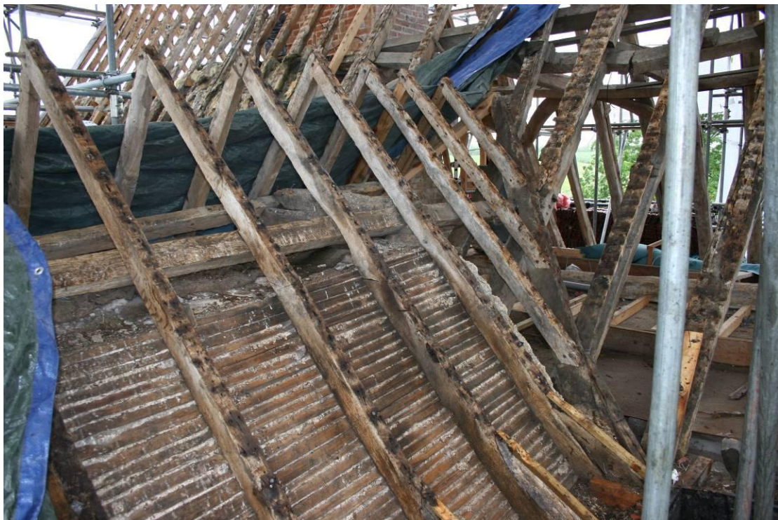
Roof structure of the porch.
