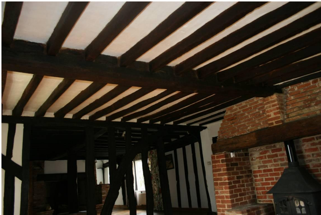
The exposed beams over the Sitting Room.
