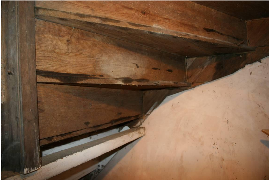
The soffit of the stairs in the Living Room.
