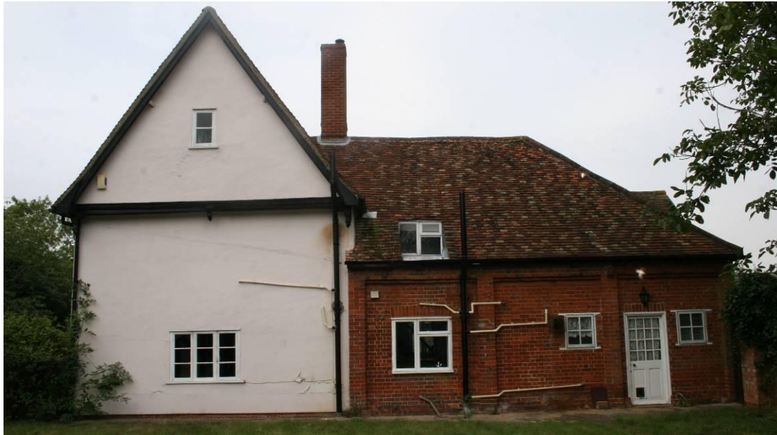
The eastern elevation of the House and Rear Range.
