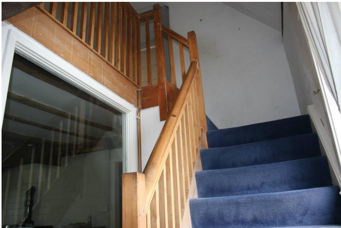
Distressed pine staircase.
