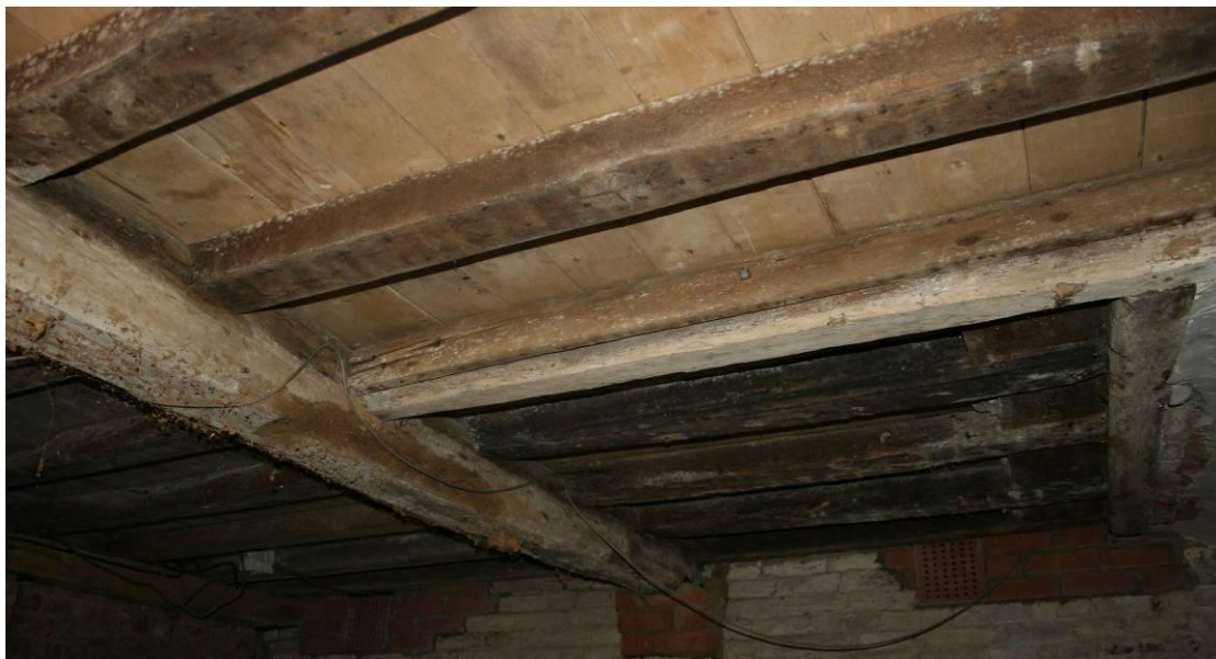
Looking N at the floor of the Lounge.
