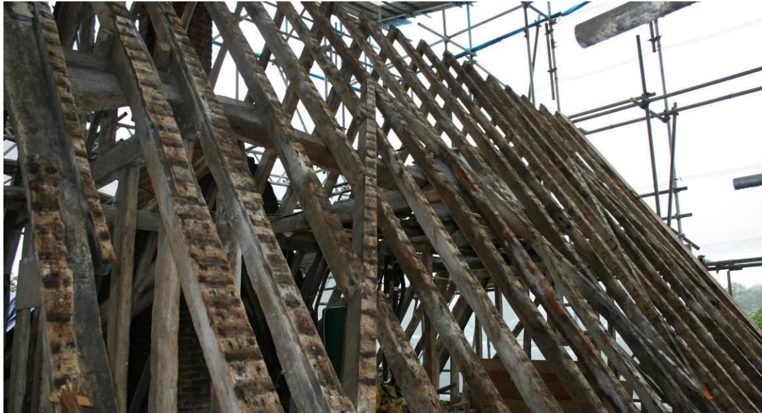
Looking NE at the roof above Bedroom 2.
