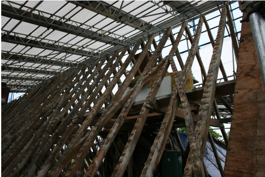
Looking NW at the roof over Bedroom 2.
