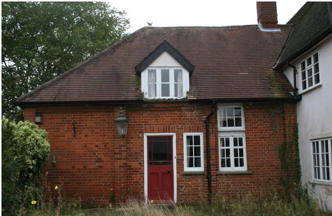
Western elevation of the Rear Range.
