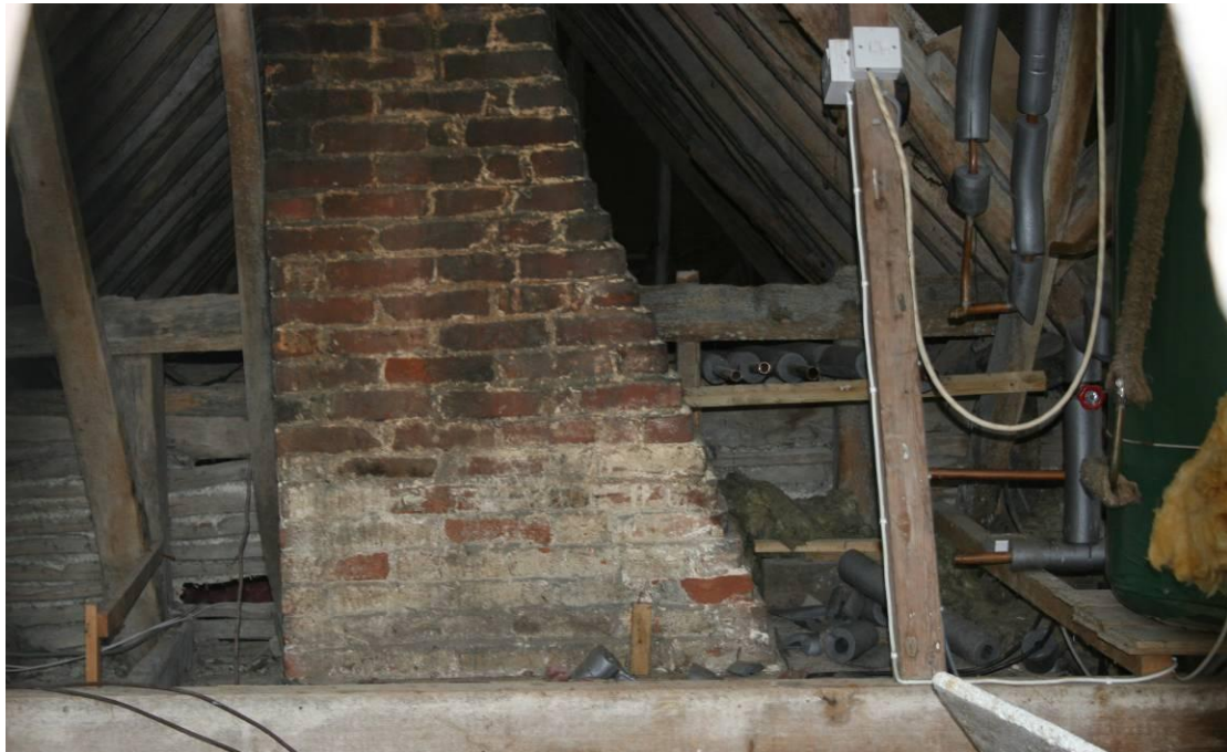
The chimney stack over Bedroom 2. Looking S.
