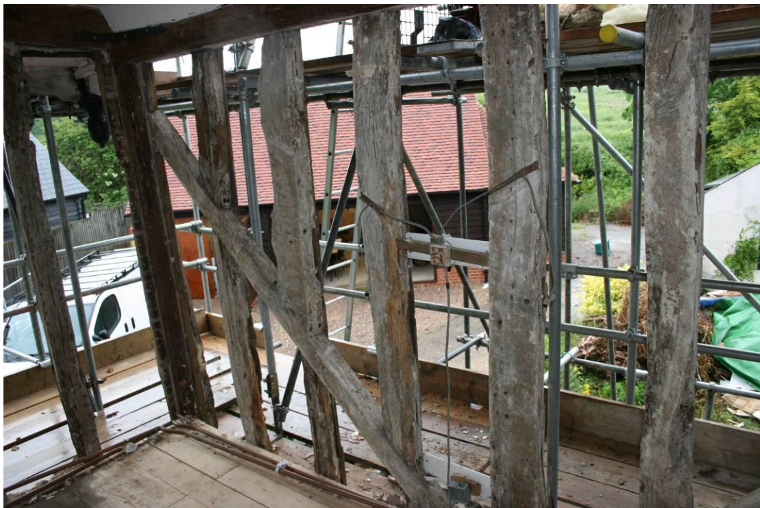
The same brace from inside the building looking NW.
