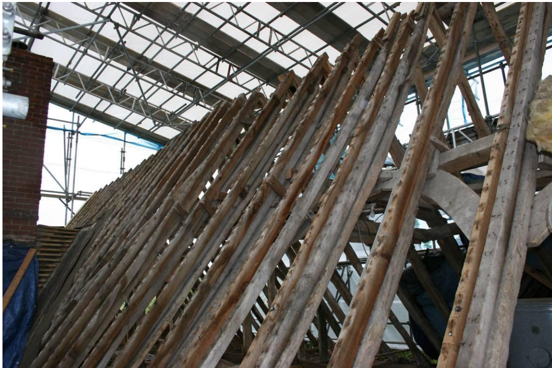
The roof over the Master Bedroom. Looking SE.
