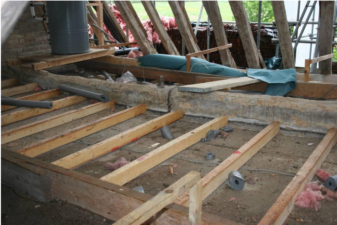
The ceiling frame above the Master Bedroom. Looking NW.
