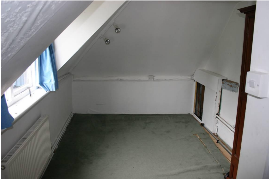
Looking E in Bathroom 3. The access leads to the bath housing and water pipes.
