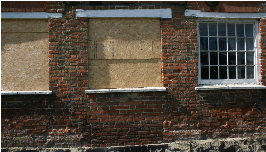
Detail of one of the blocked doorways.
