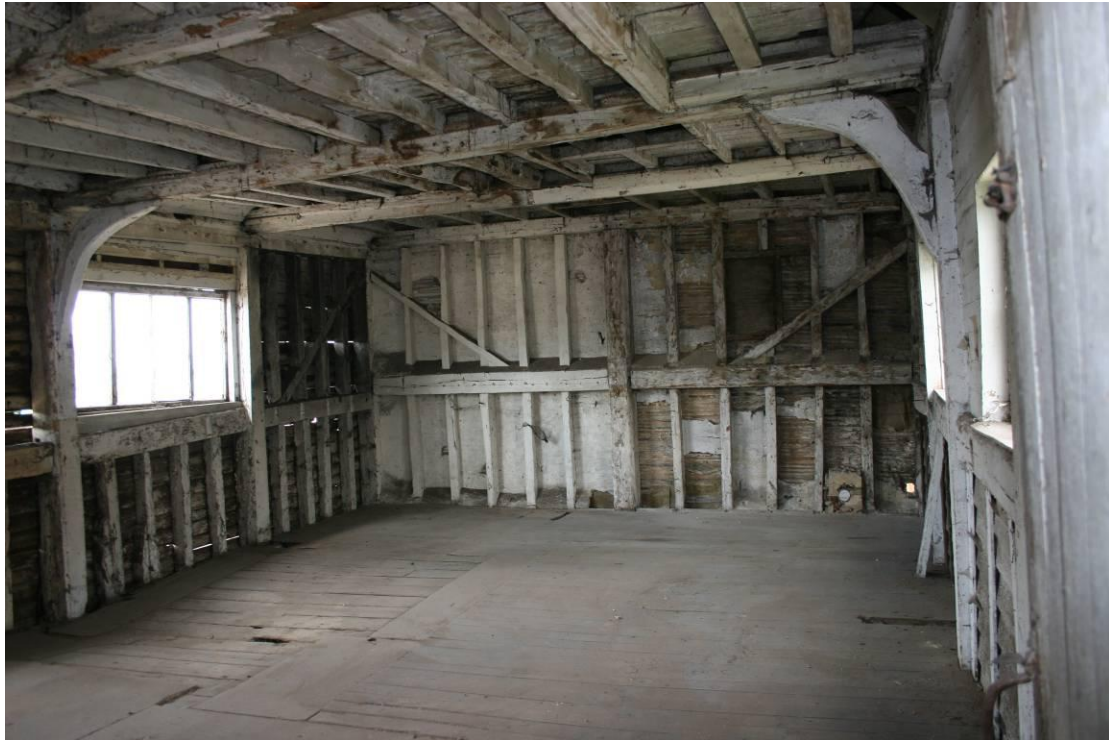
Looking N on the first floor of Building 2.
