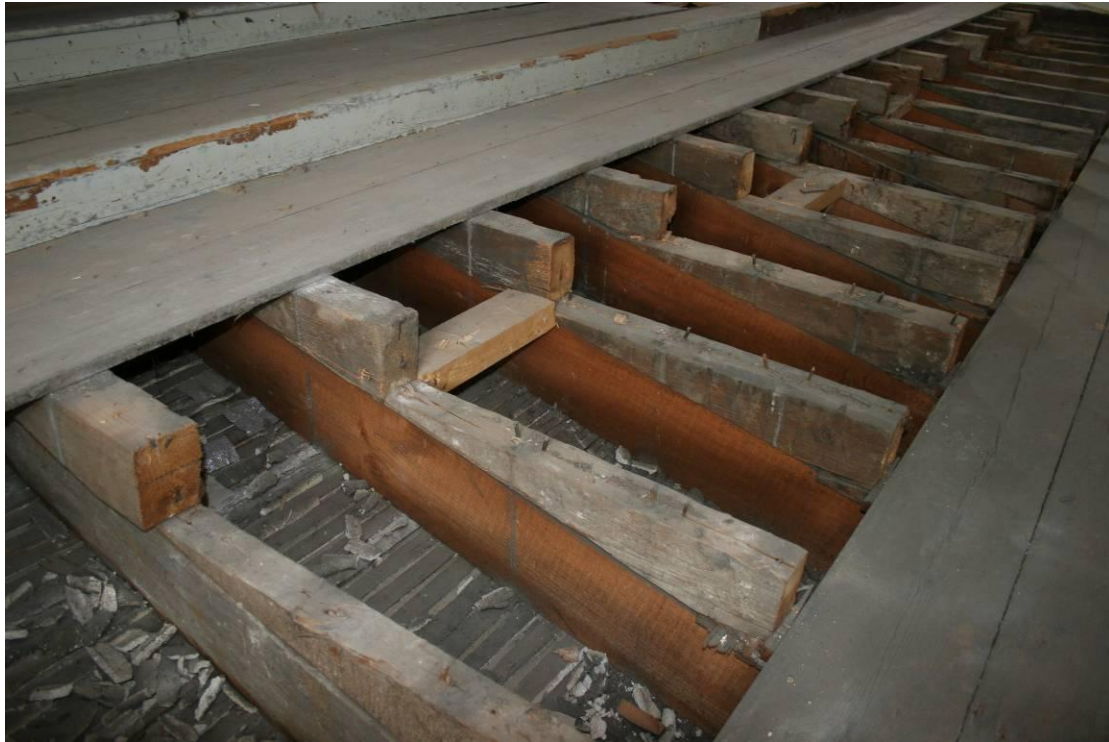
Detail of the original joinery. Looking NE.
