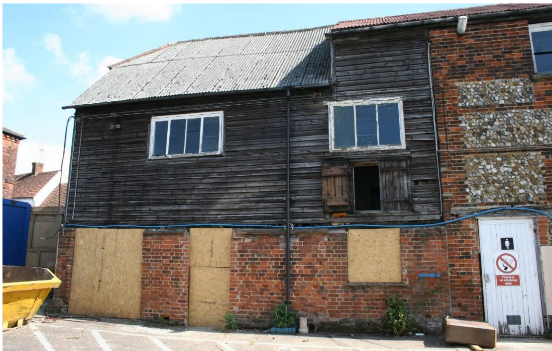
Western elevation of Building 2.
