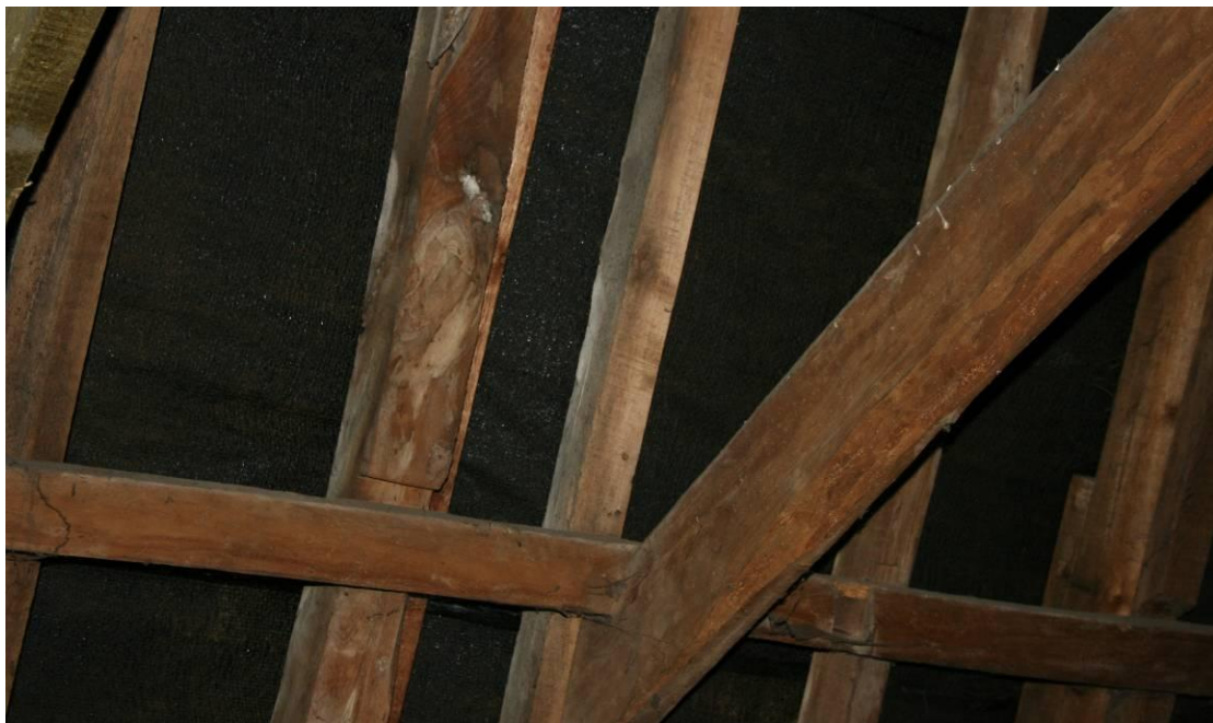
Plank collars for the repaired side purlin roof.
