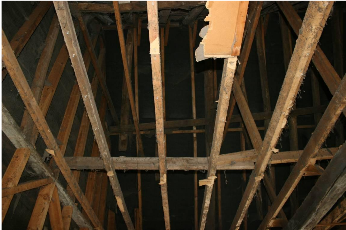
The roof over the southernmost bay. Looking W.
