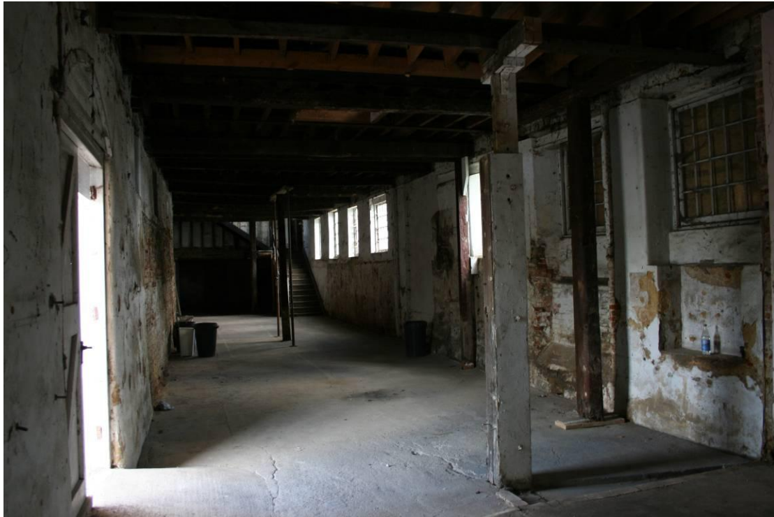
Looking N into Building 4 on the Ground Floor.
