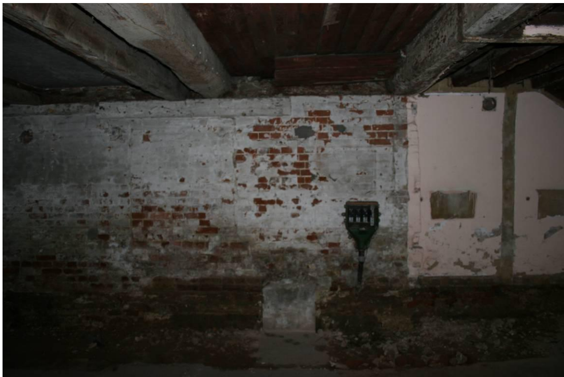
Looking E on the ground floor of Building 2.
