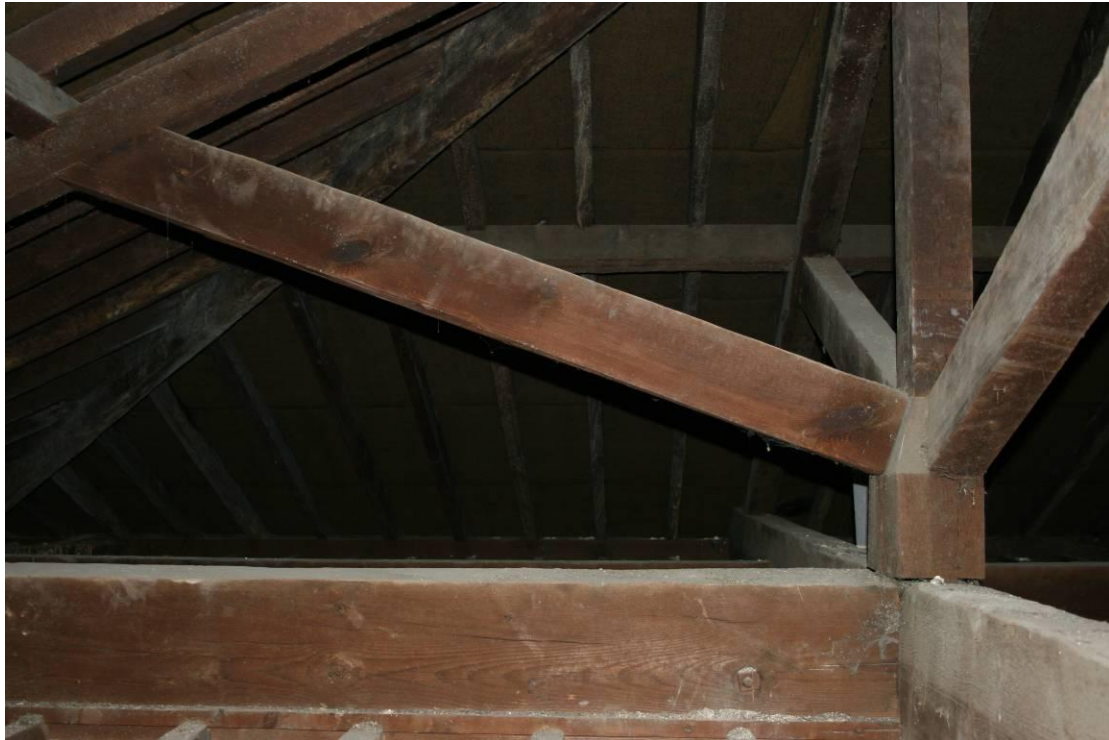
One of the two king post trusses. Looking W.
