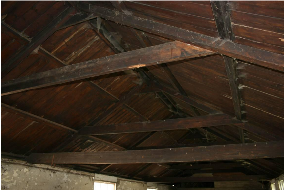
The roof above the maltings floor in Building 3.
