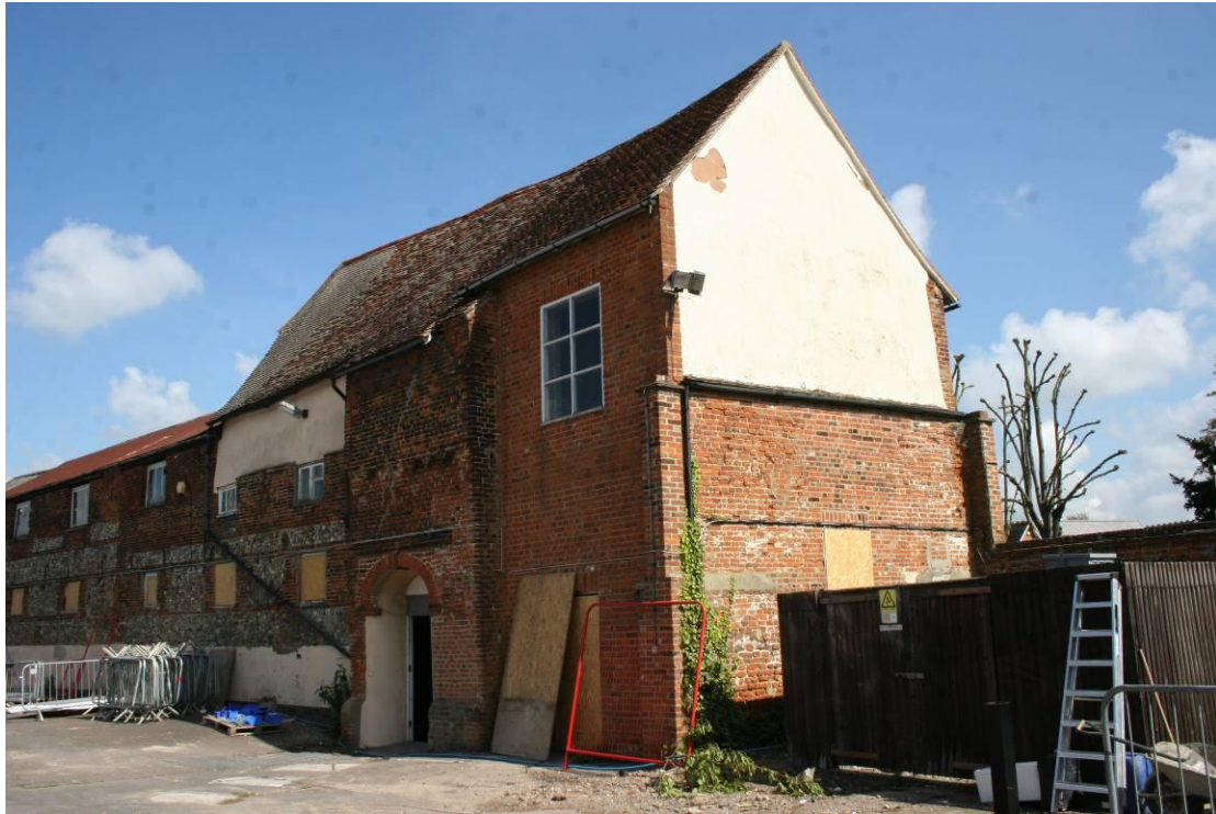
The southern elevation has been replaced in the MC20th.
