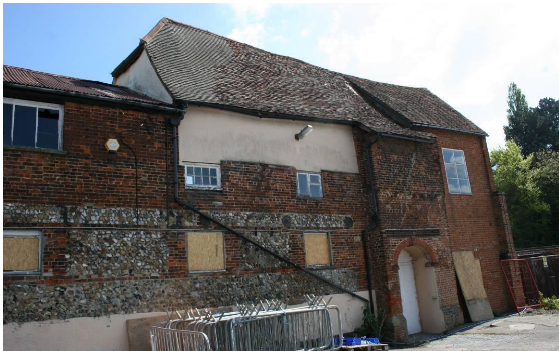
The western elevation showing the flintwork panels extending across Buildings 3 and 4.
