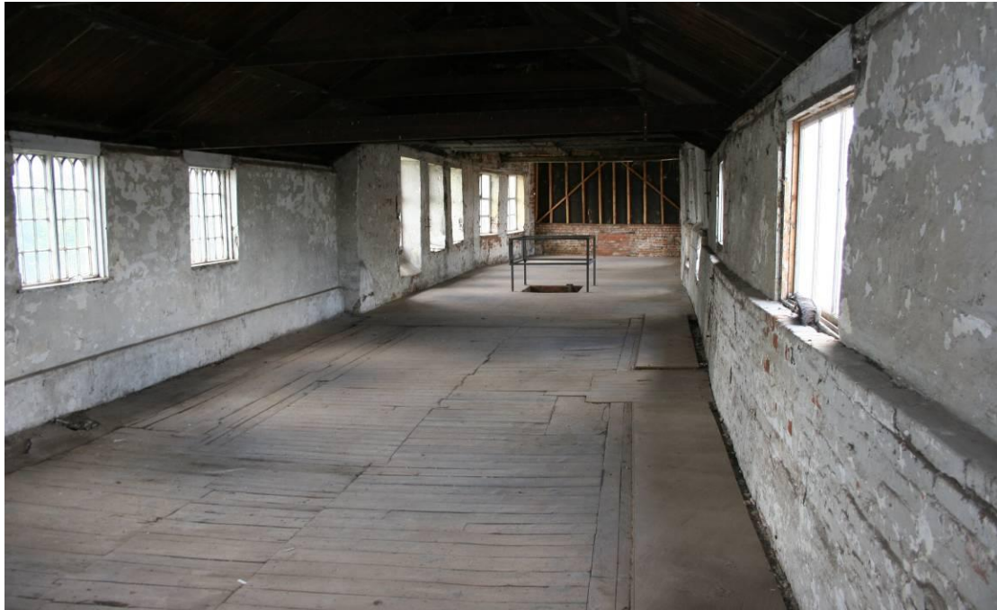
Looking S on the malting floor in Building 3.
