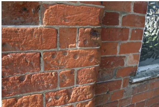
Coin bored hemispheres in the bricks.
