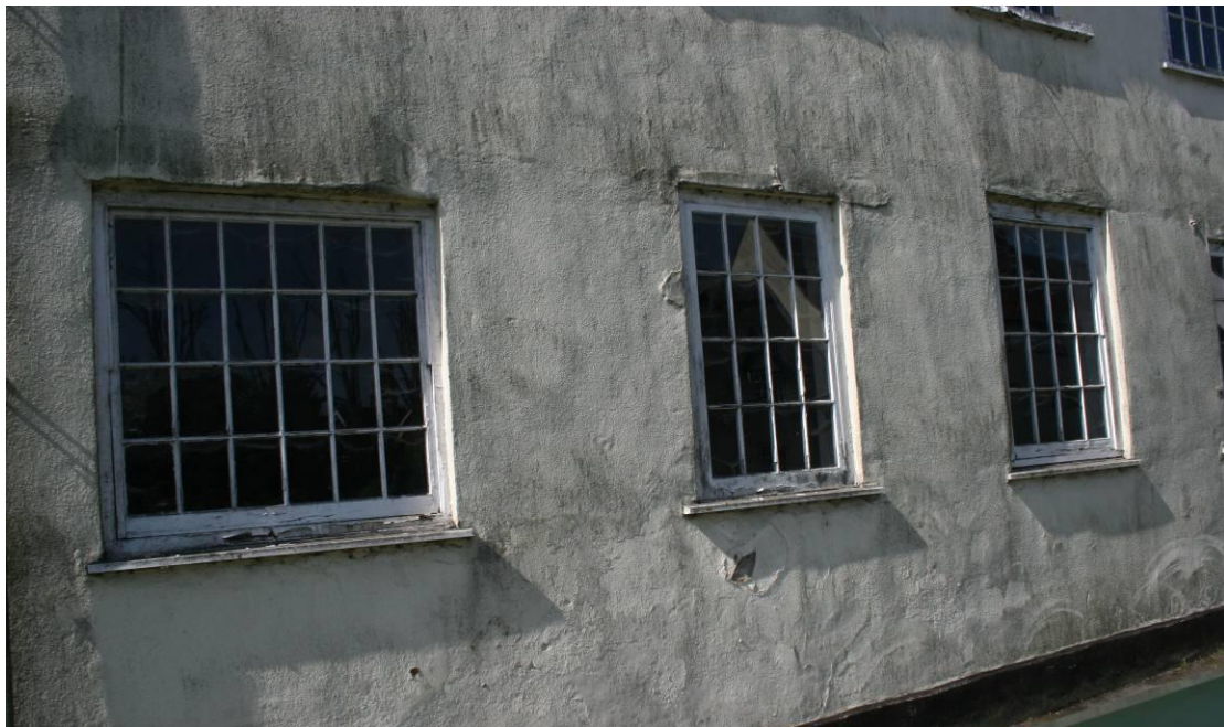
Detail of the windows on Building 3.
