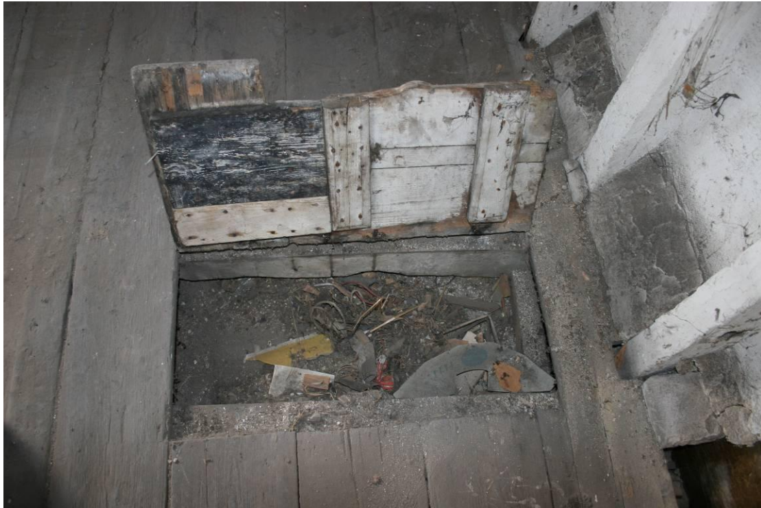
Trap door in the floor.
