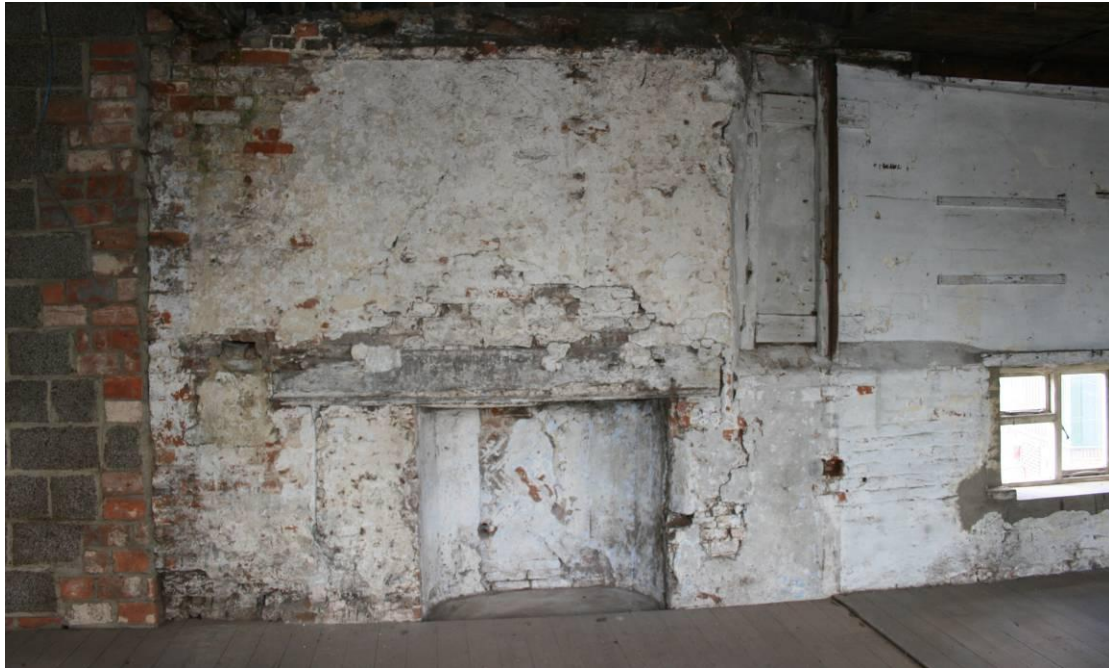
The fireplace in the western wall.
