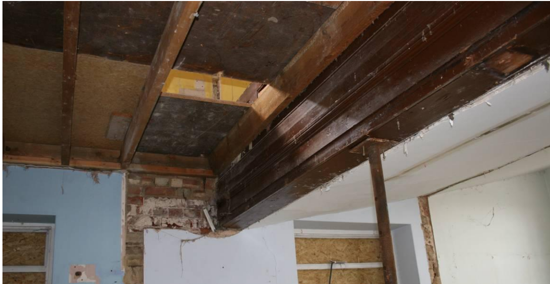
Original support beam for the balcony. Looking W.
