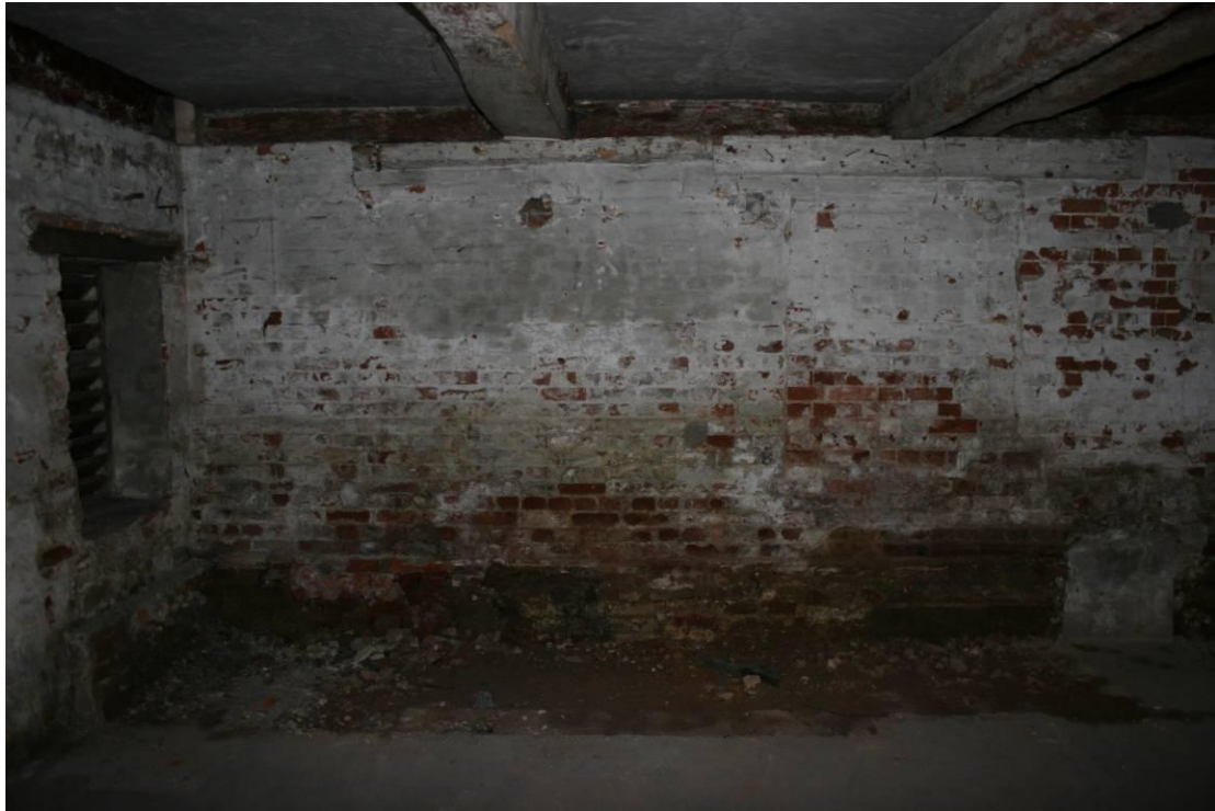
Looking S on the ground floor of Building 2.
