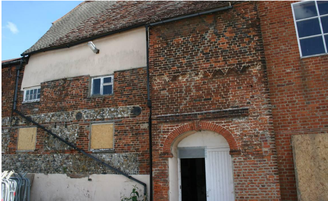
Tudor style brickwork with a Georgian segmental archway.
