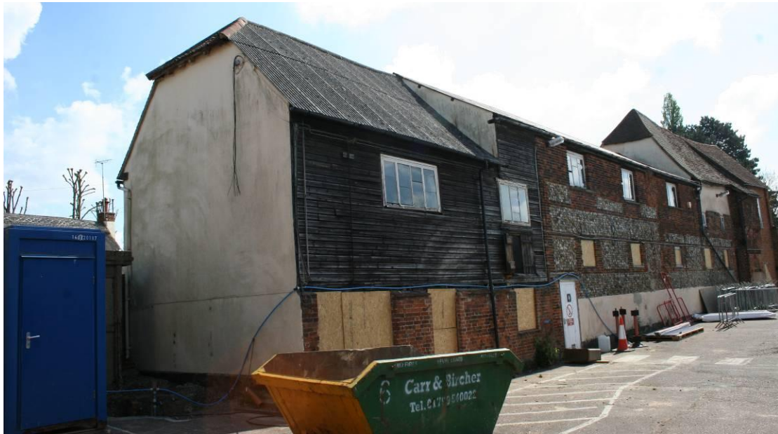
Northern elevation of Building 2.
