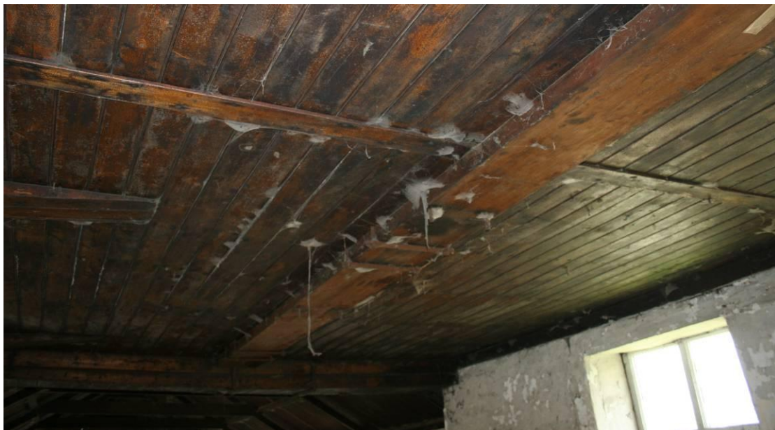
The suspended ceiling that ran right through the building. Looking N.
