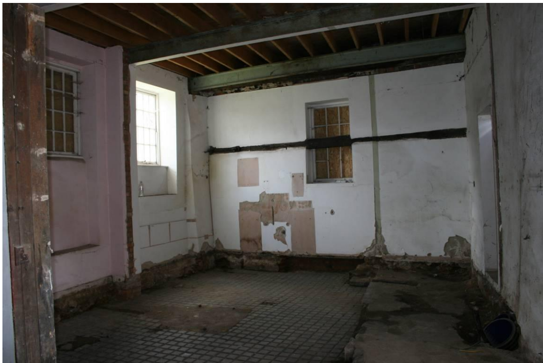
Looking S into Building 4 on the Ground Floor.
