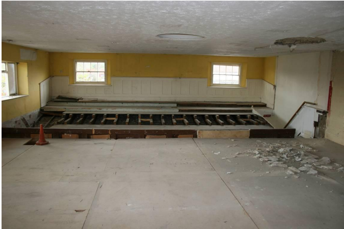
Looking N at the tiered seating from the LC20th inserted flooring.
