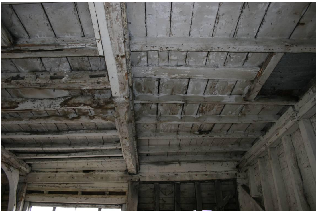
Trap door or stair trimmer in the ceiling.
