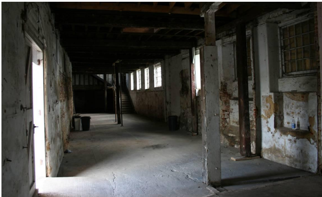
Looking N in Building 3 from Building 4 on the Ground Floor.
