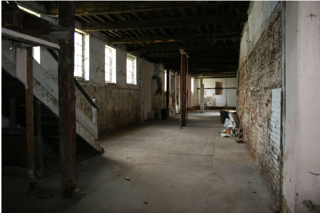
Looking S in Building 3 on the Ground Floor.
