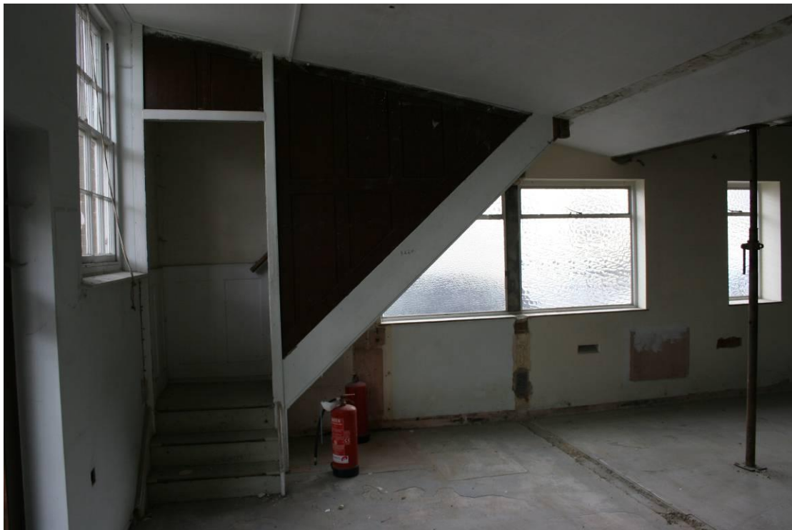
Panelled staircase up to the balcony in the NE corner.
