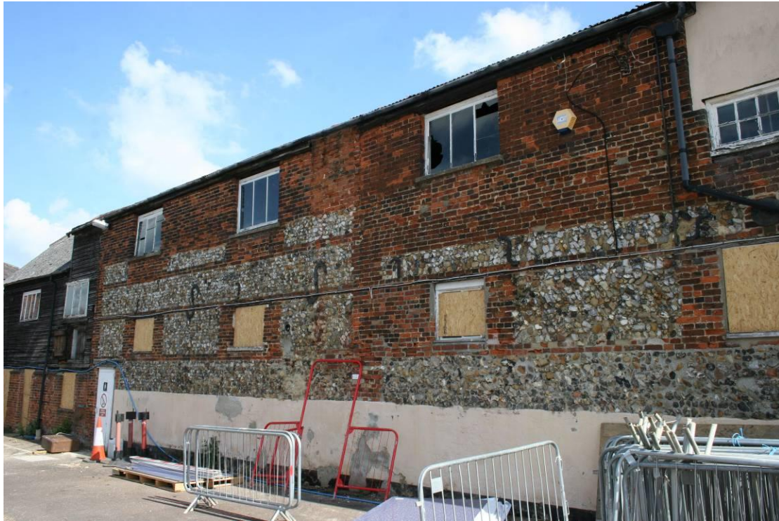
The western elevation of Building 3.
