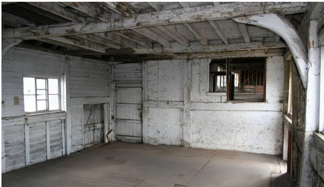
Looking S on the first floor of Building 2.
