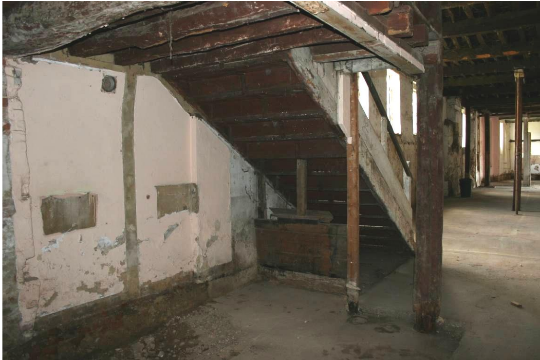
Detail of the staircase. Looking SE.
