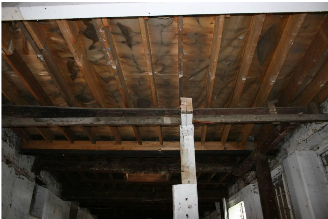
LC20th flooring supported on RSJ's. Looking N.
