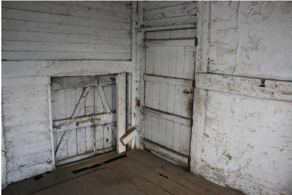
Detail of the E20th access doors. Looking SE.
