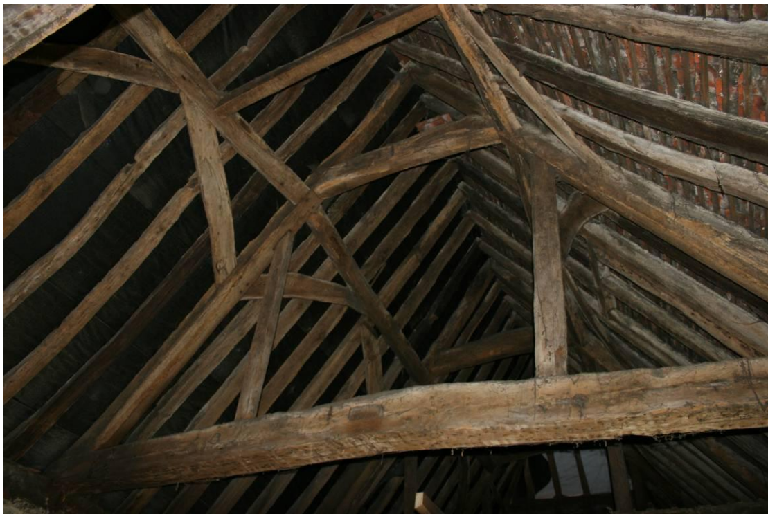
Queen post truss looking NW.
