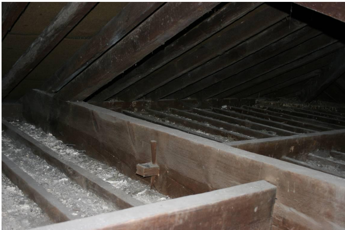
Detail of the ceiling structure looking SW. Note the keyed tenon.
