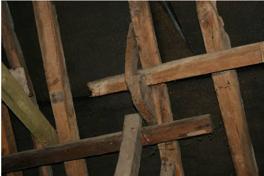
C19th and C20th repairs to the roof of Building 2.
