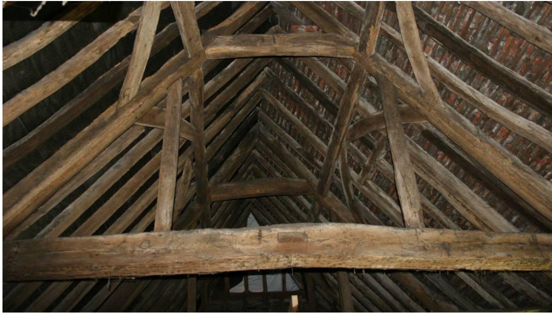
Queen post truss over Building 4. Looking SW.
