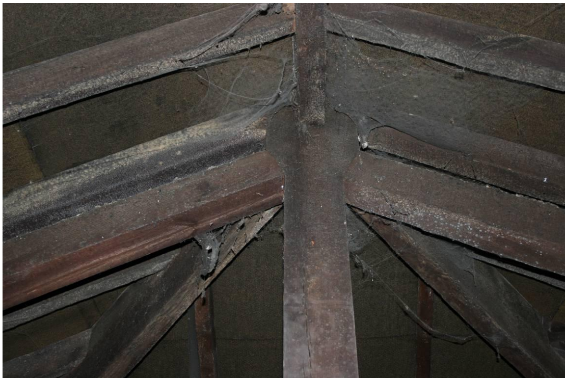
Looking up at the roof structure.
