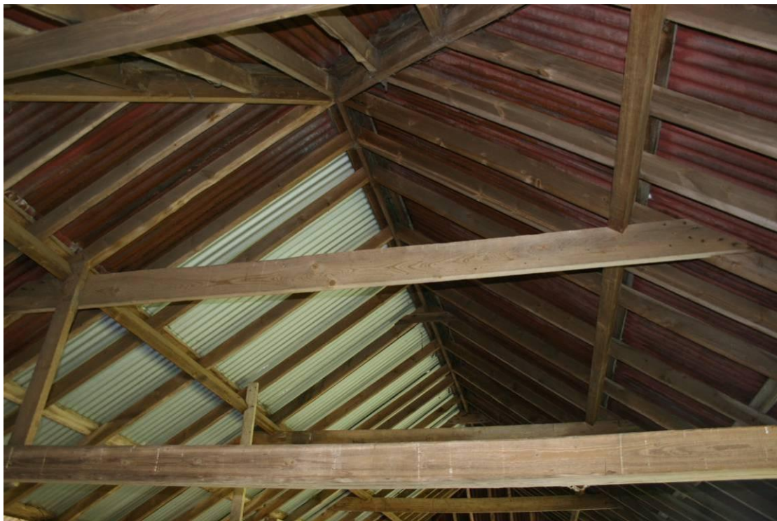
Roof structure of the Tractor Shed looking S.
