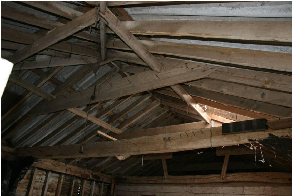
Detail of the roof structure.
