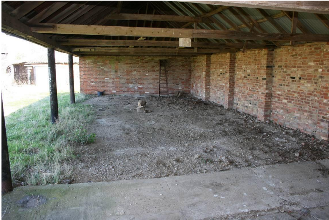
Interior of the Tractor Shed looking N.
