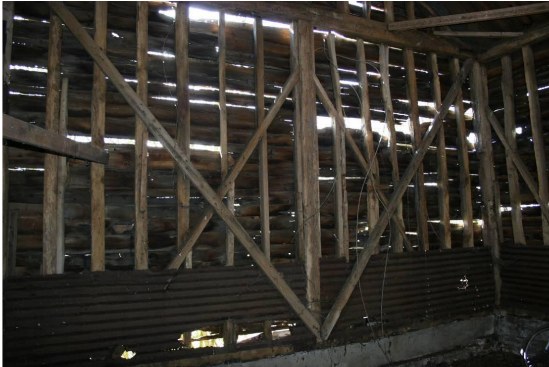
Detail of the north wall.
