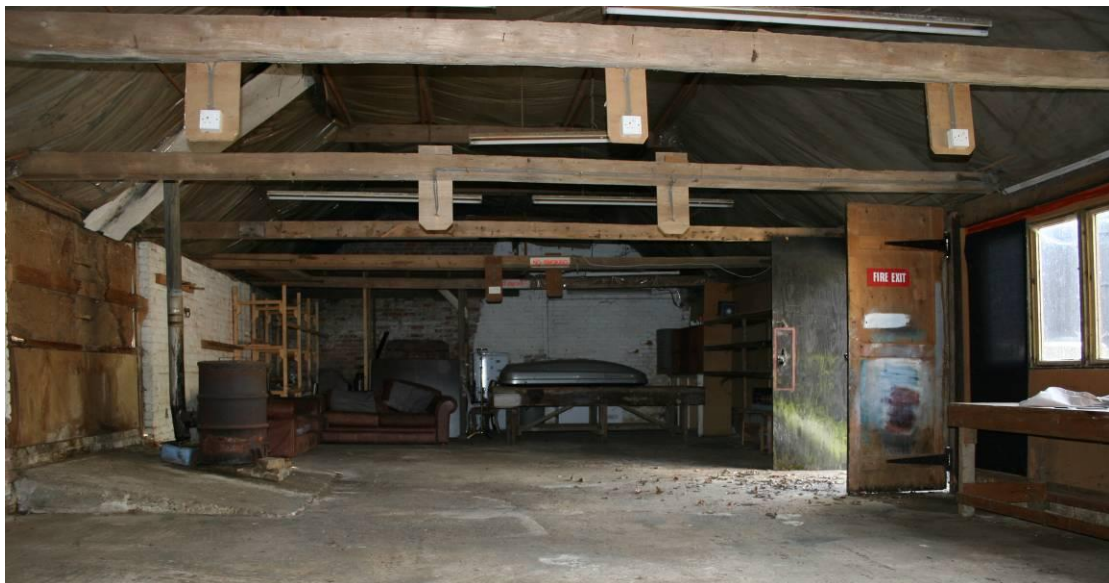
Looking W inside the Workshop.
