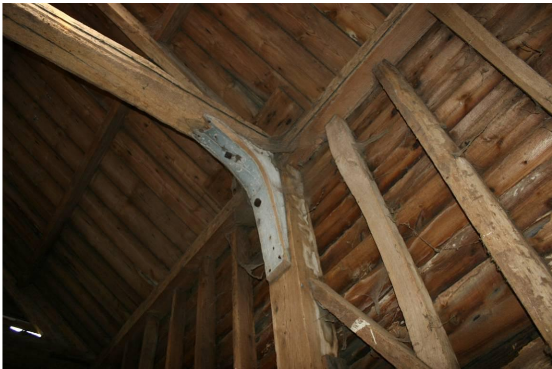
Detail of the hanging knee and tie-beam.
