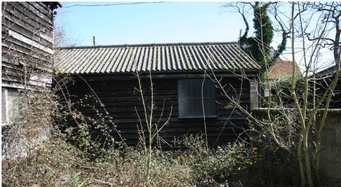
Western elevation of the Garage.
