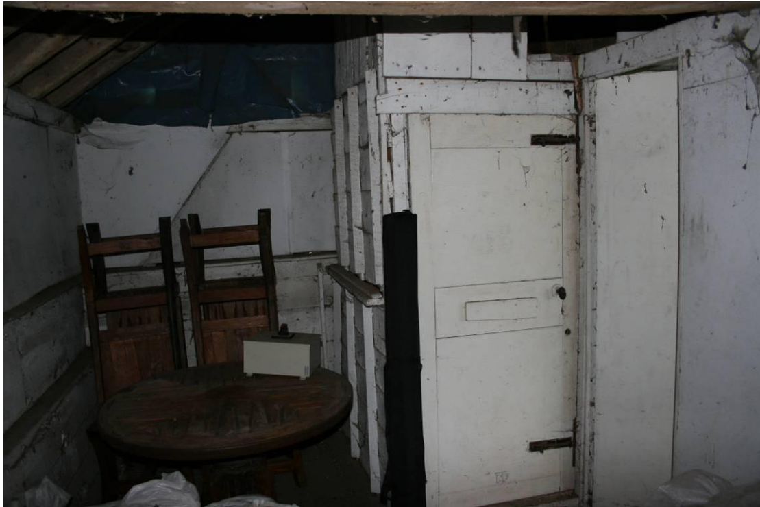
Storage area in the eastern end of the Granary.
