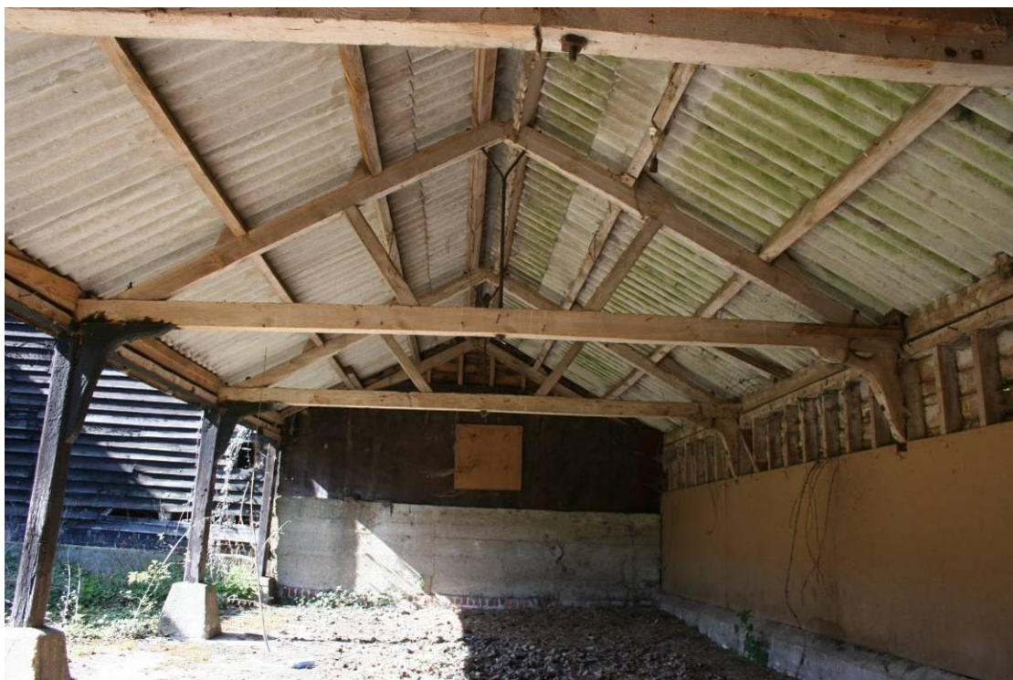
Looking E inside the Shelter.
