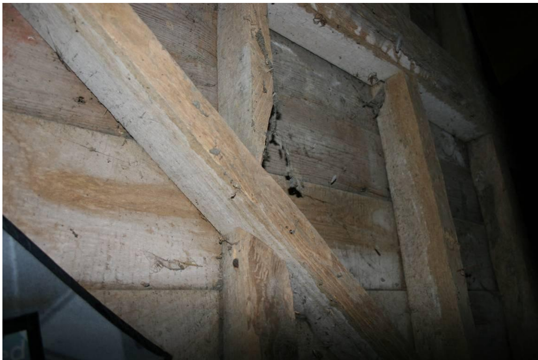
Nailed interrupted studwork in the partition wall.
