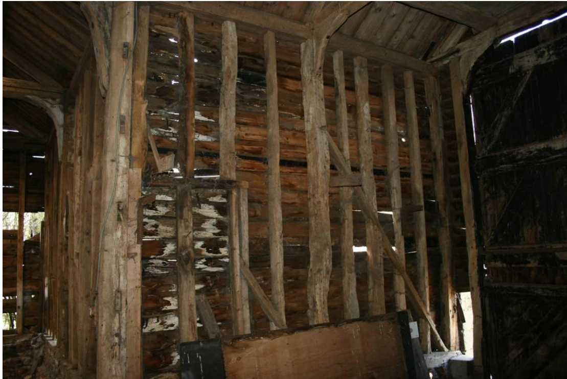
Originally the porch had doors on both sides.
