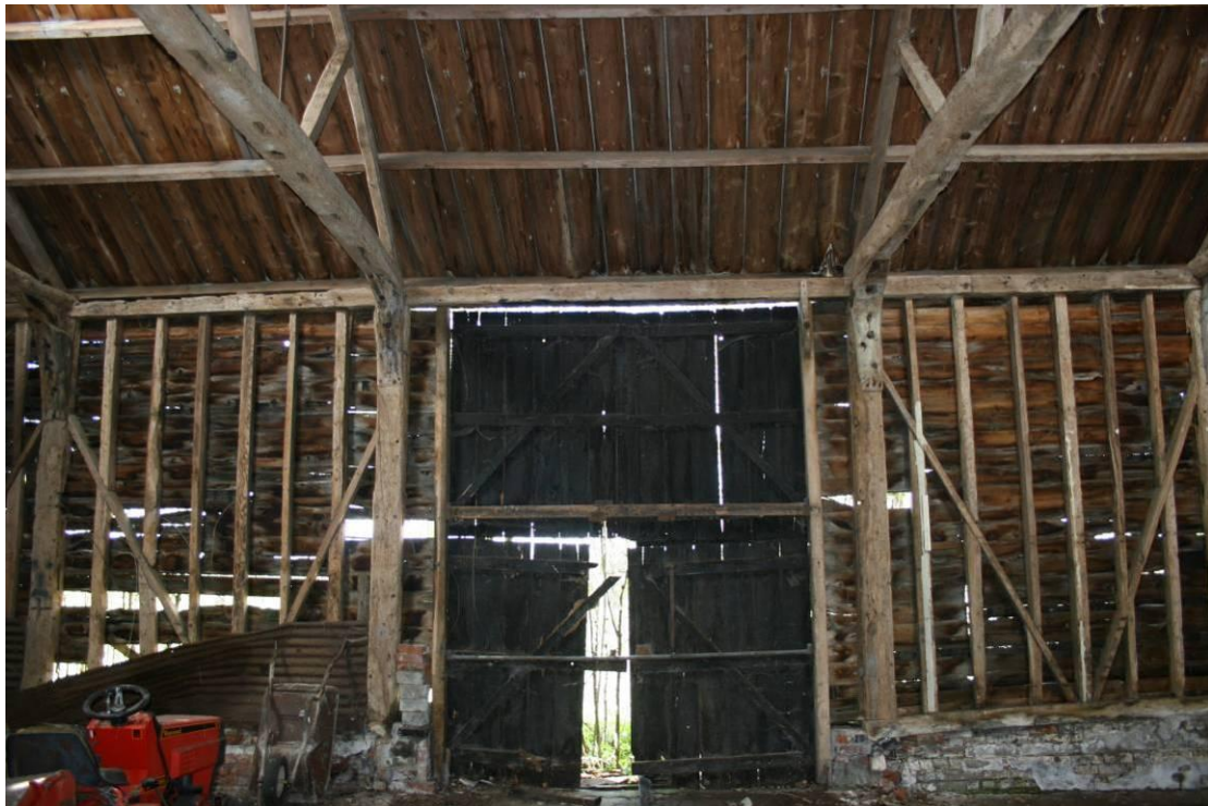
Detail of the eastern doorway.
