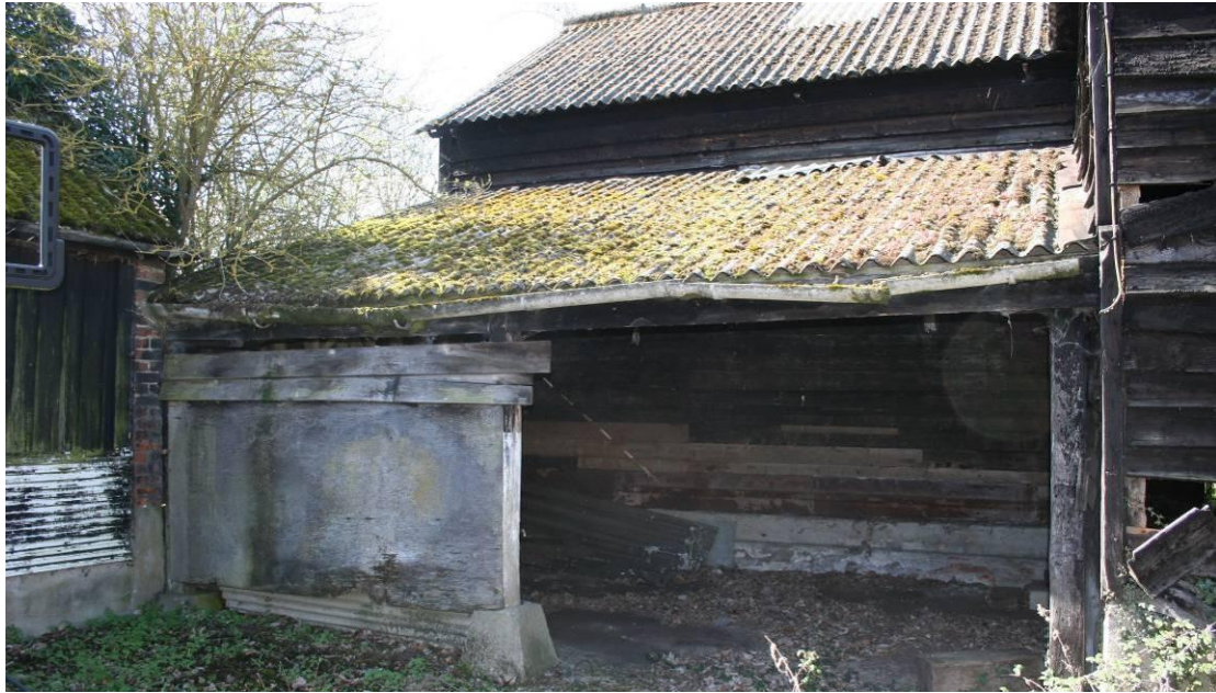
Barn Shelter looking NE.
