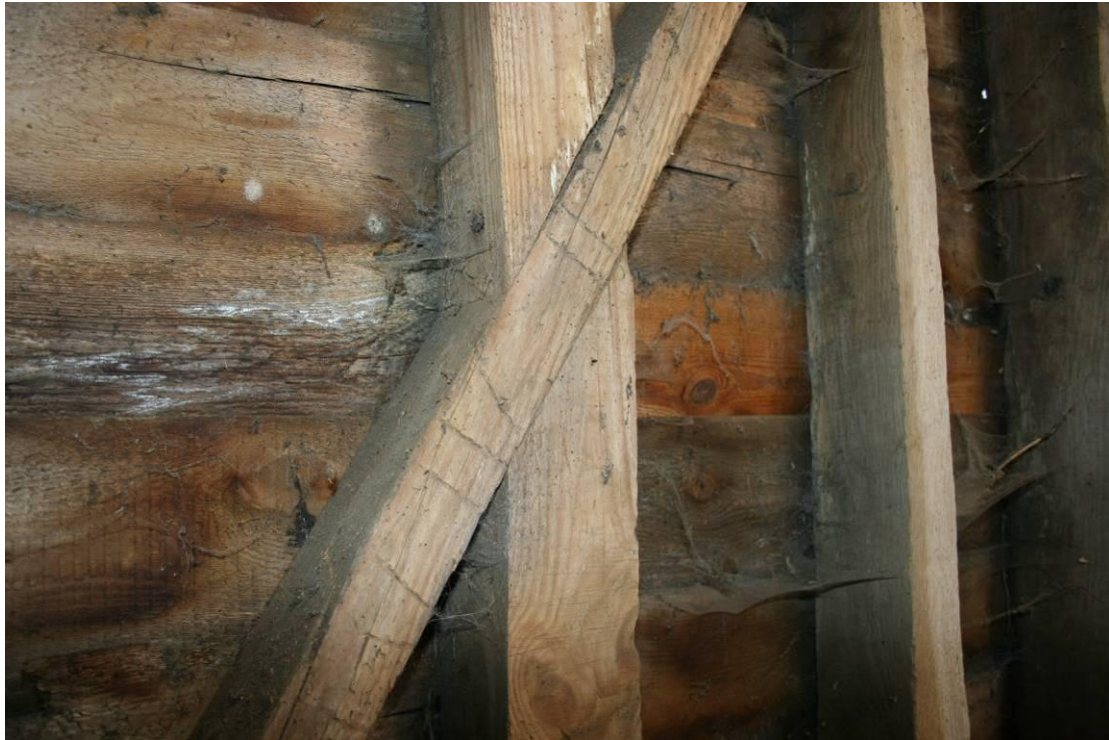
Merchant's timber marks on the primary brace.
