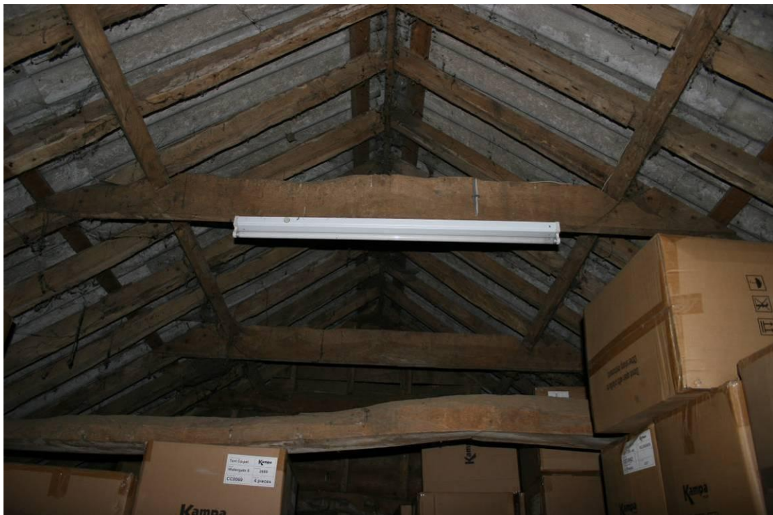
Looking E at the roof structure.
