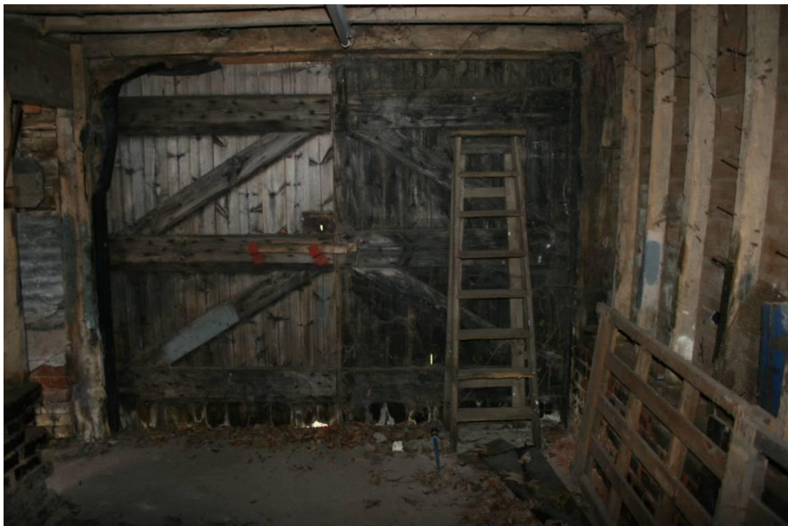
Looking E in the central bay.
