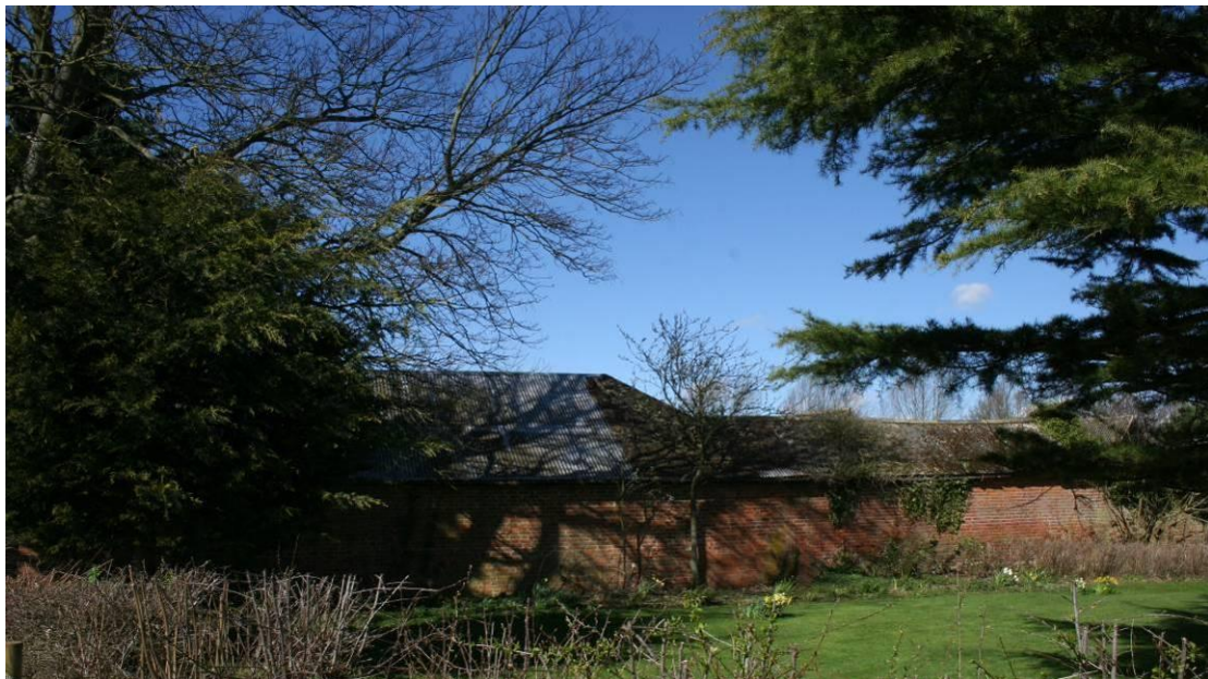
The eastern elevation of the Carpenter's Shop and the Tractor Shed.
