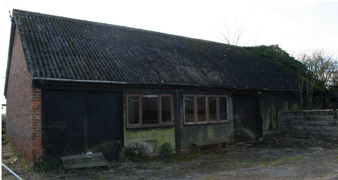
Northern elevation of the Workshop.
