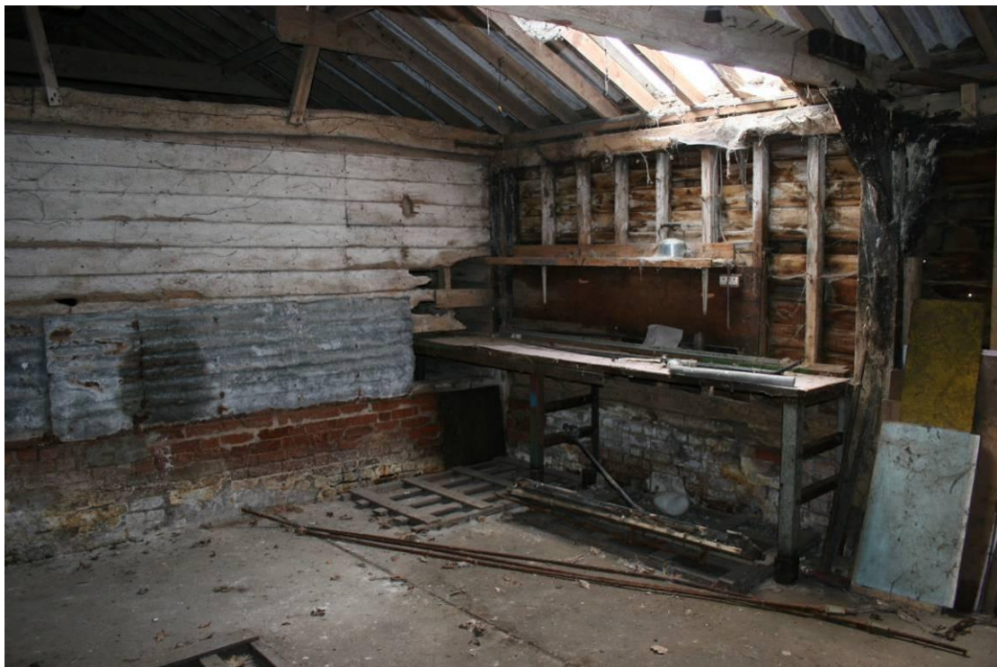
Looking SW in the northern room of the Stables.
