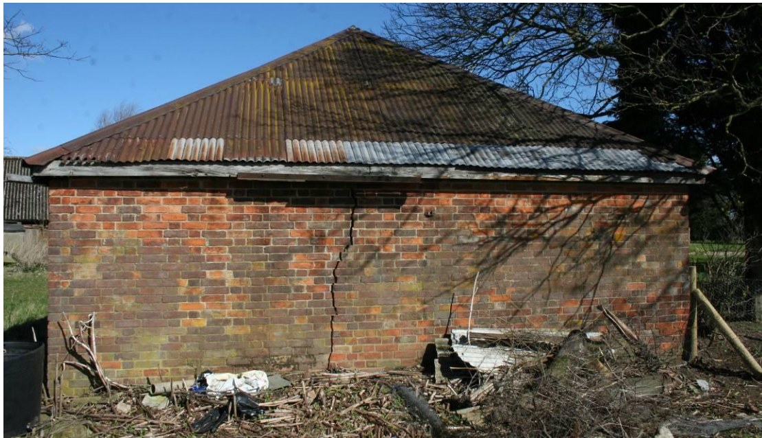
The southern wall of the Tractor Shed.
