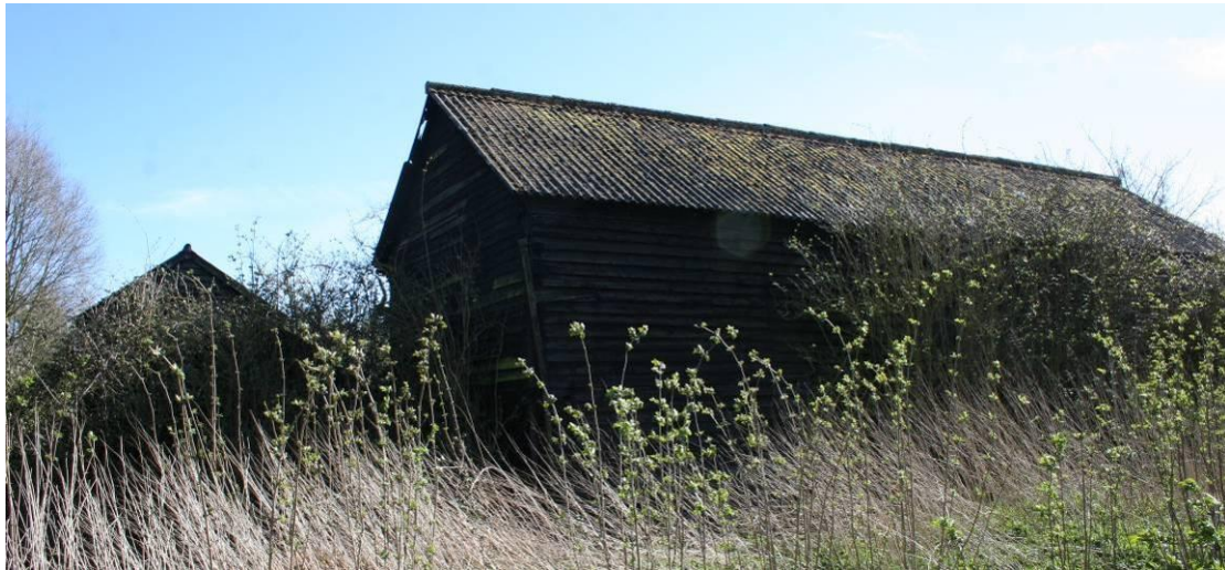
The northern and western elevation of the Barn.
