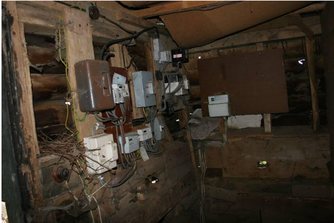
Power supply and meters are fixed to the original frame.
