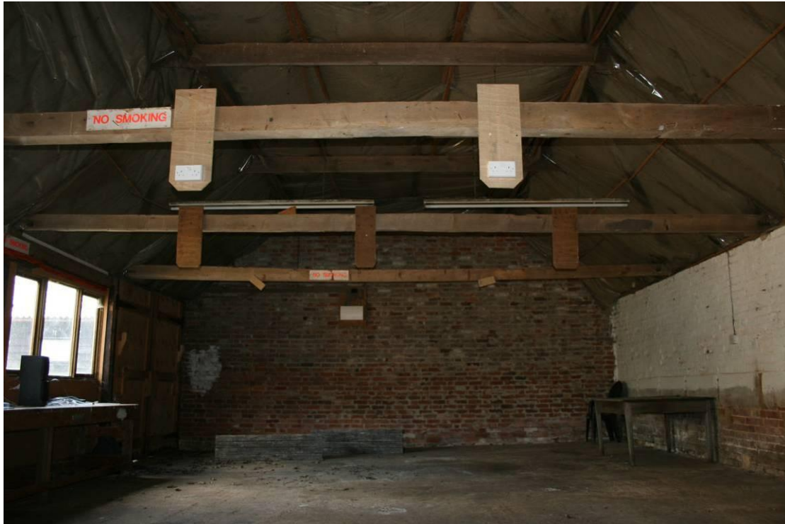
Looking E inside the Workshop.
