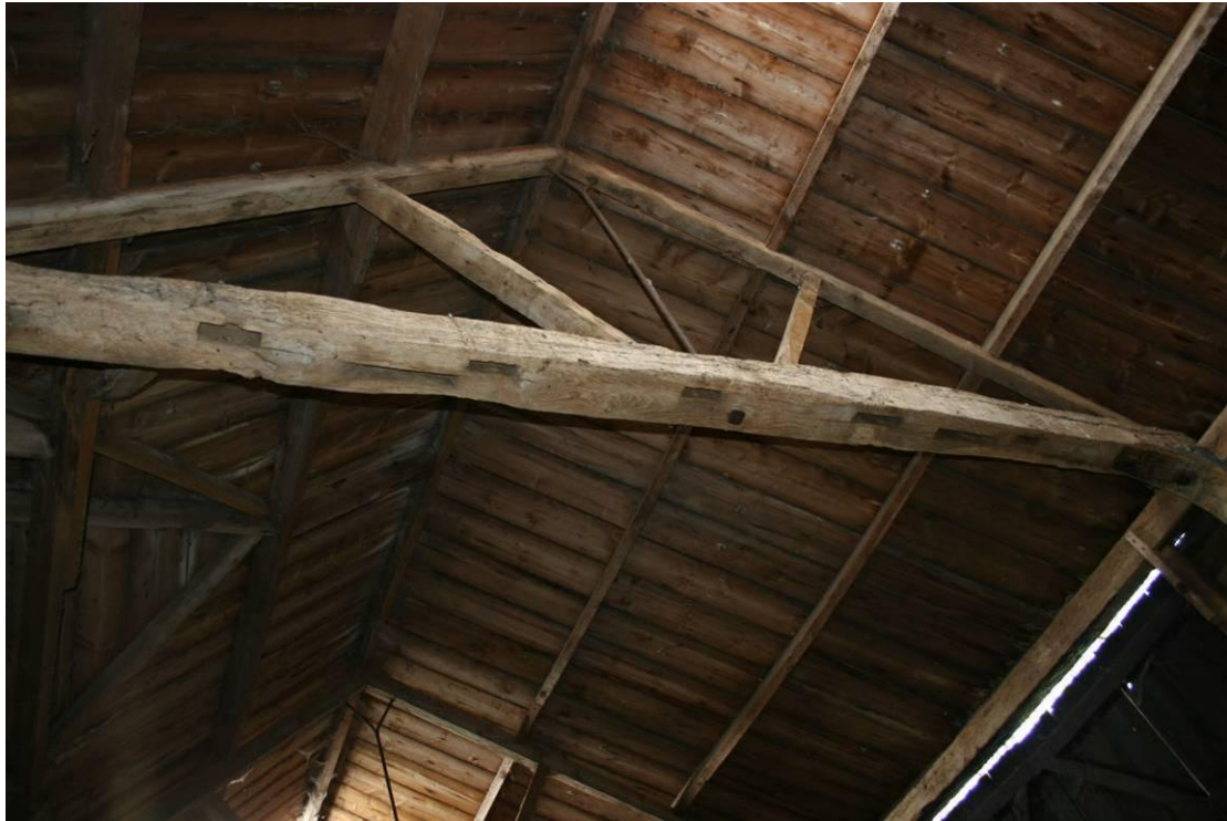
Detail of a king bolt truss. Note the reused timbers.
