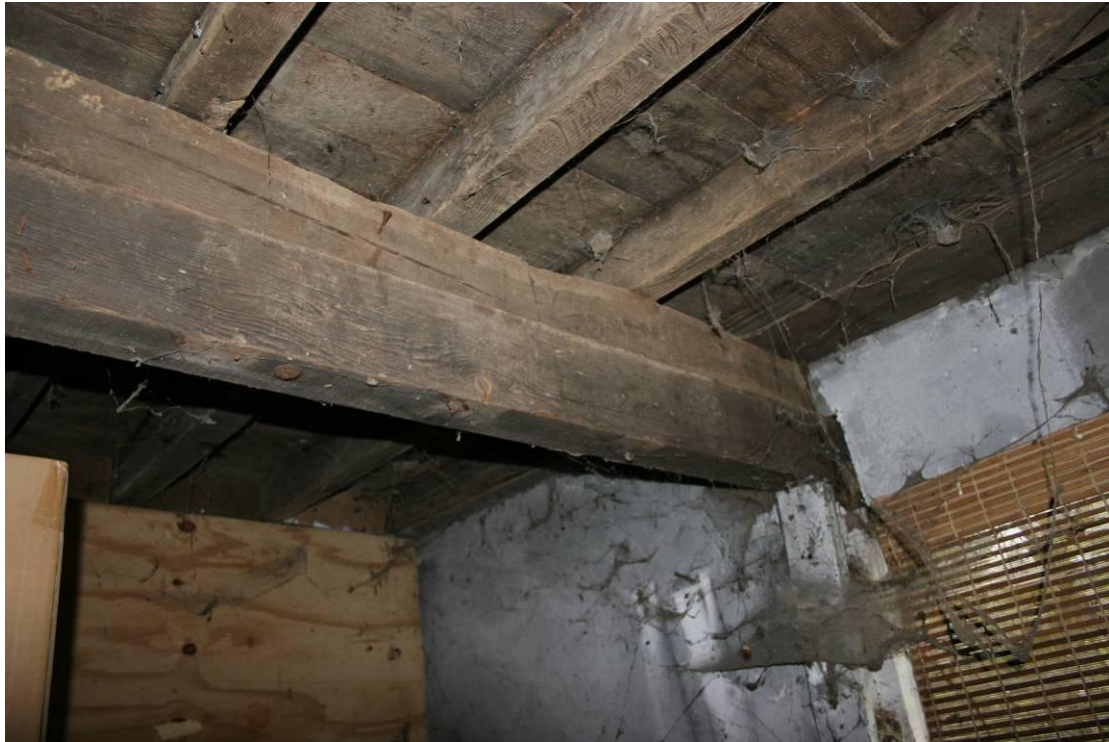
Additional support for the main joists.
