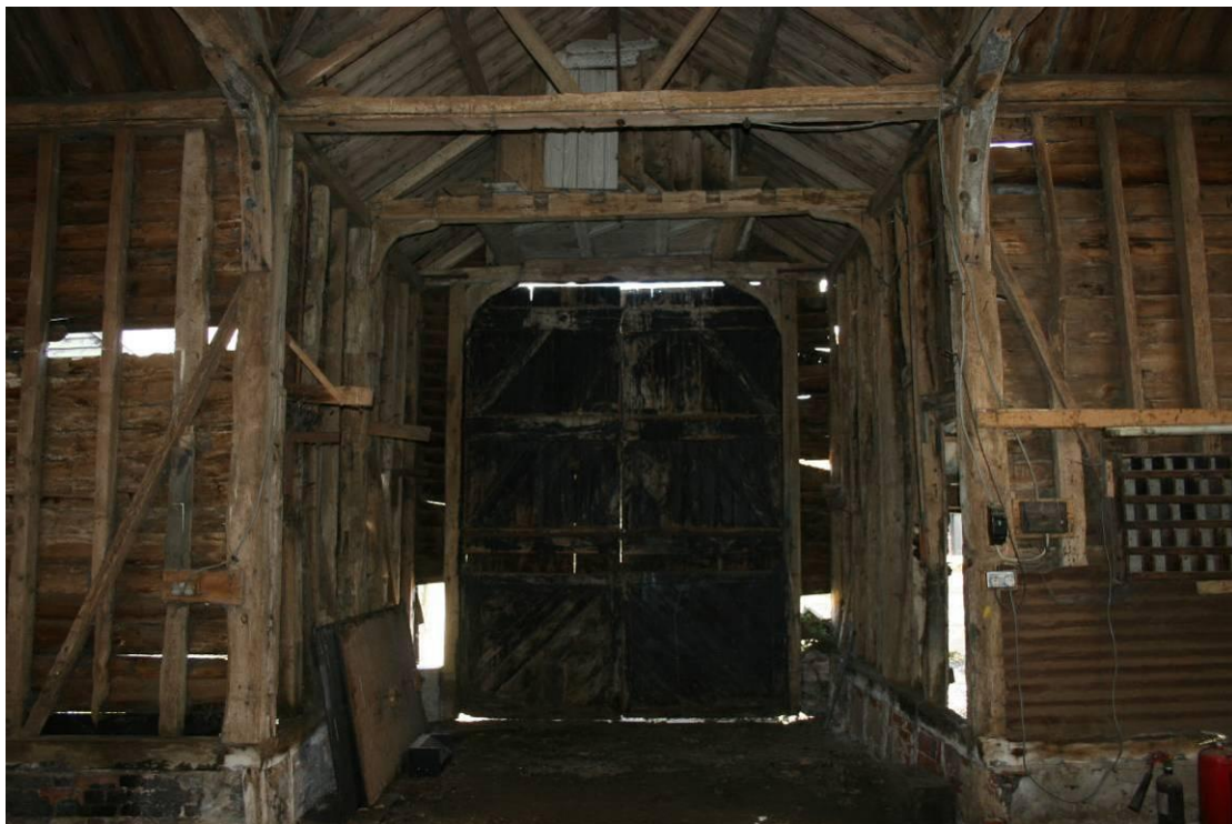
Looking E into the porch.
