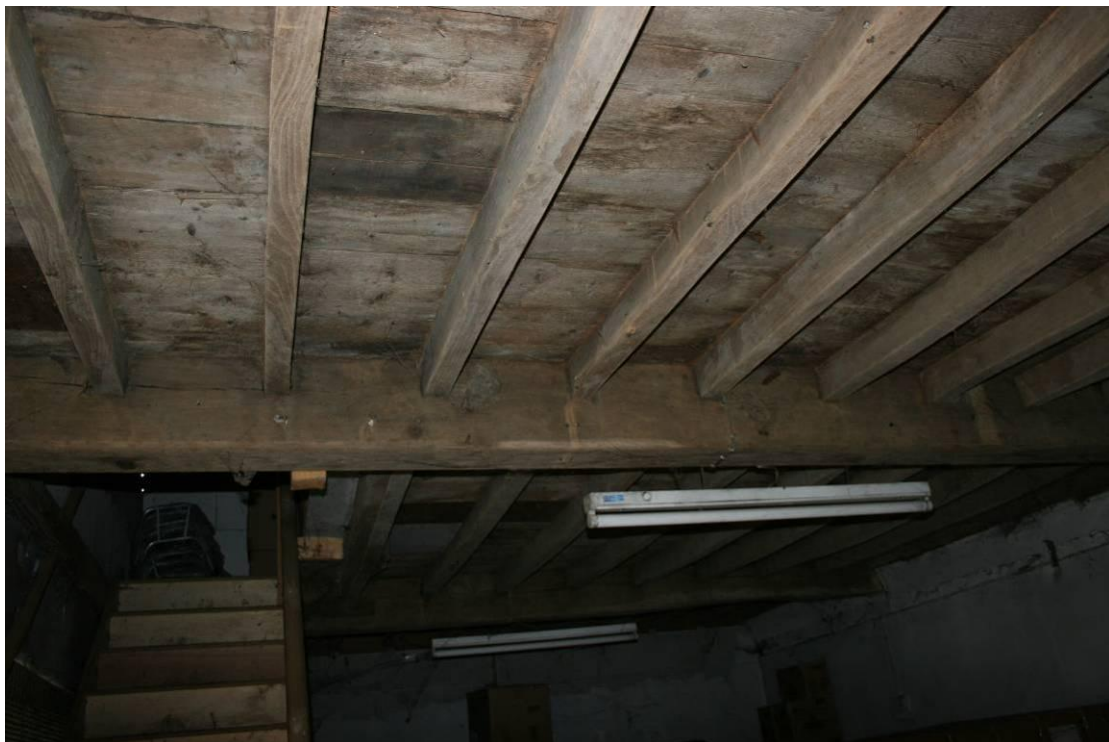
The framing of the Granary floor. Looking W.
