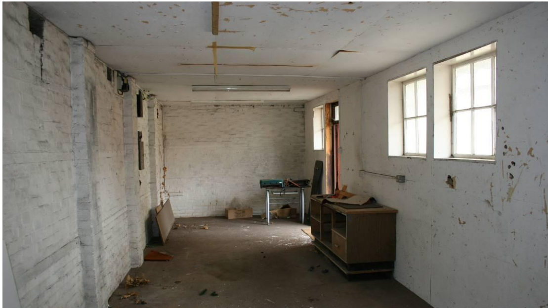
Looking S inside the Workshop on the ground floor.
