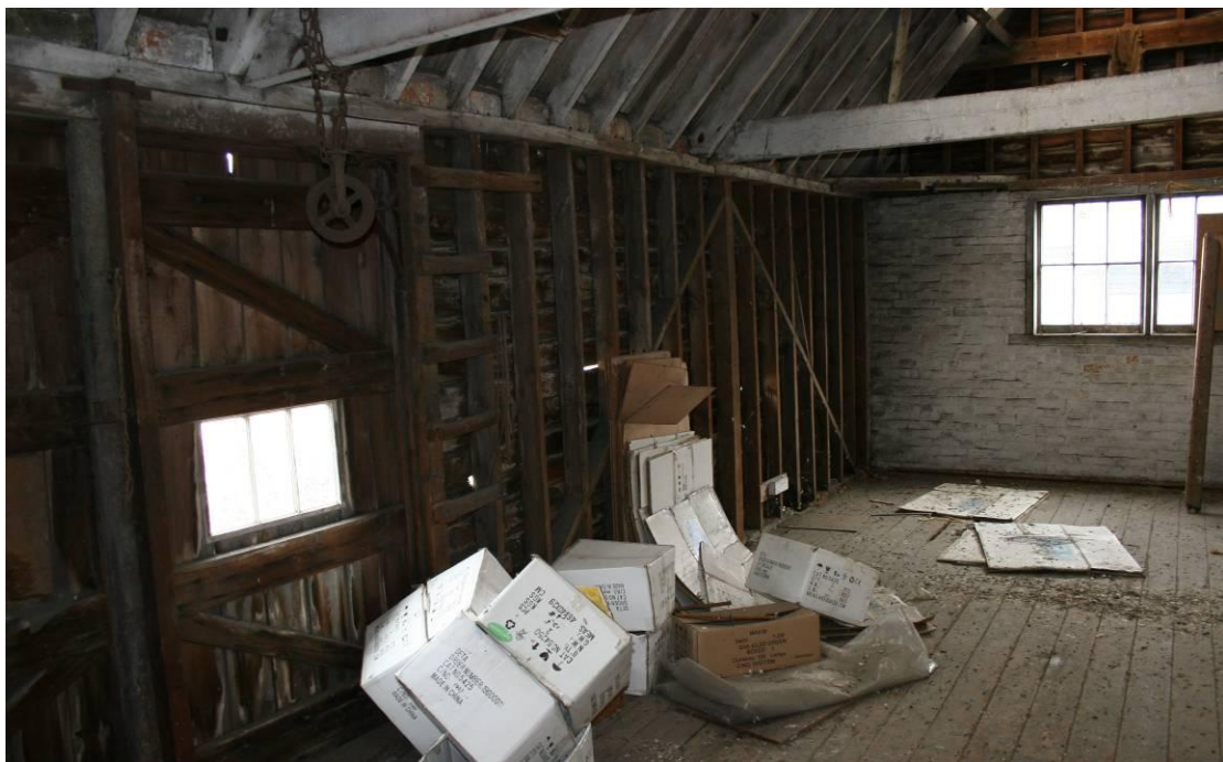
Access doors, pulley and ladder on the western wall.
