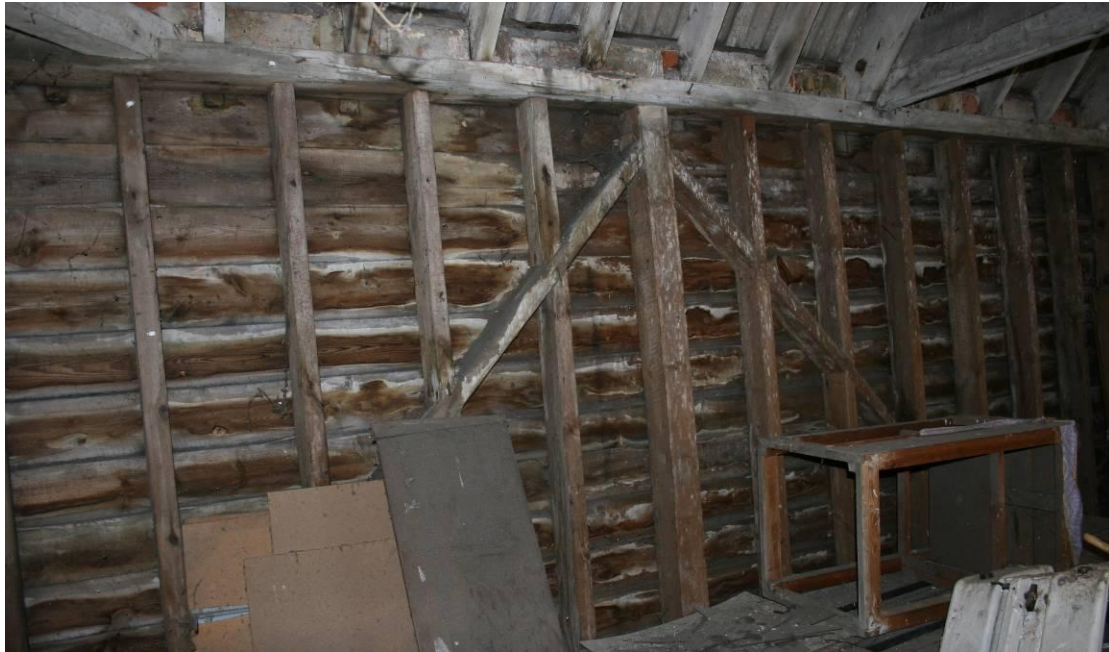
Primary braced 2x4in studwork.
