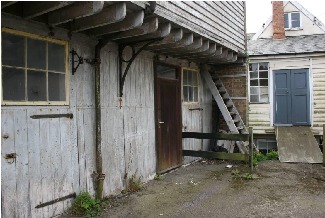
Looking SE along the jetty.
