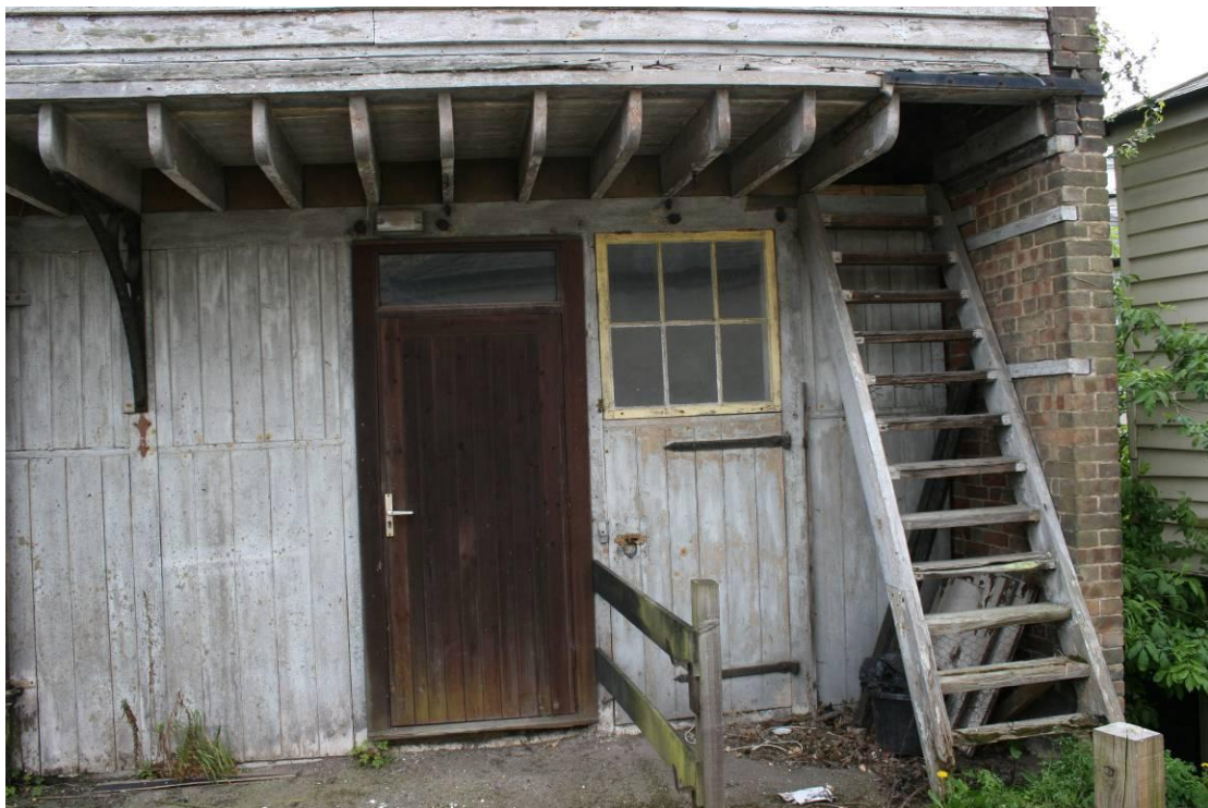
C20th additional door in the southern end.
