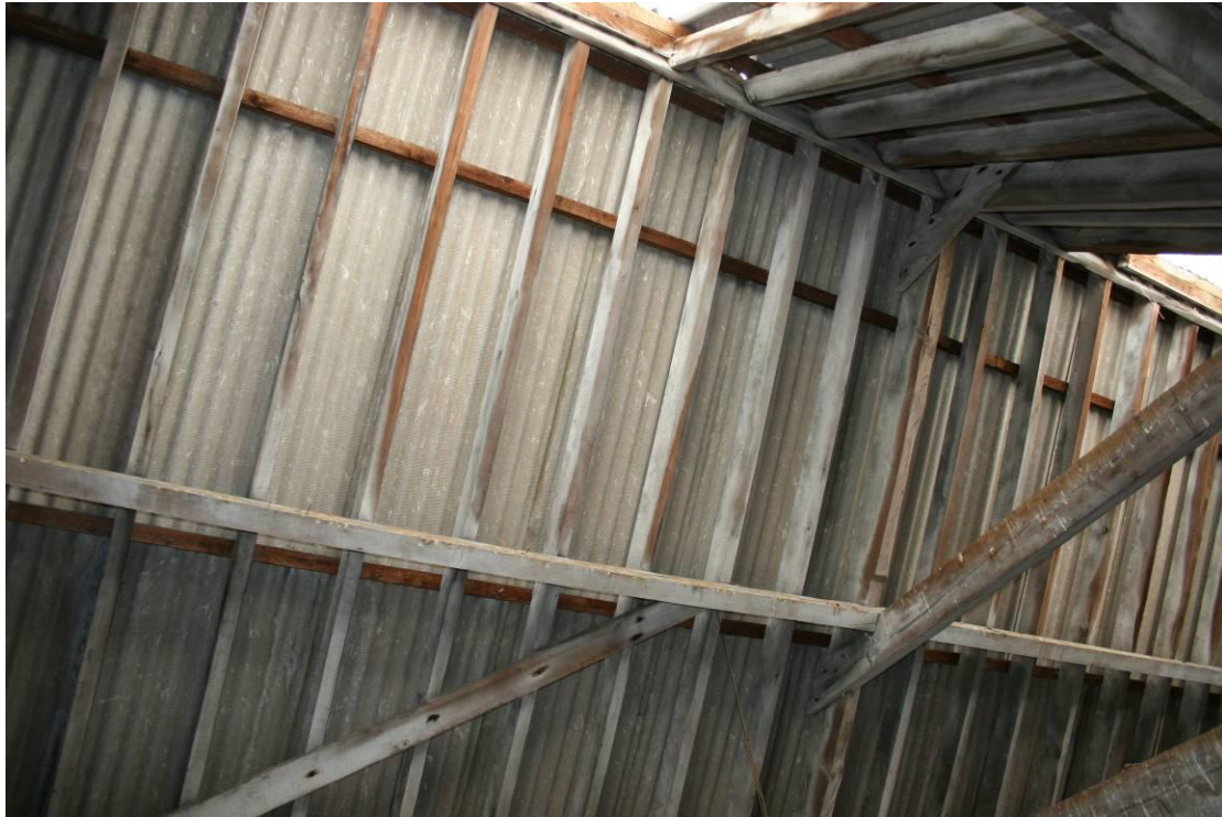
The roof structure looking NW.
