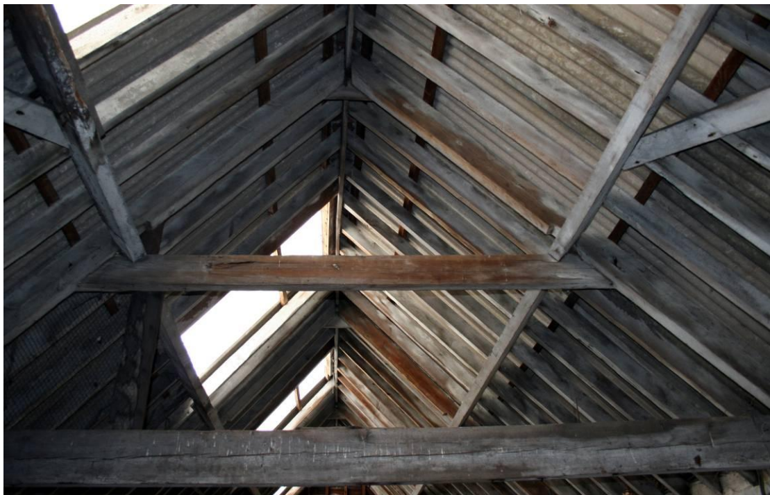
The roof structure looking N.
