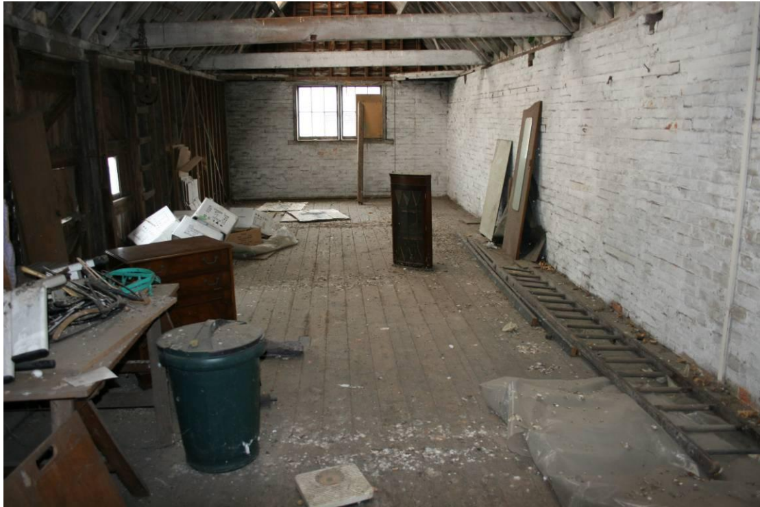
Looking N on the upper floor.
