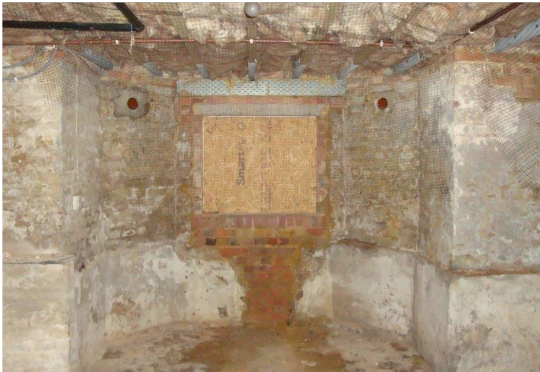
Looking E at the light well
