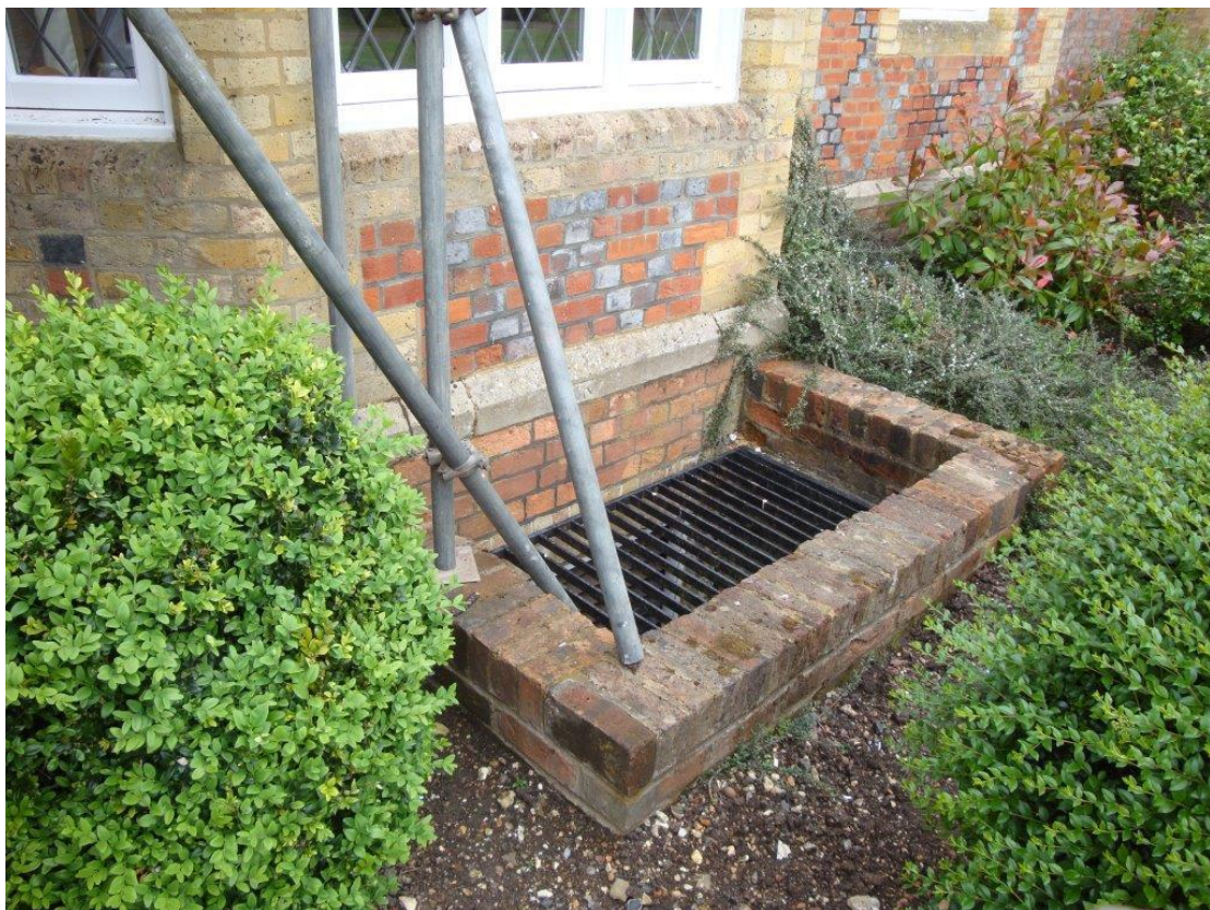
Light well to the north of the doorway.
