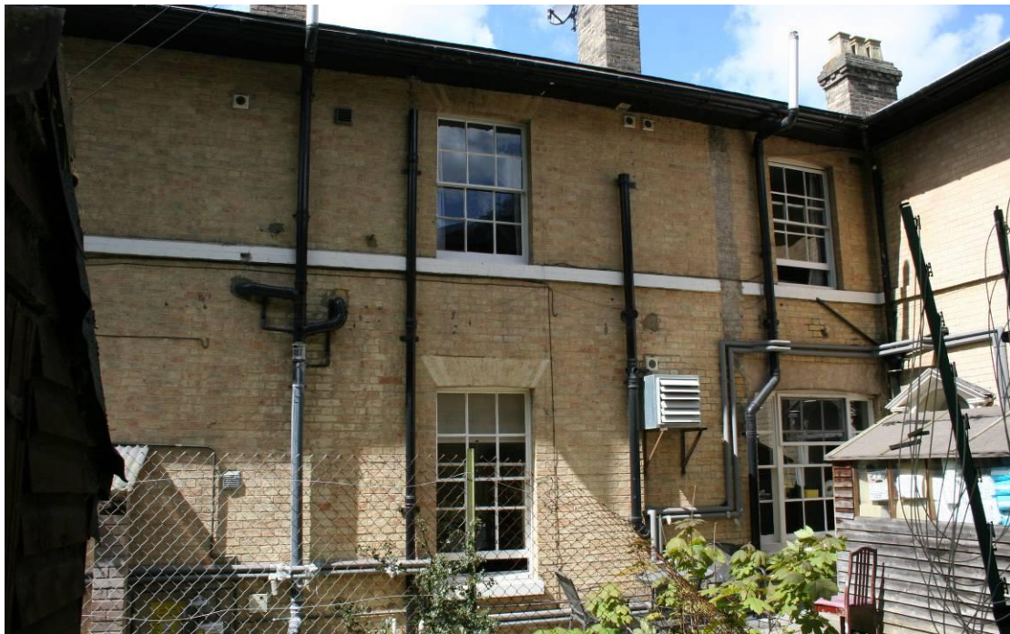
Eastern elevation of the original house
