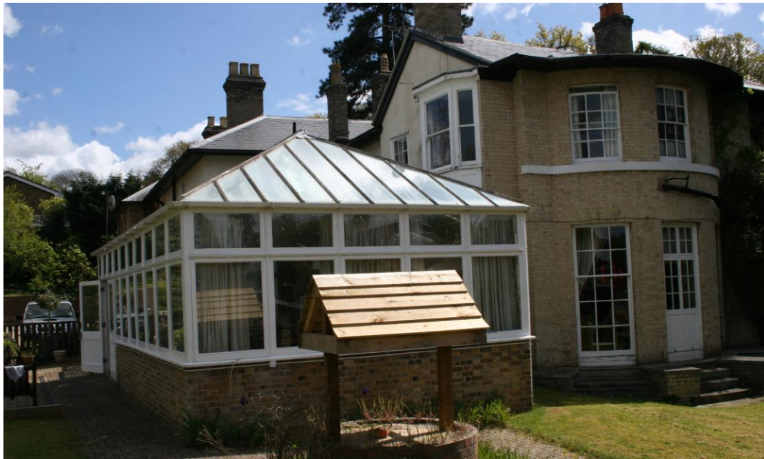
The western elevation of the conservatory.
