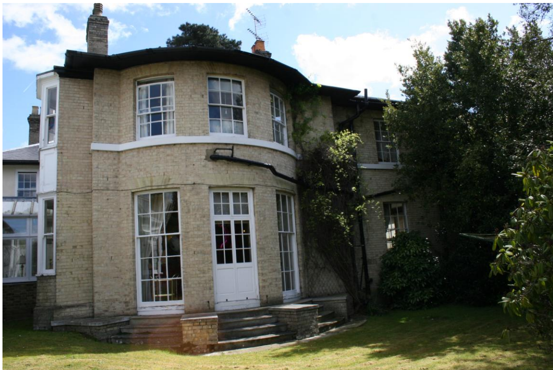
The western elevation of the original house.
