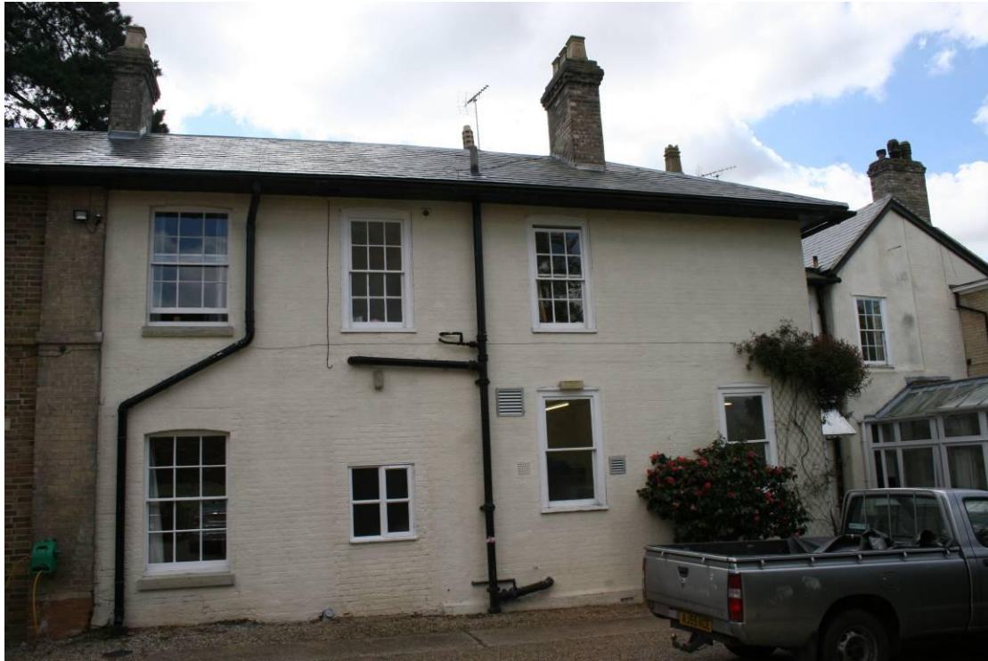
The northern elevation of the Victorian extension.
