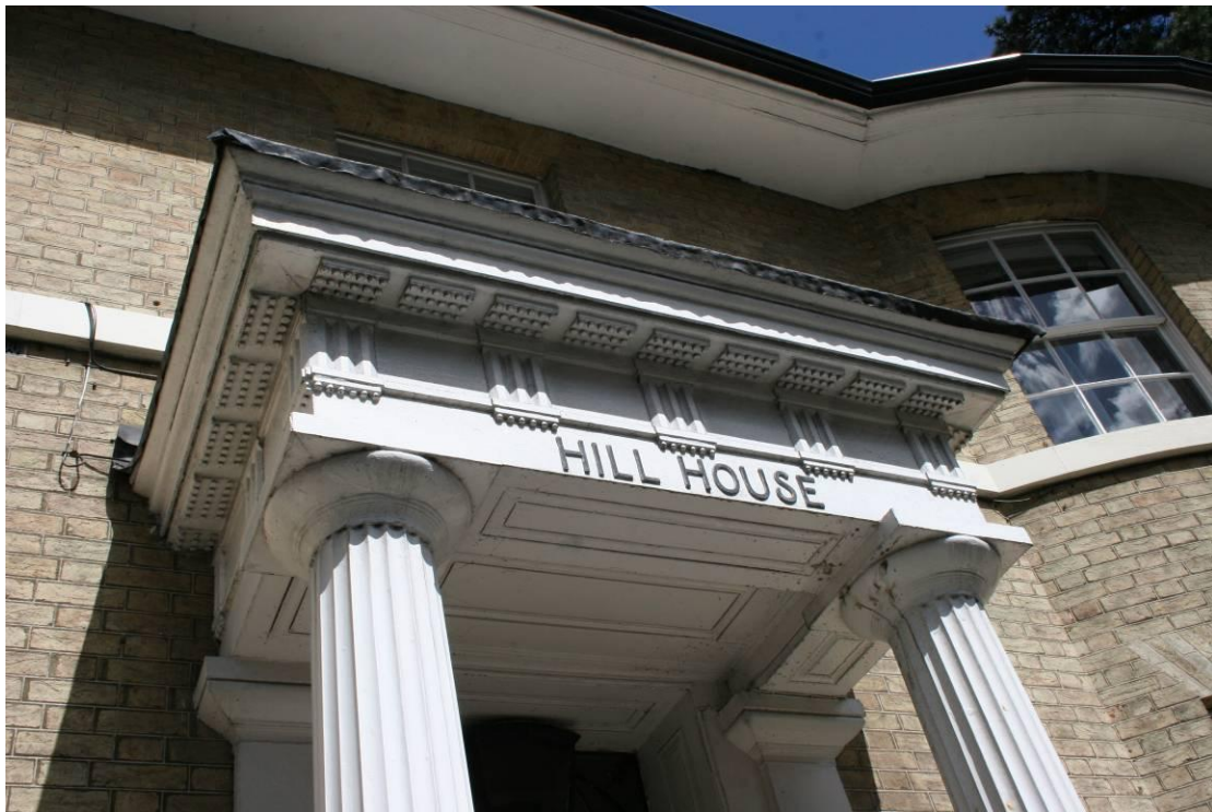
Detail of the porch with Greek detailing.
