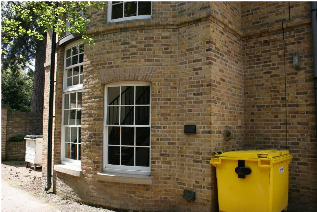
The eastern elevation of the 1988 extension.
