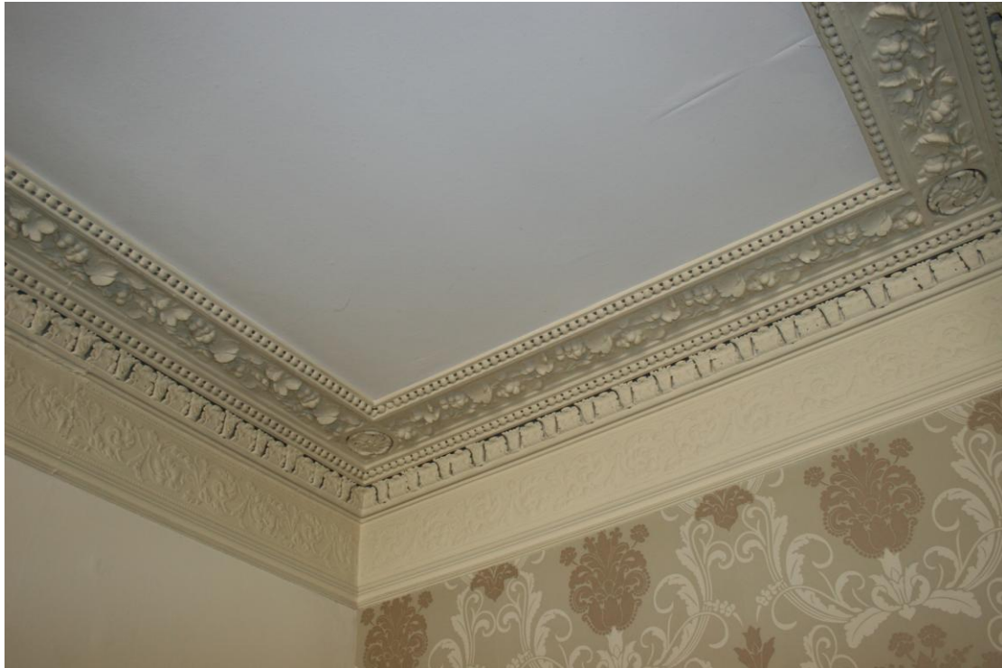
Detail of the plasterwork ceiling.
