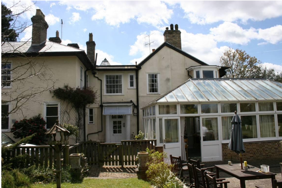
The northern elevation of the original house.
