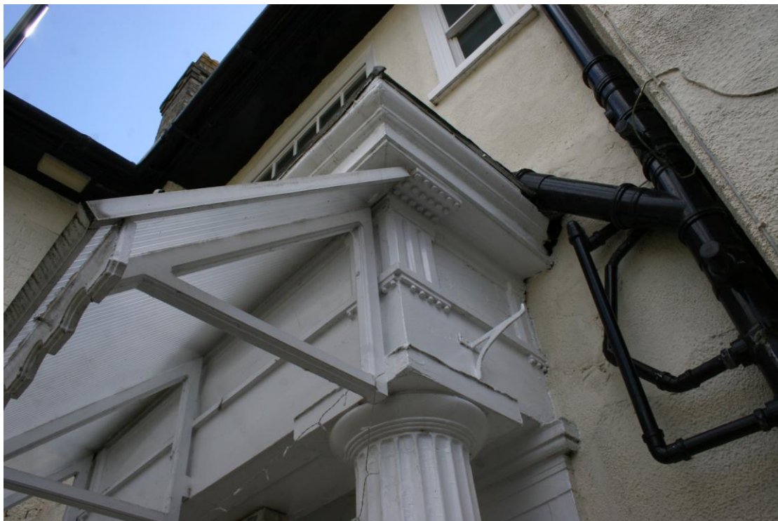
Detail of the rear porch.
