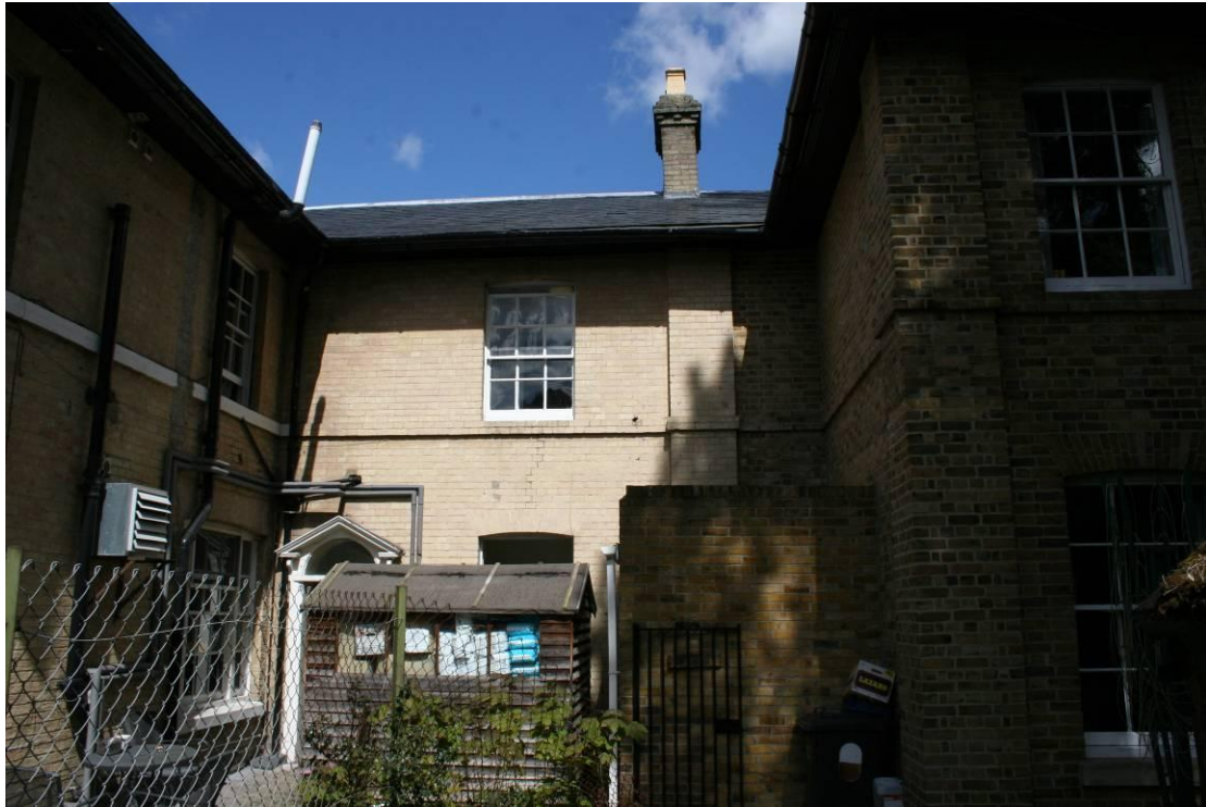
The southern elevation of the Victorian extension.
