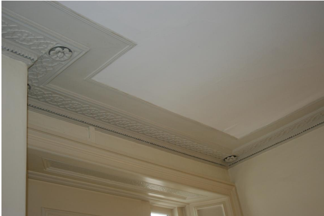
Detail of the ceiling plasterwork.
