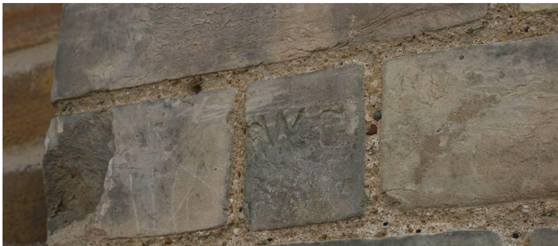
Detail of the Victorian brick work marked WG.
