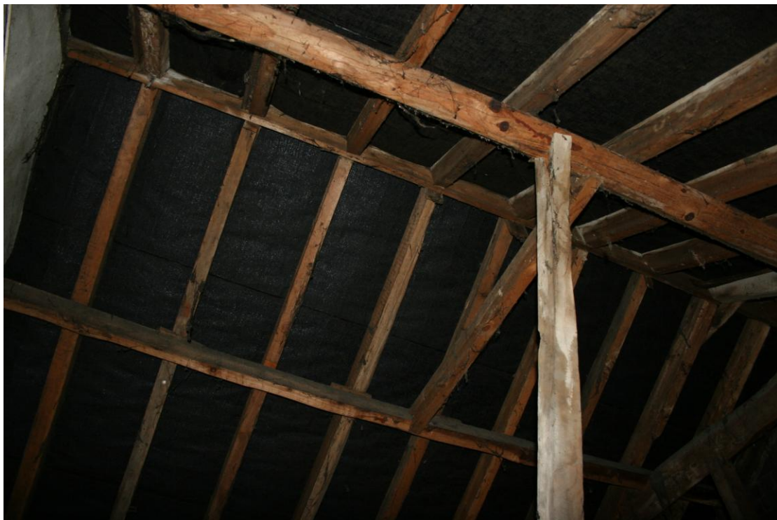
Looking SW in the main front roof.
