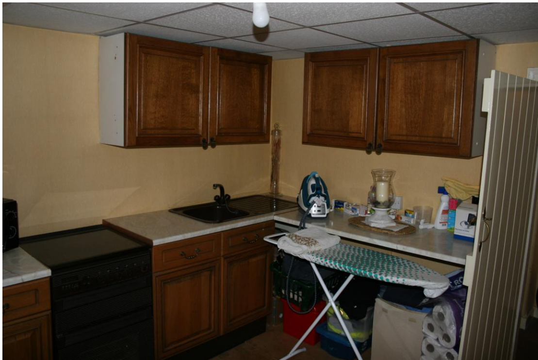
The upstairs Kitchen looking NW.
