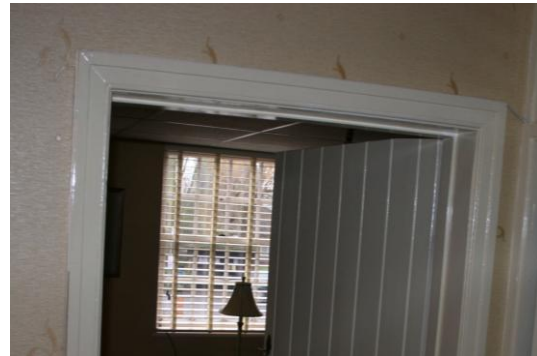
Inserted rooms have plain modern architraves while the originals have beaded doorcases.
