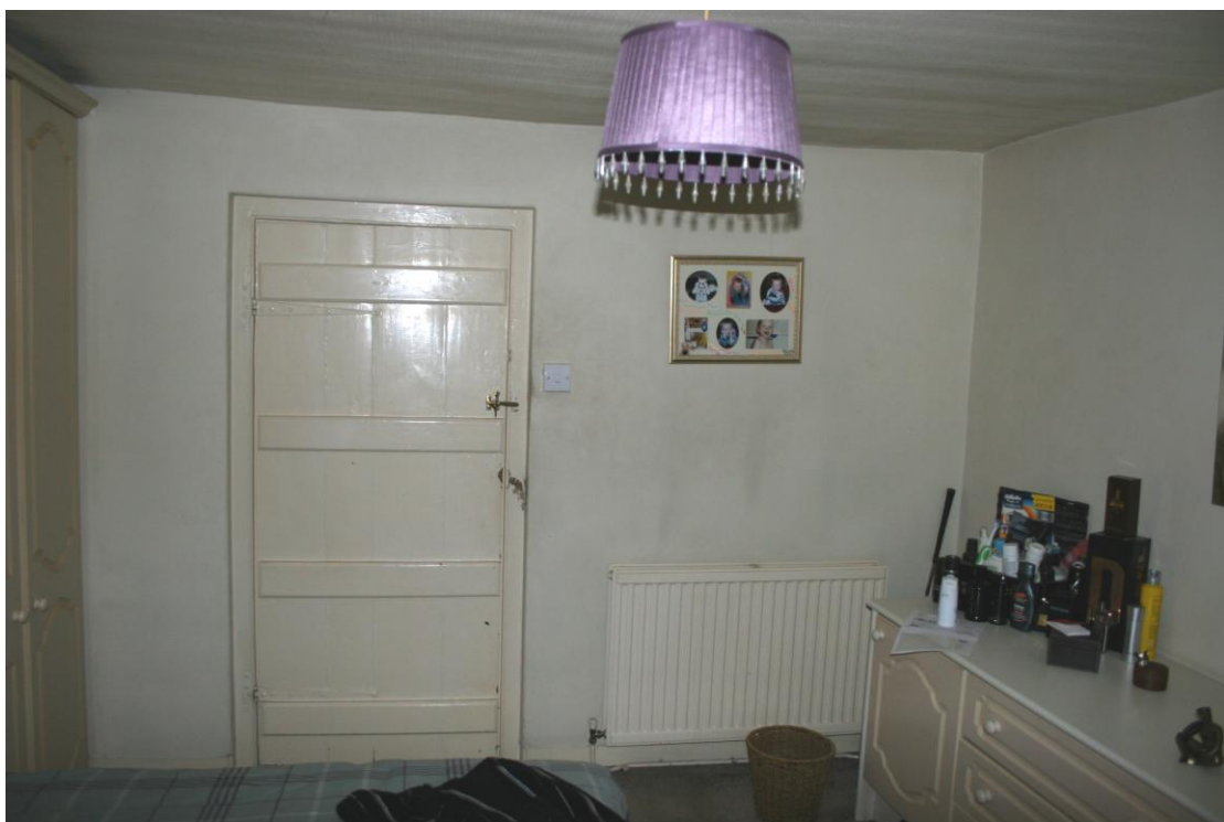
The EC19th boarded door in Bedroom 2. Looking S.
