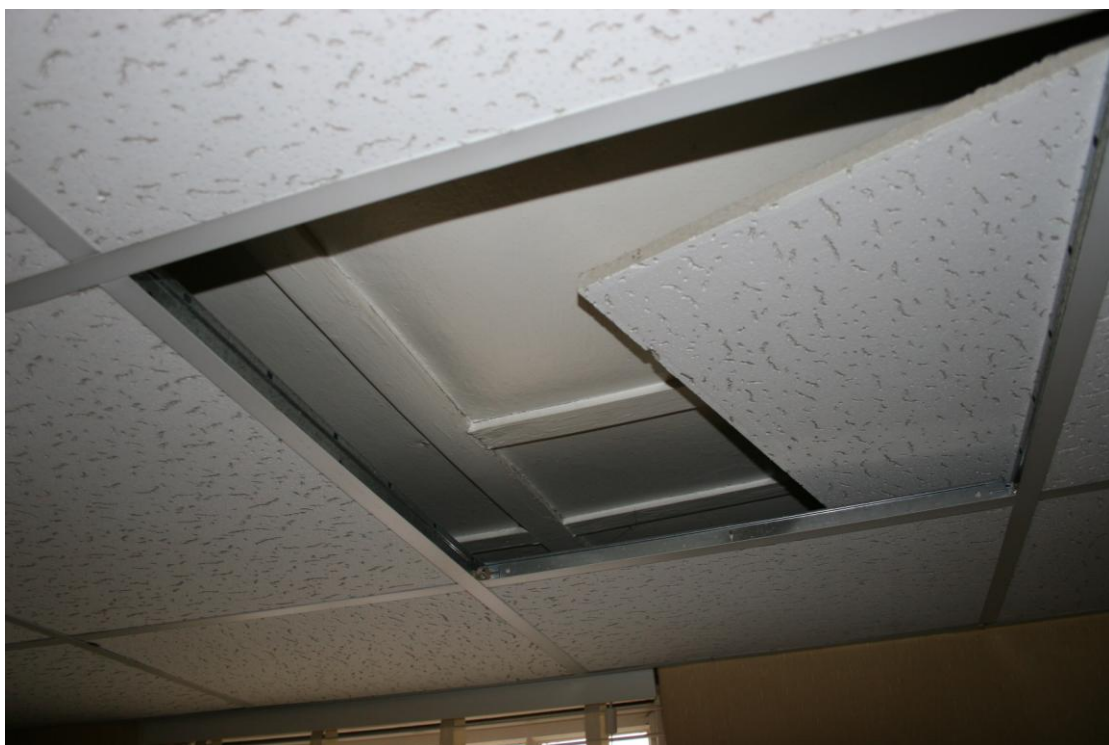
The suspended ceiling in the Kitchen hides a MC20th panelled ceiling.
