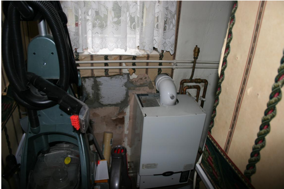
The Boiler Room looking W.
