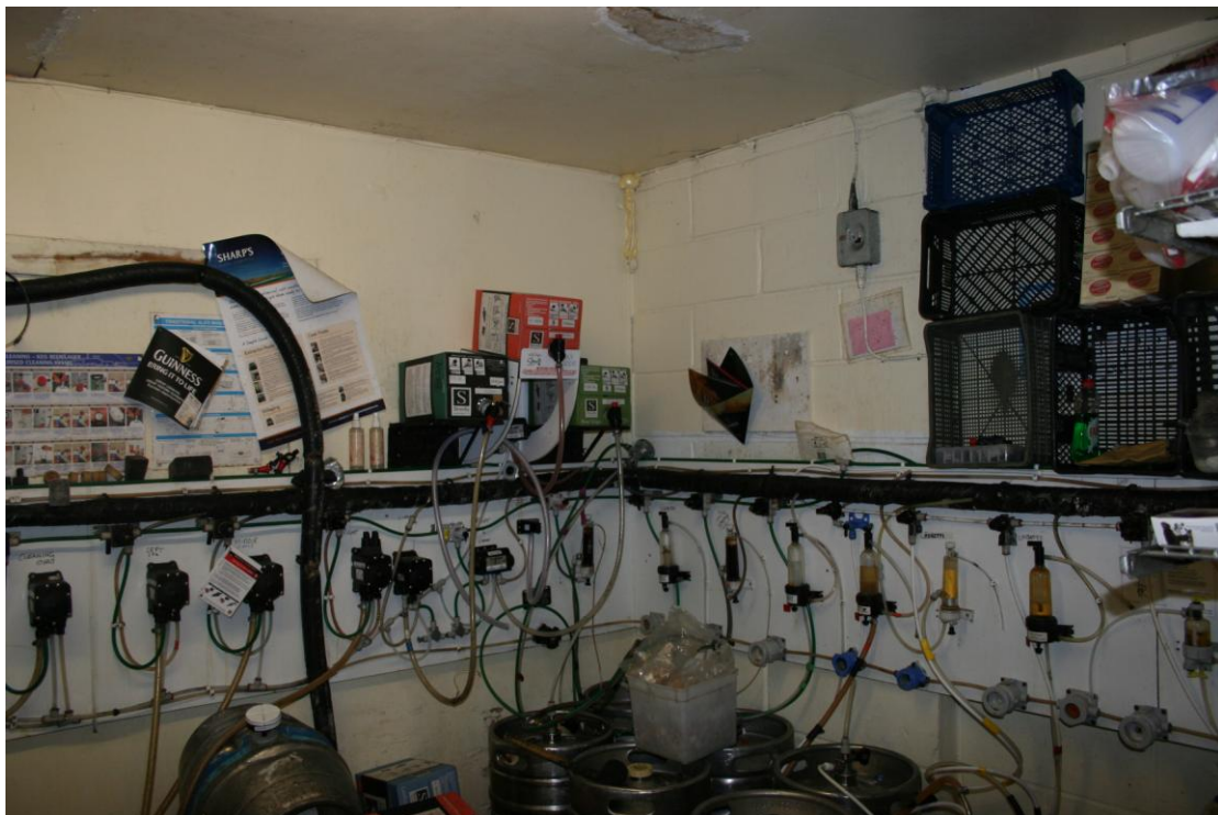
The South Store room contains the beer barrels. The wall of the House has been rendered.
