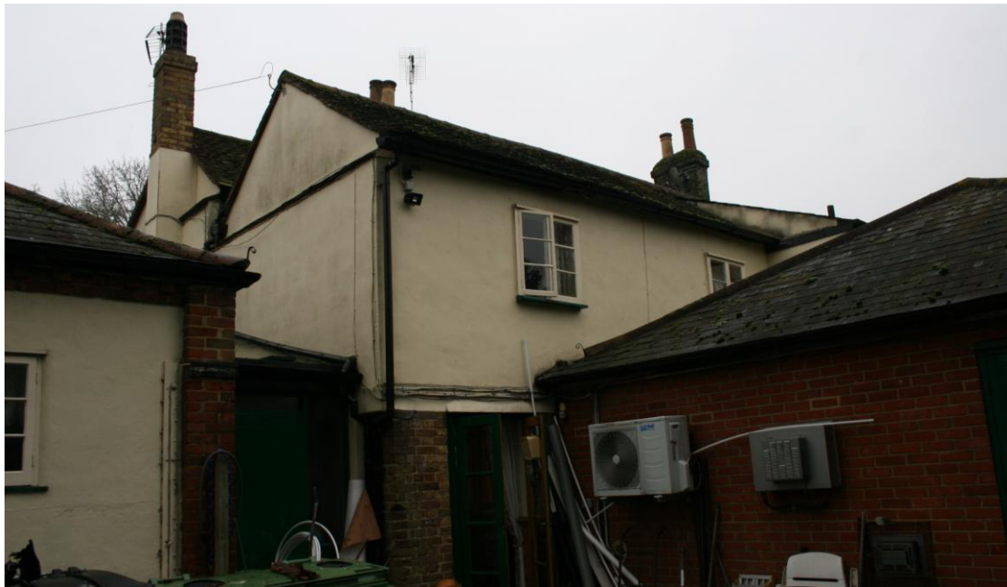
The eastern side of the rear of the House.
