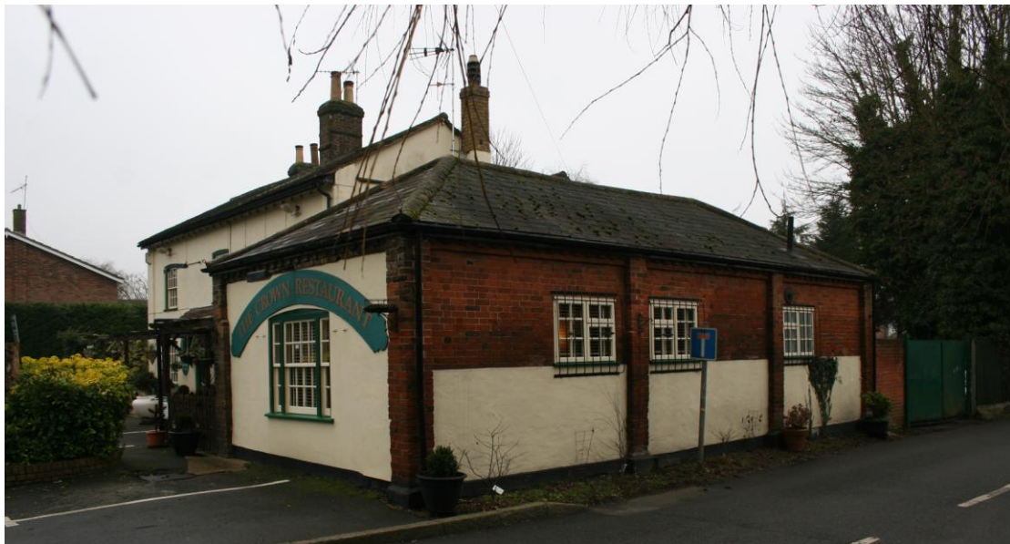
The former Stables seen from the SE.
