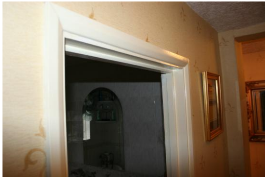
Inserted rooms have plain modern architraves while the originals have beaded doorcases.
