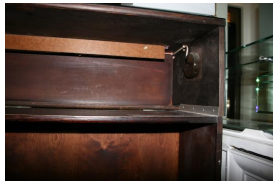
Plywood construction with hardboard and aluminium components.
