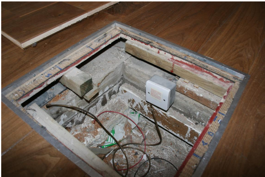
Inspection cover removed in the floor of the Front Room.
