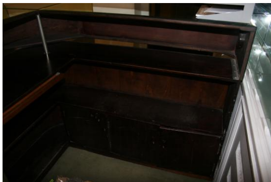
Plywood construction with hardboard and aluminium components.
