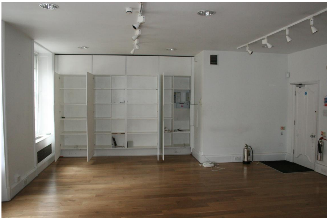
Looking W in the Front Room. The built out section houses the lift, pipes and ducting.
