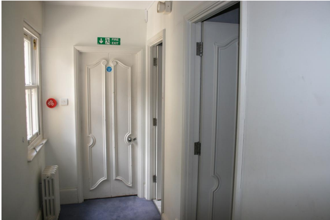
WC cubicles on the Landing near the fire escape. Looking N.
