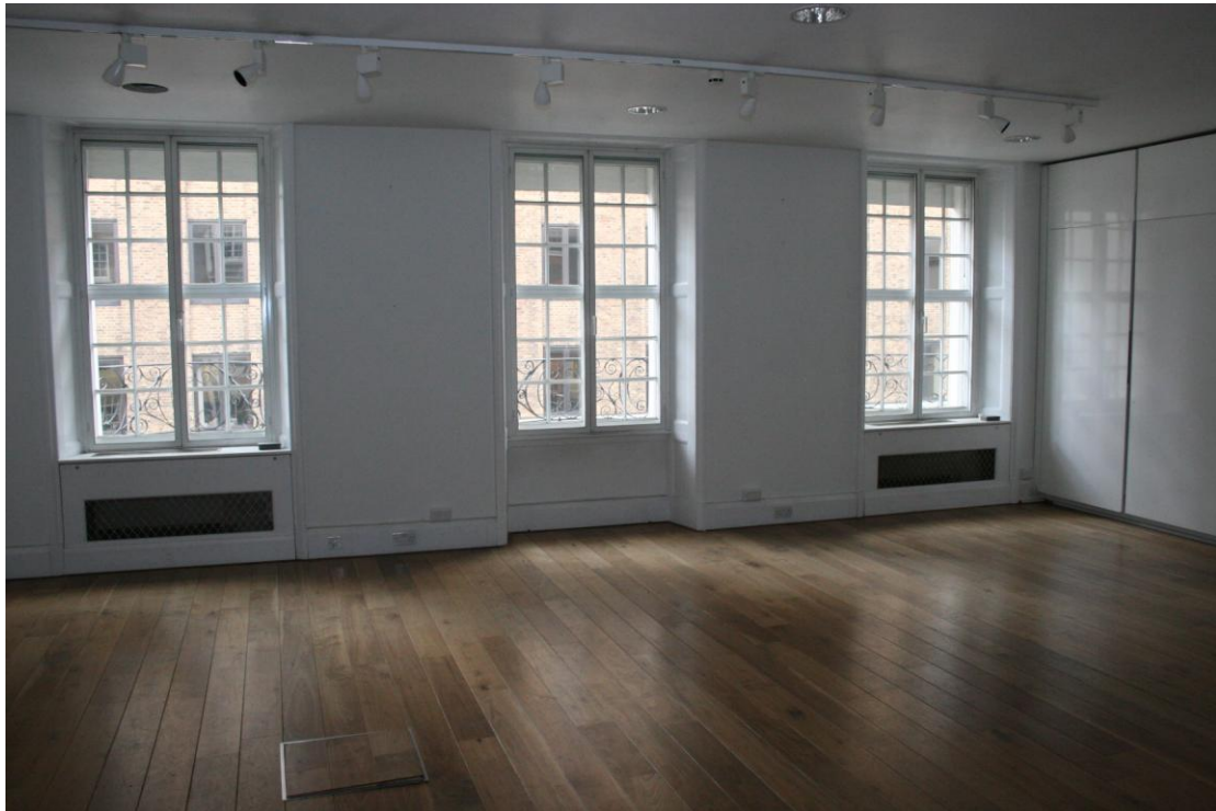
Looking S towards the front of the building. Note inspection cover in the floor.
