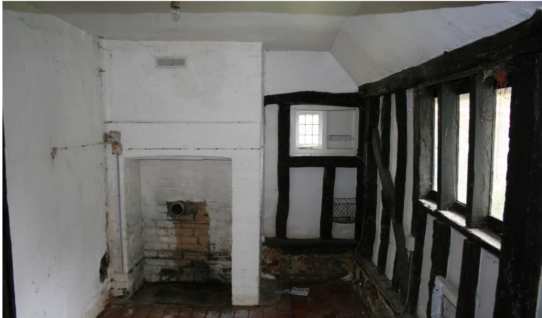
Looking N in the Hallway.
