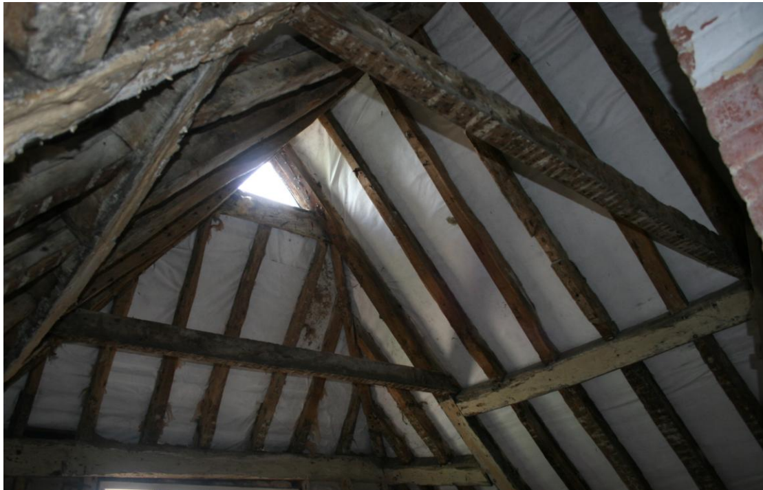
The roof structure of the Eastern Attic Room looking SE.
