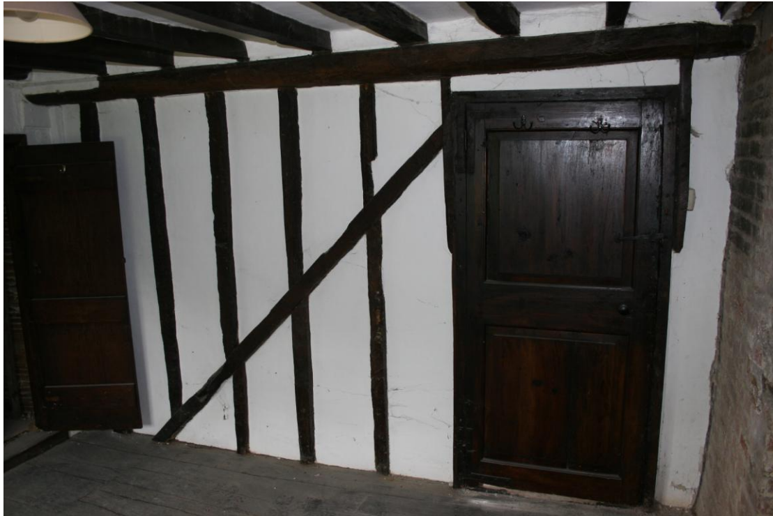
The dividing partition of the eastern side of the building.
