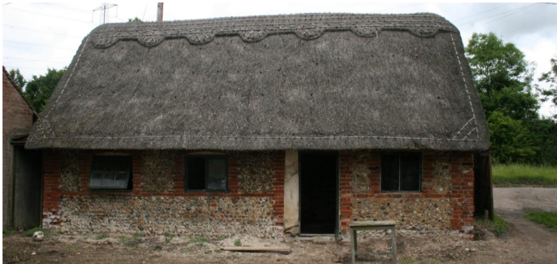
Southern elevation with new thatched roof.
