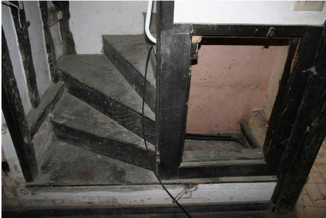
The base of the winder stair in the stair tower.
