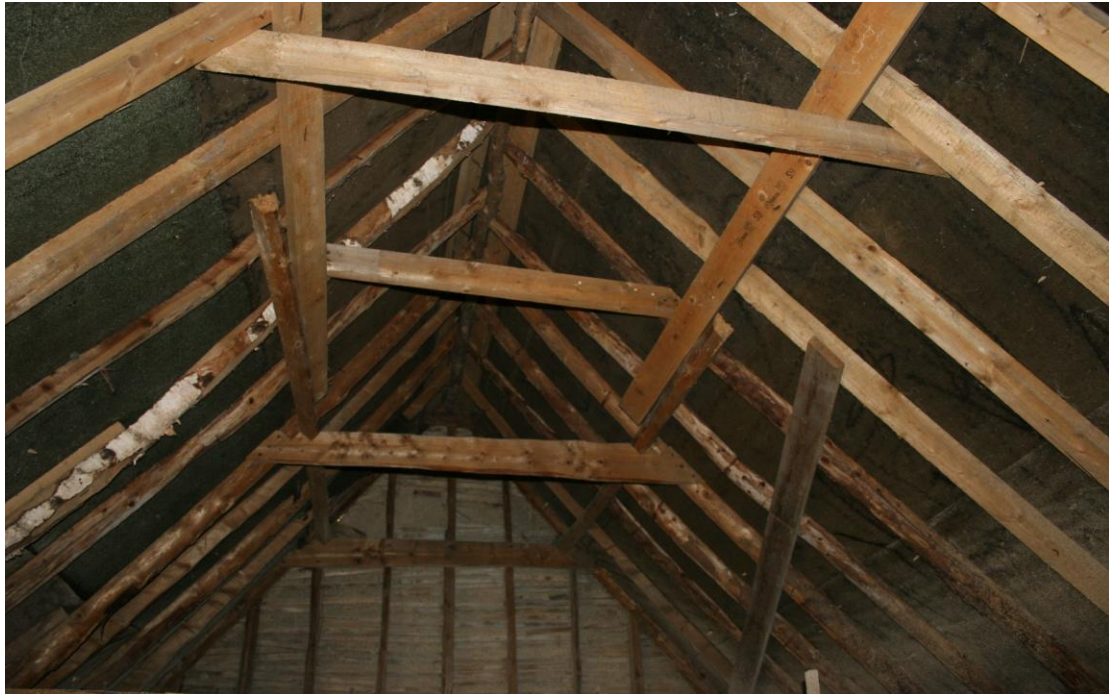
Looking W in the Stables.
