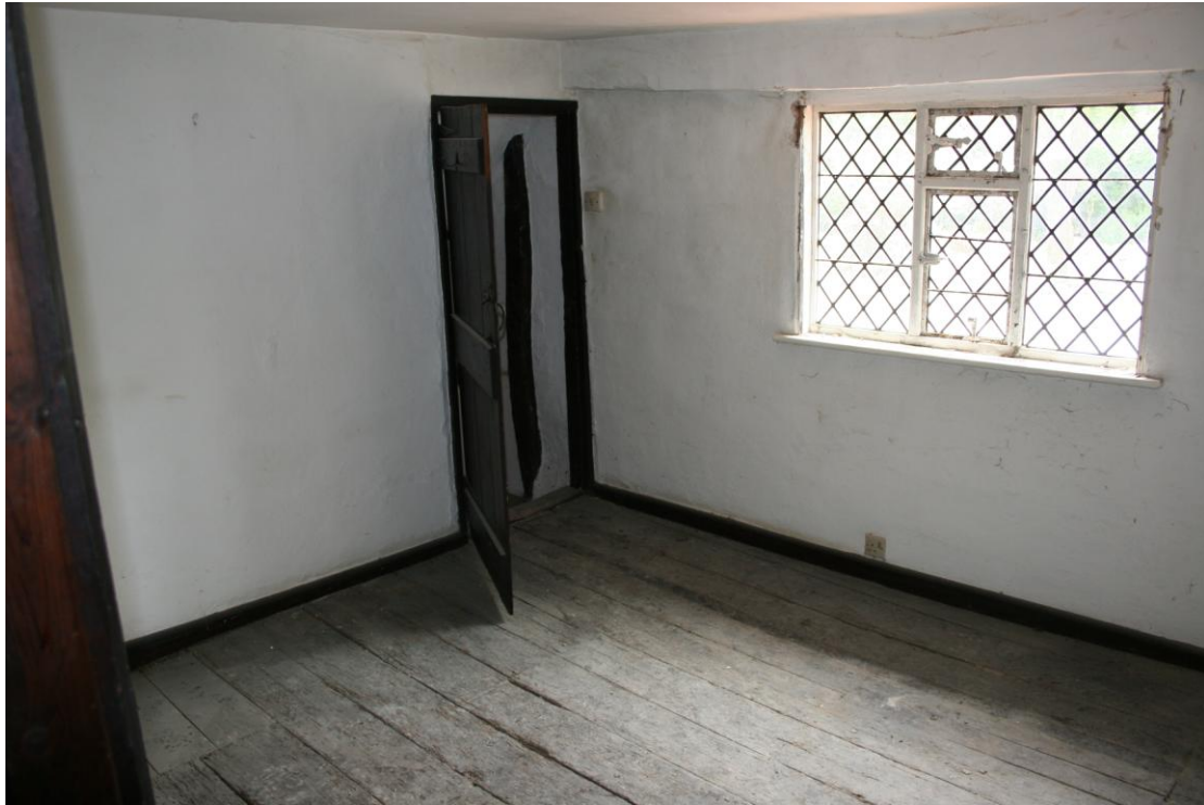
Looking SE towards the Hallway stairs in the SE Bedroom.
