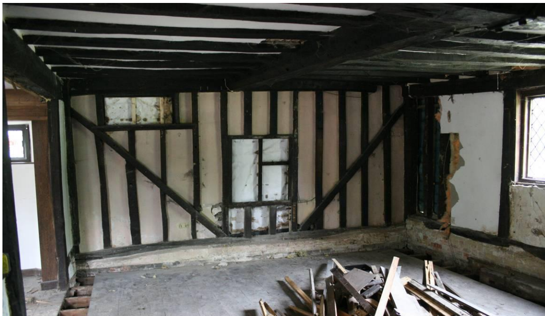
Looking W in the Sitting Room.
