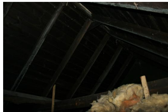
Fire damaged roof structure.
