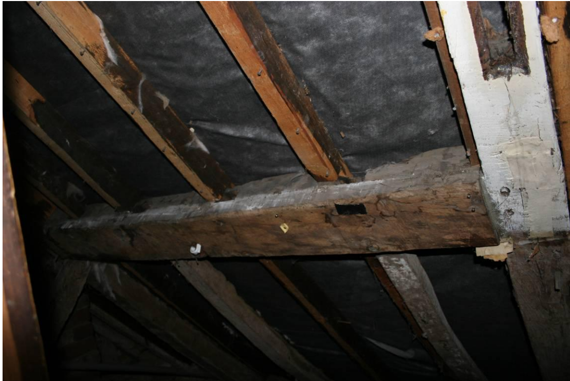
The roof above the Hallway
