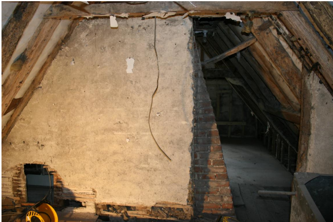
The room has been blanked off from the firestack. Looking E.
