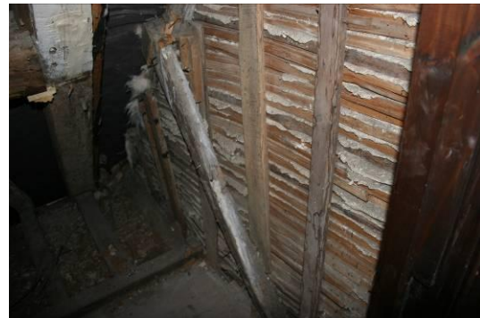
Looking SE at the stairwell wall.
