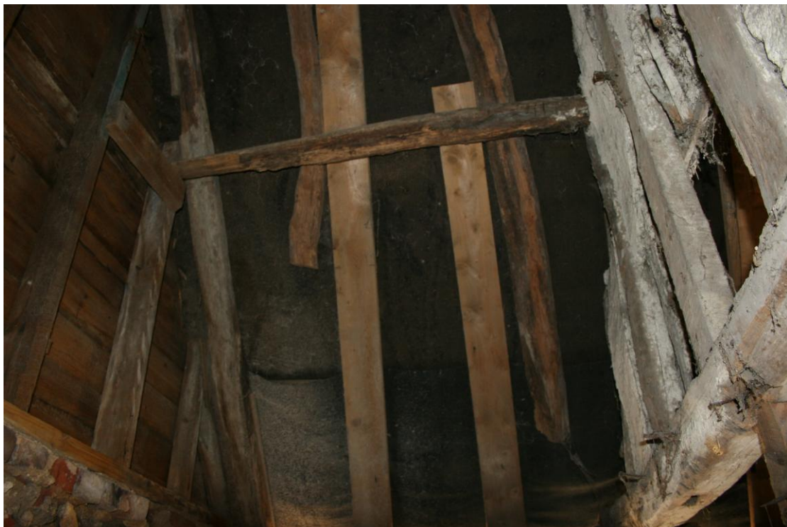
Change in the roof structure in the end bay. Looking S.
