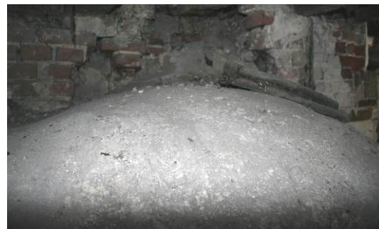
Daubed exterior of the domed oven.
