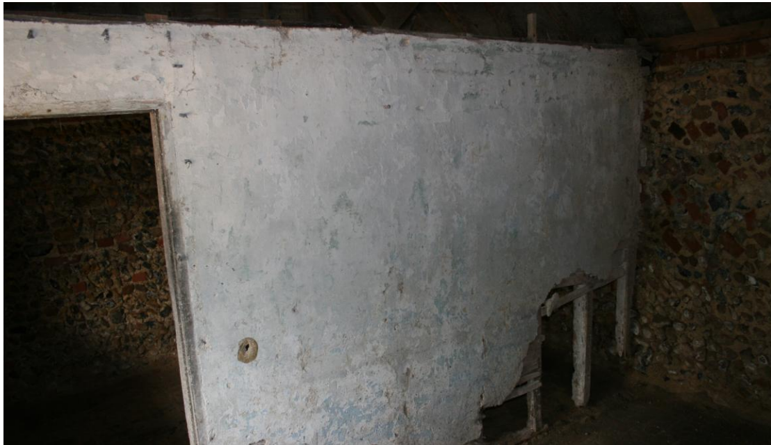
Lath and plastered partition wall between Bays 1 and 2.
