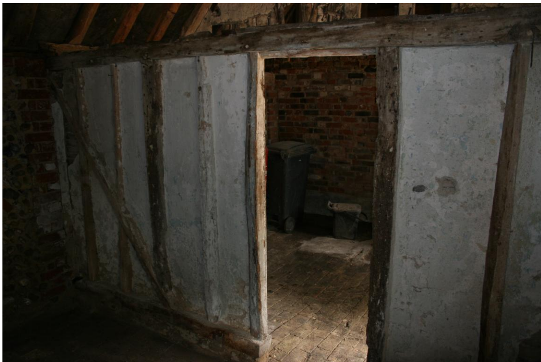
Lath and plastered partition wall between Bays 2 and 3.
