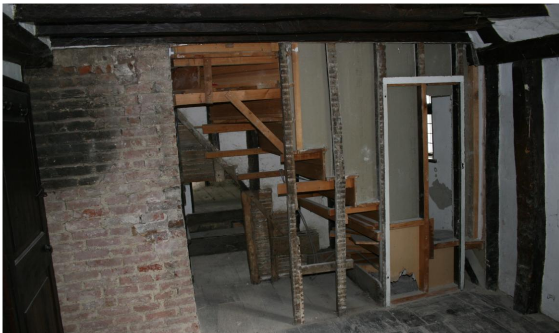
Looking W in the NE Bedroom.
