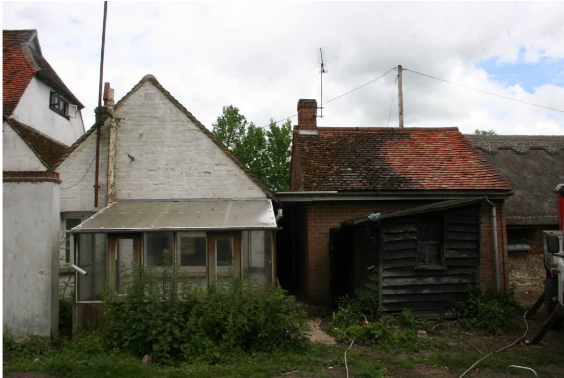
The southern elevation of the MC20th additions.
