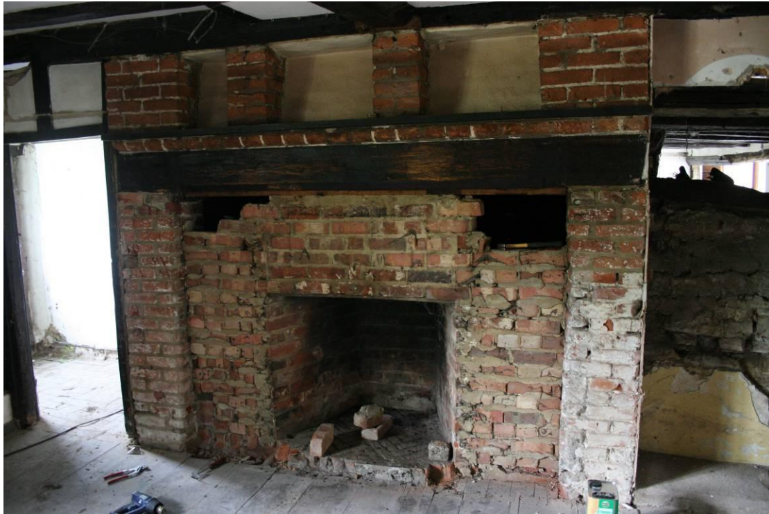
Detail of the fireplace in the Sitting Room.
