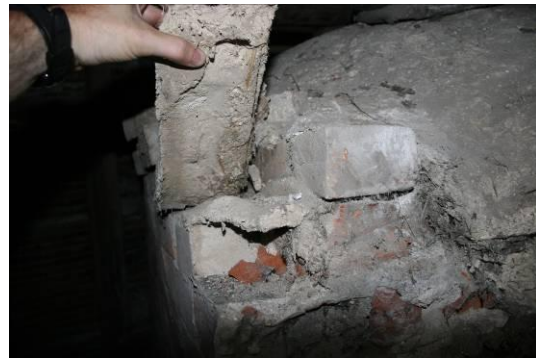
Frogged bricks in the bread oven dome.
