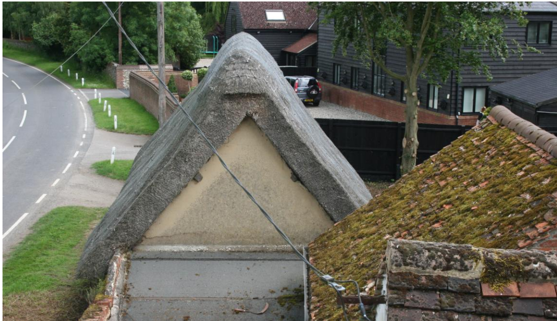
The western elevation seen from the house.
