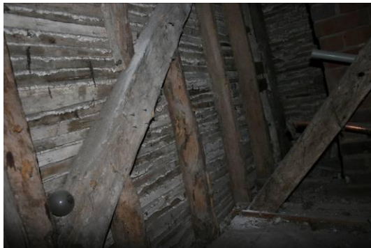
Looking N in the Hallway roof. Main frame.
