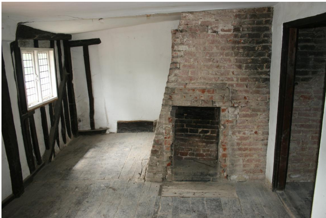
Looking W in the SE Bedroom. Note the inserted C19th fireplace.
