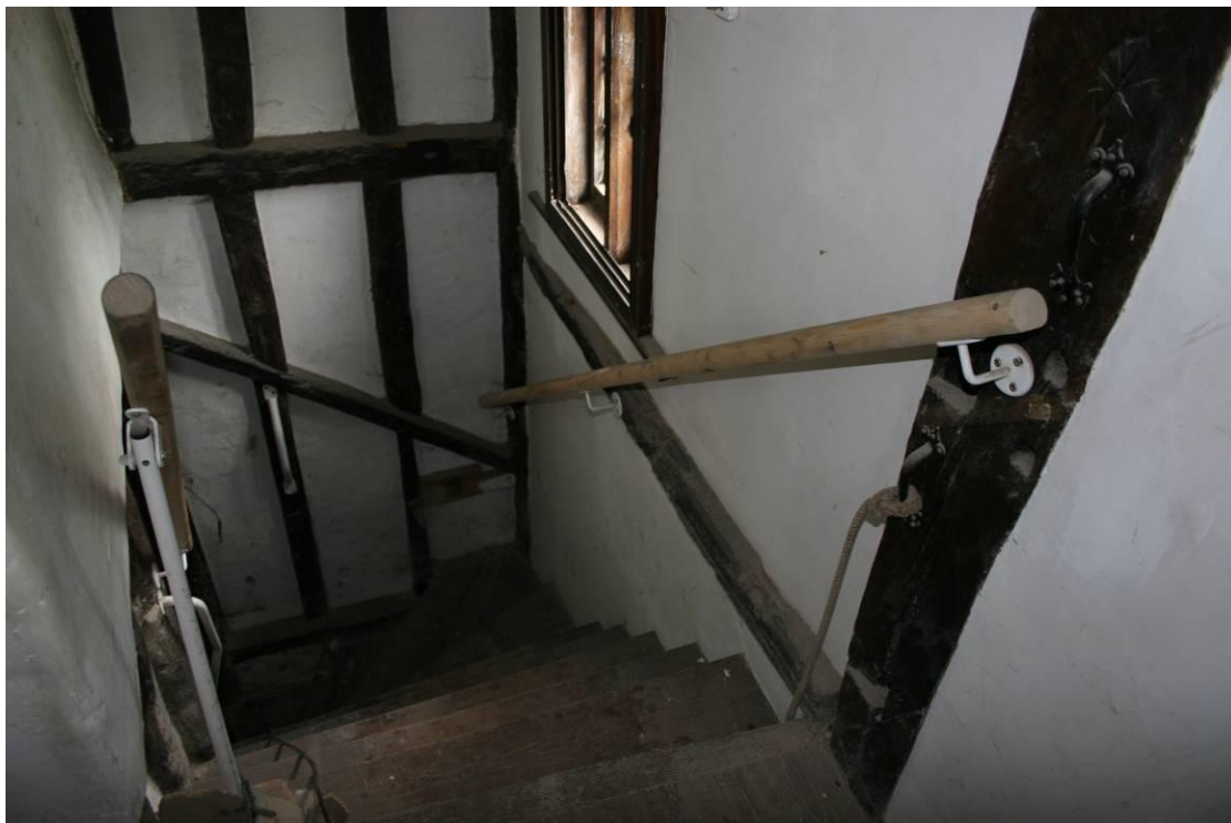
Looking down the stair tower
