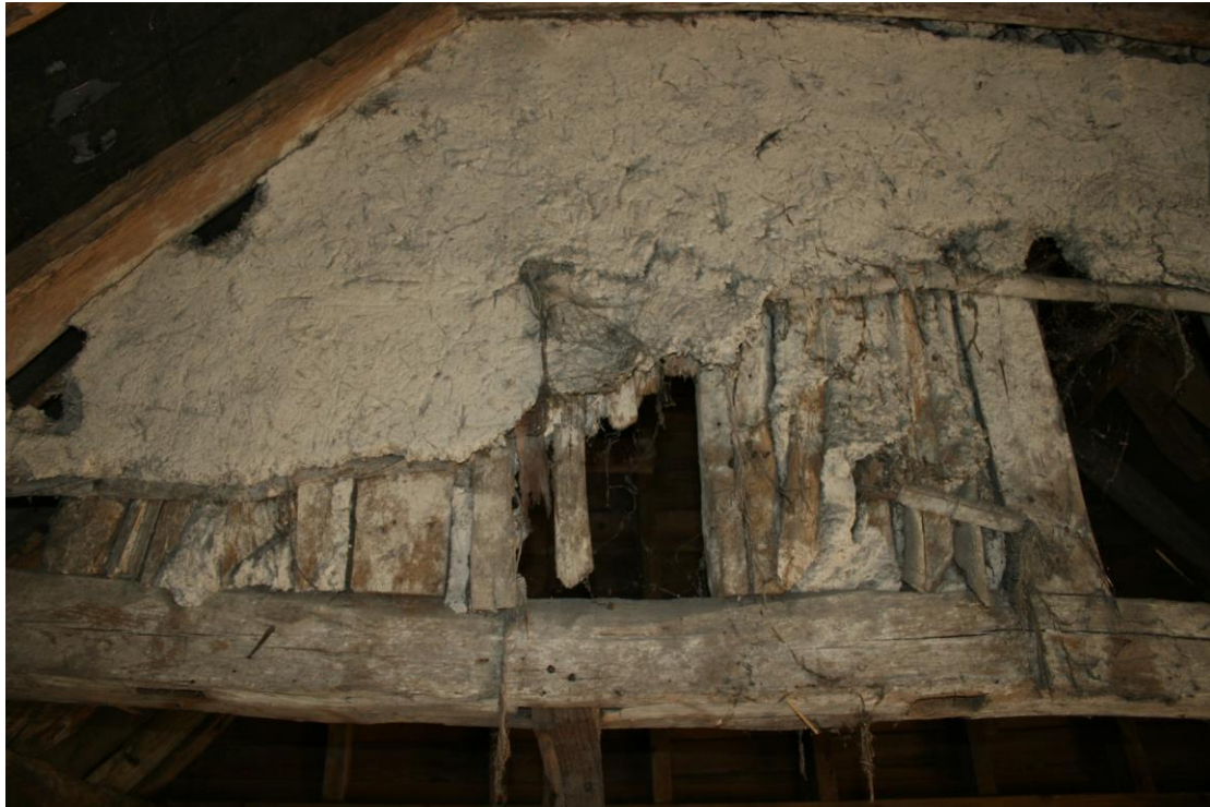
Detail of the wattle and daub panel. West side.
