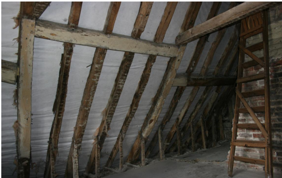
The offset butt purlin roof on the south side of the room.
