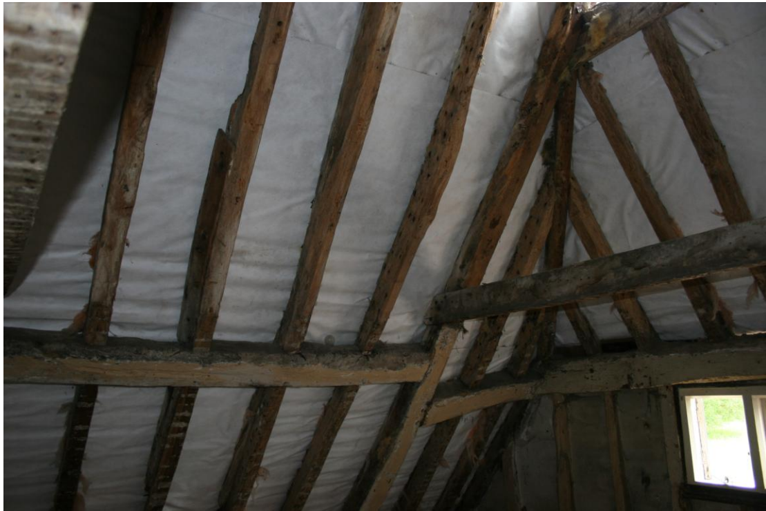
The north side of the butt purlin roof.
