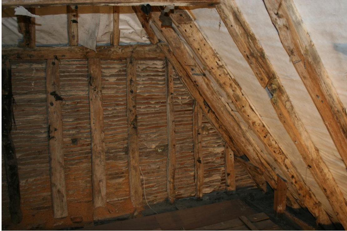
Reused rafters in the roof space. Looking NW.
