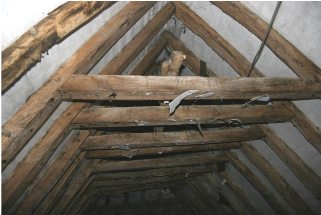
The collars of the paired rafters.
