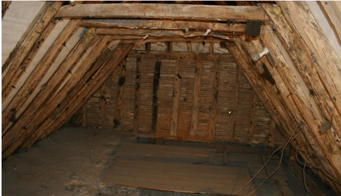
Looking W in the West Attic Room.
